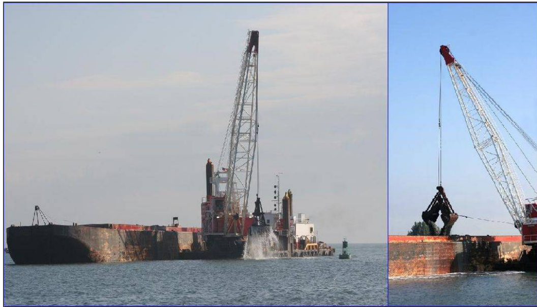
Figure 3. 47: Clamshell Dredging In Progress
