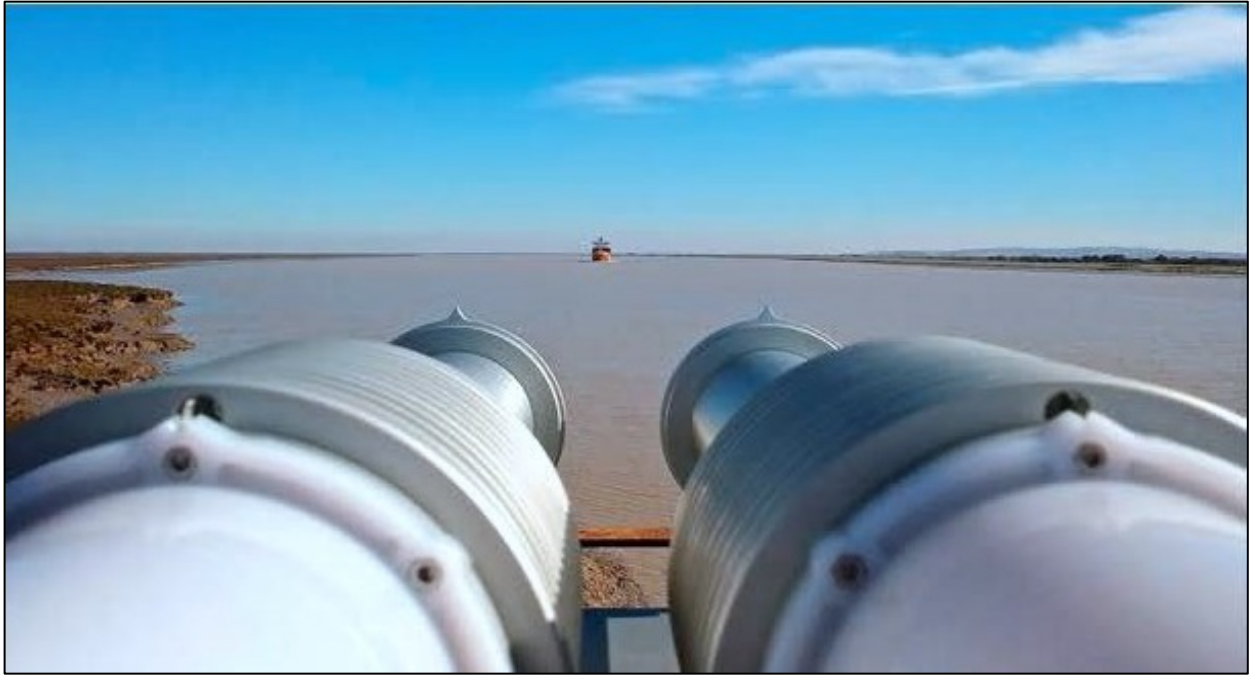
Figure 6. 14: Led Sector Lights Marking The Central Line Of The Channel In A River (Extreme Precision)
