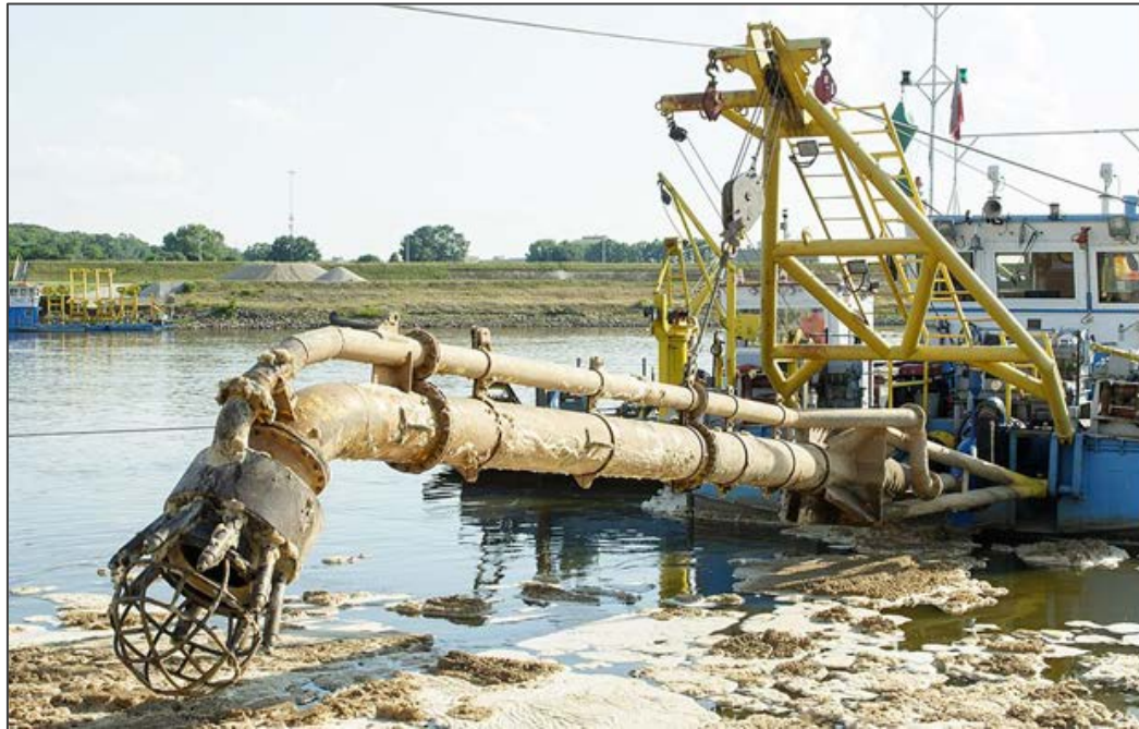
Figure 3. 43: Dredge Drag Head Of A Suction Dredge Barge On A River
