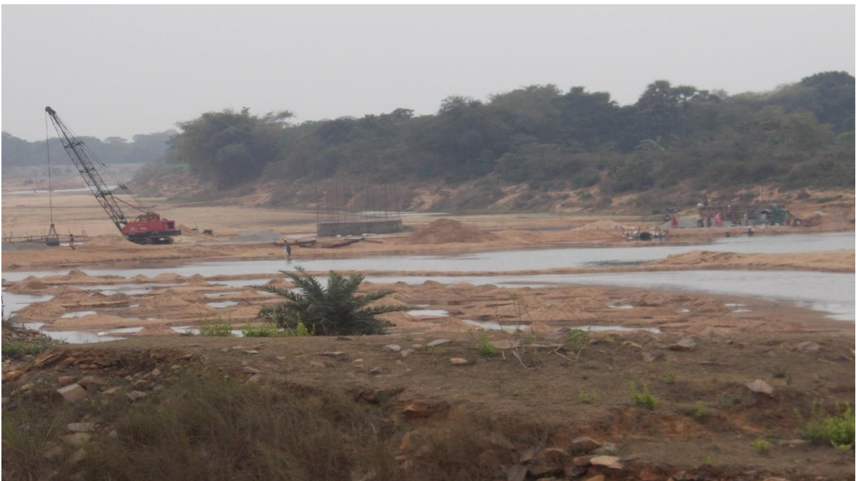
Figure 12: Under construction Dhumuda Bridge(CH:12.6km)
