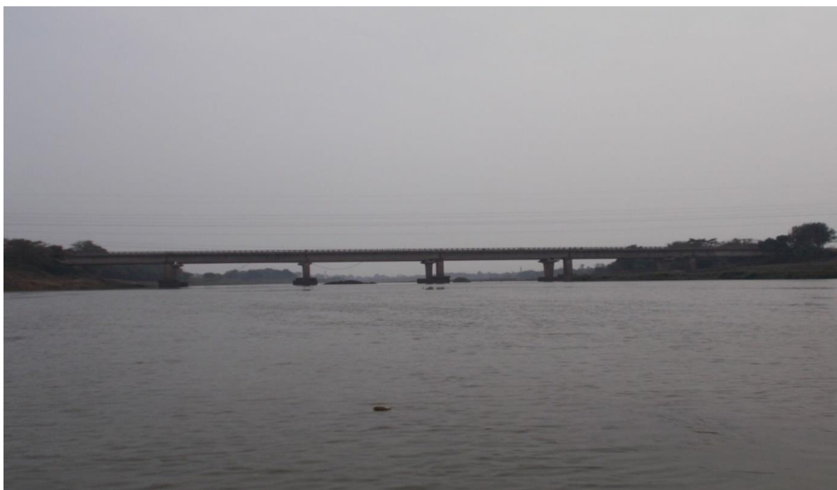
Figure 15: NH5 Bridge (CH:16.5km)
