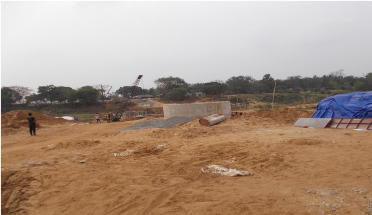
Figure 14: Under construction Palasia Bridge (CH:7.1km)
