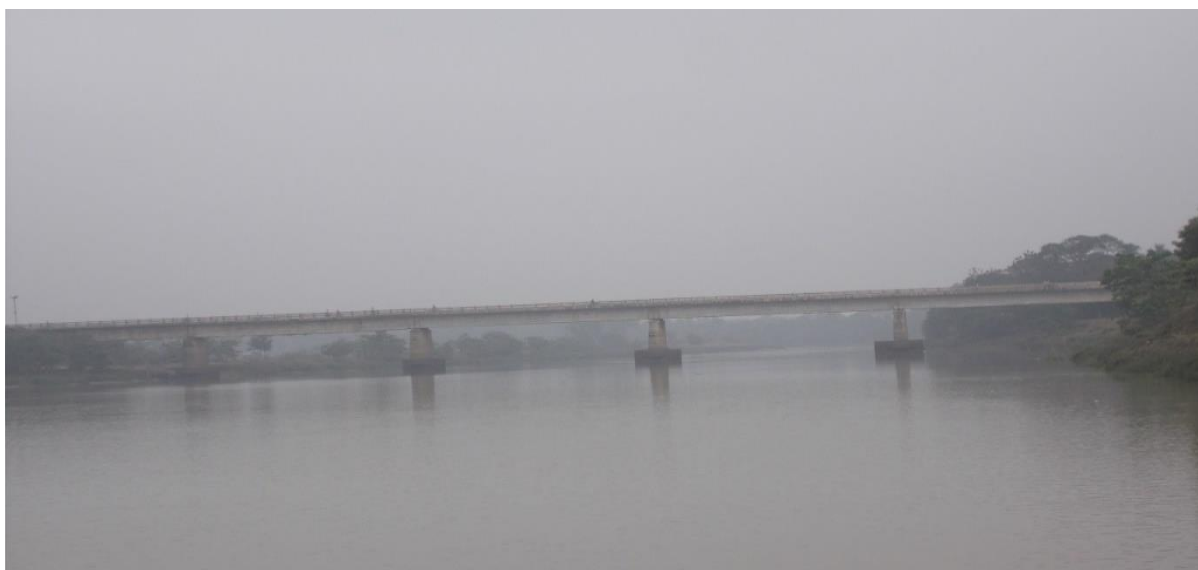
Figure 10: Balighat Bridge(Ch: 32.3km)
