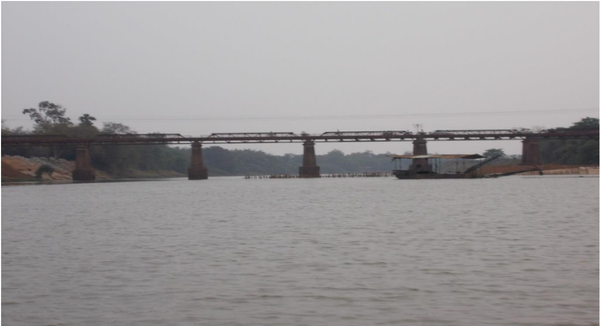
Figure 13: Fuludi Bridge (CH:19.9km)
