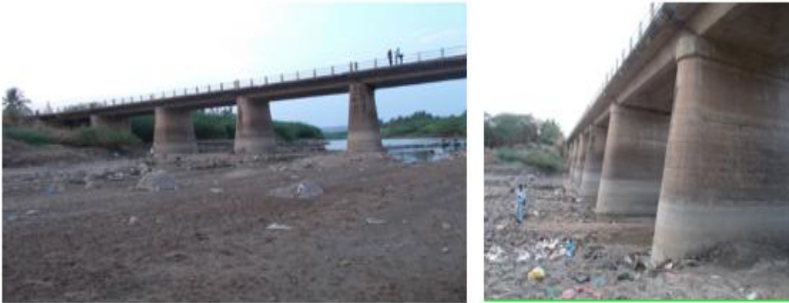
Figure 18 - Cholachagudda Bridge (ch. 80.29km)
