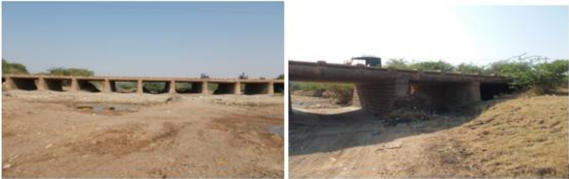
Figure 21 - Jakanuru Bridge (ch. 93.22km)
