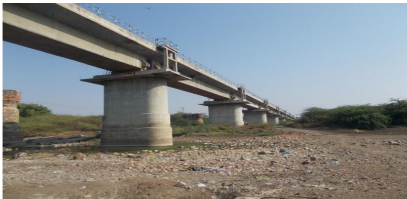
Figure 22 - Jakanuru Railway Bridge (ch. 93.59km)
