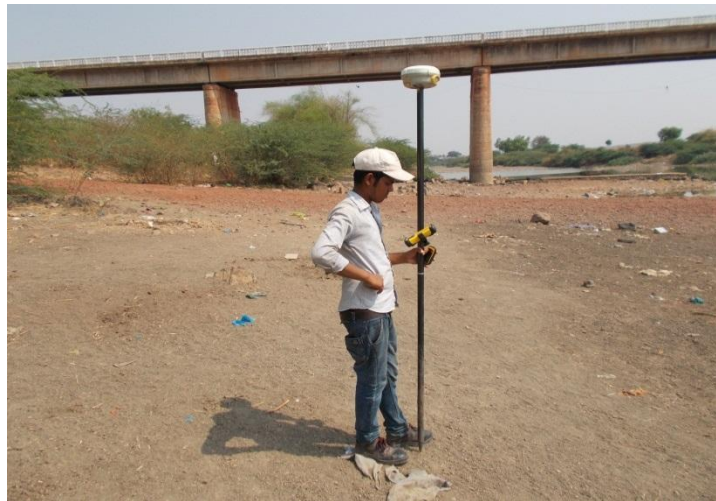
Figure 12 - Kamatagi Bridge (ch. 35.43km)
