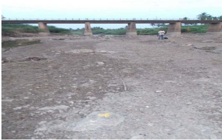
Figure 17 - Mangalur Bridge (ch. 72.90km)
