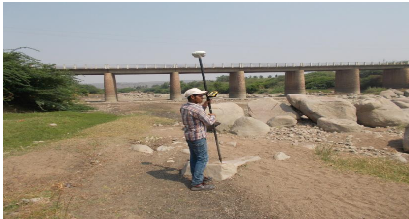
Figure 16 - Patadkal Bridge (ch. 61.78km)
