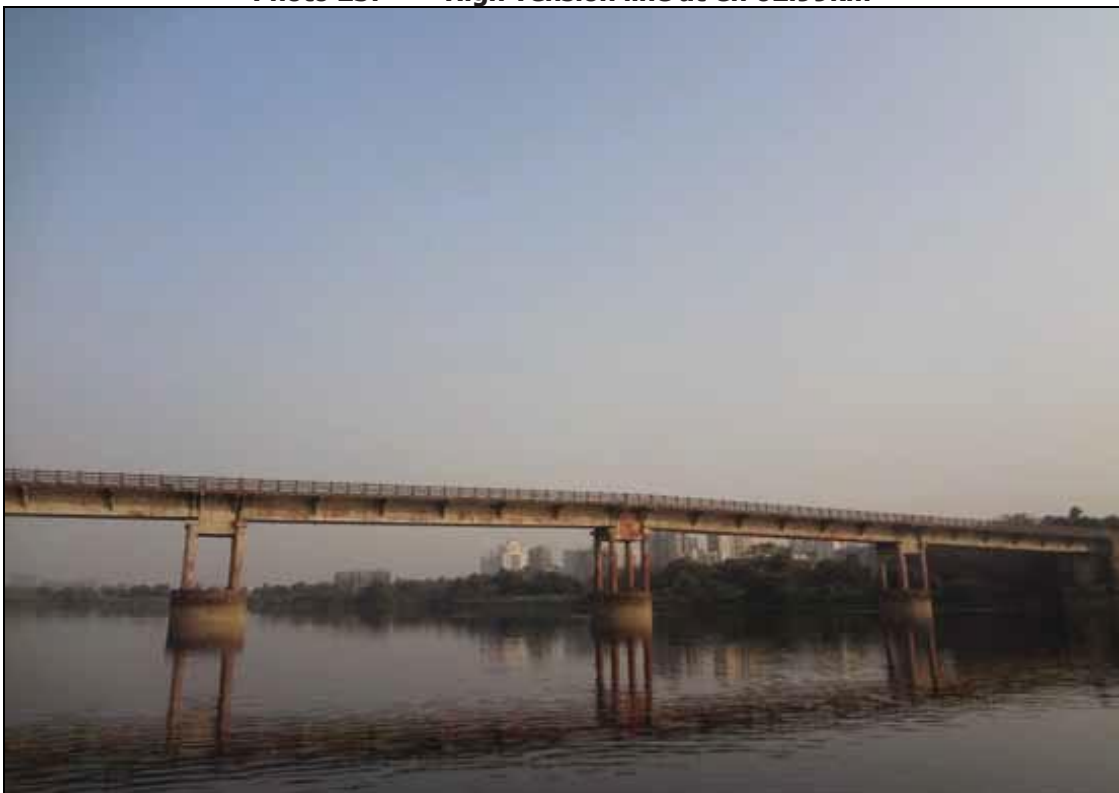
Photo 26: Kalyan Sape bridge at Ch 64.52km
