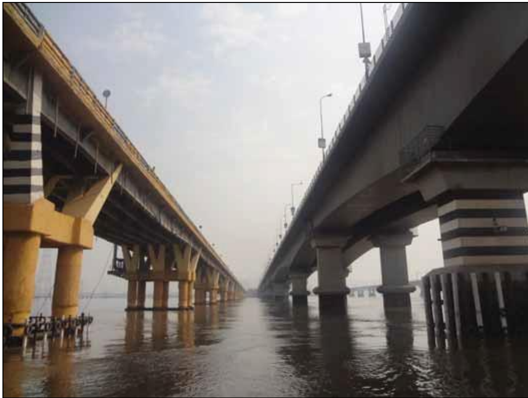
Photo 5: Vashi road bridge at Ch 19.56km
