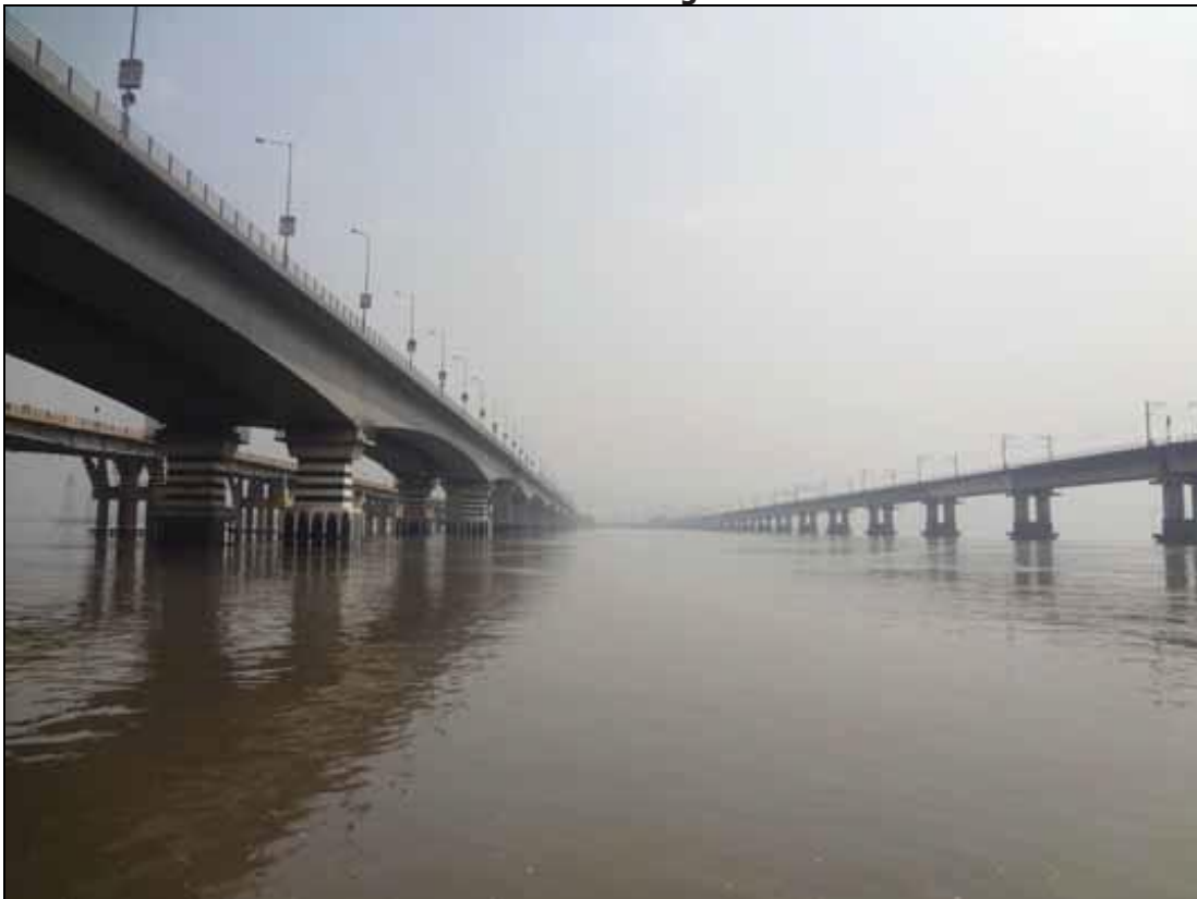
Photo 4: Vashi Road bridge at Ch 19.52km
