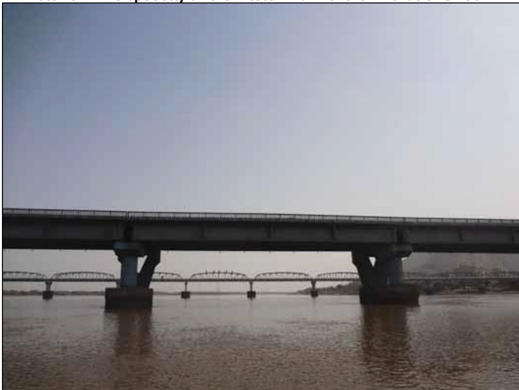
Photo 16: Nasik Expressway pipe Line Bridge at Ch 40.19km
