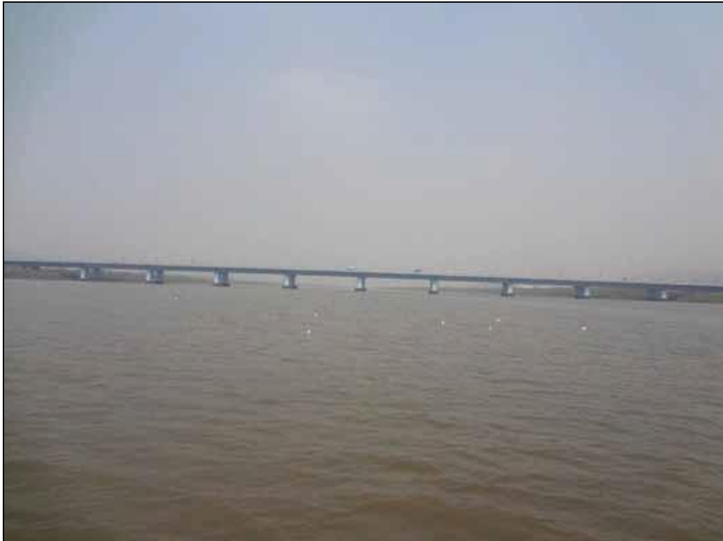
Photo 7: Airoli Road Bridge at Ch 30.00km
