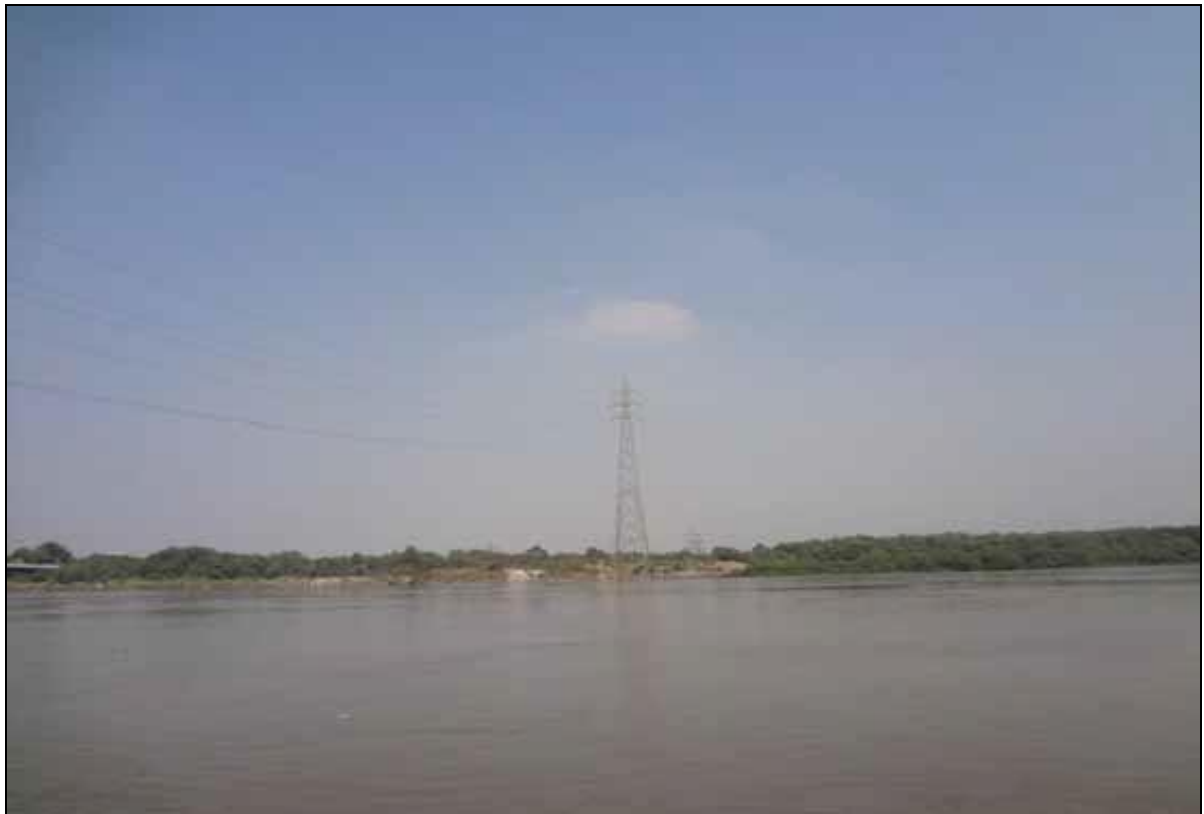
Photo 68: High Tension Line Crossing River at Ch 30.52km
