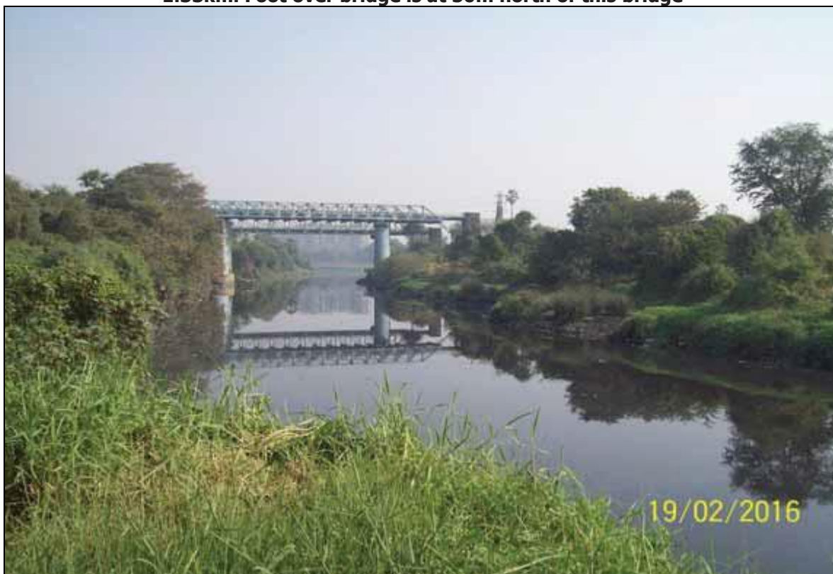
Photo 49: Showing towards north of the river at Ch 2.75km. 50m north there are two adjacent pipeline bridges
