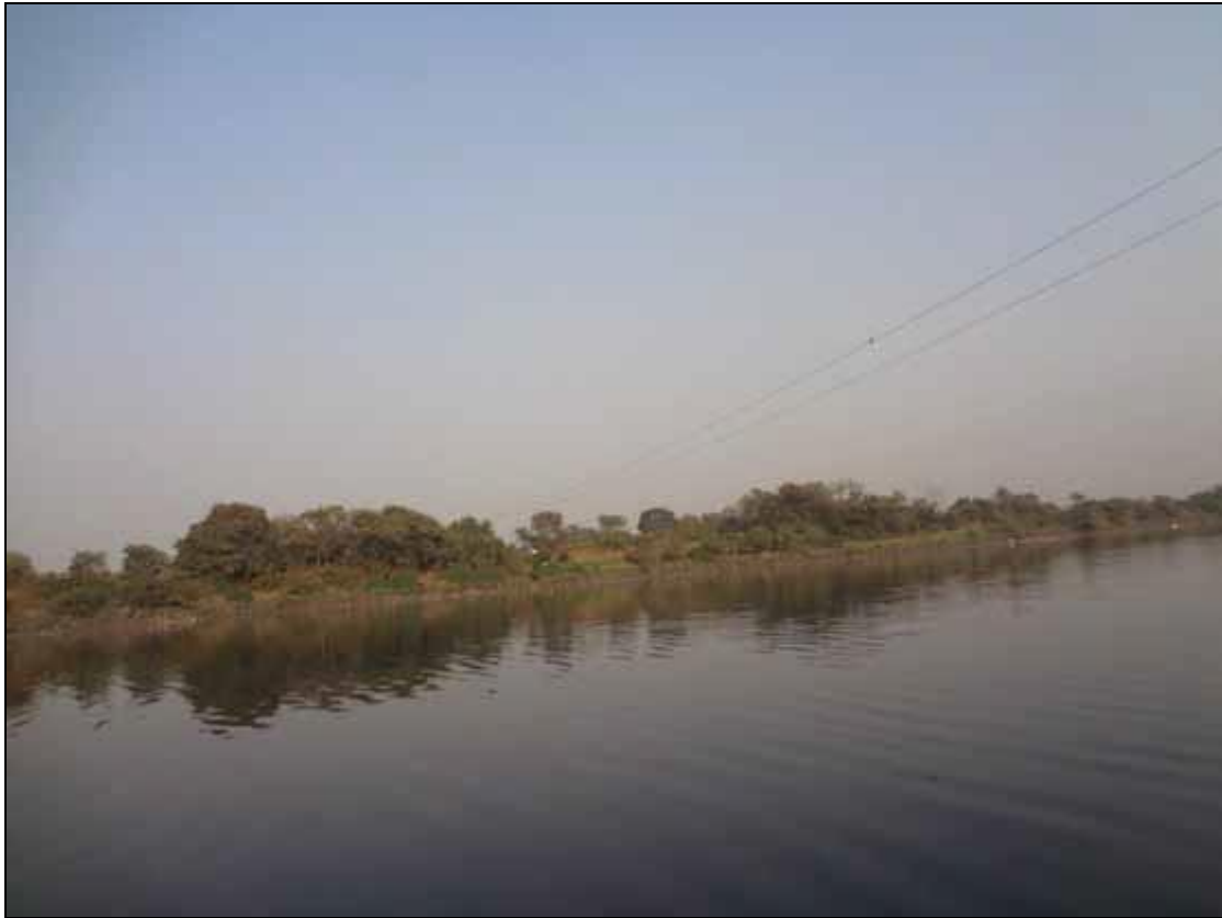
Photo 29: High Tension line crossing the River at Ch 69.82km
