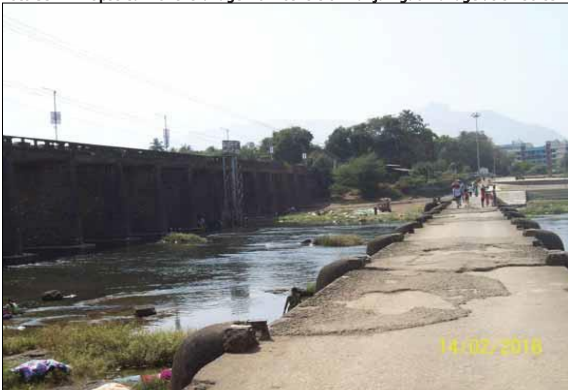
Photo 36: Badlapur Bridge and adjacent bridge at Ch 88.95km
