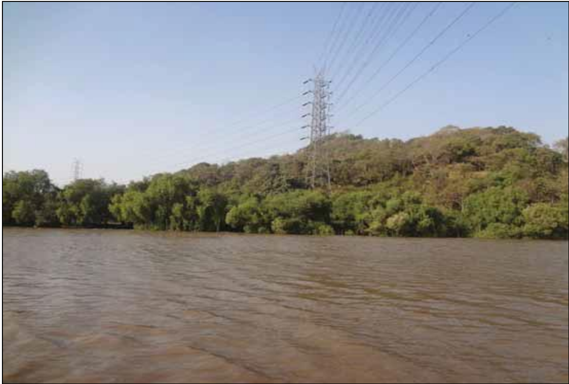
Photo 60: High Tension Line crossing the River Ch 13.51km
