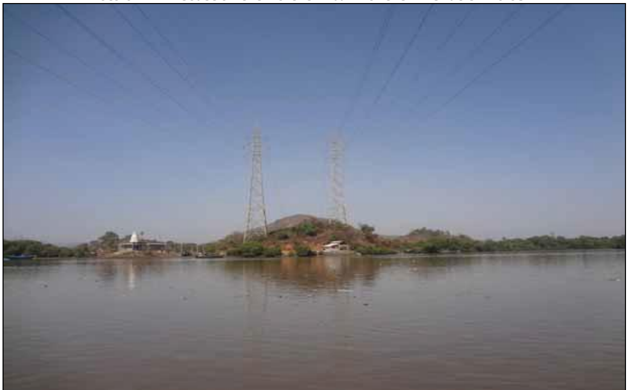
Photo 63: High tension line crossing the River at Ch 22.06km
