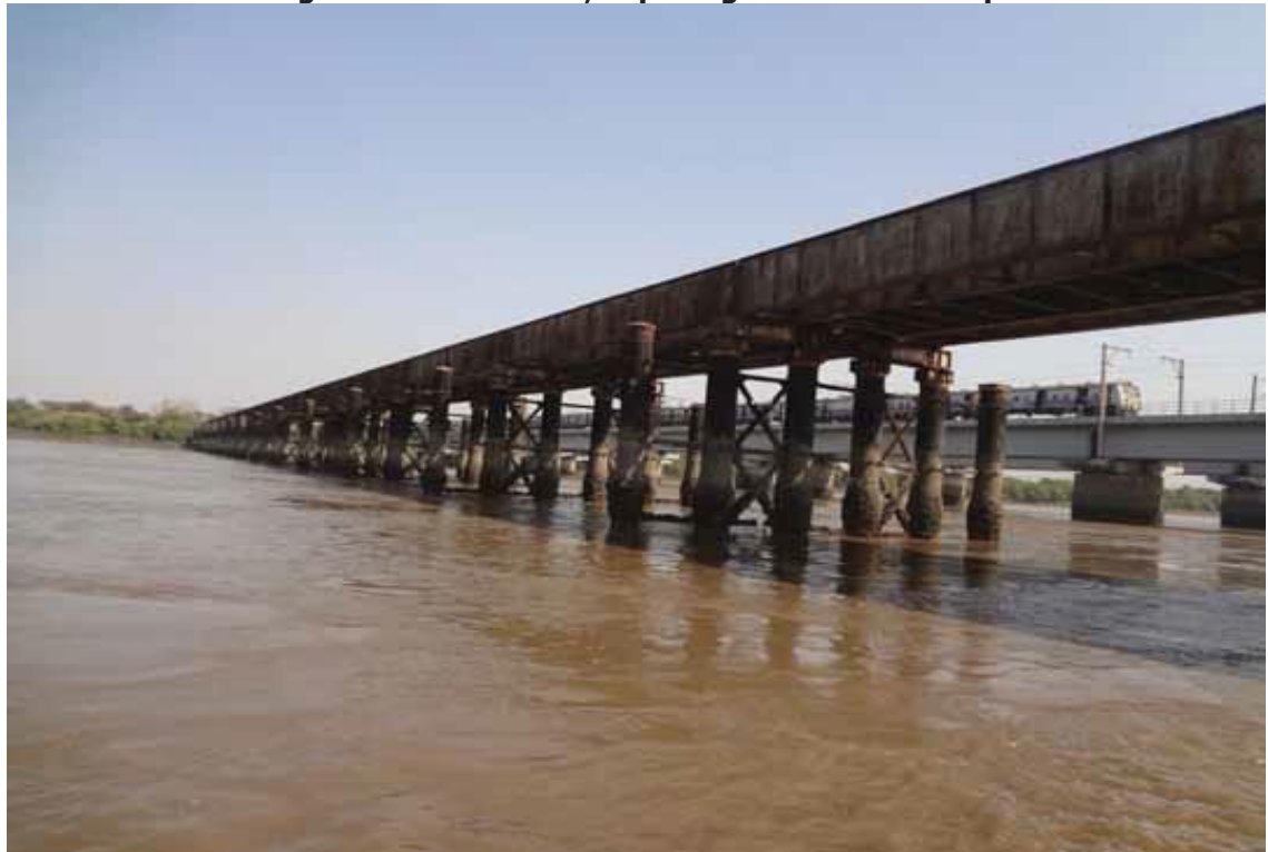
Photo 53: Mira Bhayandar old rail bridge at Ch 6.10km
