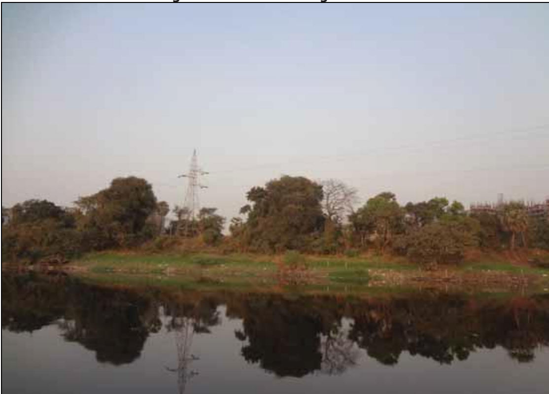
Photo 30: High Tension line crossing the River at Ch 73.39km
