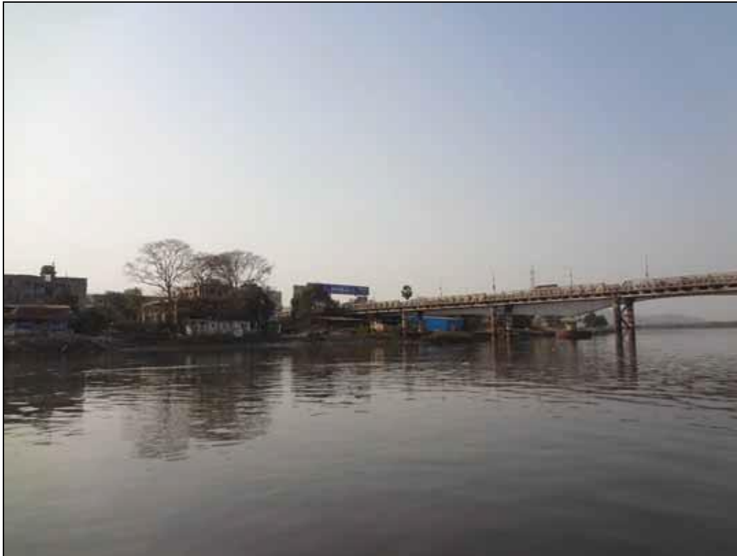
Photo 21: Kongaon old road bridge at Ch 56.14km
