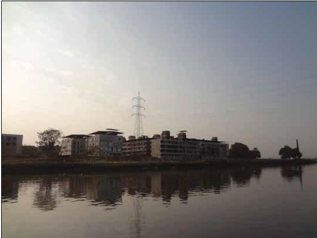
Photo 27: High Tension line crossing river at Ch 66.35km
