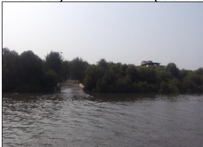
Figure 2.3 : Slope Jetty on the Western Bank of the River at Chainage 37.50km (19°10'50.2"N 72°58'59.9"E)
