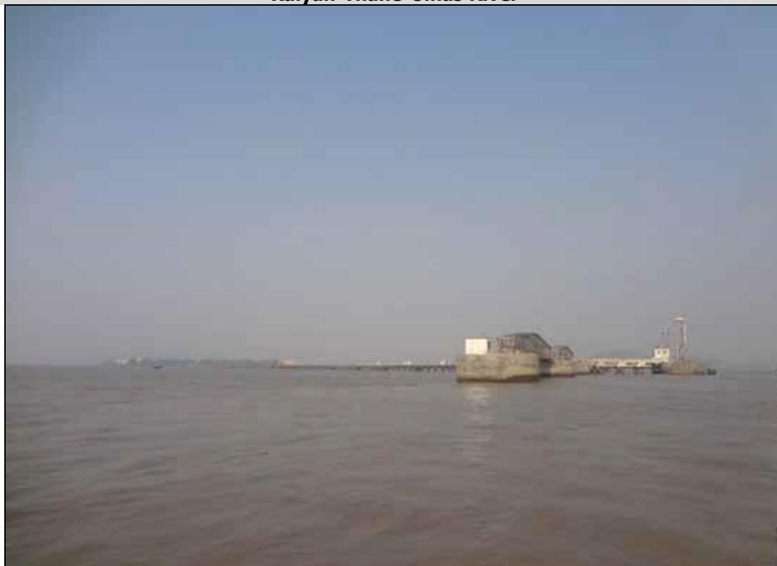
Photo 1: Jetty on the Northern Bank of River at Ch 4.00 km
