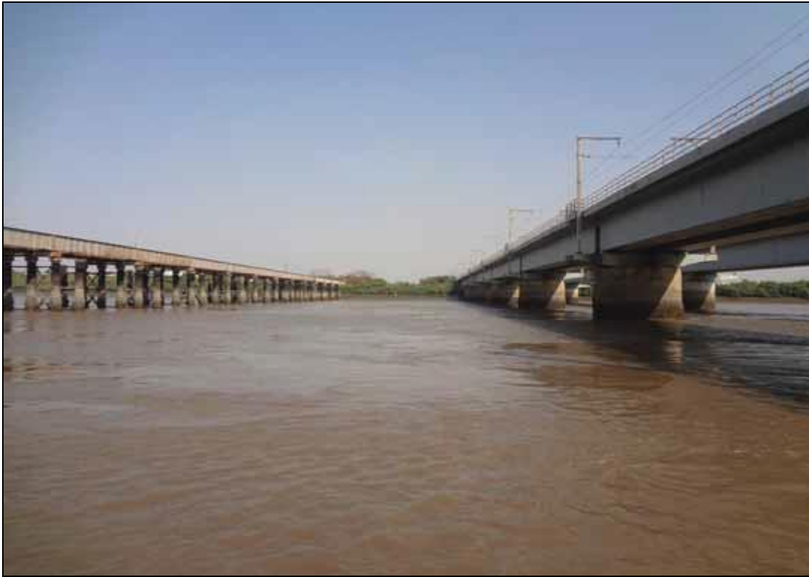
Photo 54: Mira Bhayandar new rail bridge at Ch 6.29km
