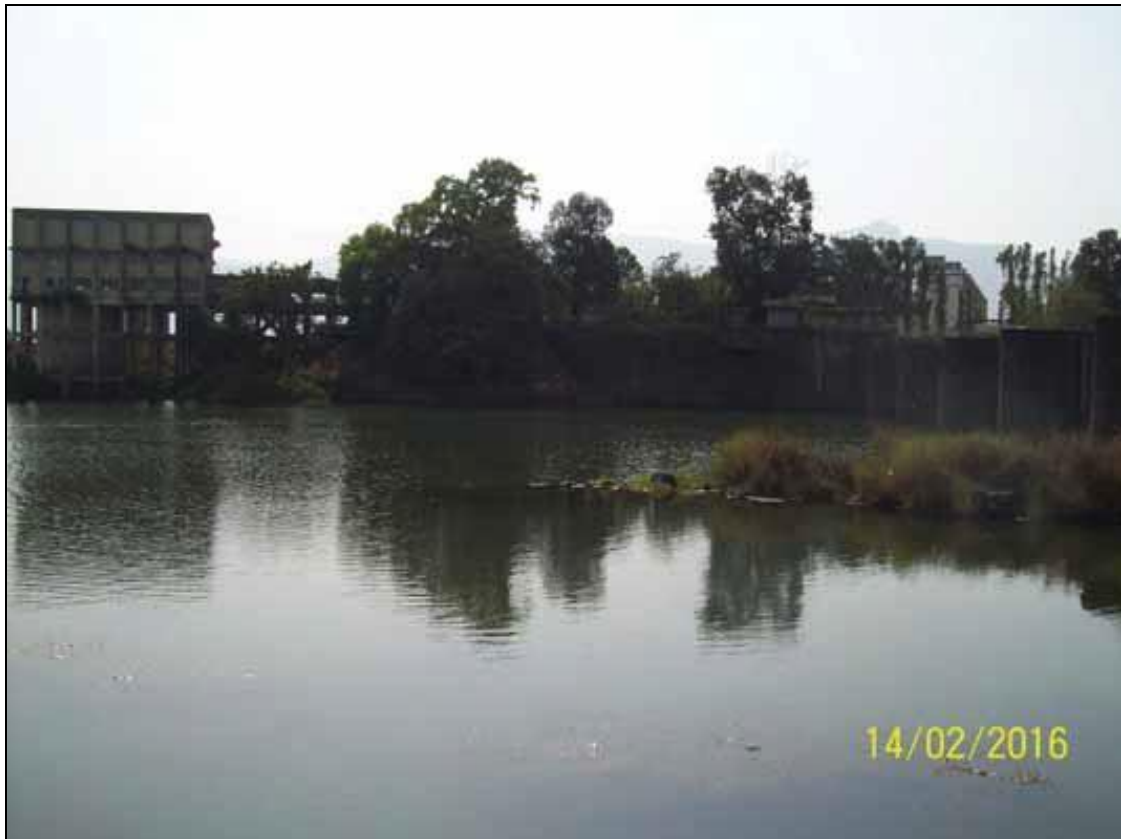
Photo 41: Water treatment plant and broken bridge at Ch 90.82km
