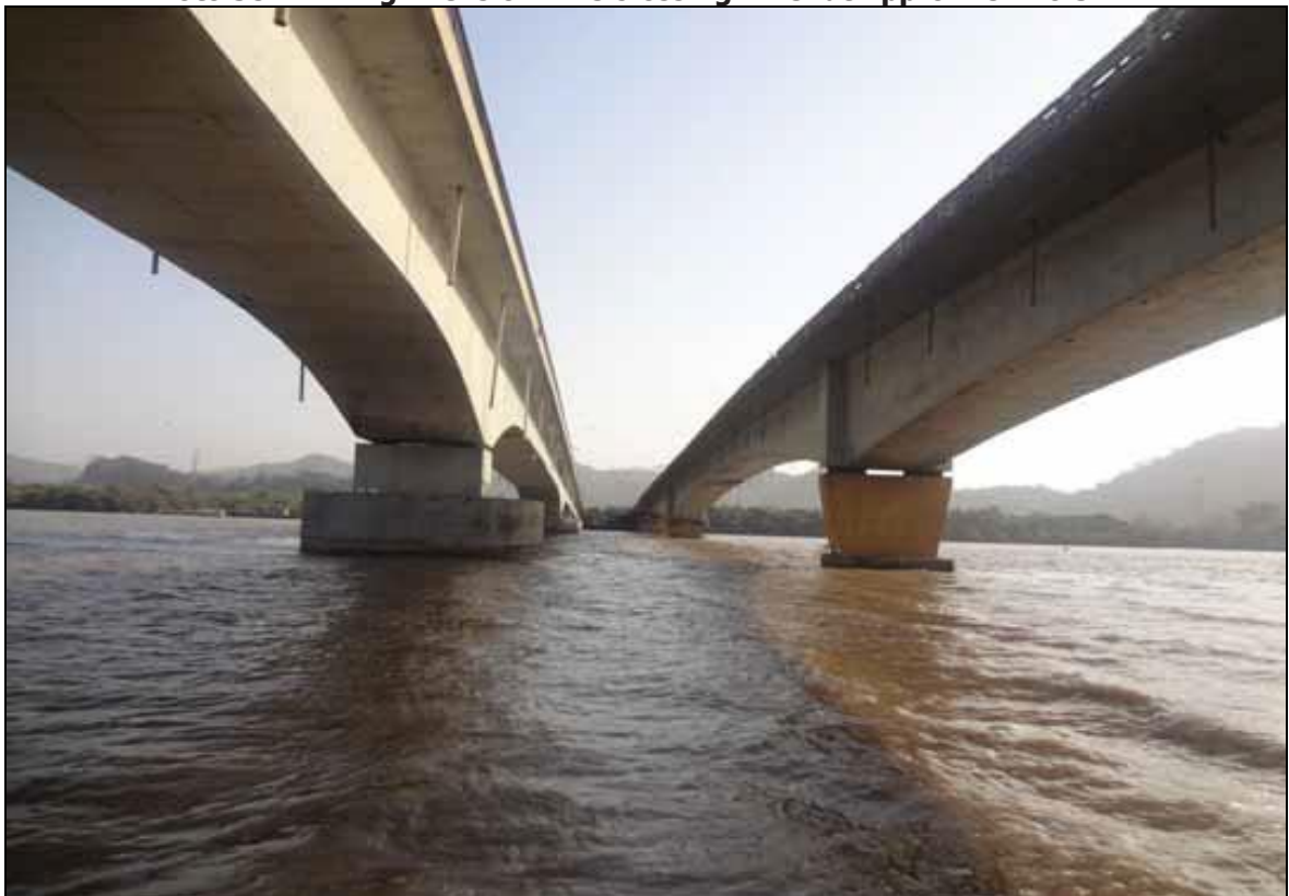
Photo 59: Mira Bhayandar Road bridge at Ch 13.51km
