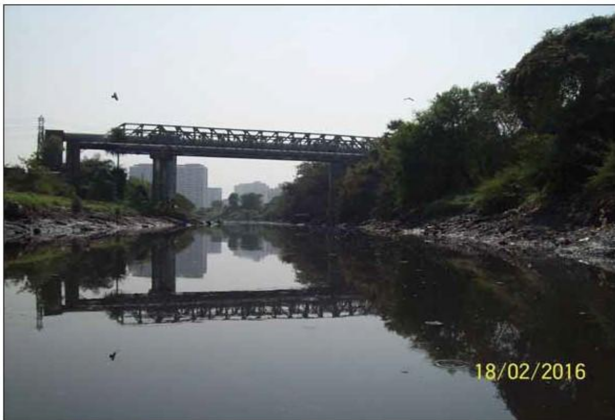
Photo 51: Pipeline bridge towards Kalyan at Ch 3.16km
