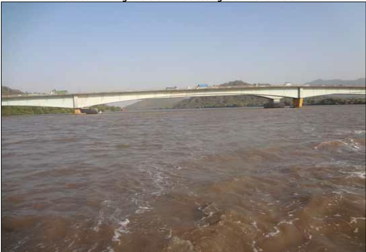
Photo 61: Mira Bhayandar Road bridge Ch 14.198 km
