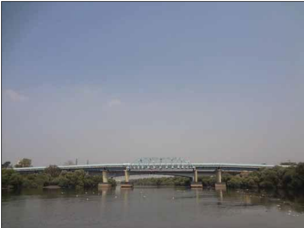
Photo 13: Kalwa pipe line bridge at Ch 37.03km
