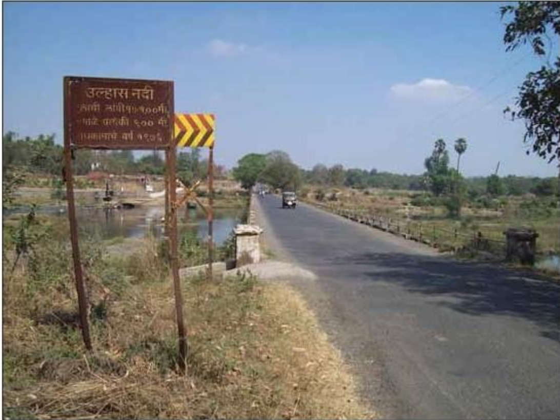
Photo 45: North of the bridge towards Malegaon at Ch 111.23km
