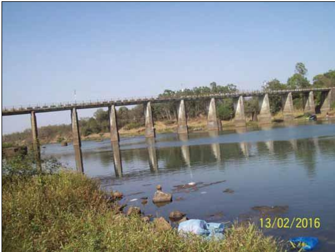
Photo 43: Pashan Road Bridge from Ch 100.94km
