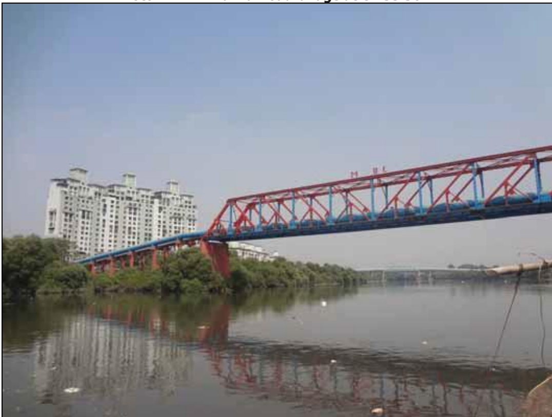
Photo 12: Kharegaon pipe line bridge at Ch 36.46km
