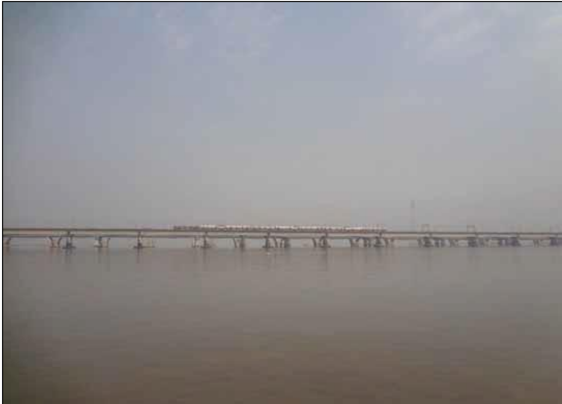
Photo 3: Vashi Rail bridge at Ch 19.52 km
