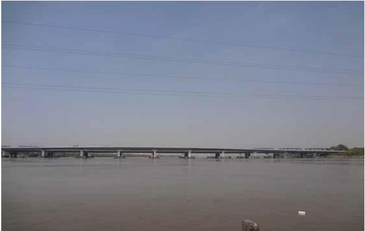
Photo 66: Kasheli Road Bridge at Ch 29.969 km
