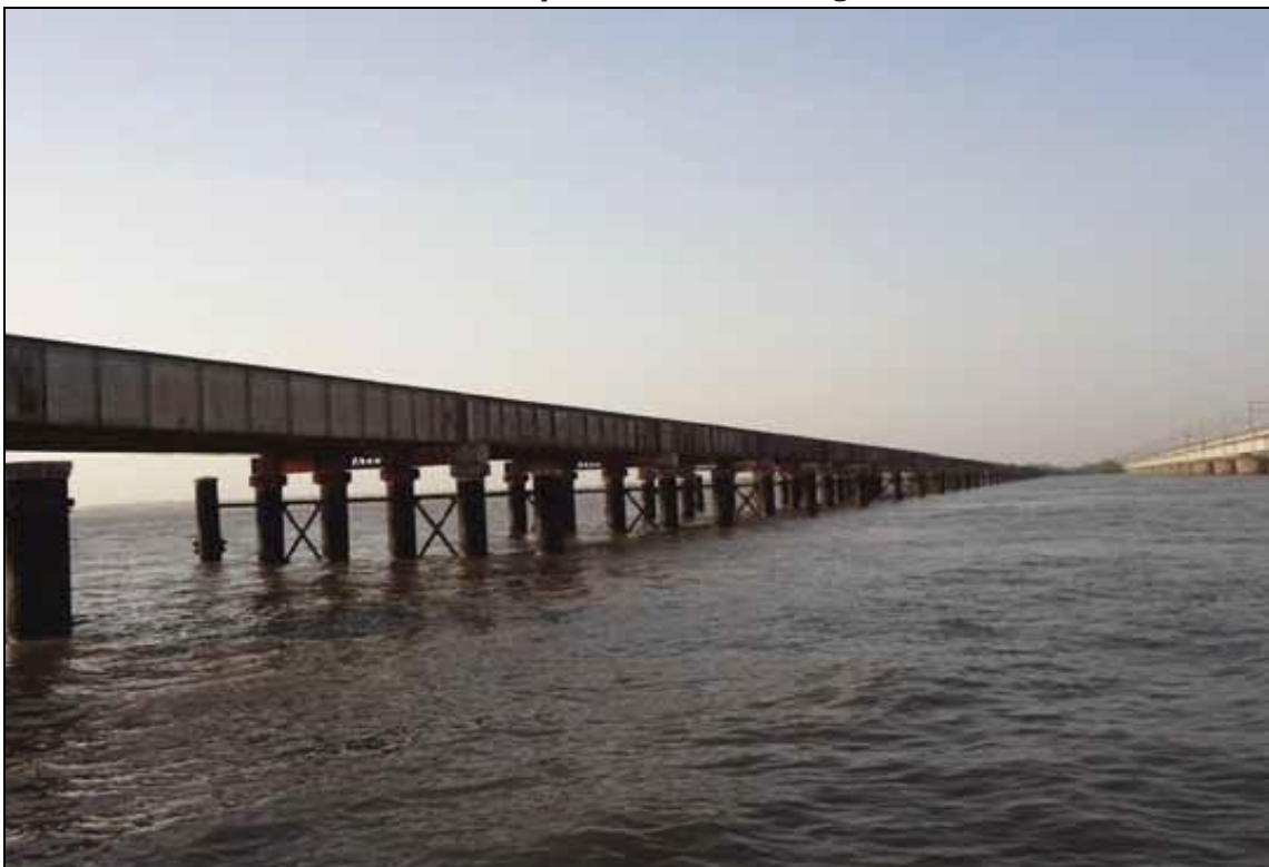
Photo 55: Mira Bhayandar old rail bridge at Ch 6.68km
