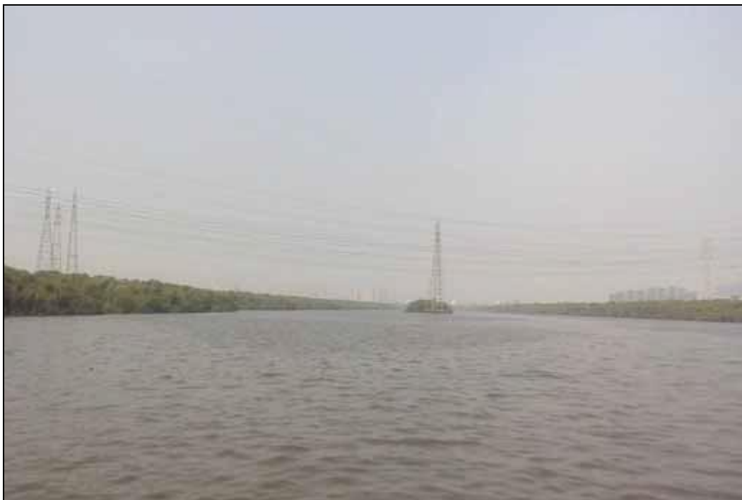
Photo 8: High Tension Power Line crossing River at Ch 31.93 km
