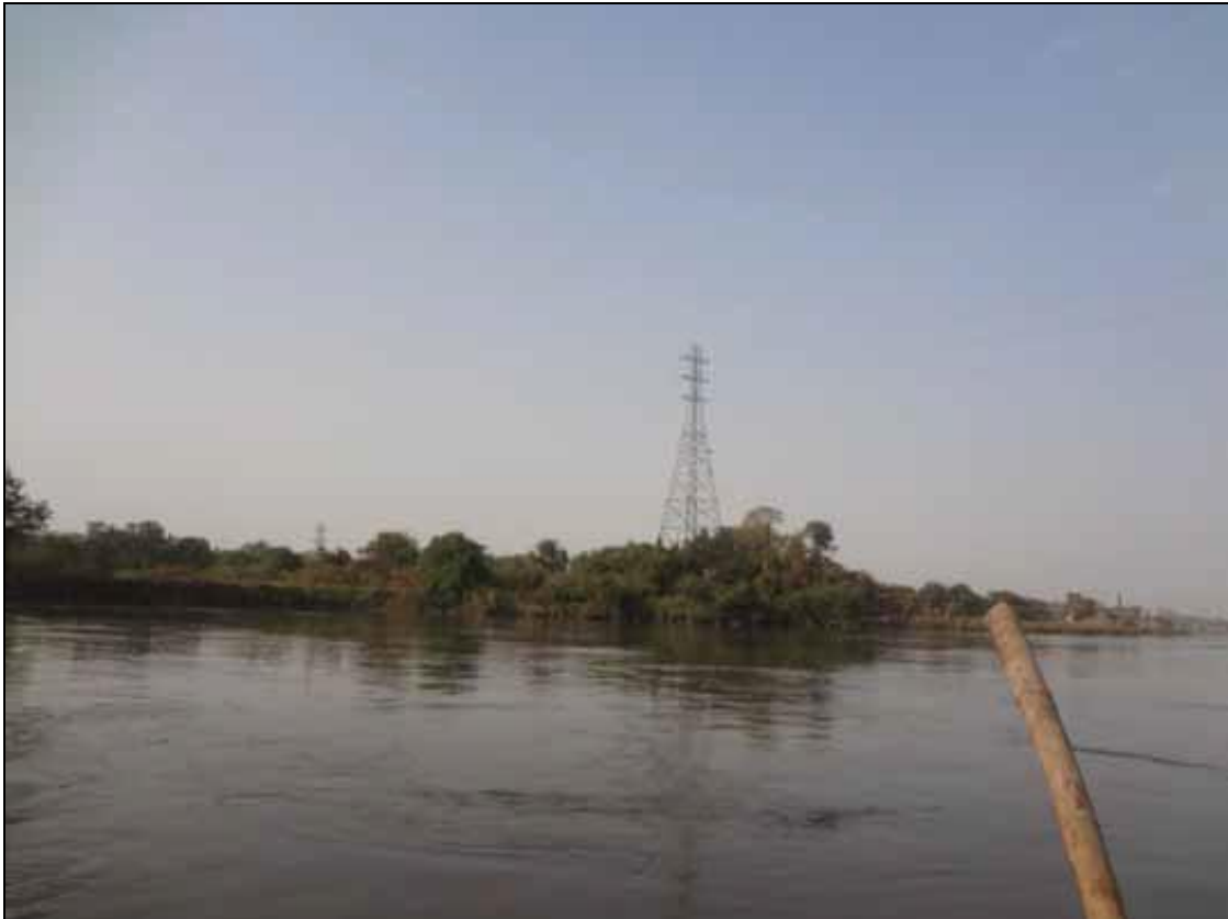
Photo 25: High Tension line at Ch 62.99km
