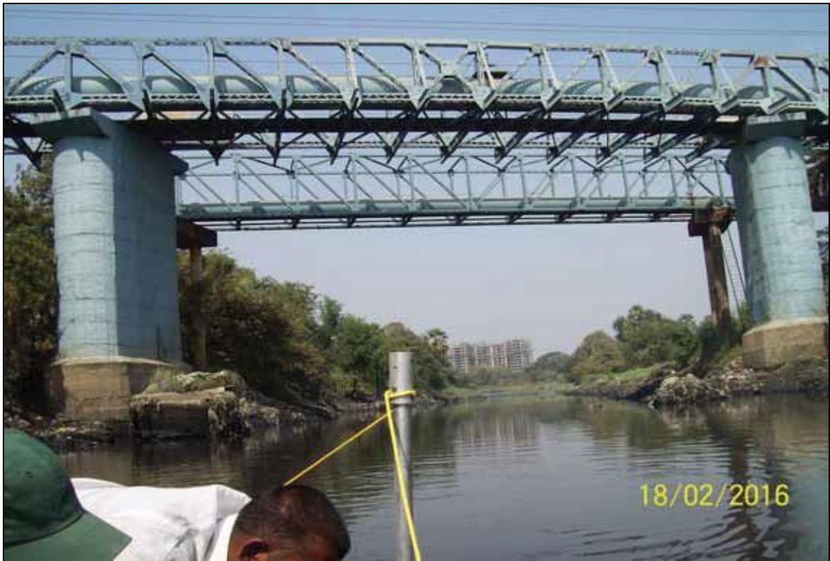
Photo 50: Showing twin pipeline bridge at Ch 2.94km
