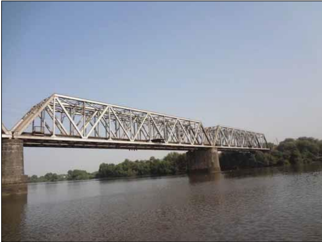
Photo 19: Bhiwandi - Dombivli Rail Bridge at Ch 50.70km
