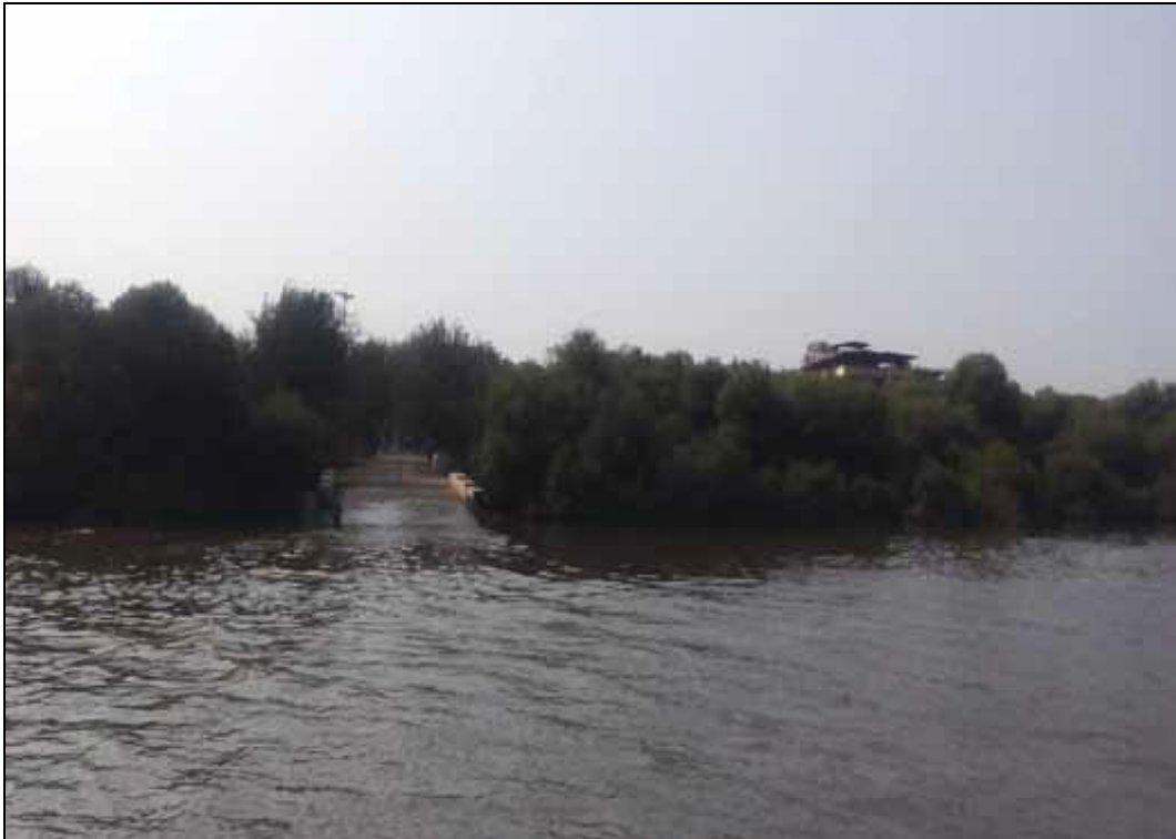
Photo 15: Slope Jetty on the Western Bank of the River at Ch 37.50km
