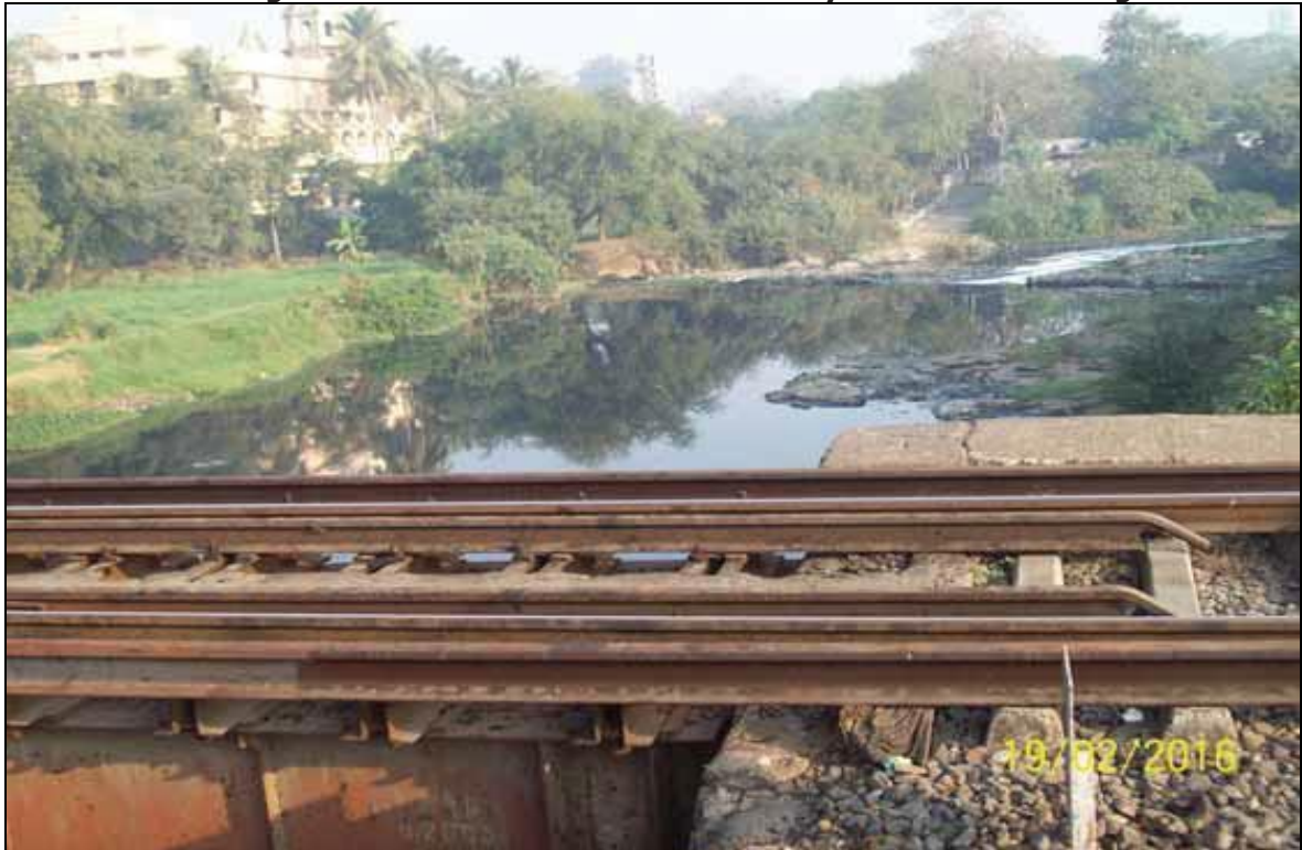
Photo 47: Showing towards north of river from Railway Bridge at Ch 1.00km
