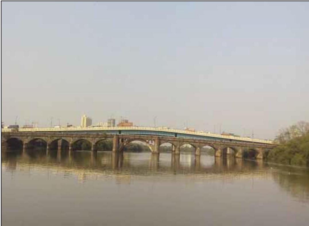
Photo 11: Kalwa Road bridge at Ch 35.36km
