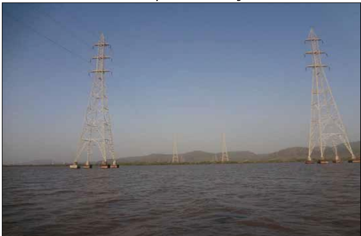
Photo 57: High Tension Power line crossing River. at Approx. Ch 10.31km
