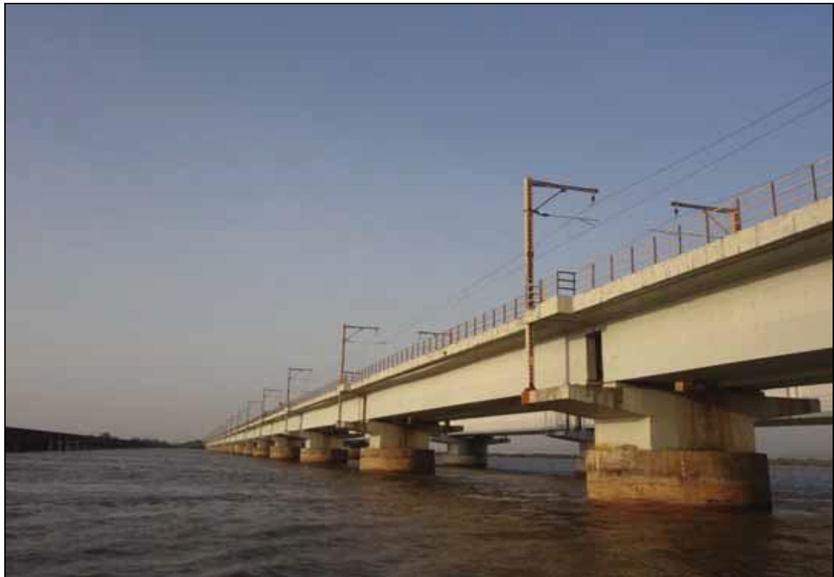
Photo 56: Mira Bhayandar new rail bridge at Ch 6.29km
