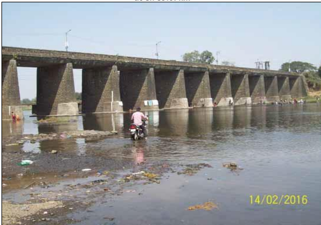
Photo 38: Badlapur Bridge at Ch 89.07km
