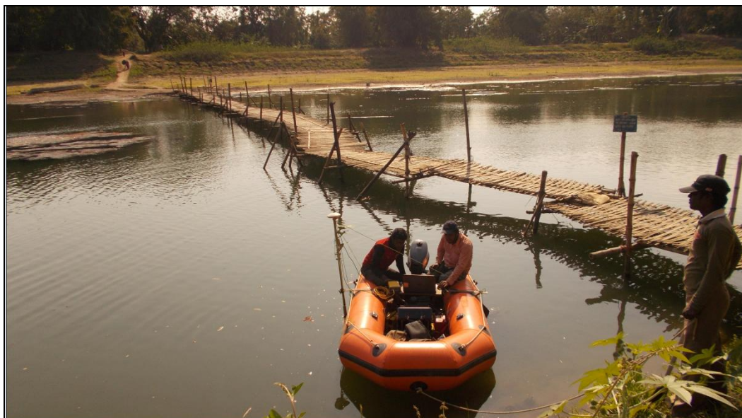
Figure 7-Bamboo Bridge (Chainage- 4.019 km)
