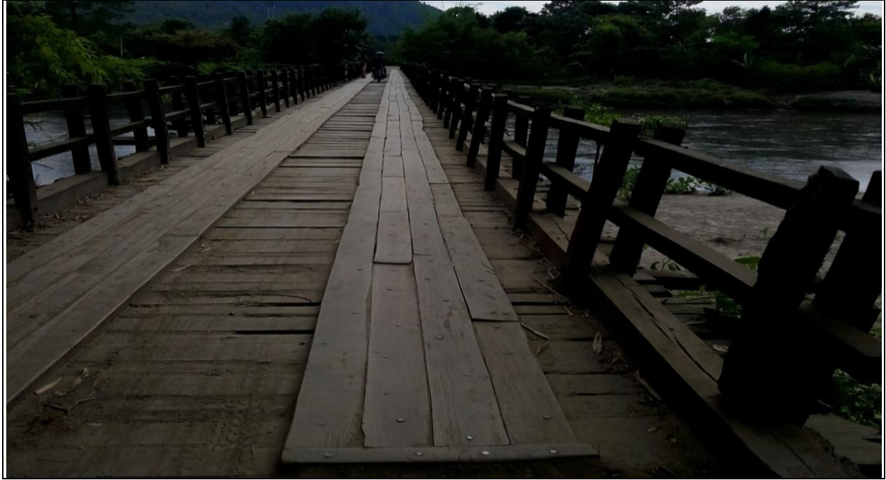
Figure 11- Wooden Bridge (Chainage-17 km)
