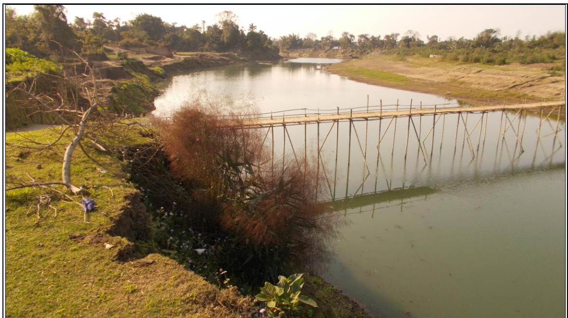
Figure 20-Bamboo Bridge (Chainage-50.703 km)
