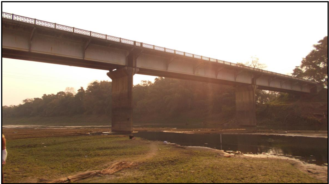
Figure 19 RCC Bridge (Chainage-63.202 km)
