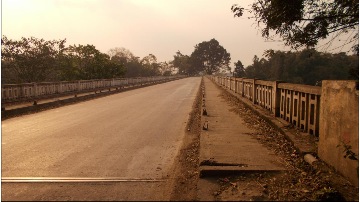
Figure 14- RCC Bridge (Chainage-34.294 km)
