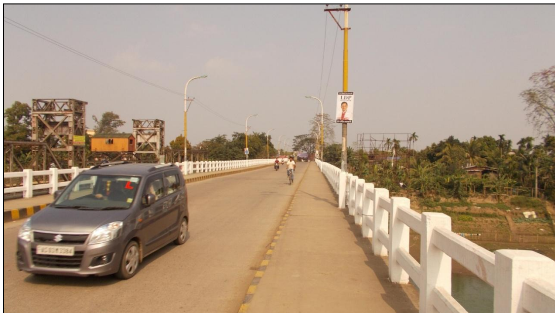
Figure 17- RCC Bridge (Chainage- 42.575 km)
