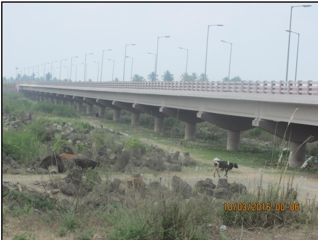
10: Mananadu Bridge at Chainage 14.4 km
