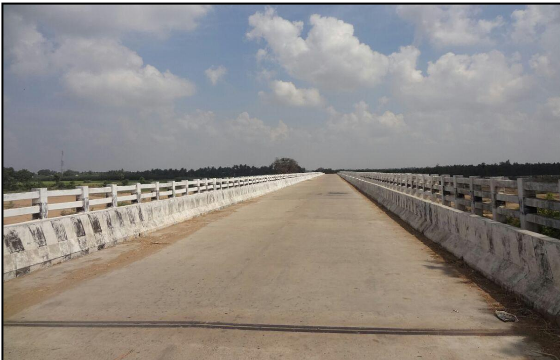
18: Paiyur Bridge at chainage 53.0 m
