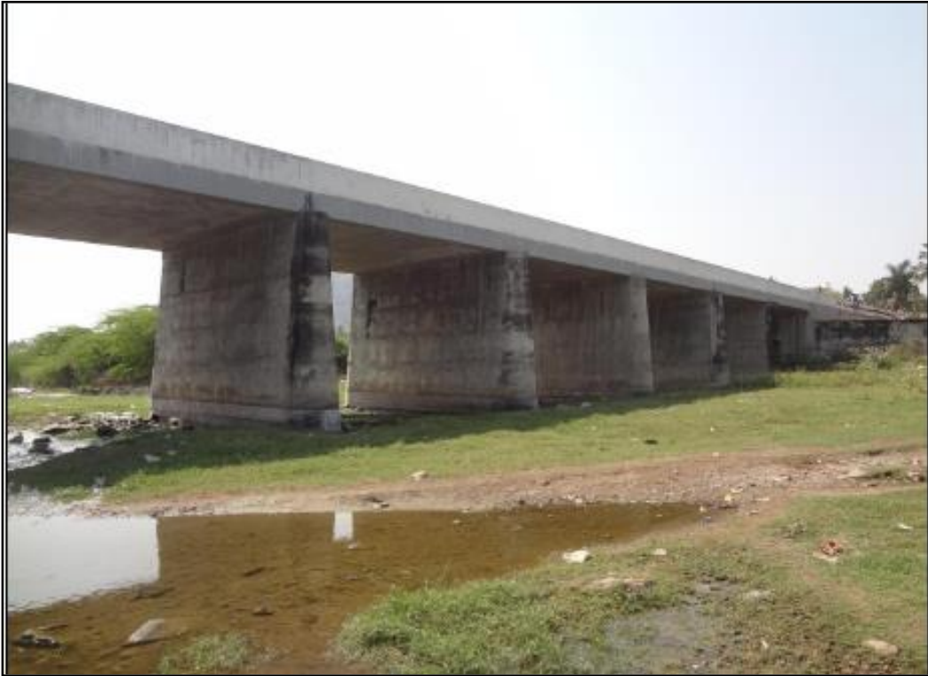
28: Raindapuram to Allapannur Bridge at ch 108.7 km
