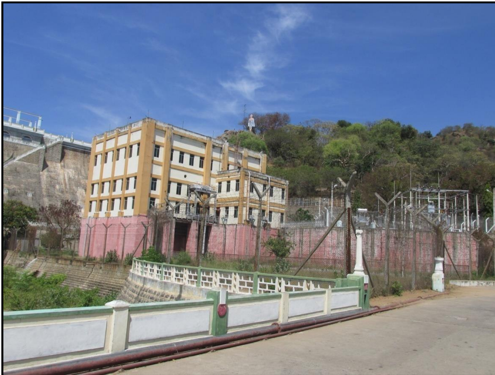
39: Powerhouse of Sathnur Dam at Chainage 125.0 km
