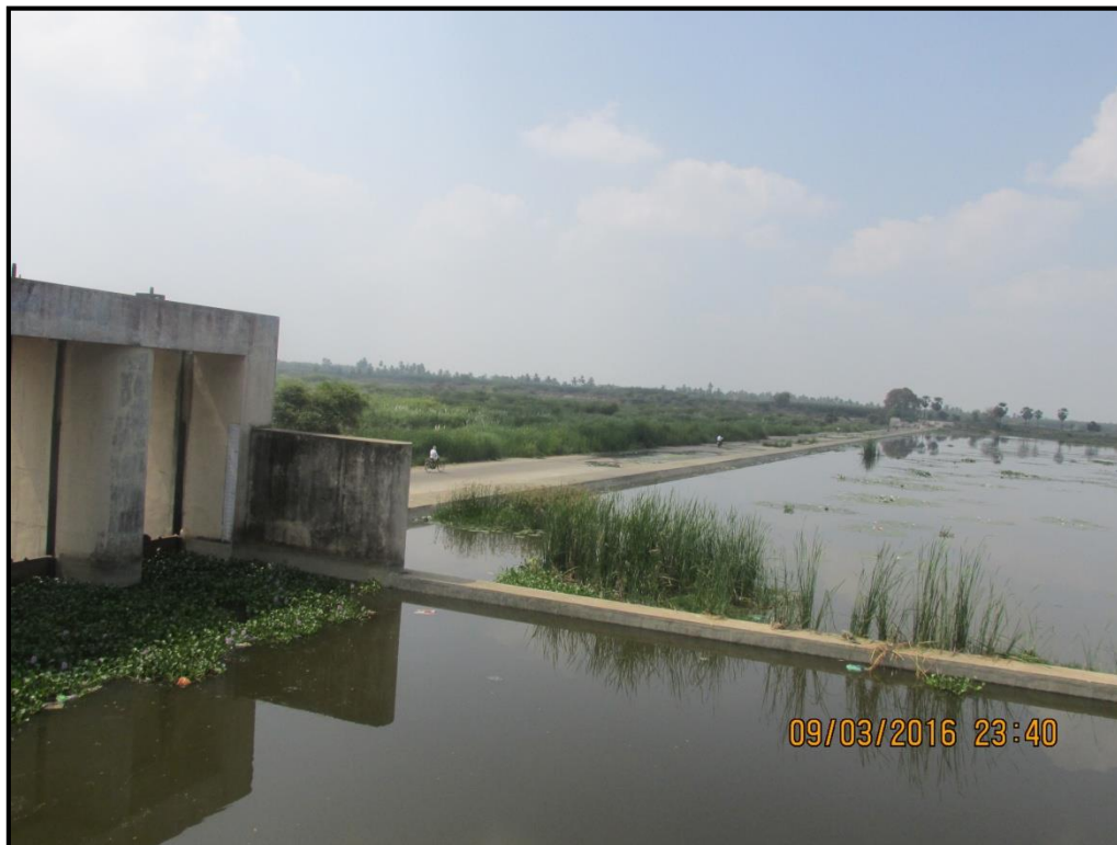
8: Marudadu Dam at Chainage 9.8 km
