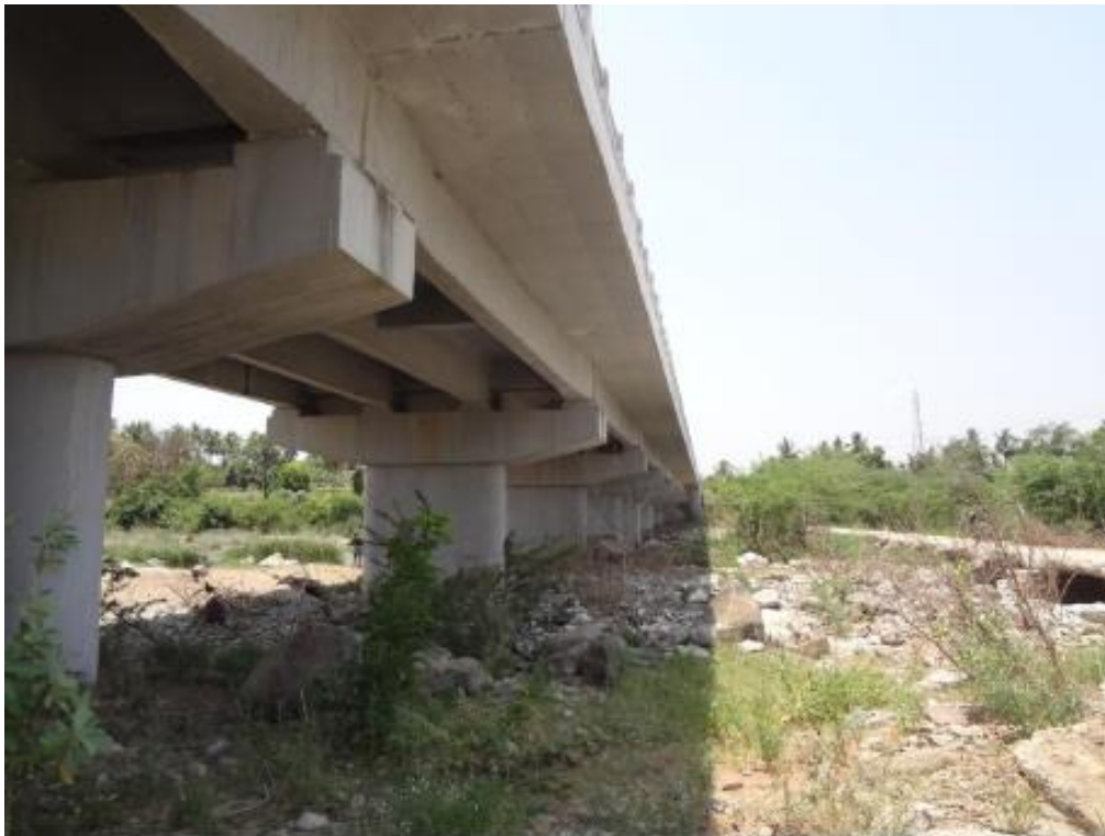
29: Kolamanjanur Bridge, VC-6m, HC-18m at Chainage 115.4 km
