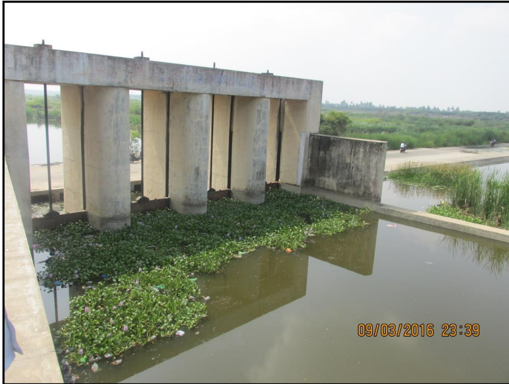
7: Marudadu Dam at Chainage 9.8 km
