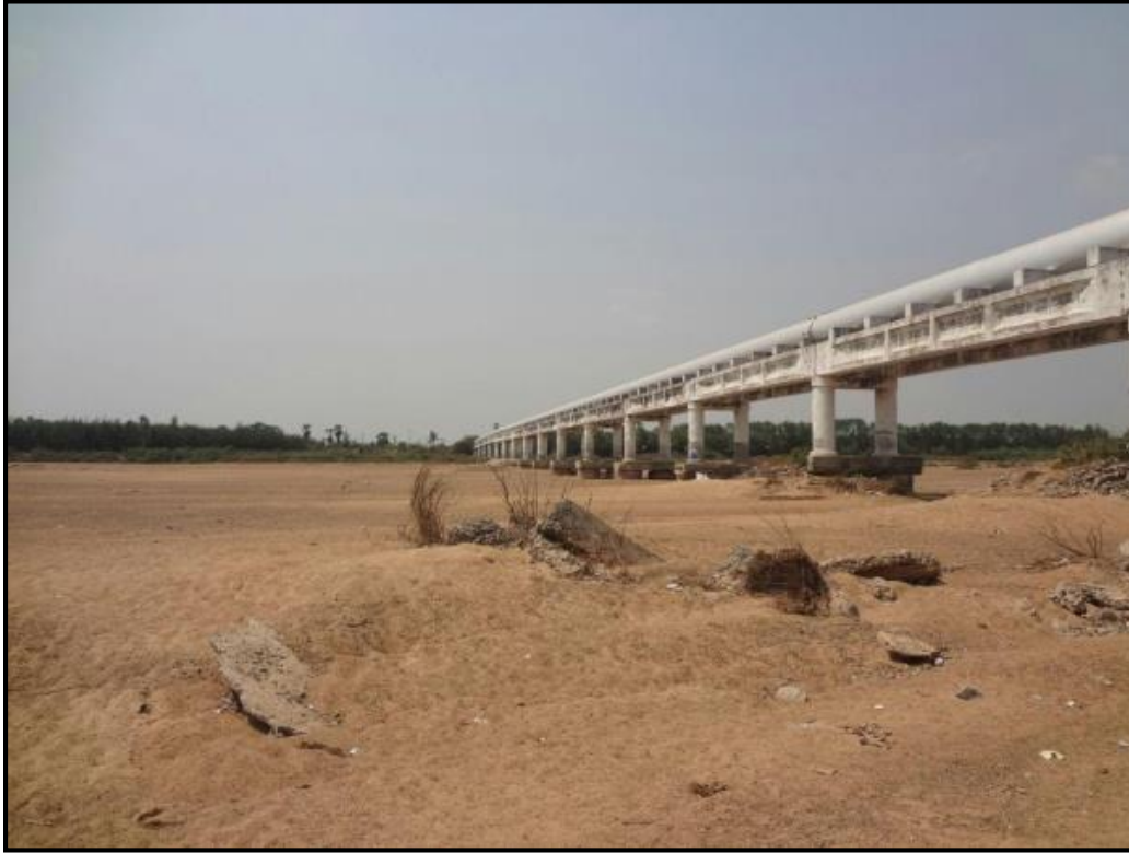
13: Veeranam Chennai Water Pipeline at Chainage 29.2 km
