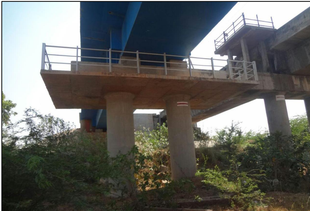
16: Railway Bridge at Chainage 42.9 km
