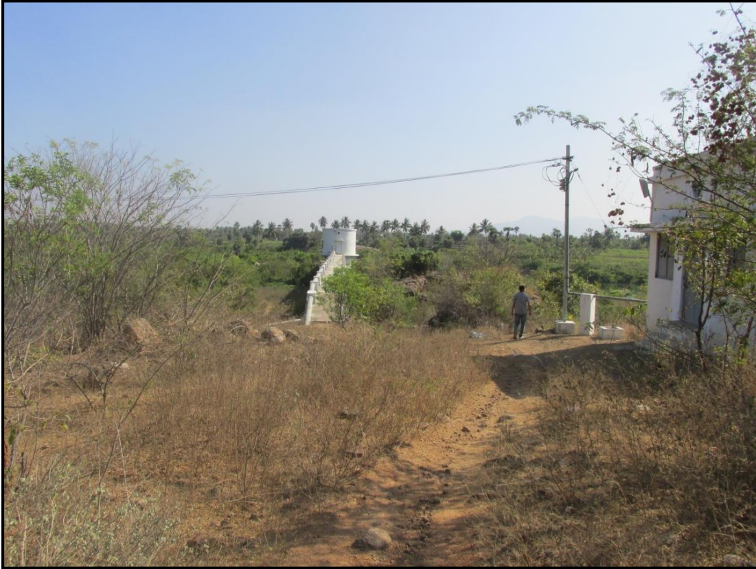
30: Water Intake on right bank at Chainage 116.8 km
