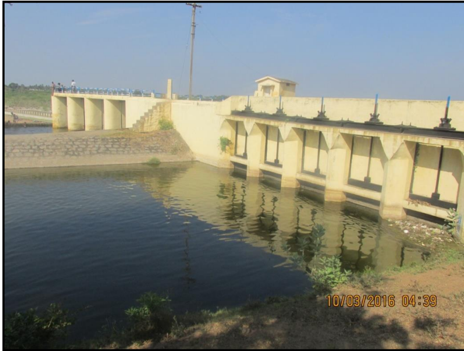
22: Tirukoilur Anicut system at Chainage 65.9 km
