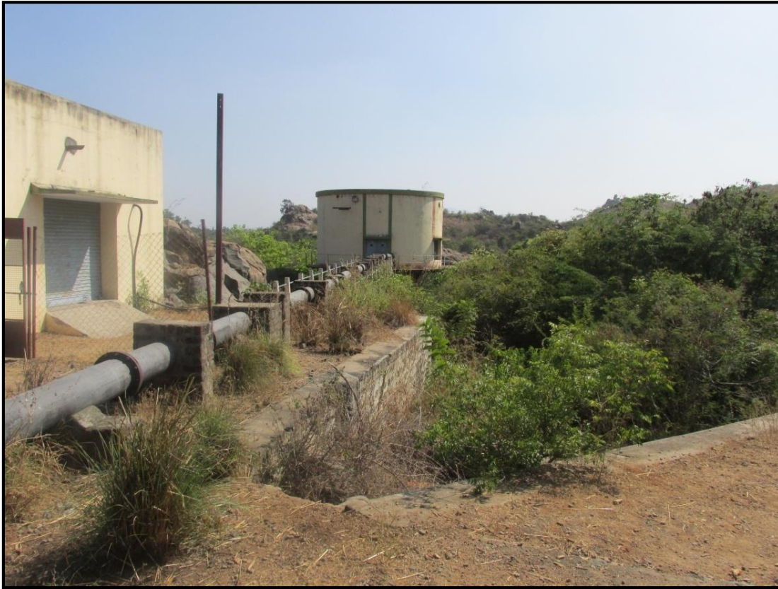
34: Water Intake on left bank at Chainage 118.1 km
