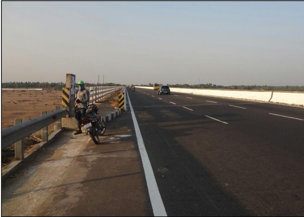
15: Villupuram Bridge VC-4m, HC-18m at Chainage 41.7 km
