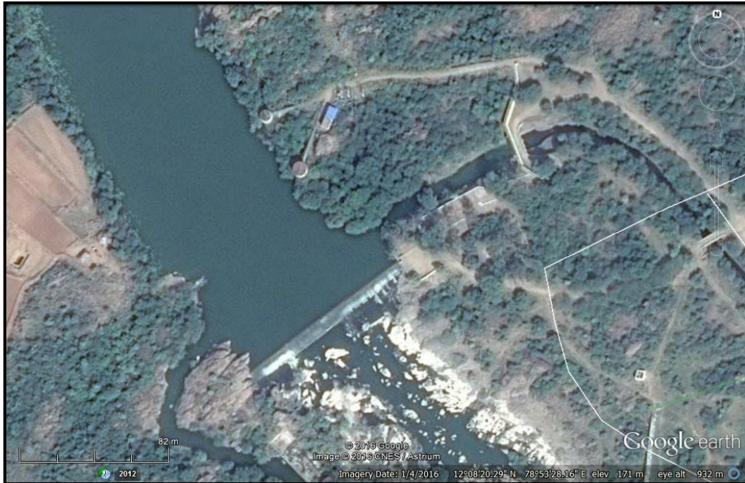
33: Google layout of Pickup Dam at Chainage 117.2 km
