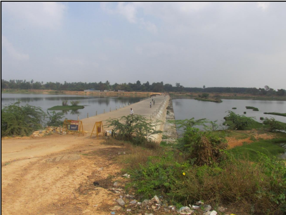
4: Kumandanmedu Ground Bridge at Chainage 4.4 km
