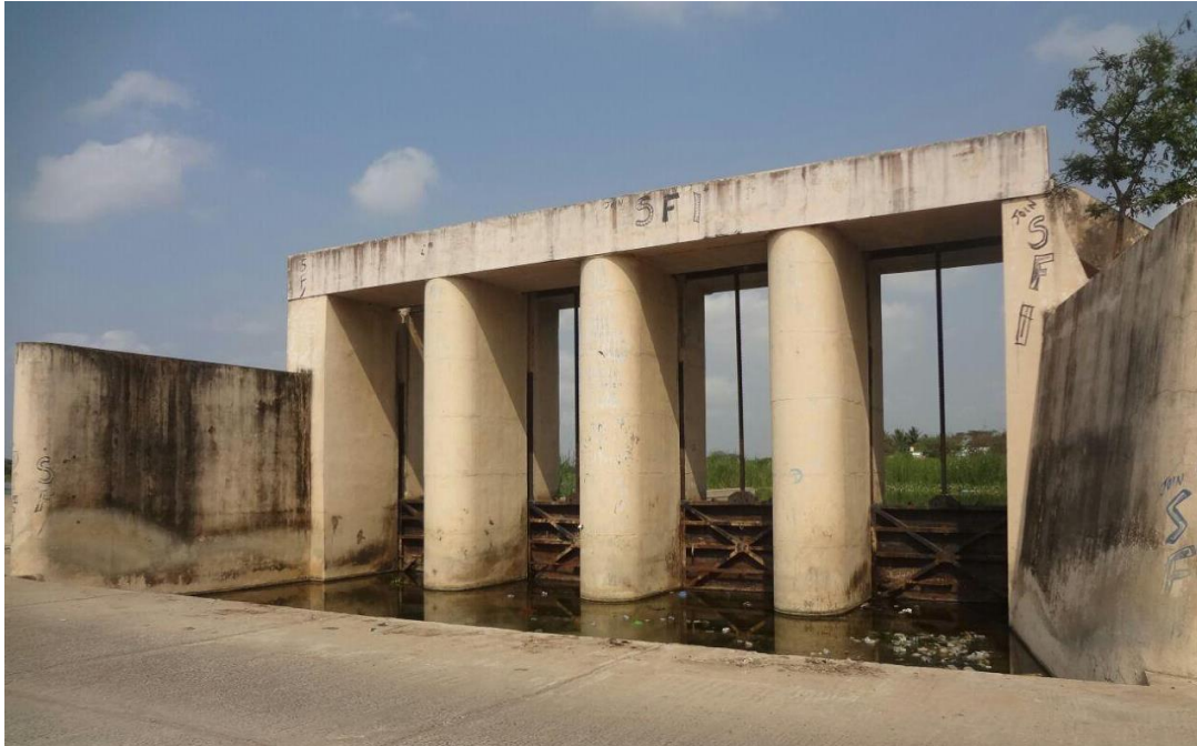
9: Marudadu Dam at Chainage 9.8 km
