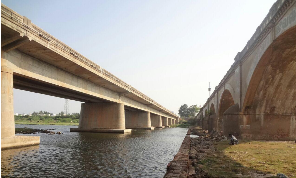
3: Road Bridge at Ponniyar River Mouth (Chainage 3.5 km)
