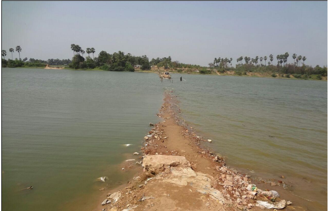
5: Local crossing at ch 5.1 km
