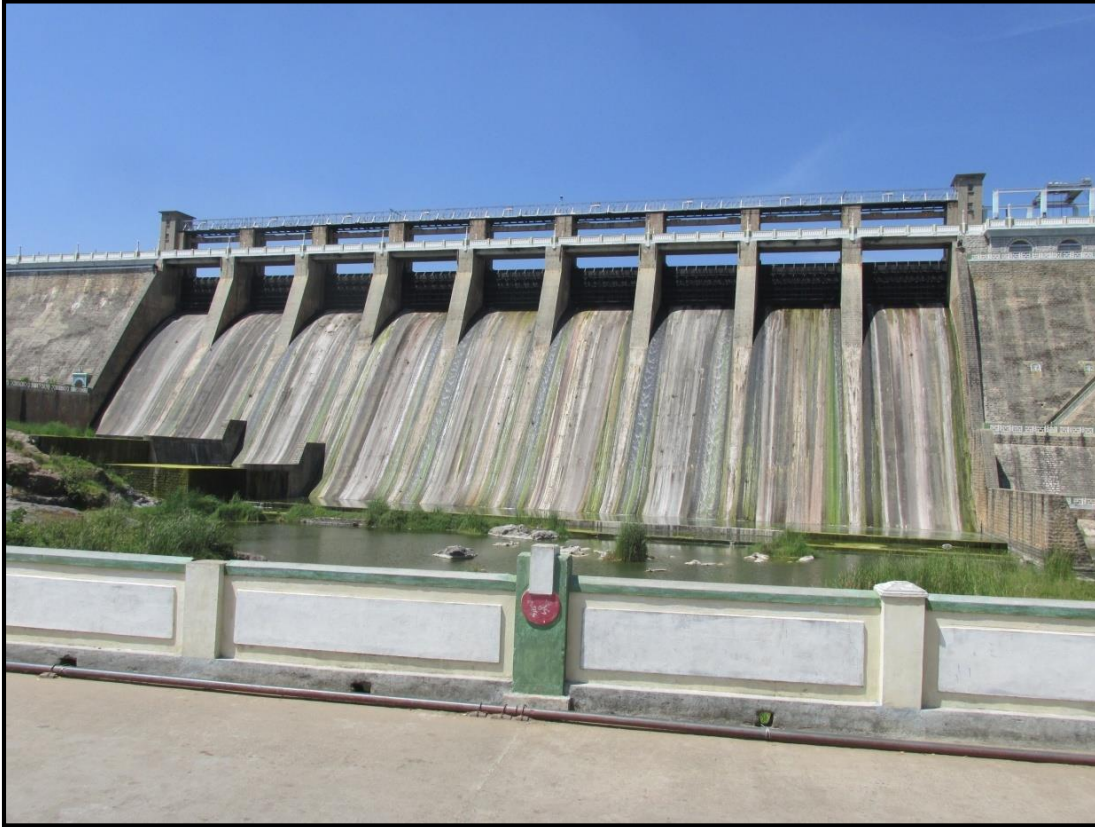
36: Sathnur Dam Project at 125 km
