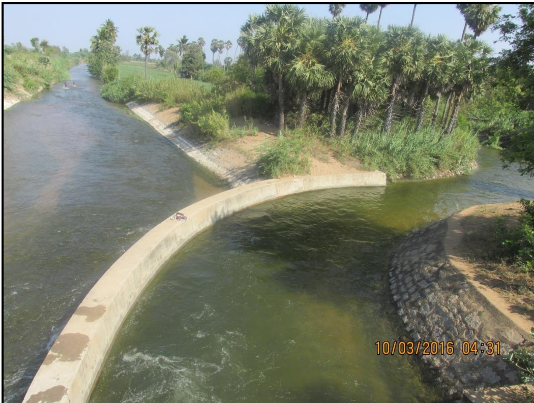
23: Tirukoilur Anicut system - Offtaking Canals- Chainage 65.9 km
