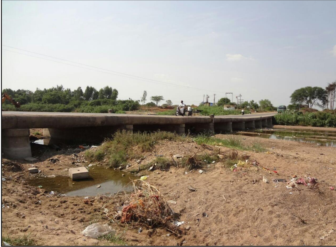
24: Malanurpet to Thuruvam Road Bridge at chainage 86.3 km
