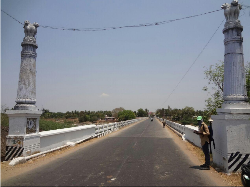
26: Vazhavachanur to Moongalthuraipet Bridge at ch 101.2 km
