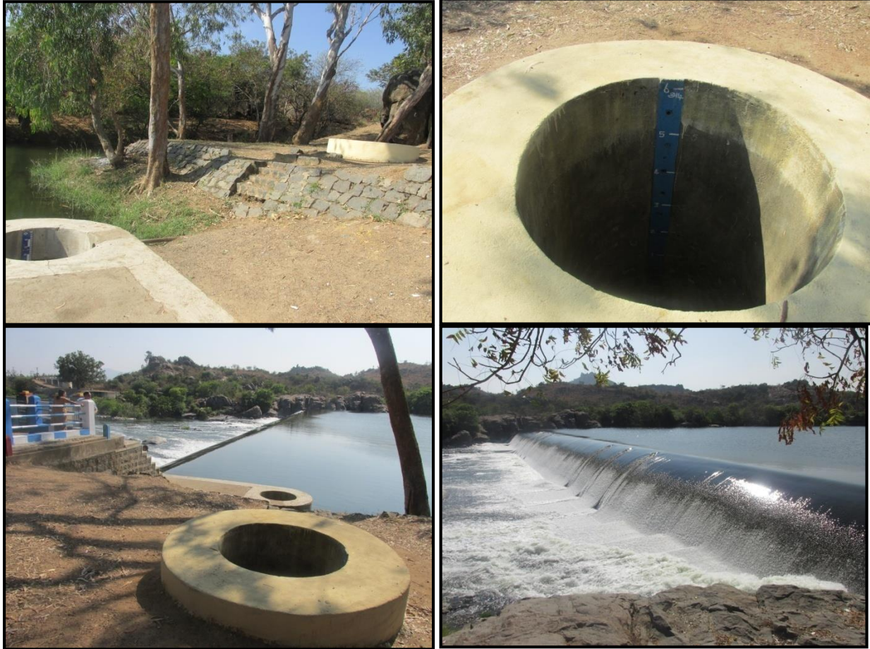
32: Pickup Dam at Chainage 117.2 km
