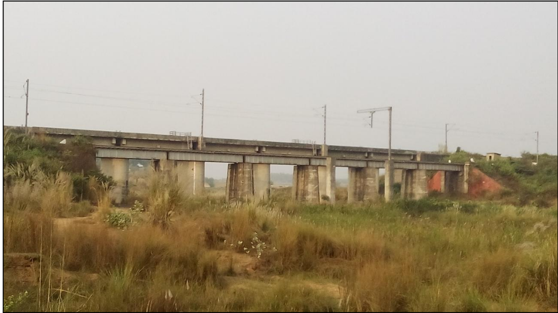
Figure 35-Rail Bridges (Chainage- 133.800 km and 134.310 km)
