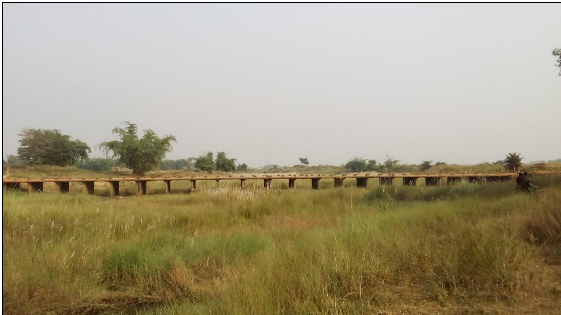
Figure 33- RCC Bridge (Chainage- 123.250 km)
