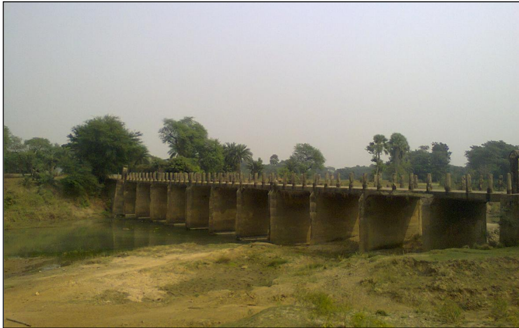
Figure 22- RCC Bridge (Chainage- 74.650 km)
