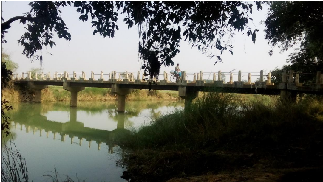
Figure 15- RCC Bridge (Chainage- 54.613 km)
