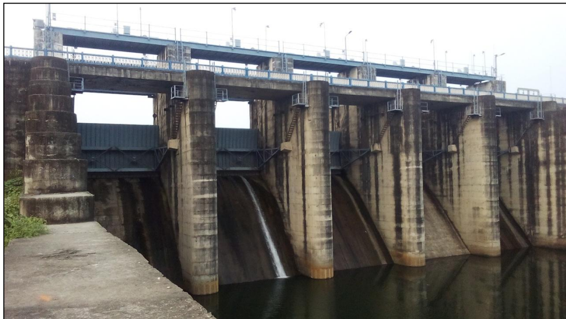
Figure 36-Nil Nirjan Dam (Chainage-135.165 km)
