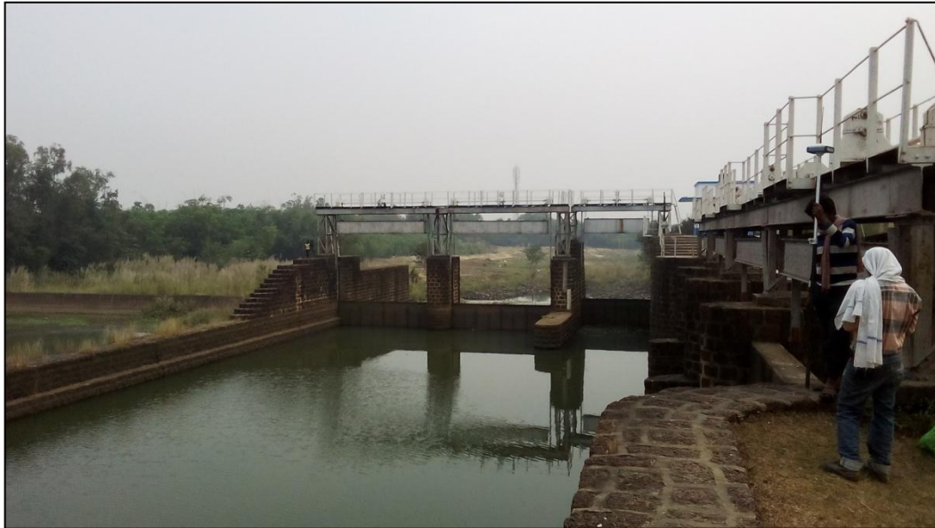
Figure 32- Check Dam (Chainage- 129.00 km)
