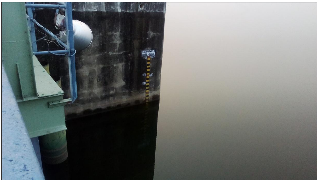
Figure 63- Bakreswar Dam Site near Chinpai village (Chainage-135.165 km)
