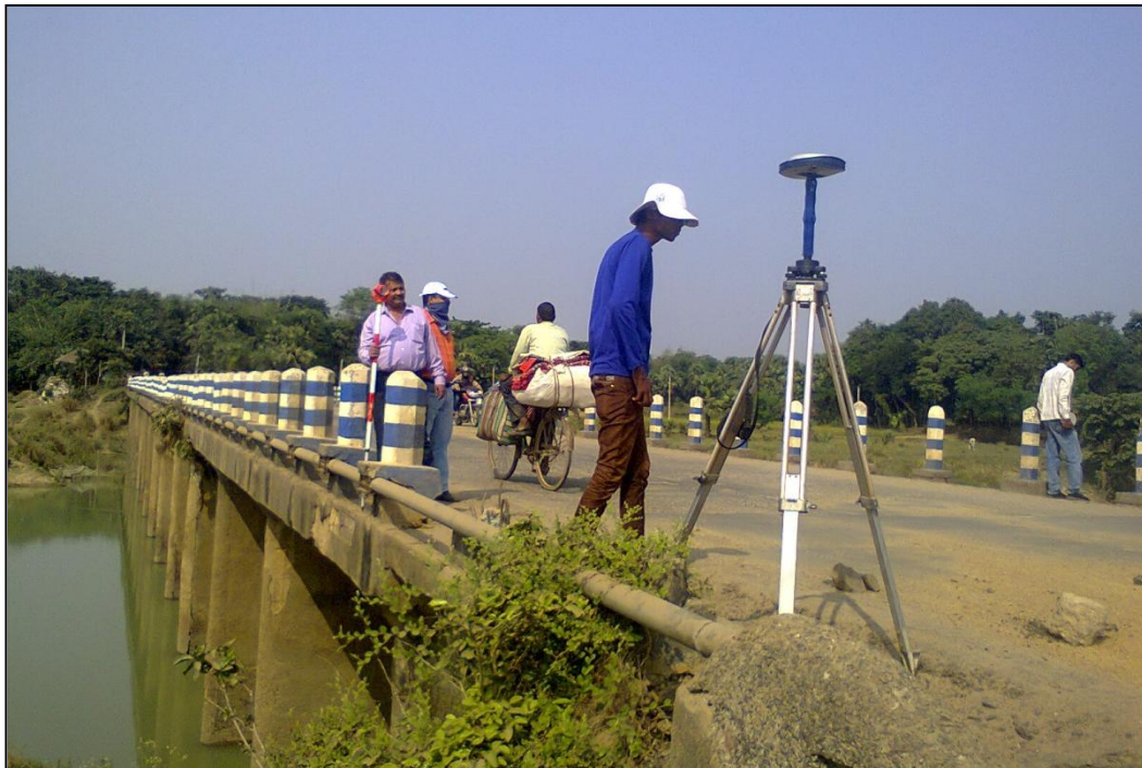
Figure 19- RCC Bridge (Chainage- 65.650 km)
