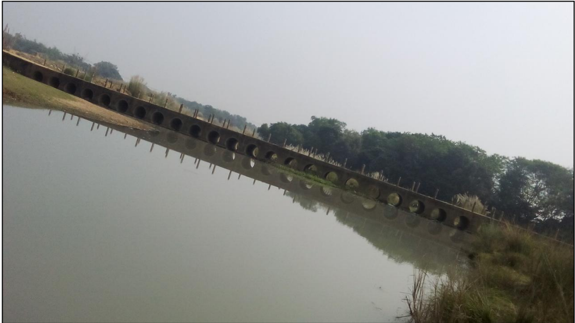
Figure 6-Pipe Bridge (Chainage- 18.855 km)
