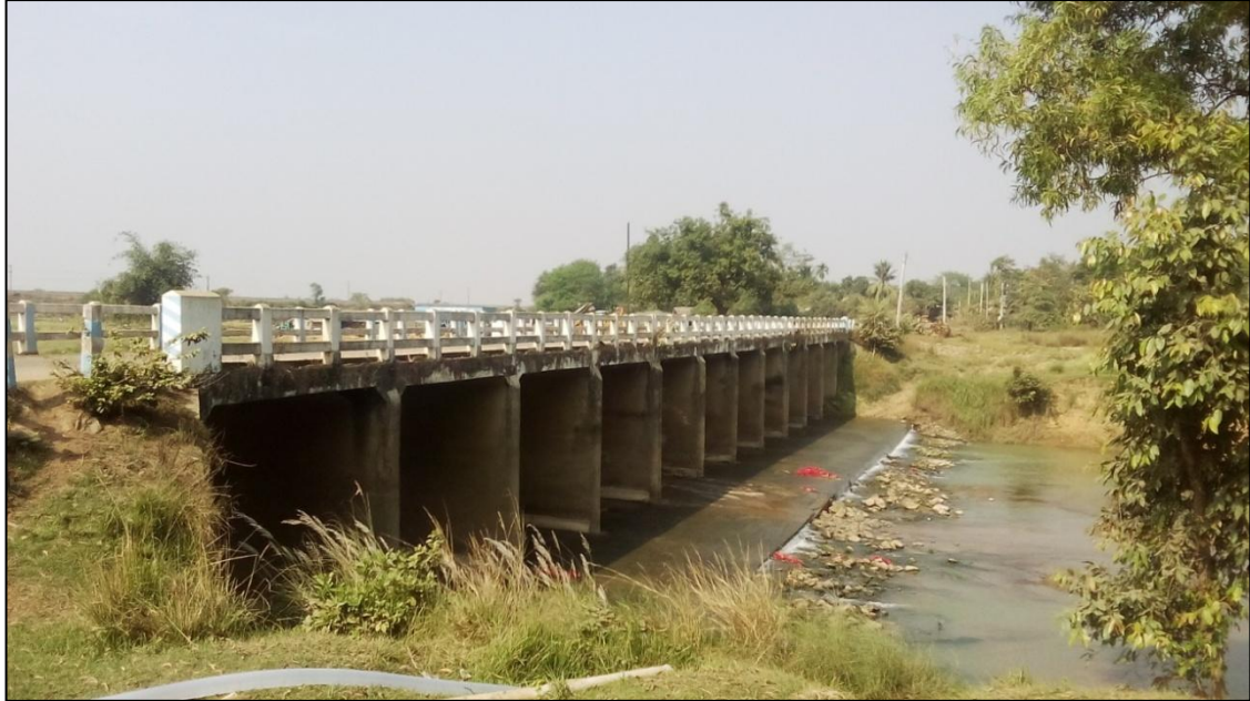
Figure 26- RCC Bridge (Chainage- 90.630 km)
