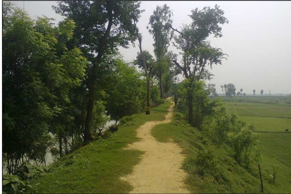
Figure 58- Embankment near the bank side near Ibrahimpur (Chainage -18.900 km)
