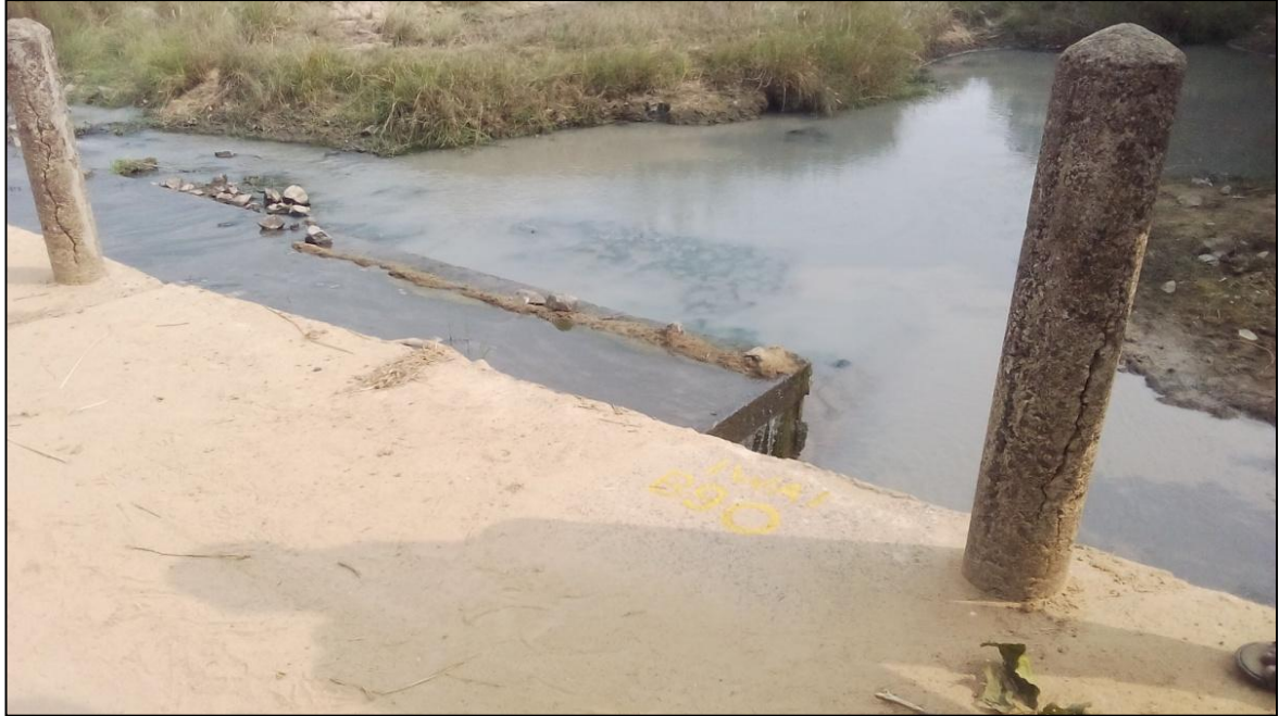
Figure 30- Check Dam (Chainage- 119.200 km)
