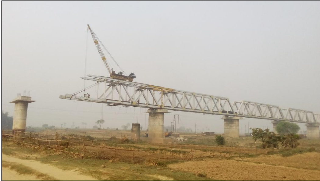
Figure 18- Under-construction Rail Bridge (Chainage- 65.755 km)
