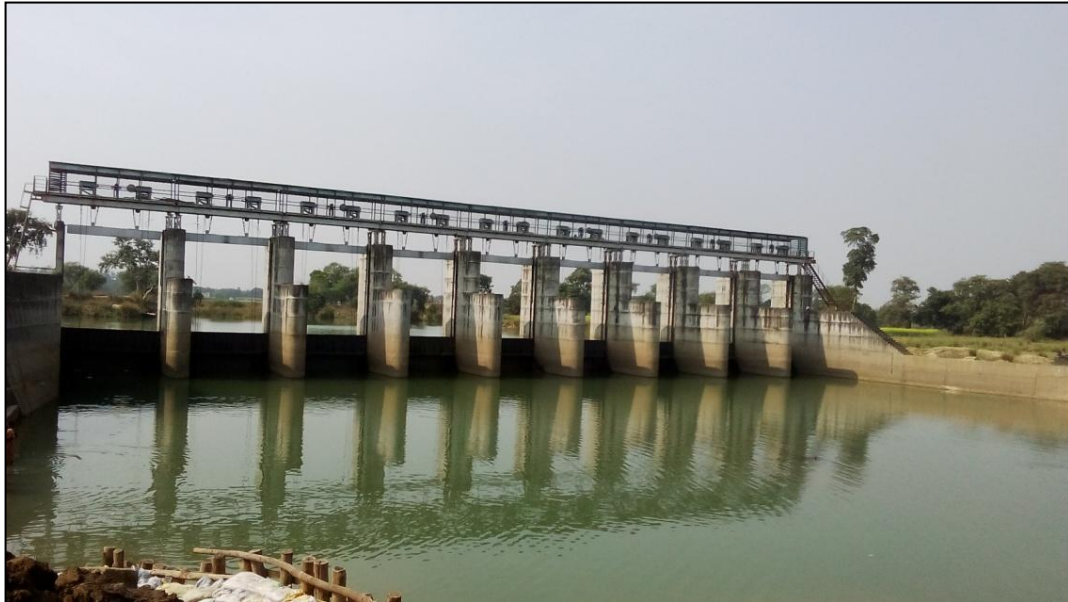
Figure 14- Check Dam (Chainage-51.400 km)
