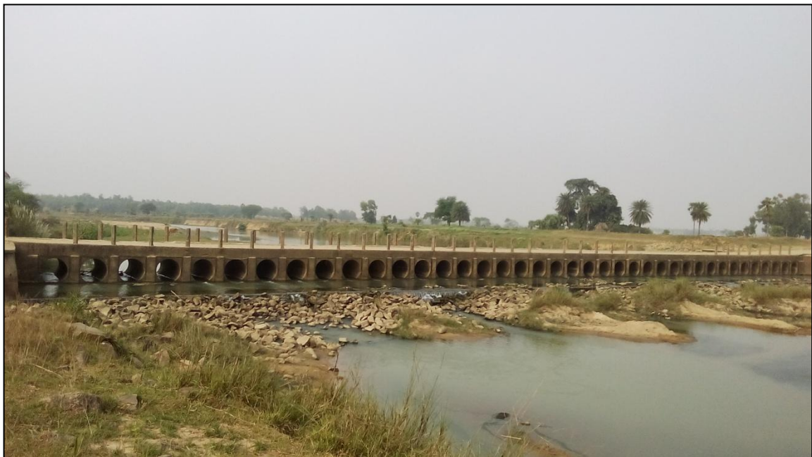
Figure 27- Check Dam (Chainage- 98.950 km)
