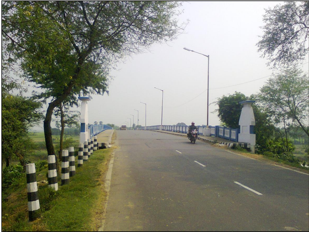
Figure 11- RCC Bridge (Chainage- 38.050 km)
