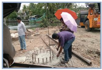
Piling work by Govt. of Kerala – Construction of lock gate at Thrikkunnapuzha in NW-3
