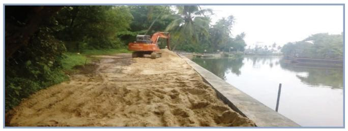
Dredging, widening of narrow canals & bank protection works in Edappallikotta - Kollam stretch of NW-3
