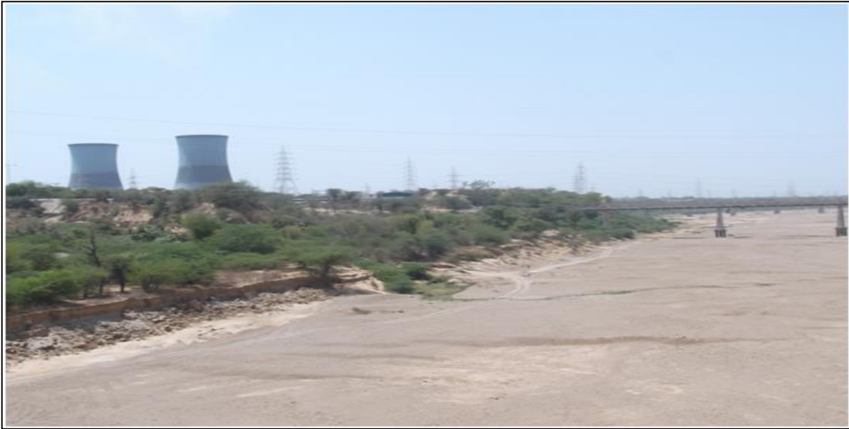
Figure 25: Condition of river stretch for Fly ash transport, Thermal power plant site.
