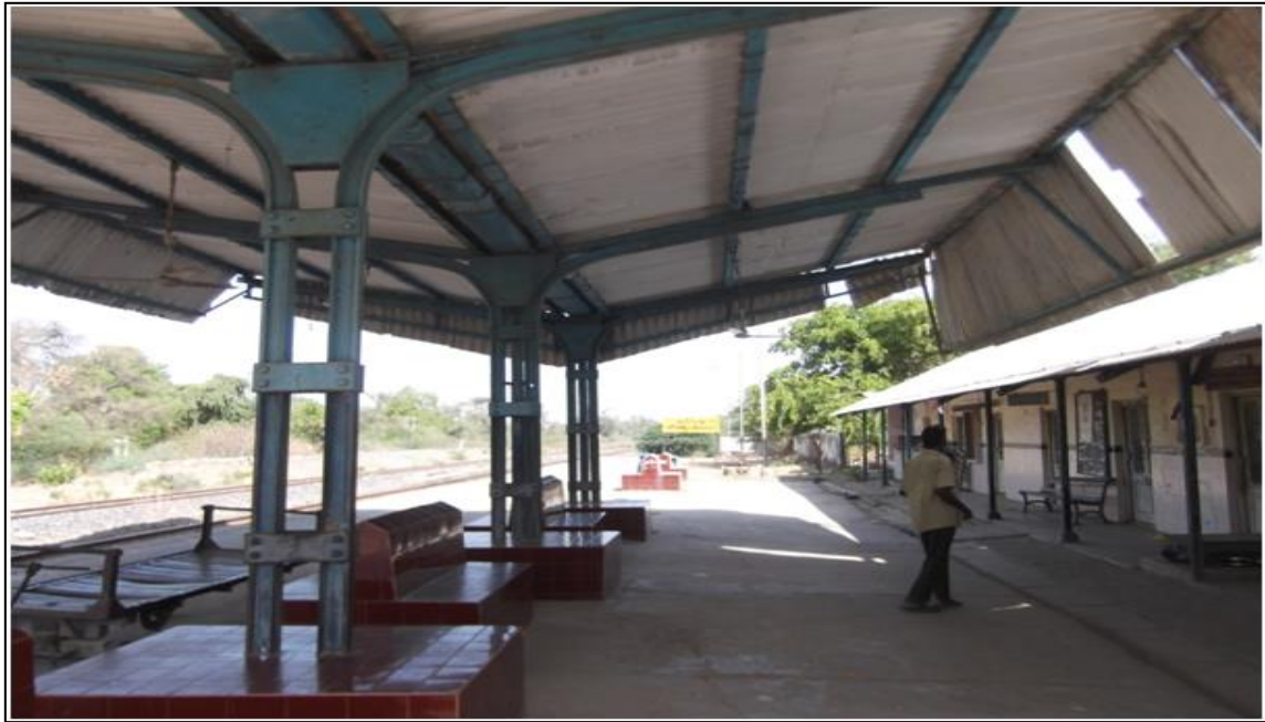
Figure 28: Prantinj Railway Station
