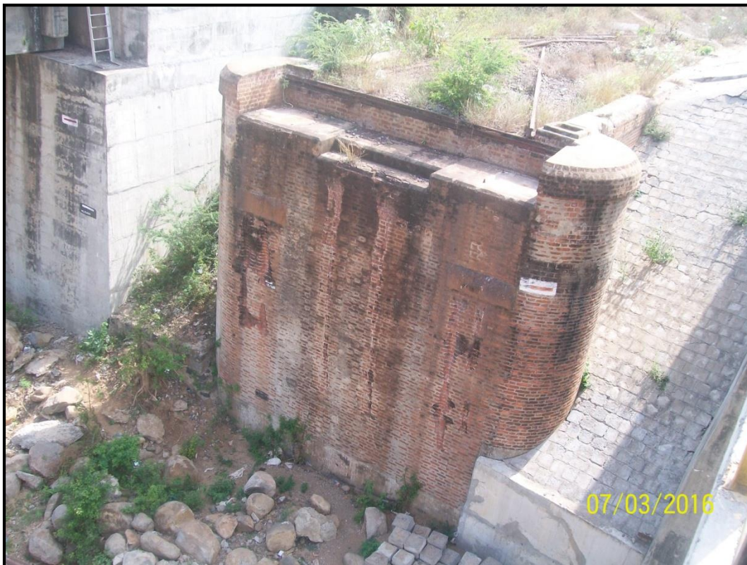
12: View of HFL mark on Padalam Railway Bridge at Chainage 26.6 km
