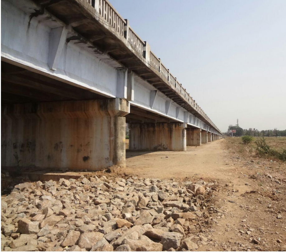
35: Rail Bridge VC 7m and HC 20m at Chainage 141 km
