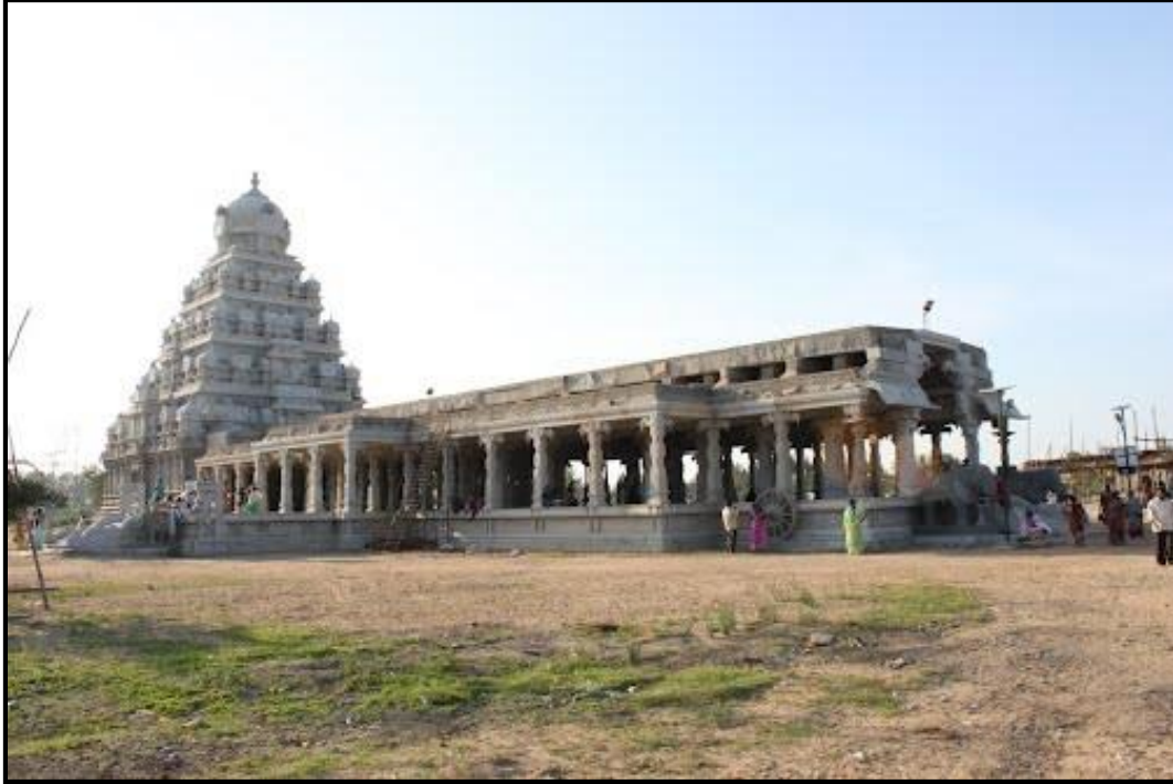
21: KANCHIMANDAPAM TEMPLE at chainage 85.7 km
