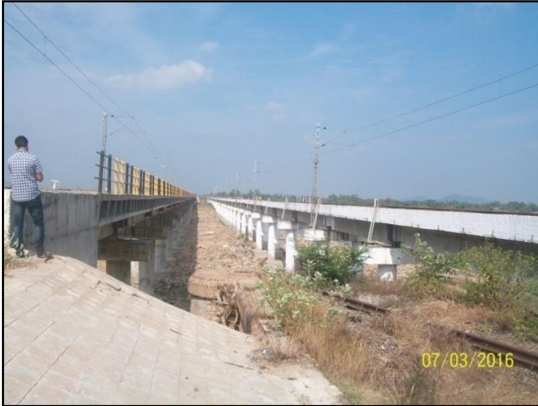
11: Padalam Railway Bridge Length-700m, VC-8.5m, HC-18m at Chainage 26.6 km
