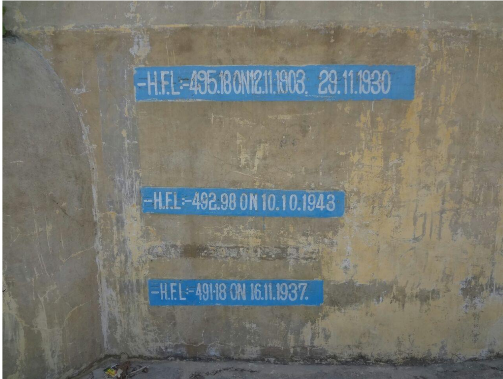
25: View of Old Dam (not in use) towards South and HFL values at Chainage 108.6
