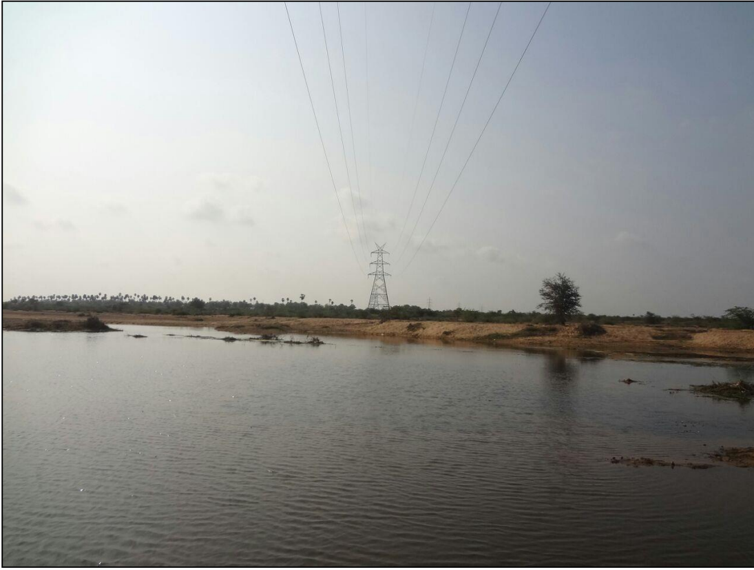
19: HT line VC-18m, HC-300m at Chainage 72.7 km
