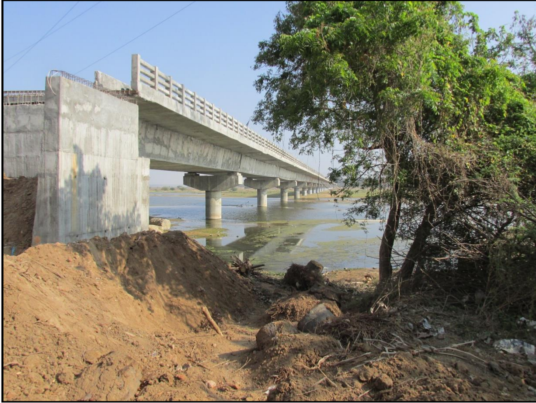
31: SIPCOT, BHEL BRIDGE (BRIDGE UNDER CONSTRUCTION) at Ch 120.7 km
