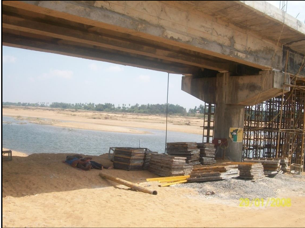
7: Idaiyathur under Construction Bridge at chainage 15.9 km
