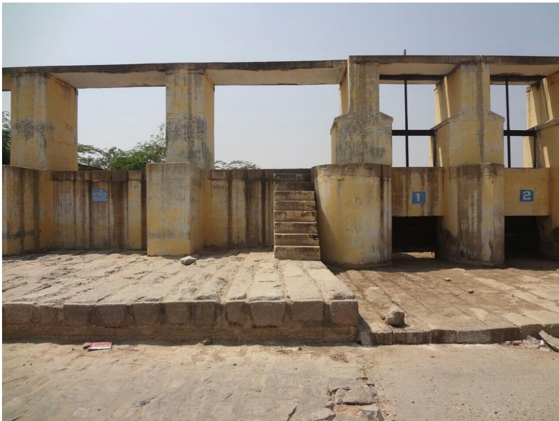
26: View of Old Dam at Chainage 108.6 km
