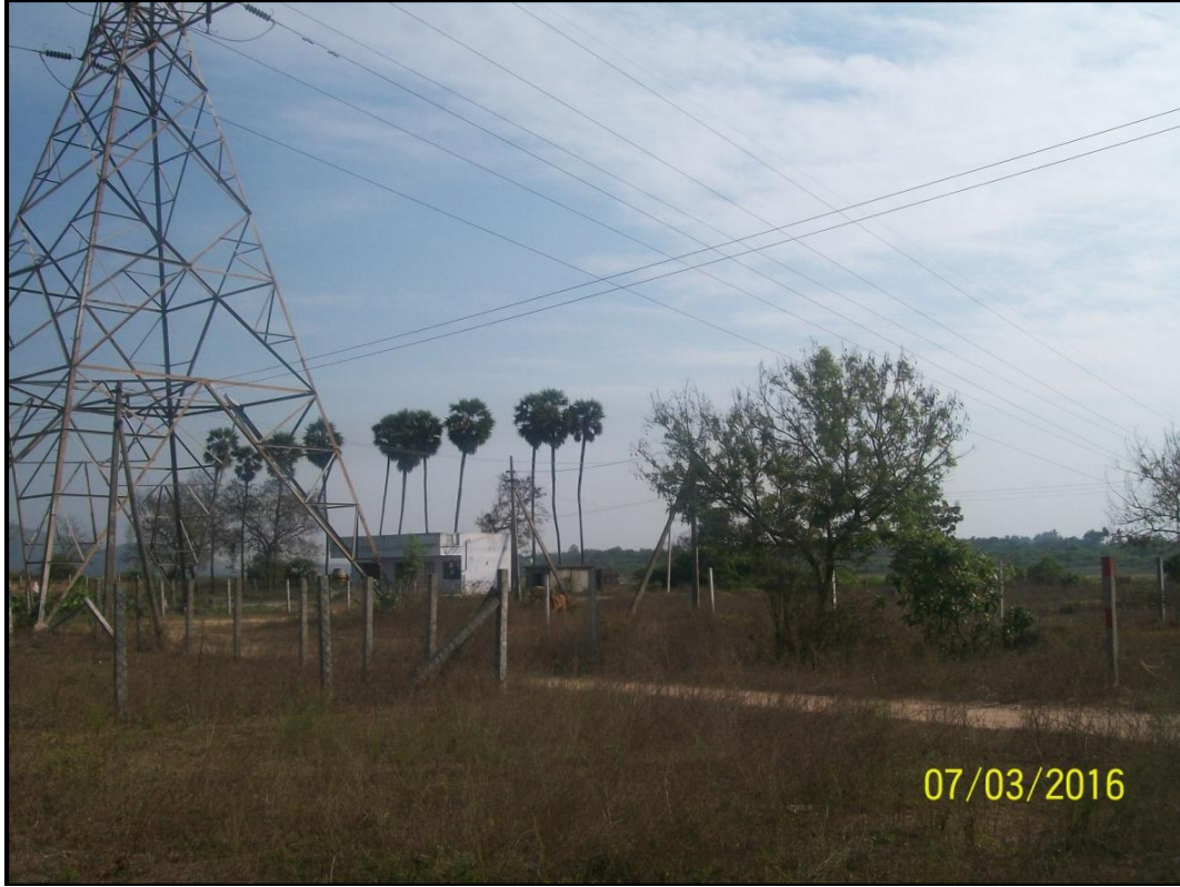
15: HT Line crossing Palar River at Chainage 40.3 km
