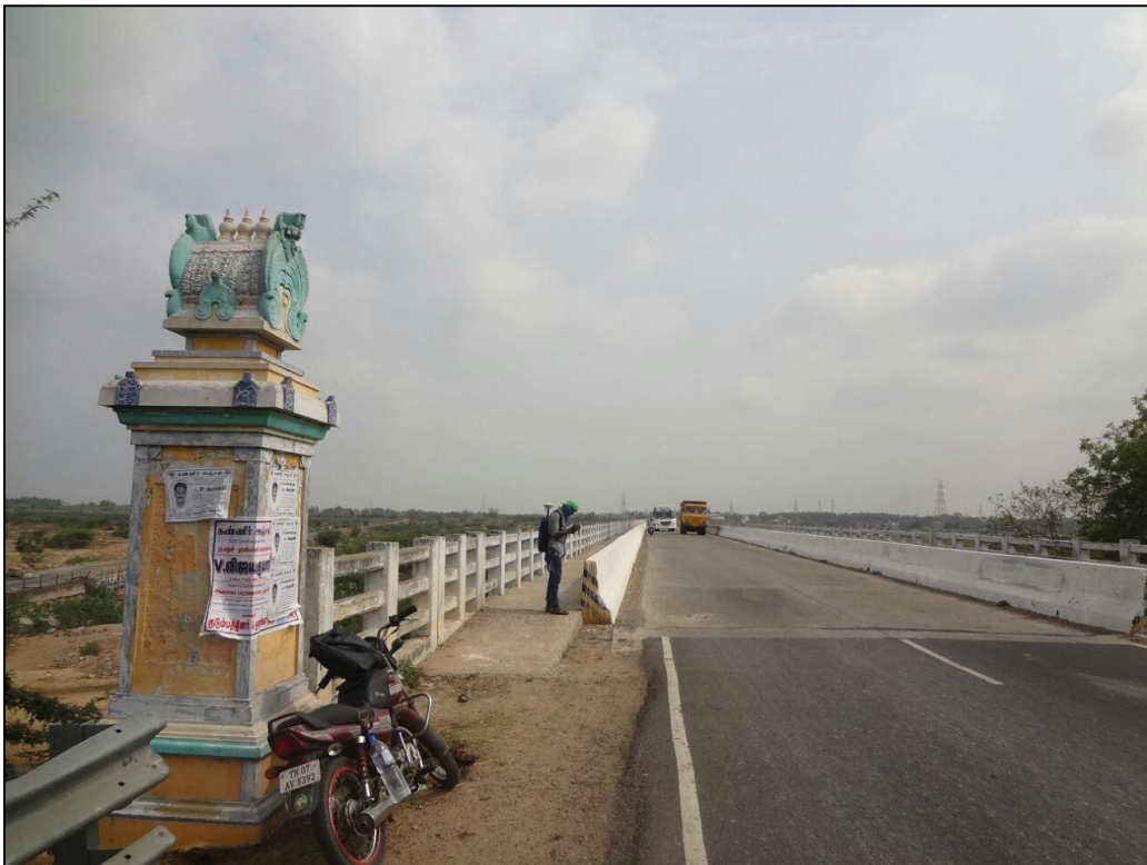
20: Arcot - Kanchipuram Bridge VC-5m, HC-12m and Length -700m at Chainage 73.5 km
