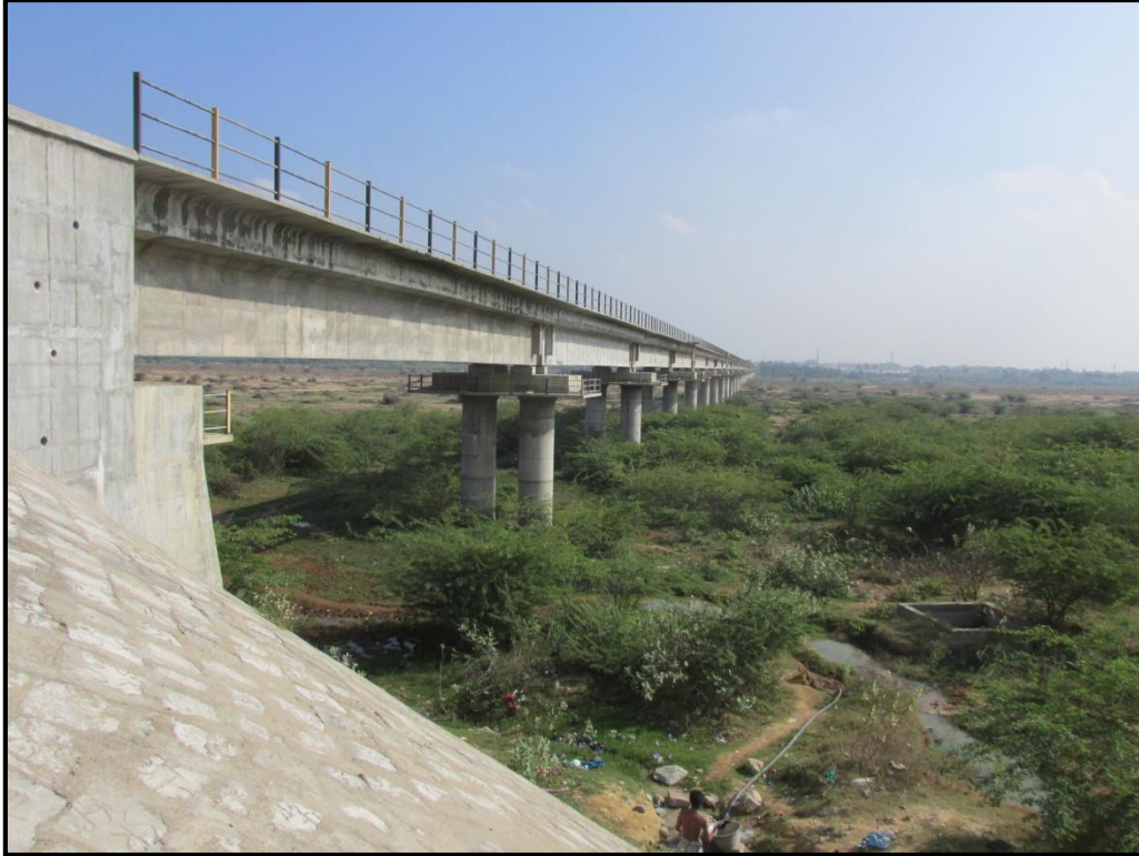
29: Railway Bridge at Chainage 116.4 km
