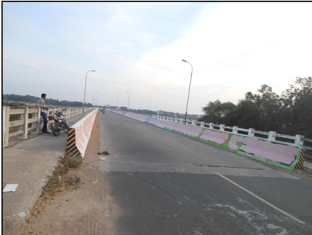
18: UTHRAMEERUR BRIDGE at chainage 69.6 km
