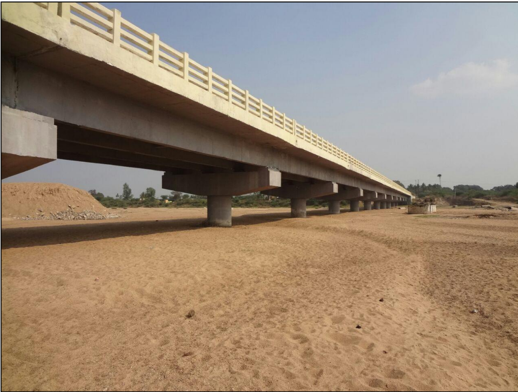
22: Pudur Mamandur Bridge extn, VC-4m, HC-15m, Length-300m at Ch 93.0 km
