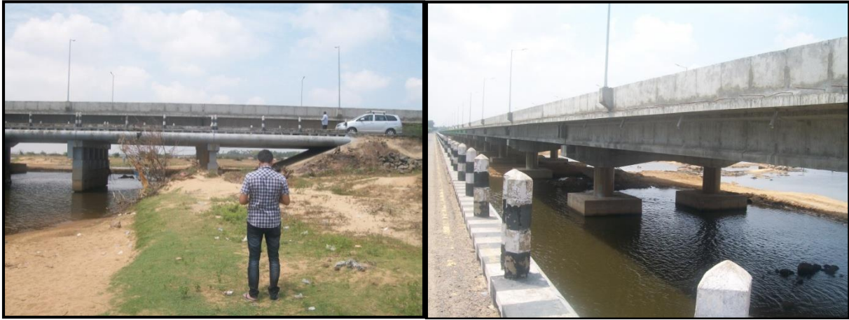
3: Pudupattinam Road Bridge at Chainage 3.5 km
