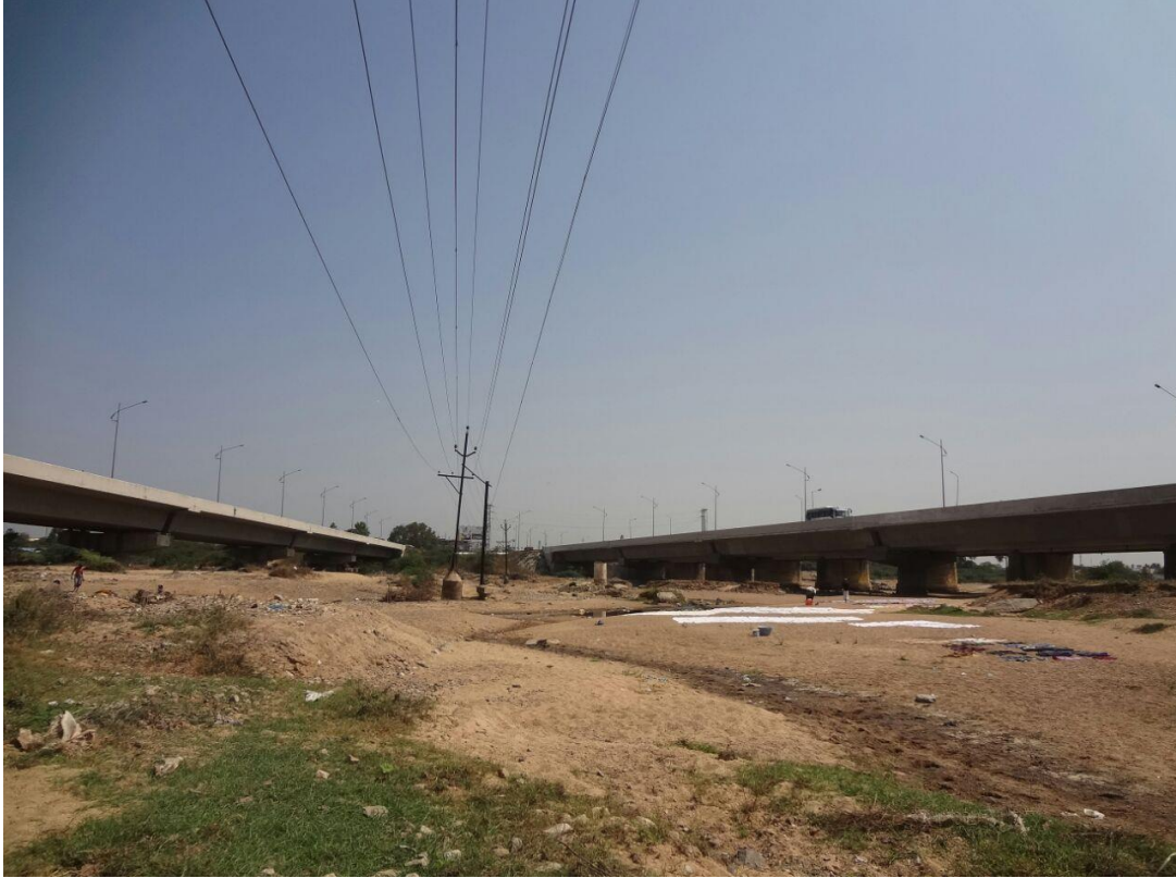
27: Electric line and two bridges (Arcot-Ranipet) at Chainage 115.2 km
