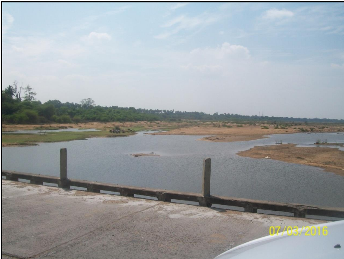
10: Vallipuram Bridge HC 2.5m VC 3m at chainage 19.6 km
