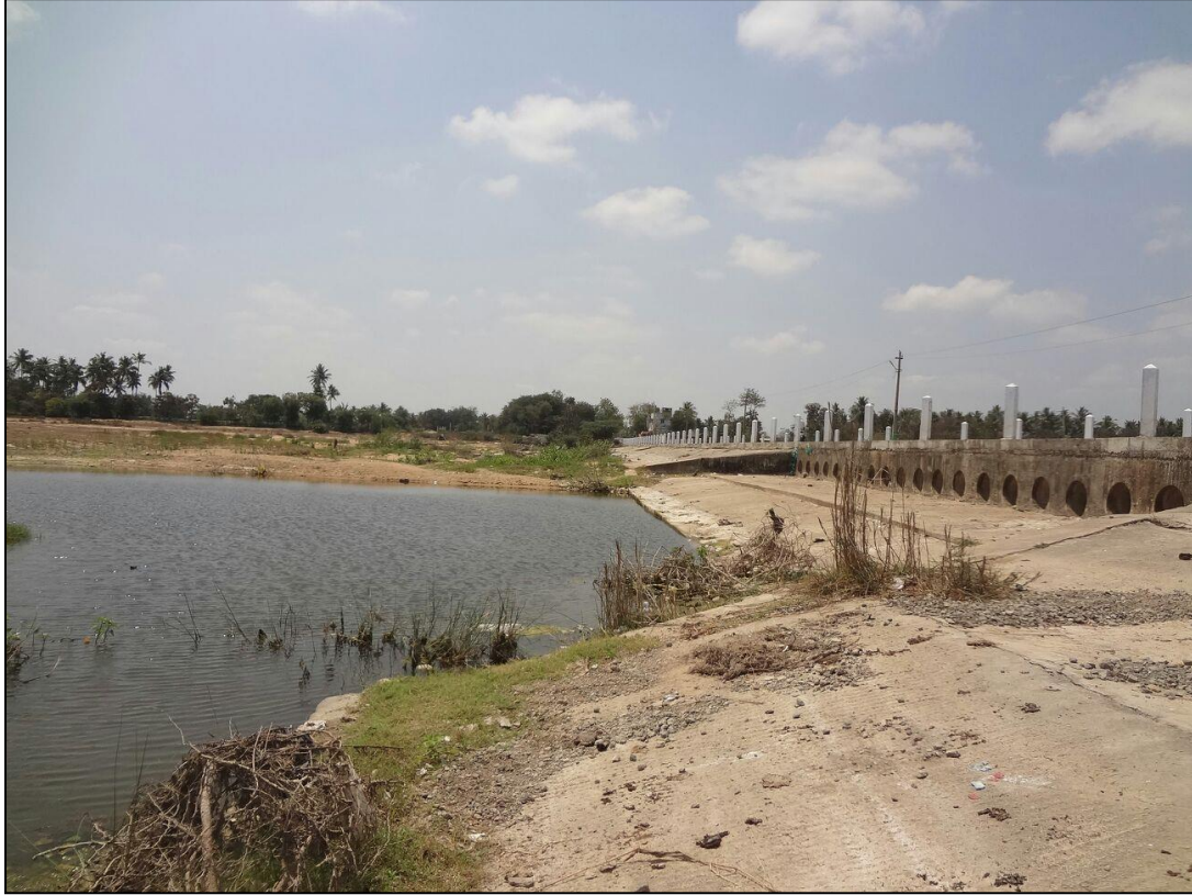
17: Palar Walazabad ground bridge at Chainage 57.9 km
