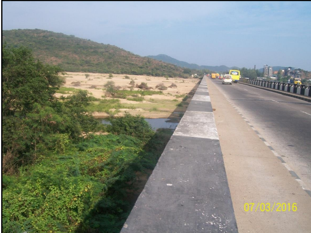
14: CHENGALPATTU BRIDGE (Chennai-Trichi Highway) at chainage 33.7 km
