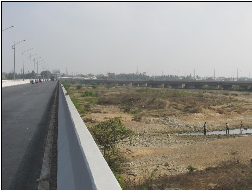
28: Two bridges (Arcot-Ranipet) at Chainage 115.2 km
