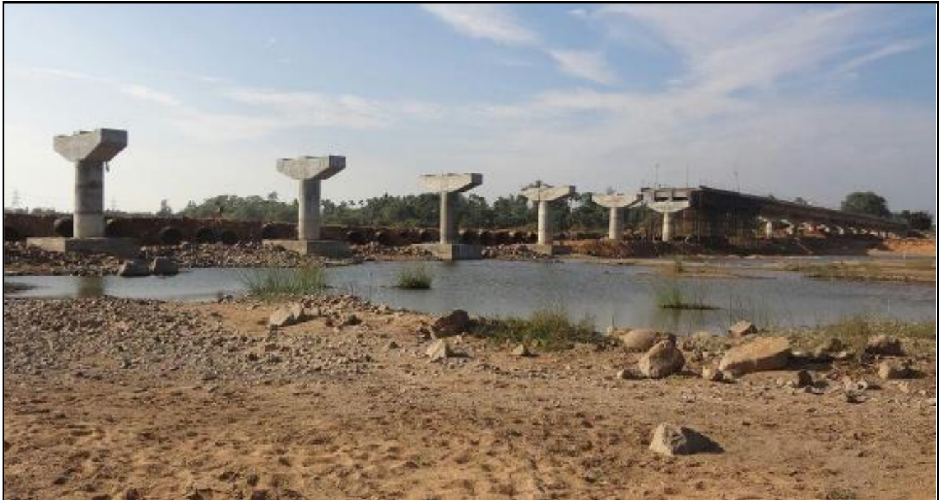
6: Idaiyathur under Construction Bridge at chainage 15.9 km
