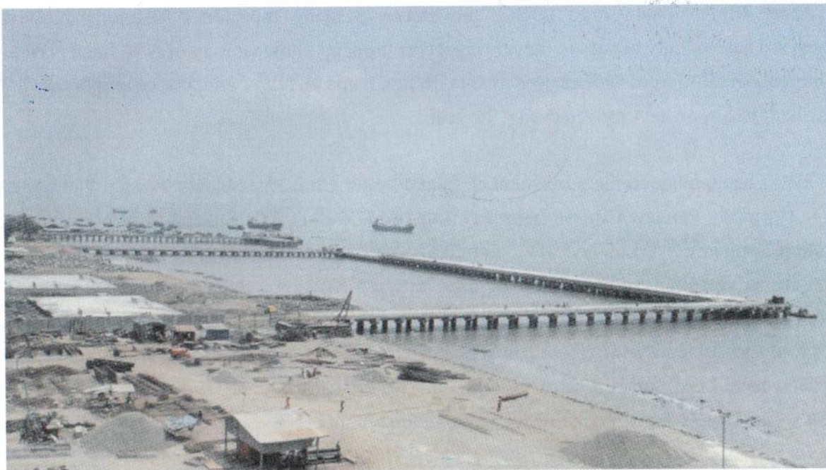
Construction of Port & backup facilities at Sittwe
