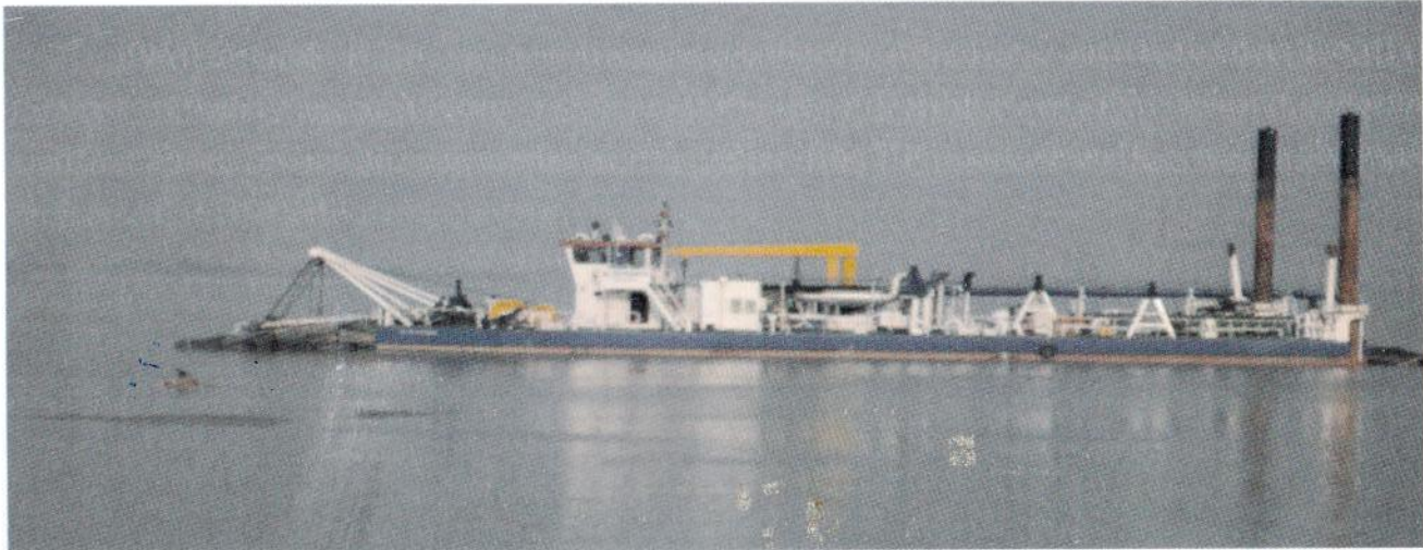
A picture of Dredging executed on National Waterway-1
