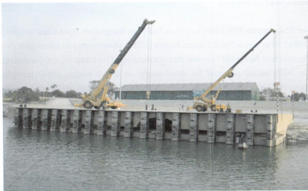
RCC low level jetty at Pandu Port with Mechanical Handling Equipment
