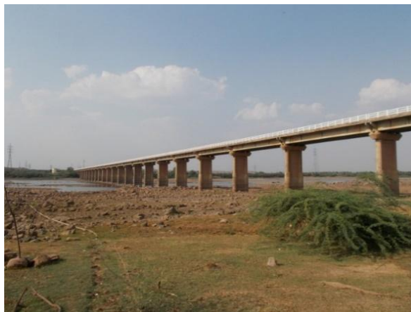
Figure 137 - Highway Bridge at Almatti village (ch. 571.58km)
