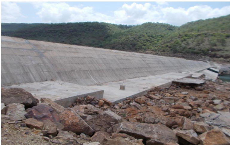
Figure 44 - Check Dam at Srisailem
