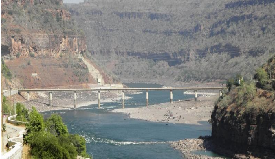
Figure 45 - Bridge near Sundipenta (Ch.142.02km)
