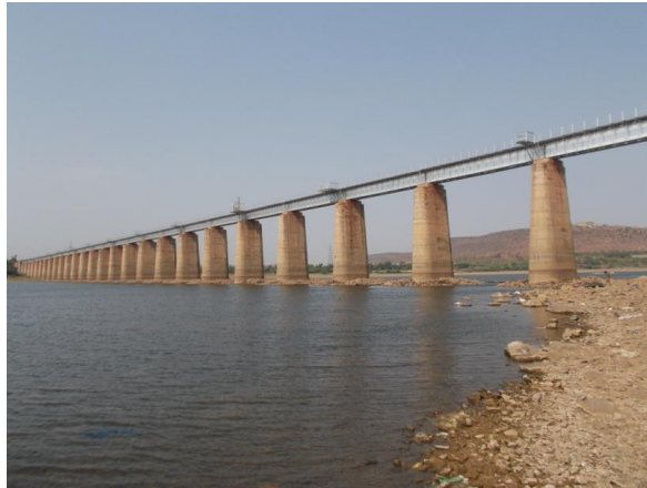
Figure 136 - Korthi Kohar Railway Bridge (ch. 571.85km)
