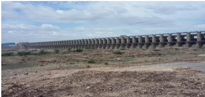
Figure 74 - Priyadarshini Jurala Dam/Barrage (ch. 325.57km)
