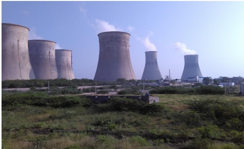
Figure 84 - Raichur Thermal Power plant (ch. 367.61km)
