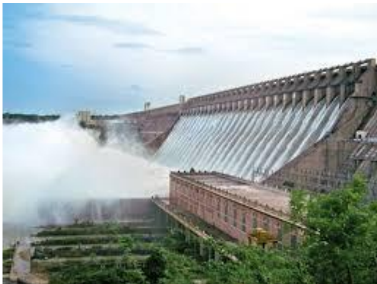
Figure 159 - Nagarjuna Sagar Dam (ch. 44.40km)
