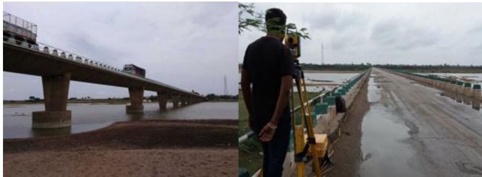
Figure 100 - Golden Bridge (ch. 433.54km)
