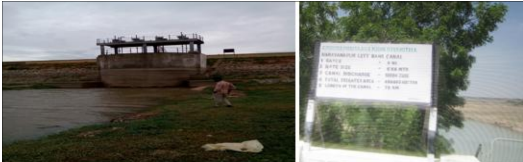
Figure 119 - Narayanapur Left Bank canal
