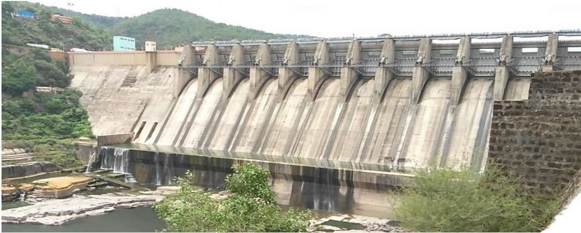
Figure 47 - Srisailem dam (ch. 143.97km)
