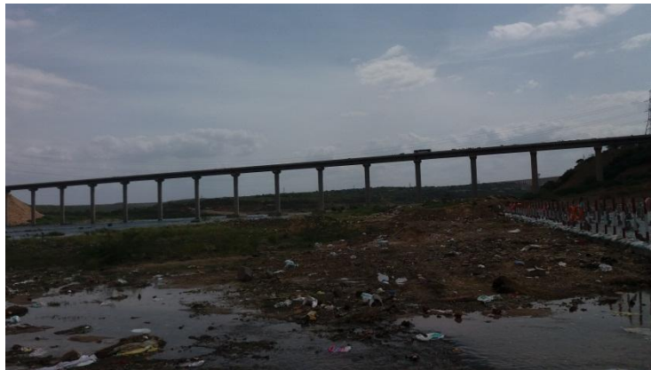
Figure 23 - Highway Bridge Downstream of Krishna River (ch. 42.41km)
