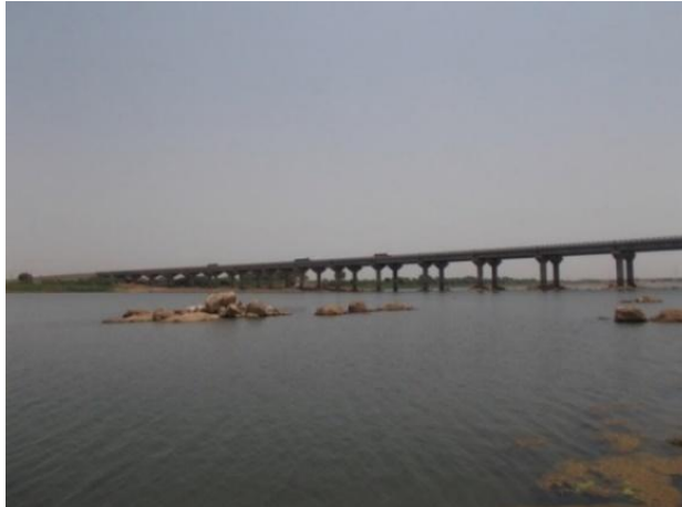
Figure 129 - Sholapur Mangalore Highway Bridge (ch. 569.60km)
