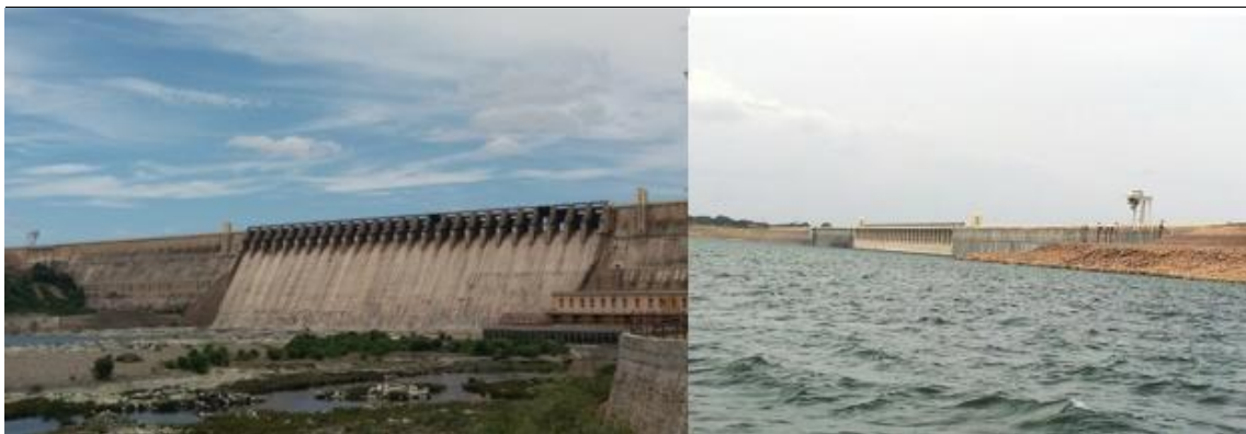
Figure 25 - Nagarjuna Sagar Dam (ch. 44.40km)
