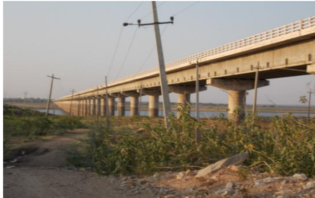
Figure 138 - Korthi Kolhar Bridge at Rolli (ch 597.52km)
