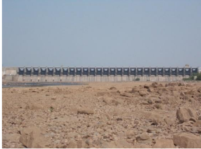
Figure 133 - Almatti Dam (ch. 573.48km)
