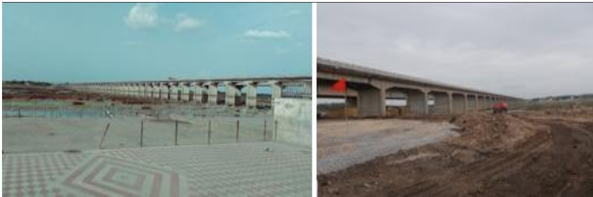
Figure 67 - Bichhupalli Highway Bridge (ch. 292.78km)
