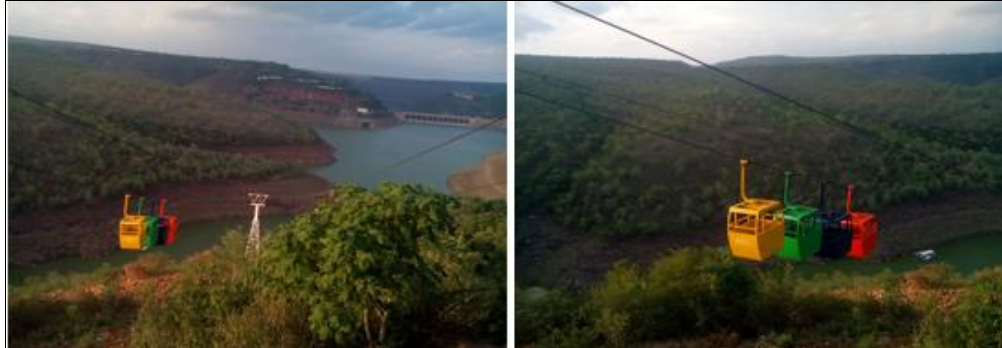
Figure 48 - Ropeway Services at Srisailam
