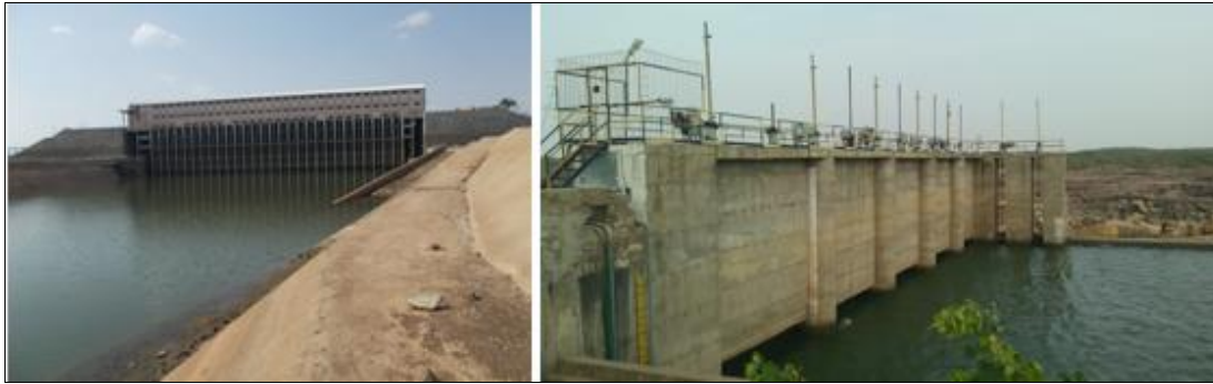
Figure 115 - Geddamari weir house near Geddamari village (ch. 484.14km)
