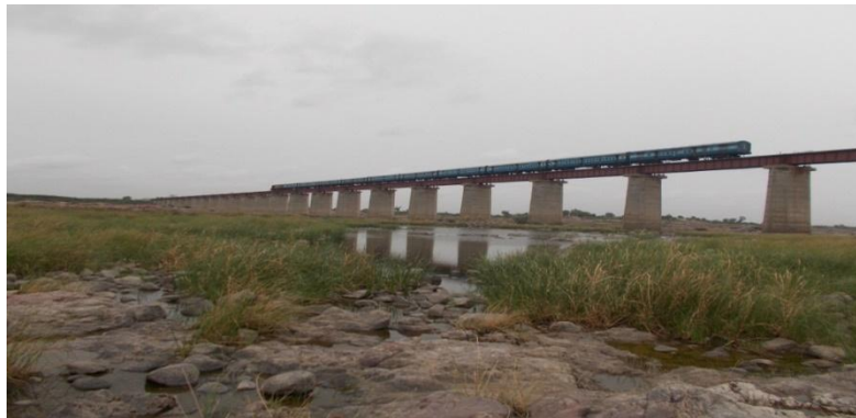
Figure 72 - Yenkampeta Railway Bridge (ch. 307.63km)
