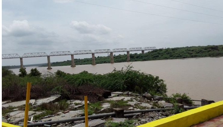
Figure 16 - Pondugula Railway Bridge (ch. 0.43km)
