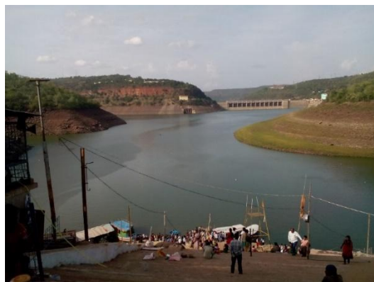
Figure 50 - Local Ferry Ghat at Srisailam (ch. 145.10km)
