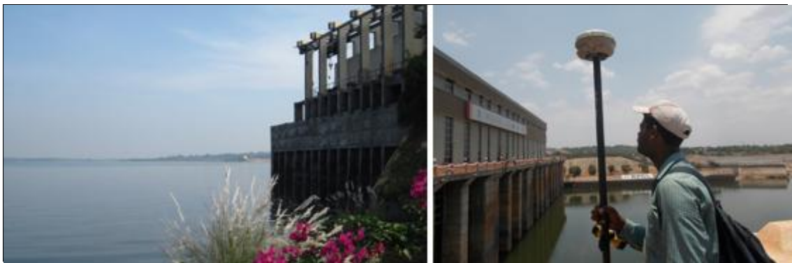
Figure 135 - Hydro Electric Power plant at Almatti Dam right bank (ch. 573.48km)
