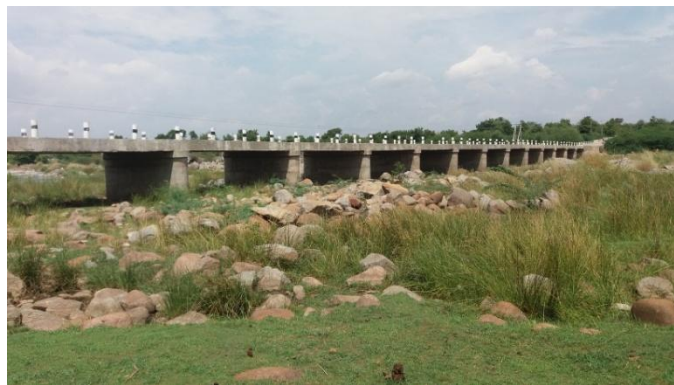
Figure 114 - Bridge near Hanchinal village (ch. 490.96km)
