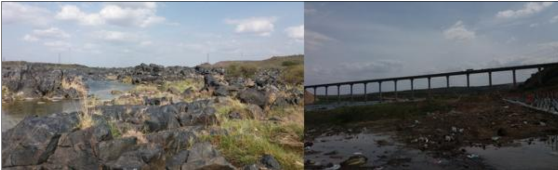
Figure 28 - Downstream of Nagarjuna Sagar Dam presence of rock boulders and dry patches
