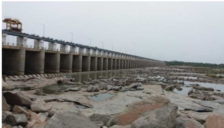
Figure 92 - Gugal Bridge cum Barrage (ch. 395.09km)
