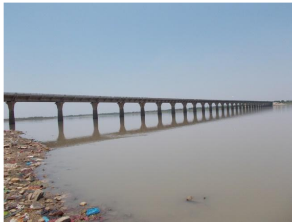
Figure 128 - Dhannur Bridge (ch.541.49km)
