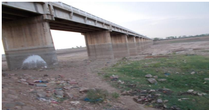
Figure 143 - Galgali Bridge (ch. 636.2km)
