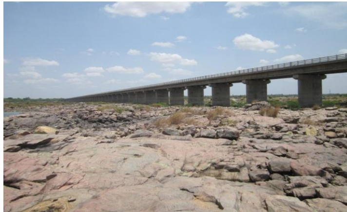
Figure 111 - Bridge downstream of Narayanapur Dam (ch. 510.00km)
