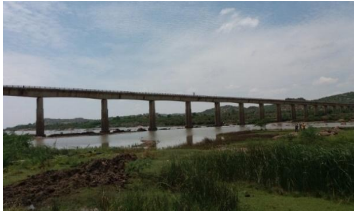
Figure 105 - Tintani Bridge (ch. 469.32km)
