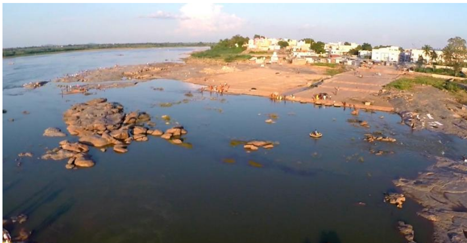
Figure 64 - Convergence point of Tungabhadra and Krishna (ch. 260.64km)
