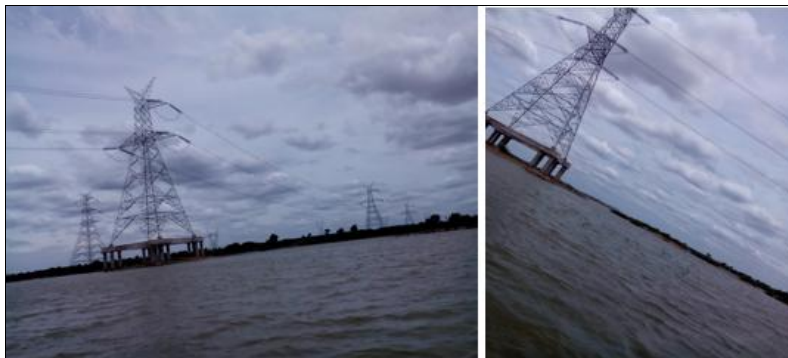
Figure 95 - High-Tension Line at Koppara village upon Krishna River (ch. 408.206km)
