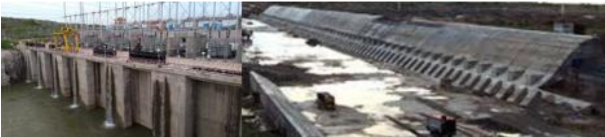
Figure 73 - Lower Jurala Hydroelectric power project (ch.317.43km)
