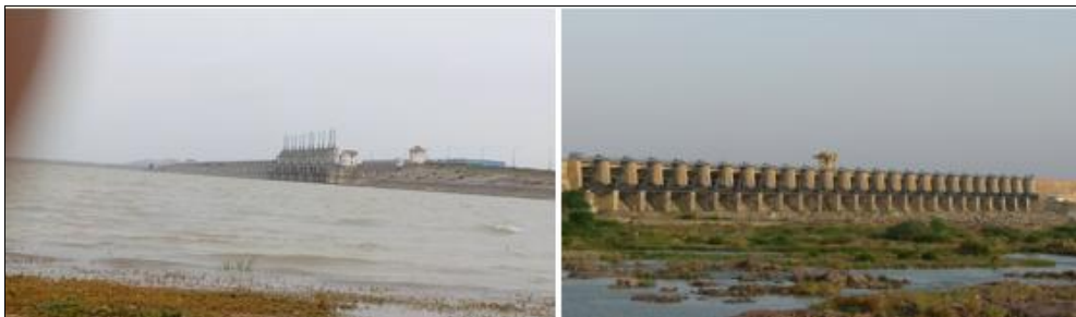
Figure 118 - Narayanapur Dam (ch.510.84km)
