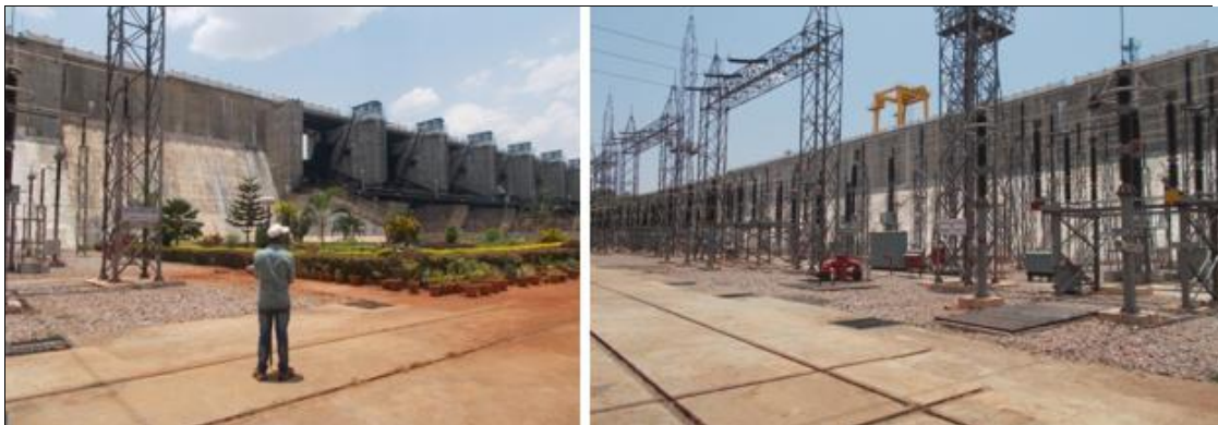
Figure 134 - Almatti dam powerhouse (ch. 572.88km)
