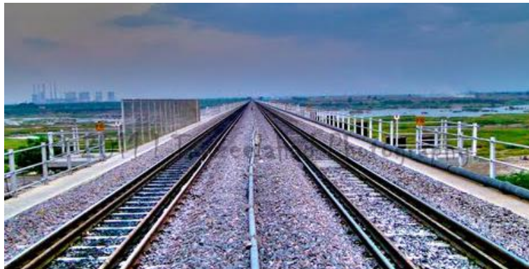
Figure 86 - Railway Bridge at Shakti Nagar (ch. 370.85km)
