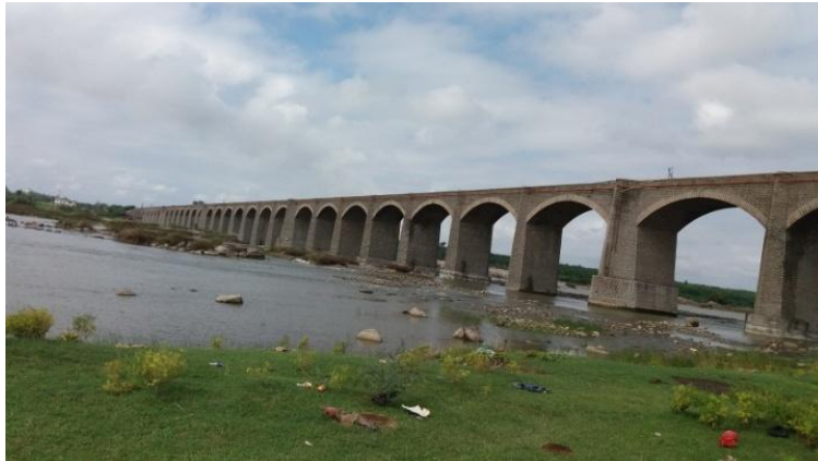
Figure 85 - Raichur Hyderabad Highway Bridge at Deosugur (ch. 367.34km)
