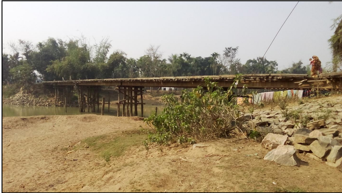
Figure 16- Wooden Bridge (Chainage – 26.031 km)
