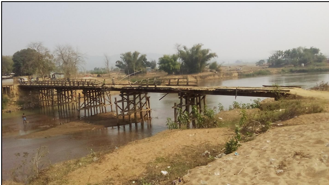
Figure 15- Wooden Bridge (Chainage – 22.019 km)
