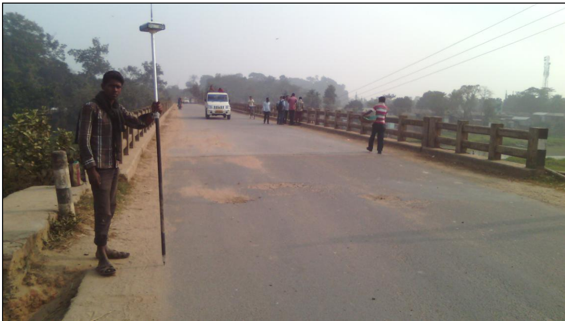
Figure 12- RCC Bridge (Chainage-18.675 km)
