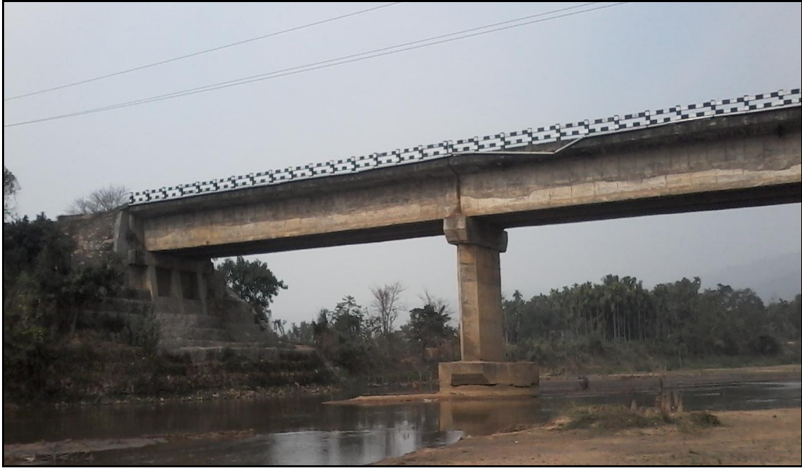
Figure 19 - RCC Bridge (Chainage-31.652 km)
