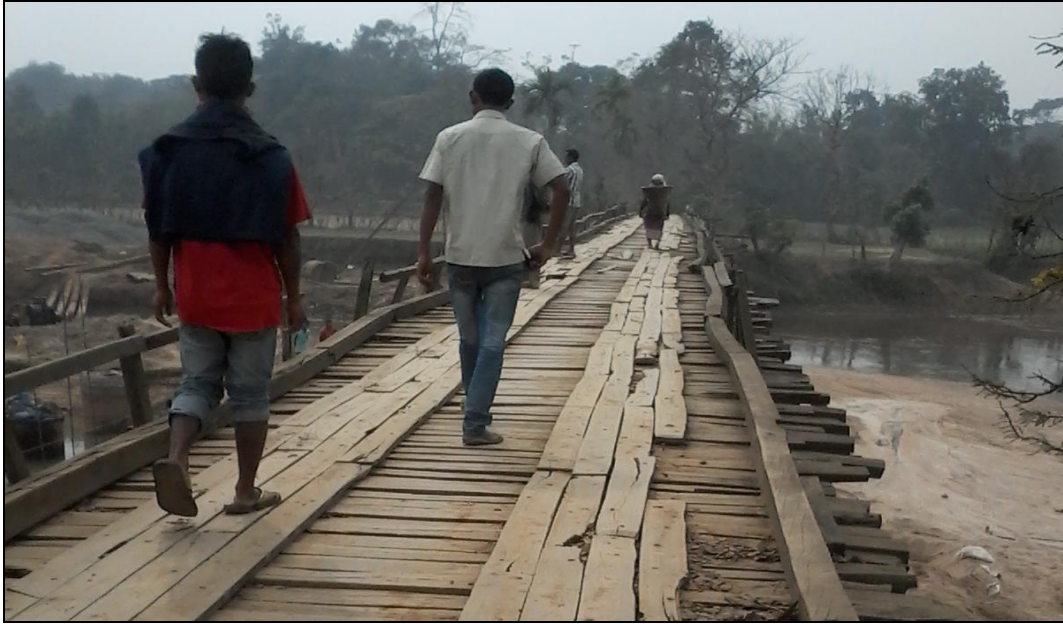
Figure 8- Wooden Bridge (Chainage – 0.700 km)
