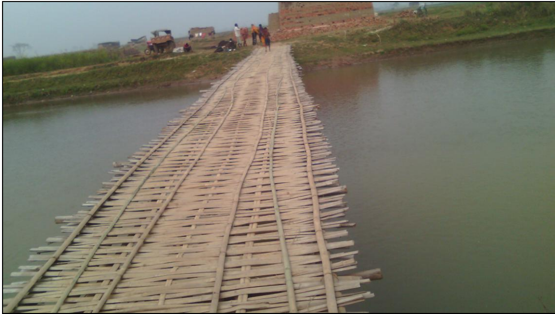
Figure 11-Bamboo Bridge (Chainage- 13.621 km)
