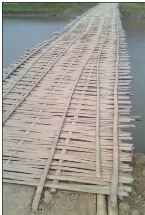
Figure 17- Bamboo Bridge (Chainage-24.320 km)
