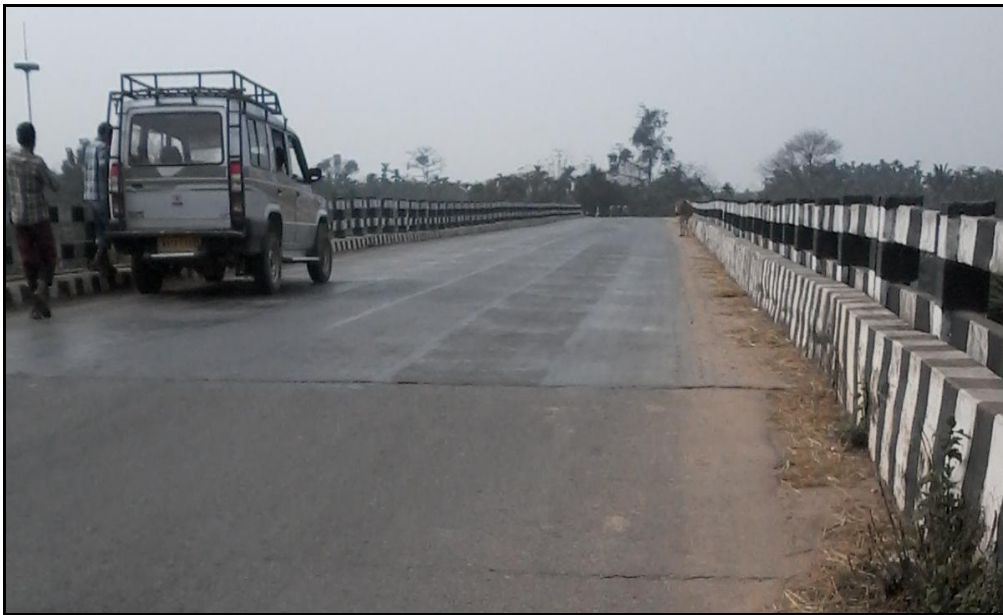
Figure 6- RCC Bridge (Chainage -0.000 km)
