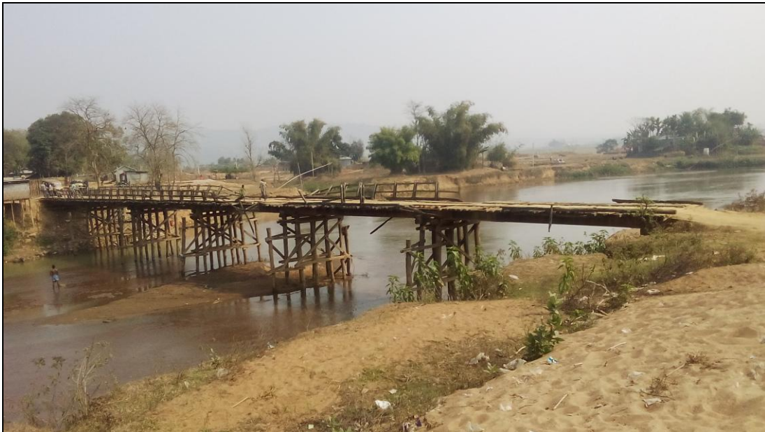
Figure 9- Wooden Bridge (Chainage- 0.966 km)
