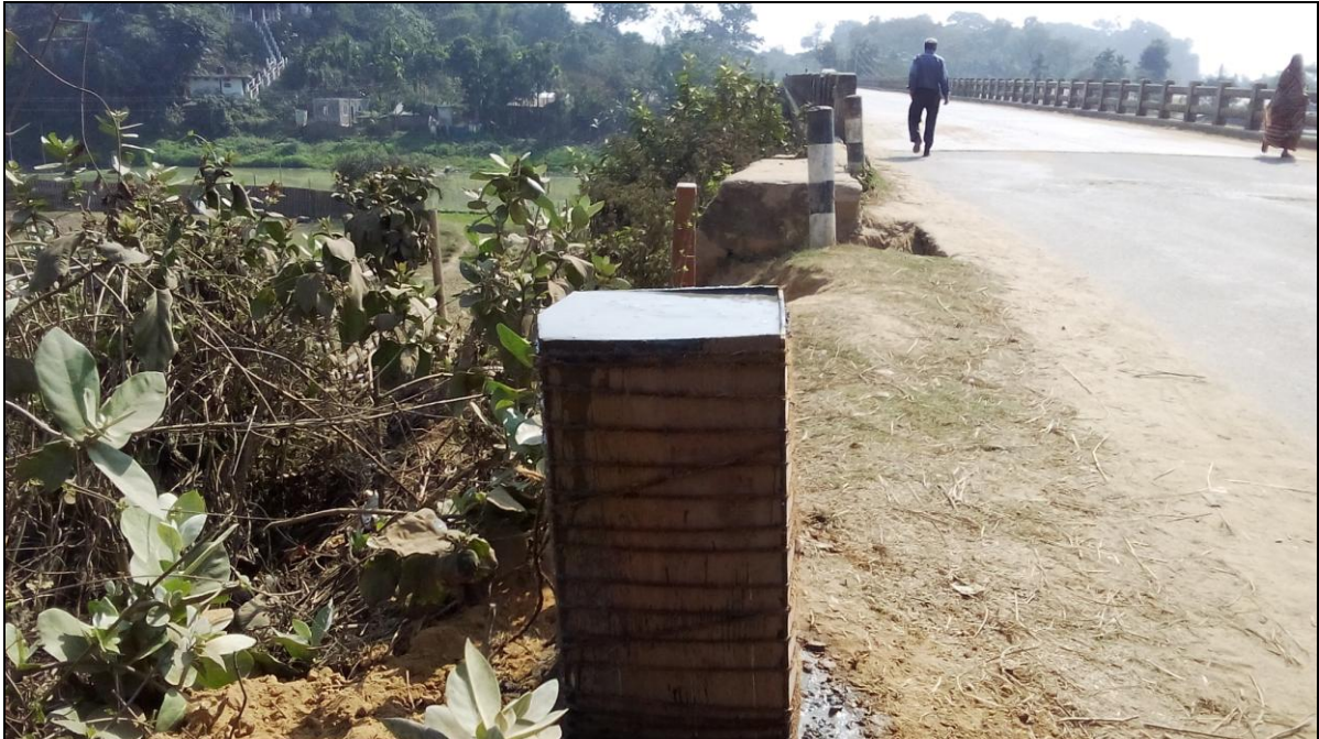
Figure 20- RCC Bridge (Chainage-39.580 km)
