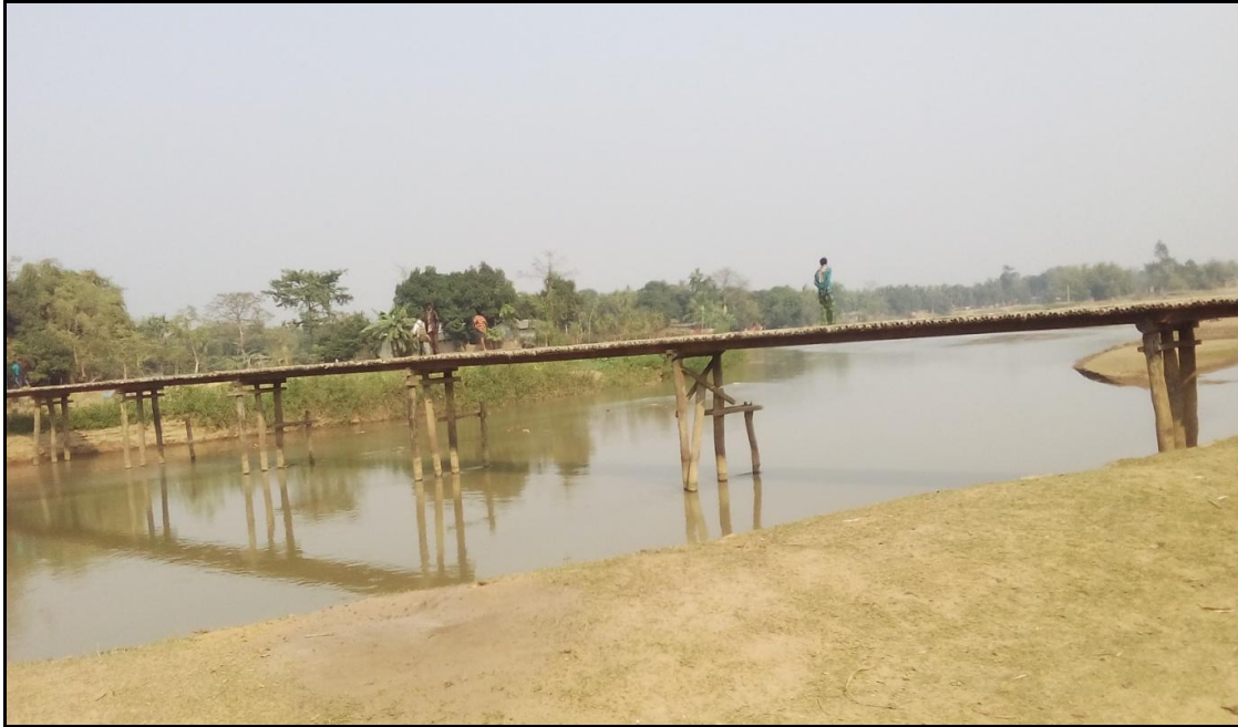
Figure 22- Wooden Bridge (Chainage- 45.590 km)
