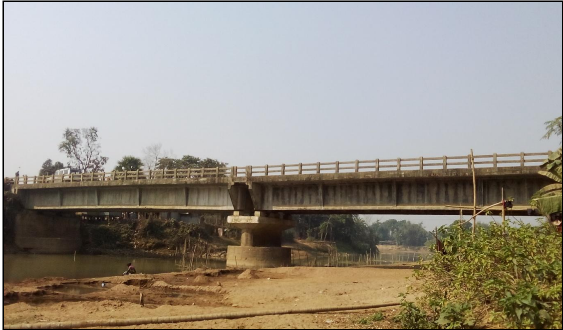
Figure 14- RCC Bridge (Chainage -27.447 km)
