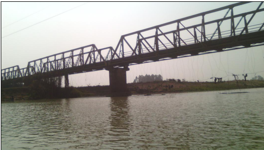
Figure 7- RCC Bridge (Chainage- 1.120 km)
