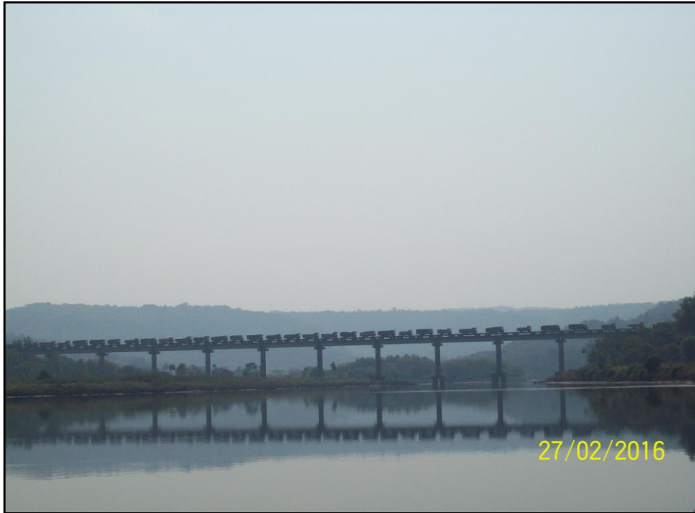
Photo 19: Railway Bridge crossing river at Ch 45.11km (17°09'51.6"N, 73°28'46.0"E)
