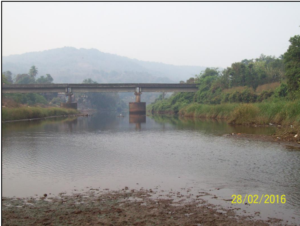
Photo 23: Asoda bridge 180 m downstream at Ch 51.98km (17°10'28.56"N, 73°32'05.51"E)
