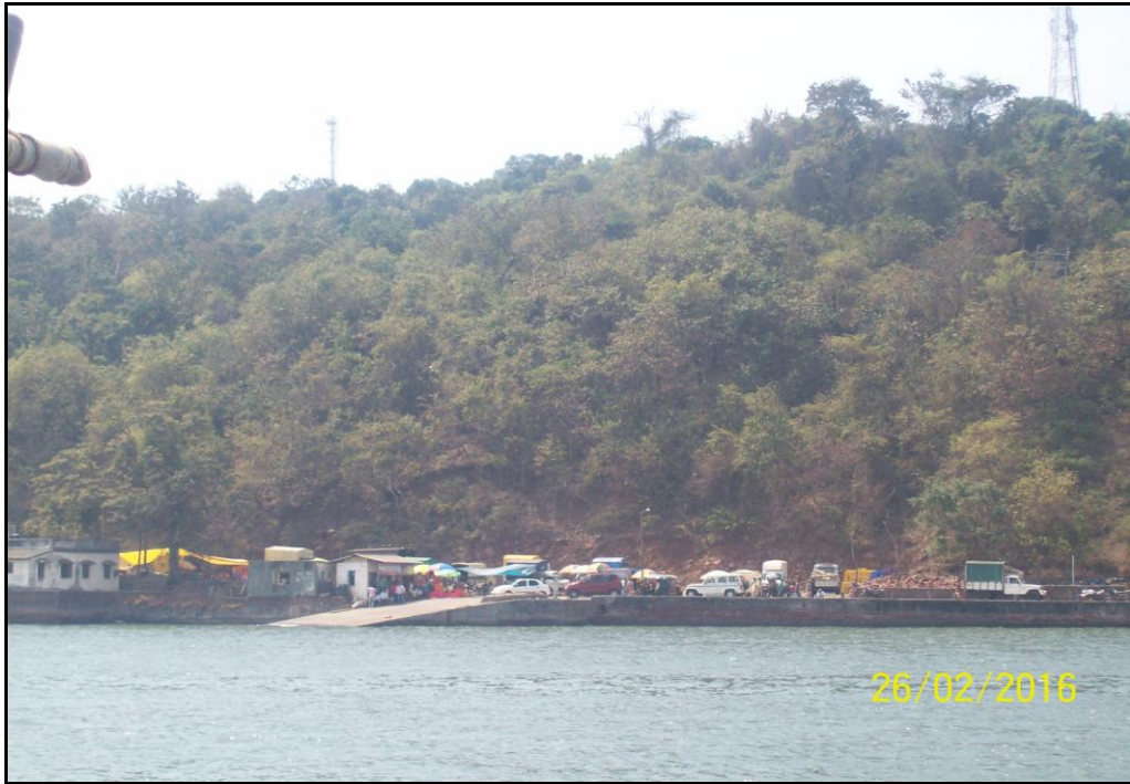
Photo 7: Jaigad Ferry Jetty on West bank of river at Ch 3.89km (17°17'31.8"N, 73°13'30.3"E)
