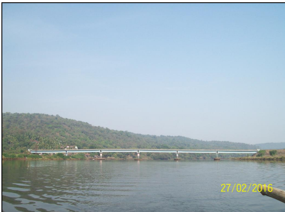
Photo 18: Phungus Road Bridge crossing river at Ch 43.95km (17°10'01.3"N, 73°28'26.7"E)
