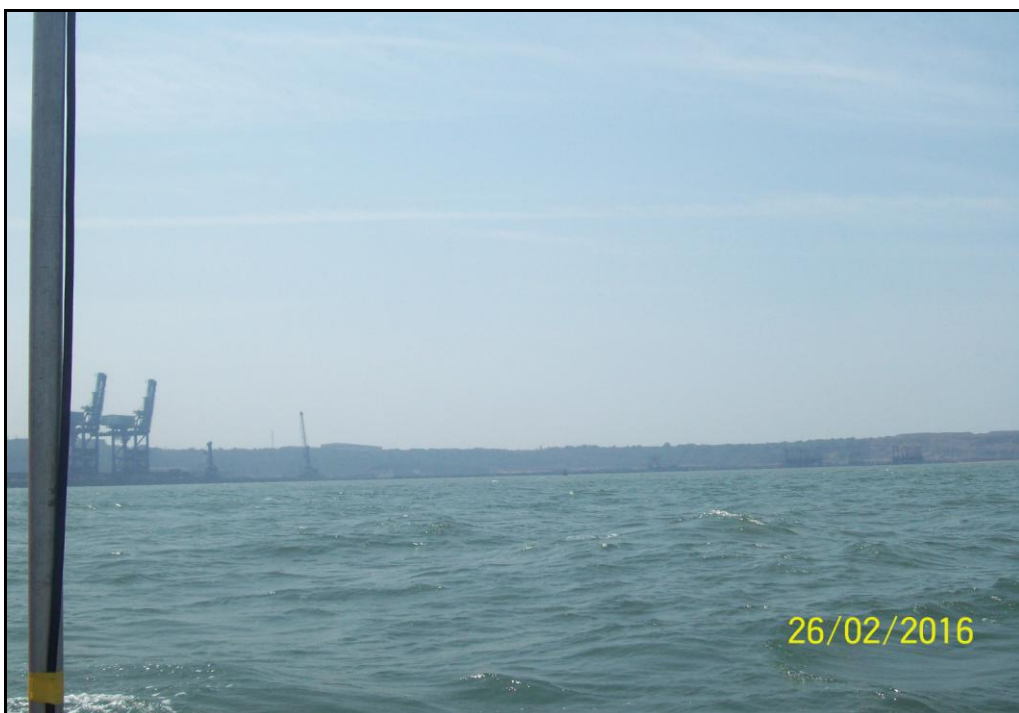
Photo 2: Jindal Port breakwater at Ch 0.67km (17°18'49.2"N, 73°12'49.4"E)
