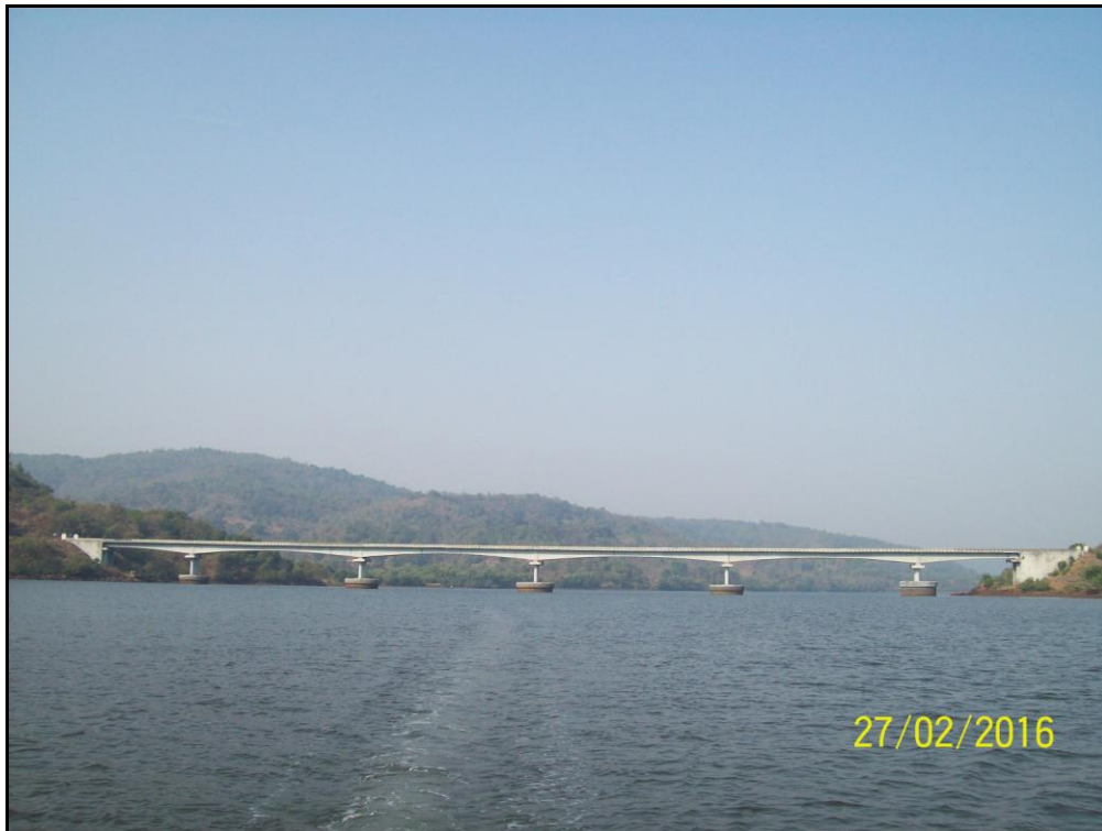
Photo 15: Bhatgaon Road Bridge from east side at Ch 34.92km (17°12'41.0"N, 73°25'12.5"E)
