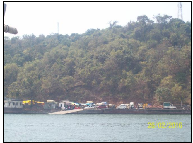
Figure 2.2: Jaigad Jetty at Chainage 3.9km
