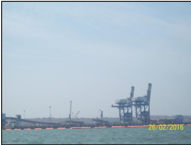
Figure 2.1: JSW Port at Chainage 3.6km
