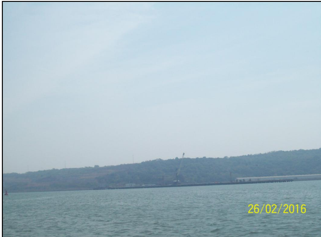
Photo 5: Chauqula Port Jetty on West bank of river at Ch 3.65km (17°17'39.7"N, 73°13'30.16"E)
