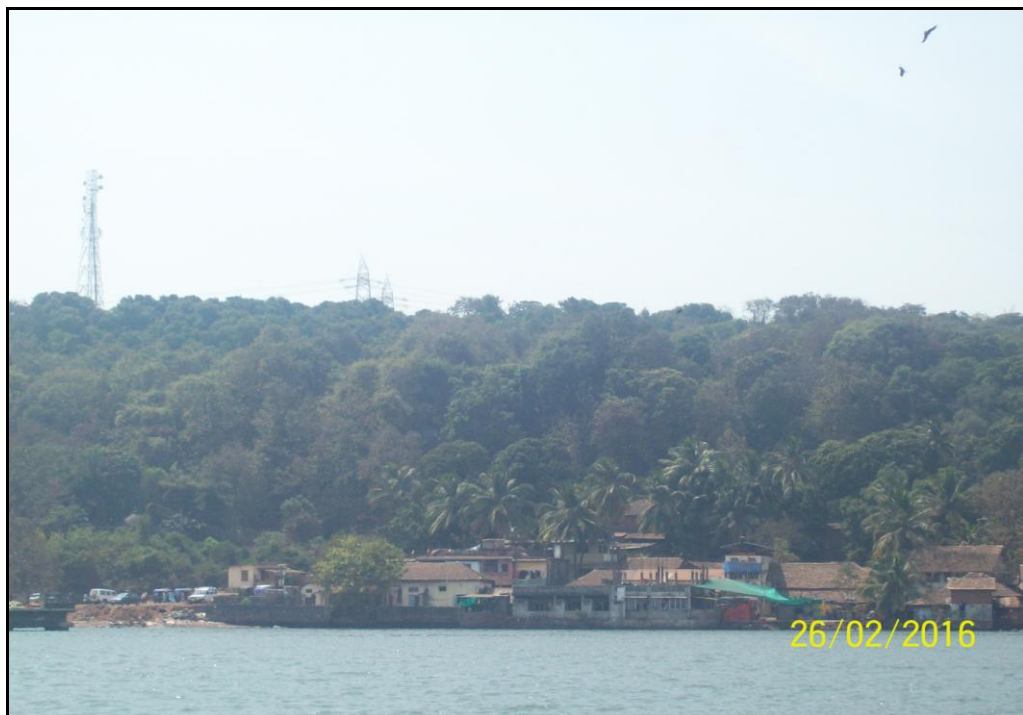
Photo 6: Jaigad Fishing Jetty on West bank of river at Ch 3.65km (17°17'39.7"N, 73°13'30.16"E)
