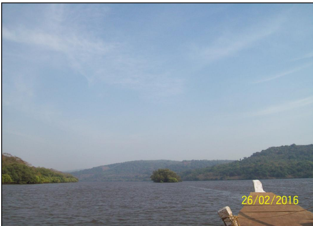
Photo 12: Shallow patch covered by Mangroves in the centre of the river at Ch 14.68km (17°16'19.4"N, 73°17'52.4"E)
