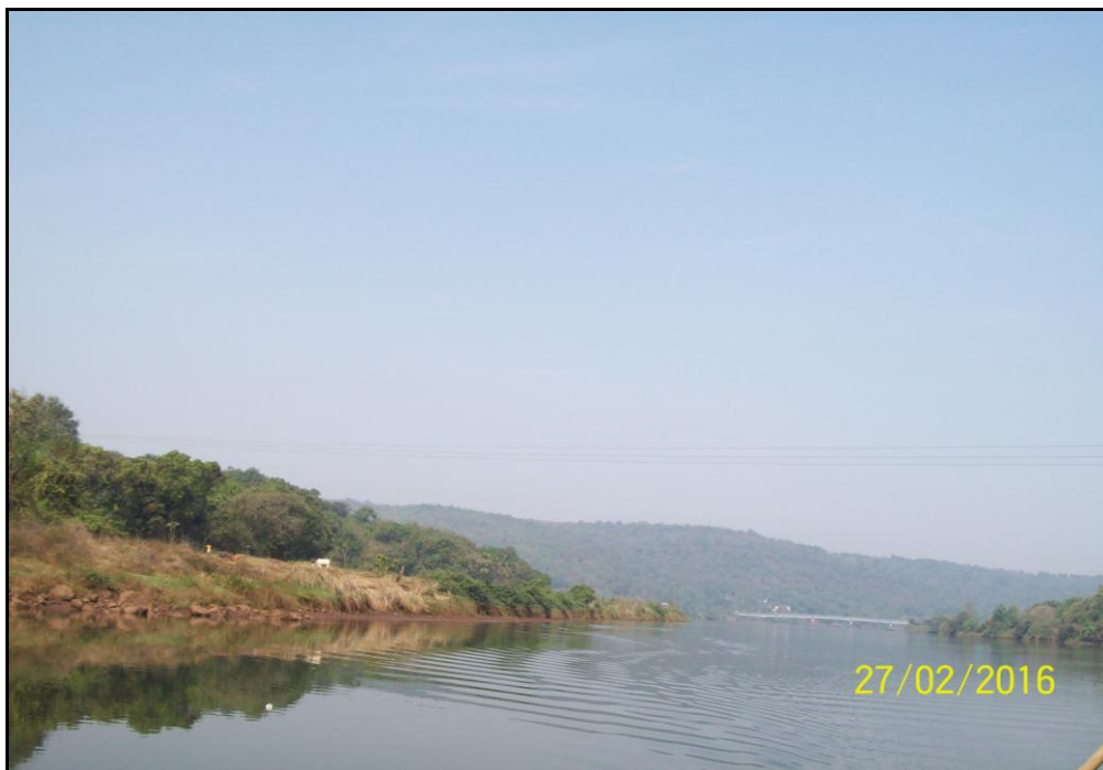
Photo 20: Electrical line crossing river at Ch 45.73km (17°09'39.0"N, 73°29'02.3"E)
