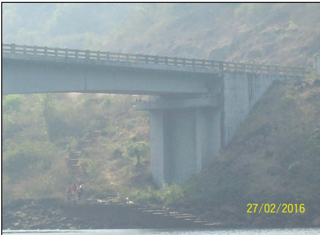
Photo 14: Bhatgaon Road Bridge at Ch 34.43km (17°12'35.3"N, 73°24'56.2"E)
