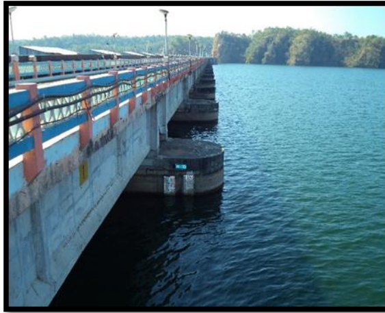
CWC Gauge at Kadana Ch 246.9 km
