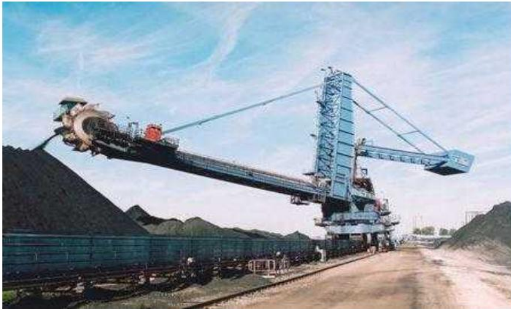
Fig No.5.8 Gantry stacker and Reclaimer
