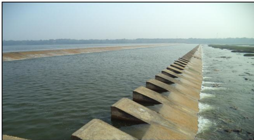
Figure 2.2 : Umeta Check Dam CH 80 km
