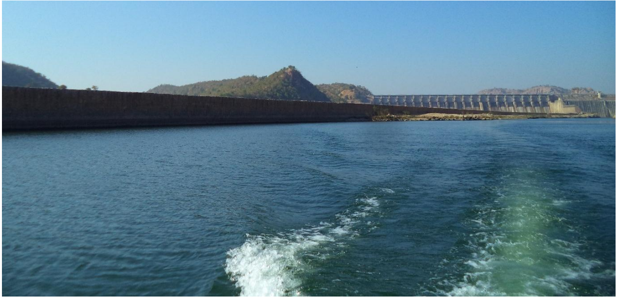
Figure 2.5 : Kadana Dam CH 246.9 km
