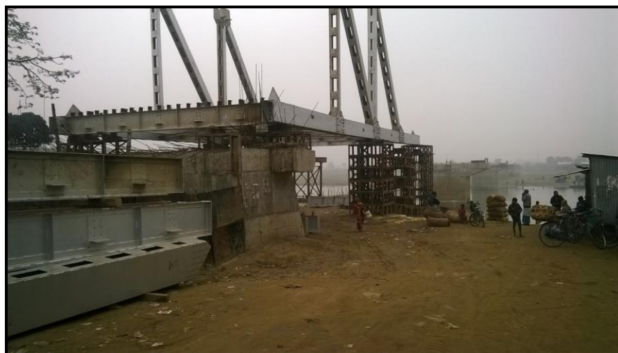
Figure 7- Under-construction Rail Bridge (Chainage -2.00 km)
