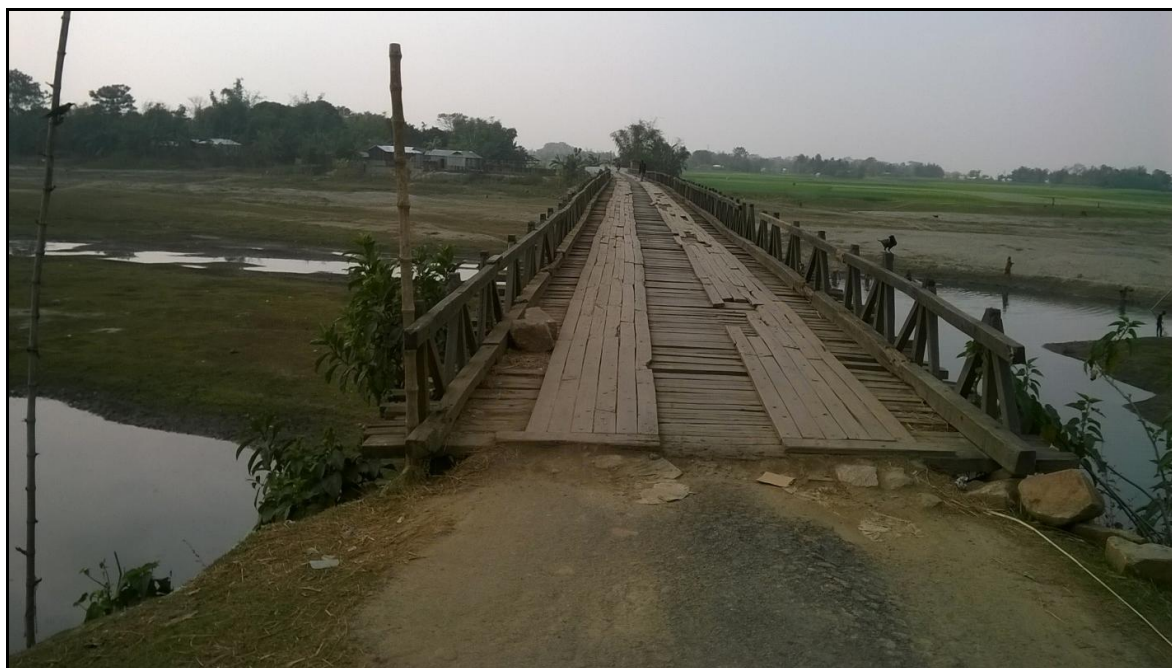
Figure 16- Wooden Bridge (Chainage - 36.751 km)
