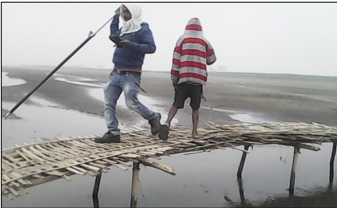
Figure 11- Bamboo Bridges (Chainage- 16.75 km and 17.443 km)
