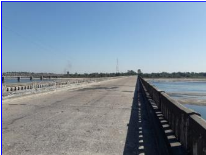
Figure 2.8 National Highway NH 52, at Chowldhowa CH 105.5 km
