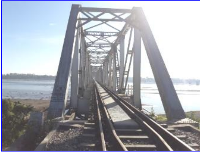
Figure 2.7 Northeast Frontier Railway track at CH 106 km
