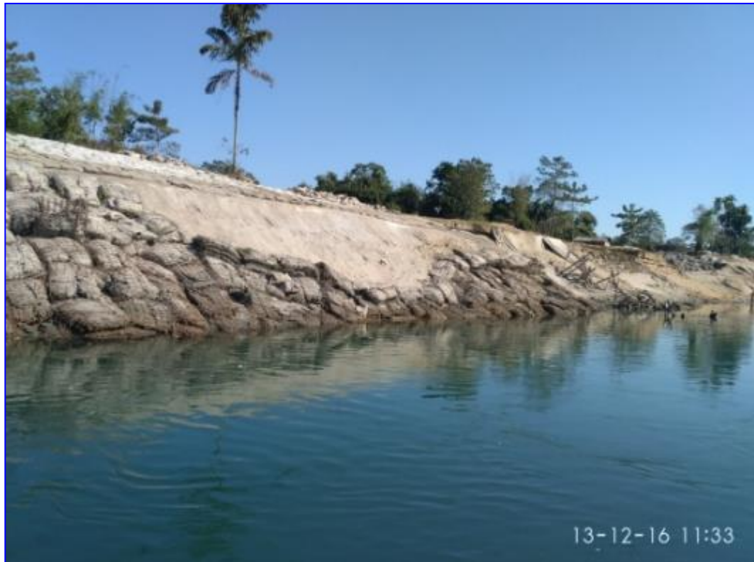
Figure 2.2 Sandbag protection on riverbank at Bhimpara
