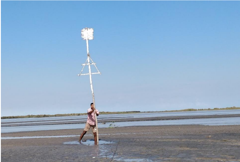
Figure 6.4 Temporary marker to demarcate navigation channel in Brahmaputra river
