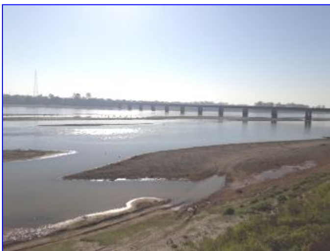
Figure 2.9 High Tension Line at CH 105.5 km - Chowldhowa
