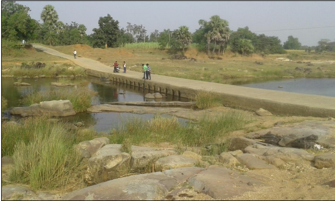
Figure 25- Check Dam (Chainage- 69.134 km)
