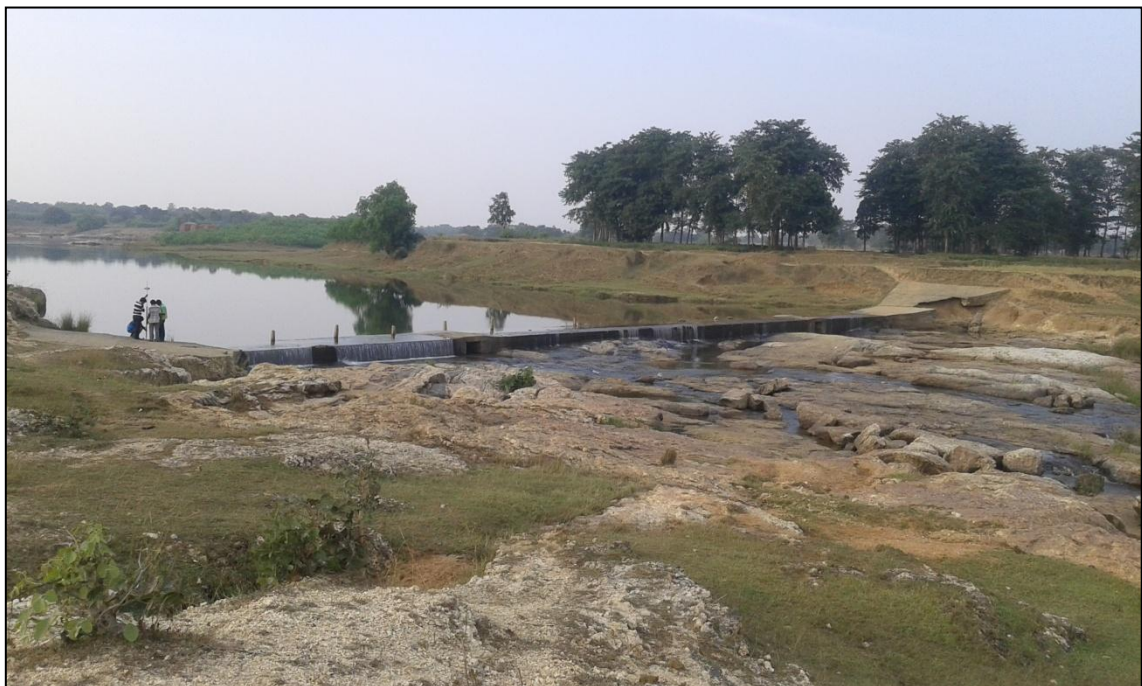
Figure 24- Check Dam (Chainage- 63.998 km)
