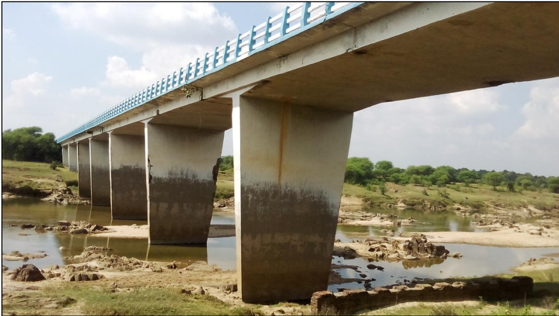
Figure 14- Manbazar RCC Bridge (Chainage-20.216 km)
