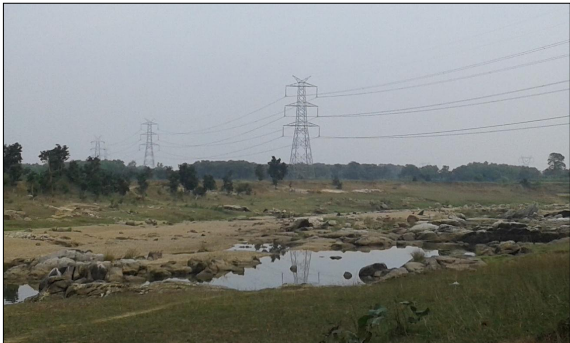
Figure 26- High Tension Lines (Chainage- 63.499 km, 63.571 km, 63.578 km and 69.120 km)
