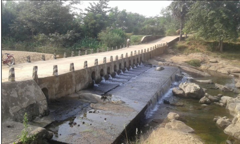
Figure 30- Check Dam (Chainage-74.338 km)
