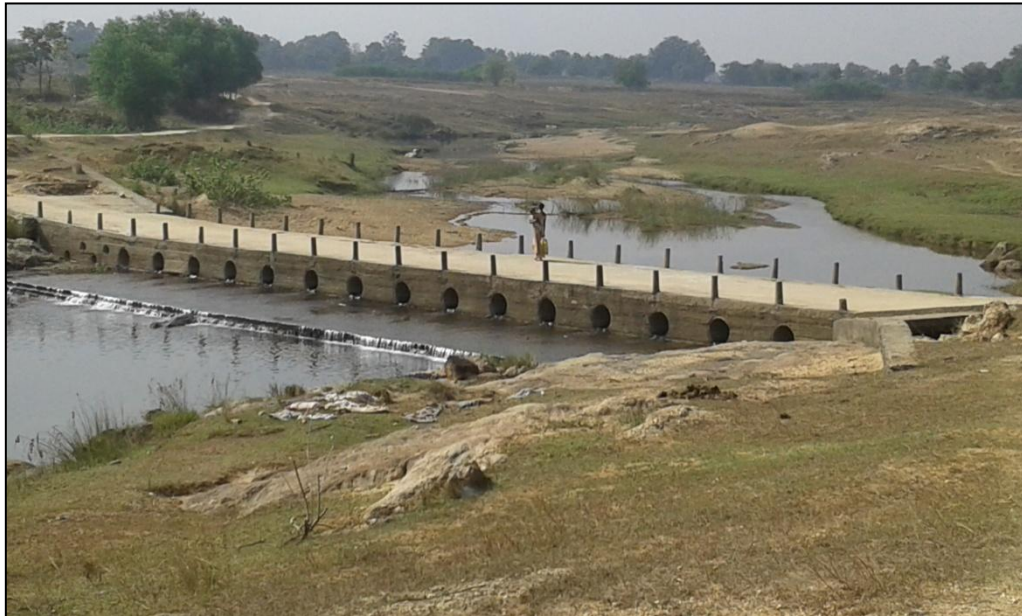
Figure 29- Check Dam (Chainage- 72.314 km)
