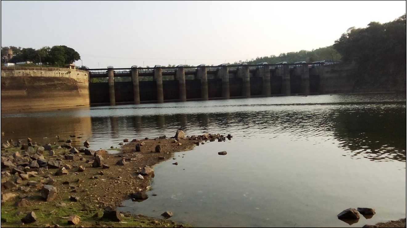
Figure 11- Mukutmanipur Dam (Chainage-0.00 km)
