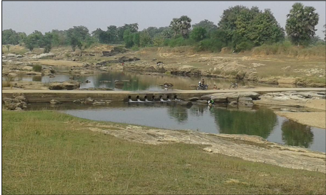
Figure 20- Check Dam (Chainage- 54.201 km)
