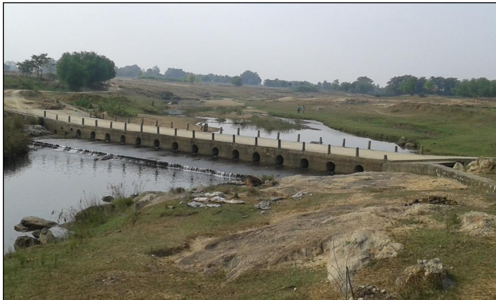
Figure 50- Check Dam (Chainage-74.338 km)
