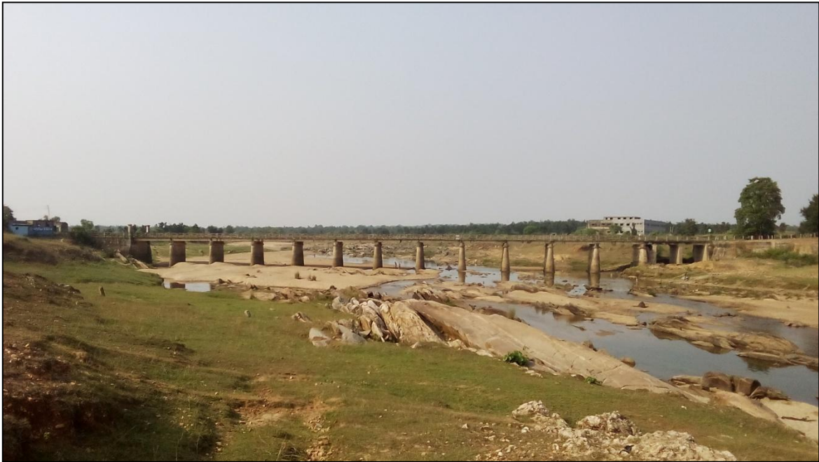
Figure 16- Duarsini RCC bridge (Chainage- 34.524 km)
