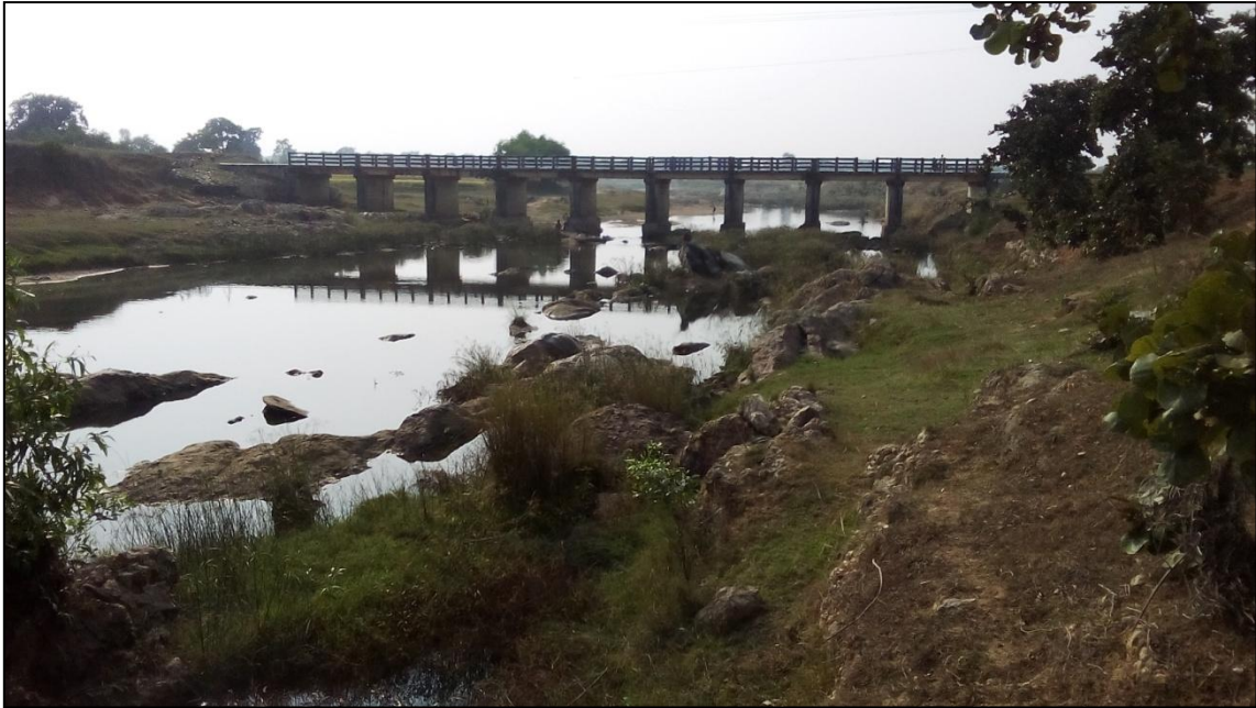
Figure 23- Bishari Kumari RCC Bridge (Chainage- 63.621 km)
