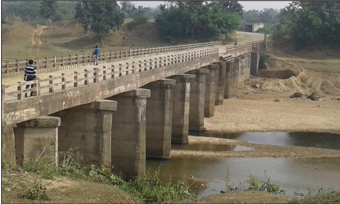
Figure 18- Ganganarayan RCC Bridge (Chainage- 46.521 km)
