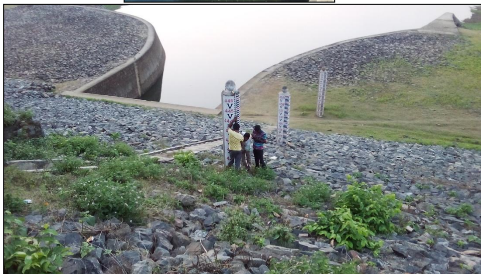
Figure 3-C.W.C Gauge at Mukutmanipur Dam site (Chainage-0.00 km)
