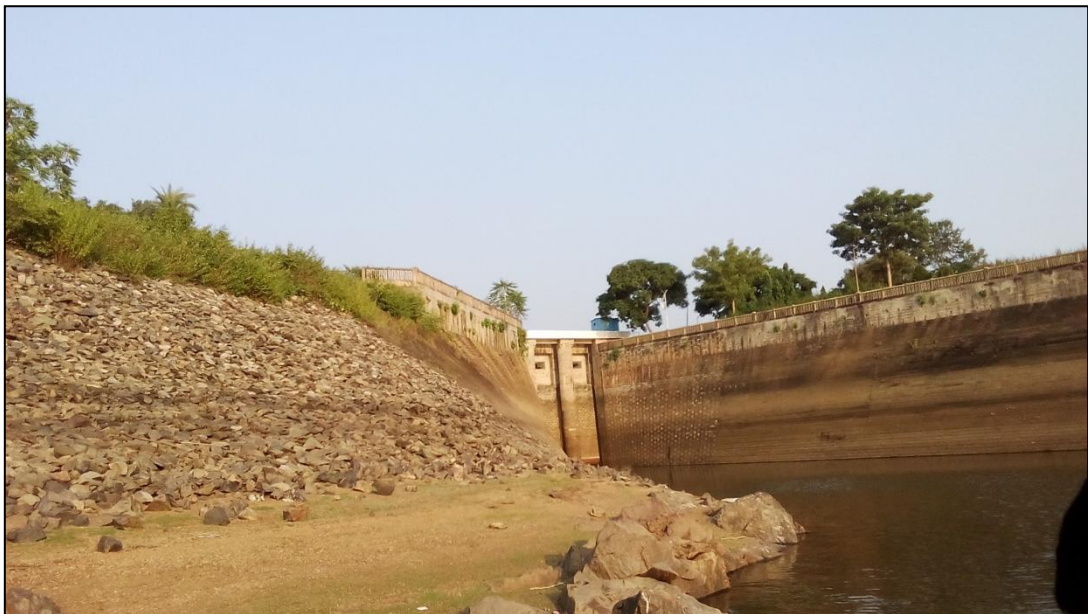
Figure 48-Reservoir Gate (Chainage-0.000 km)
