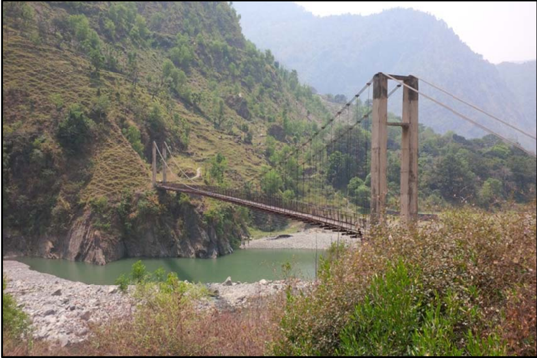
Figure 20 – Ch.41.126 Km Sherpur Bridge
