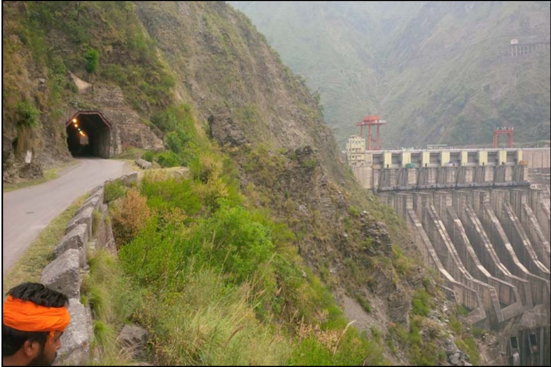
Figure 23 – Ch.44.276 Km Road Tunnel on Chamera Dam at Gandhinar
