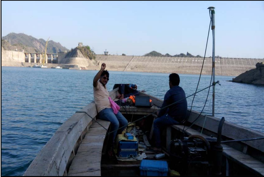
Figure 9 – Ch. 0.00 Km Ranjit Sagar Dam Axis View from Upstream Side
