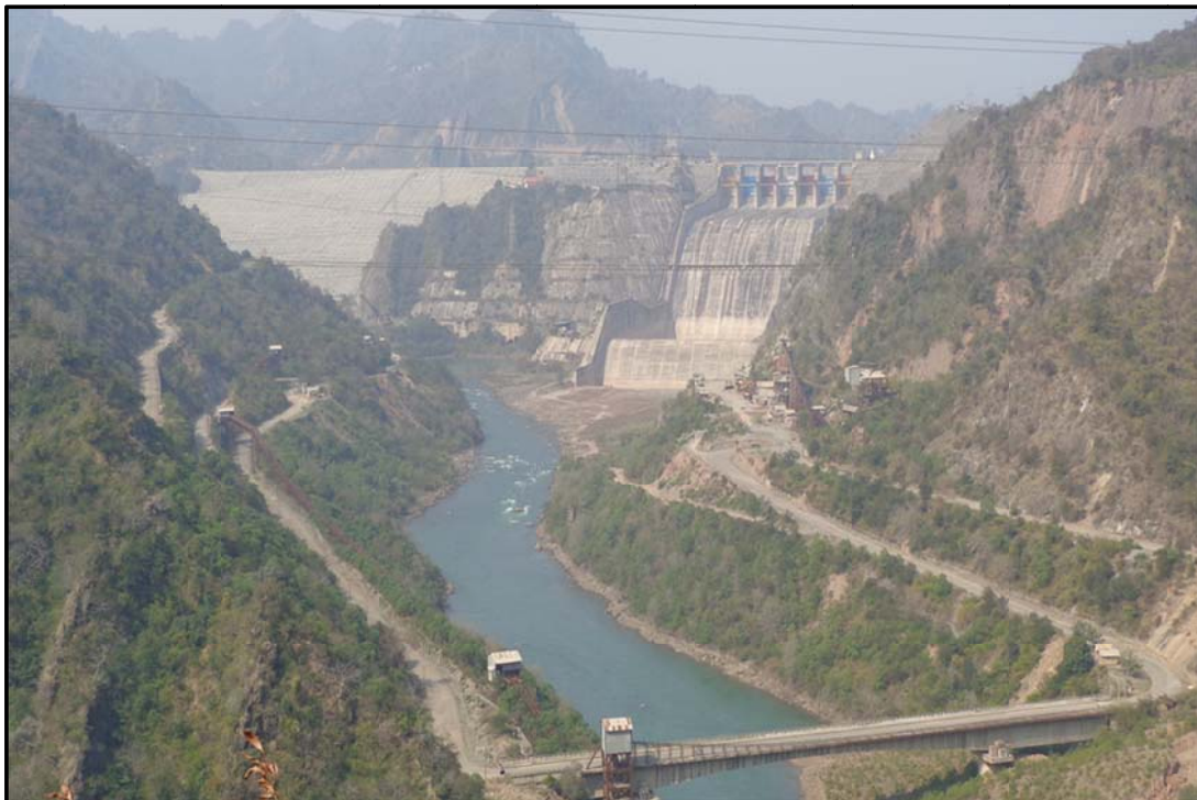
Figure 4 – Ch.0.00km Ranjit Sagar Dam
