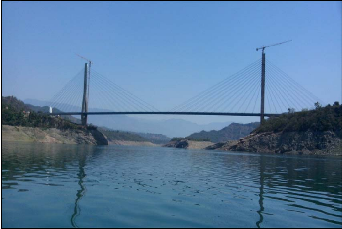
Figure 4 – Ch. 11.198 km Basohli Bridge
