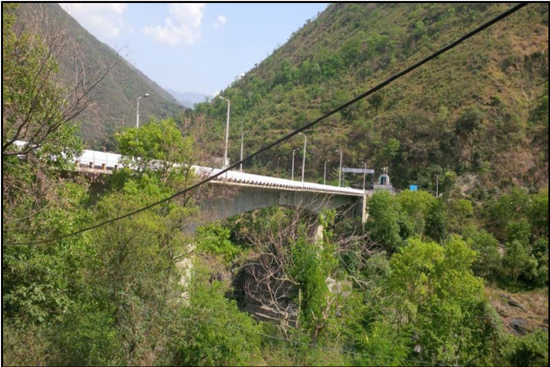
Figure 15 – Ch.32.517 Km Khairi Bridge
