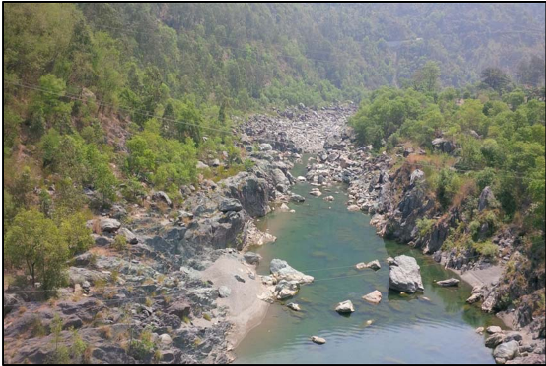
Figure 16 – Ch.32.67 Km Dry River Near Khairi Bridge
