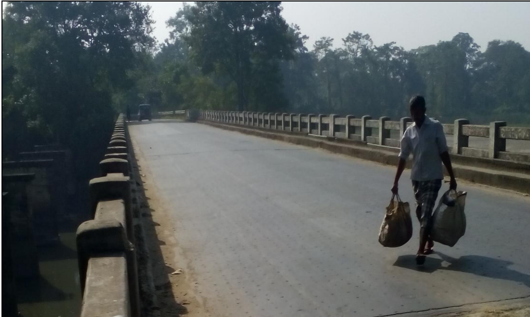
Figure 18- RCC Bridge (Chainage-42.844 km)
