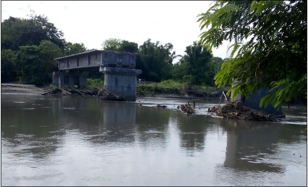
Figure 16- Under- Construction RCC Bridge (Chainage- 34.920 km)
