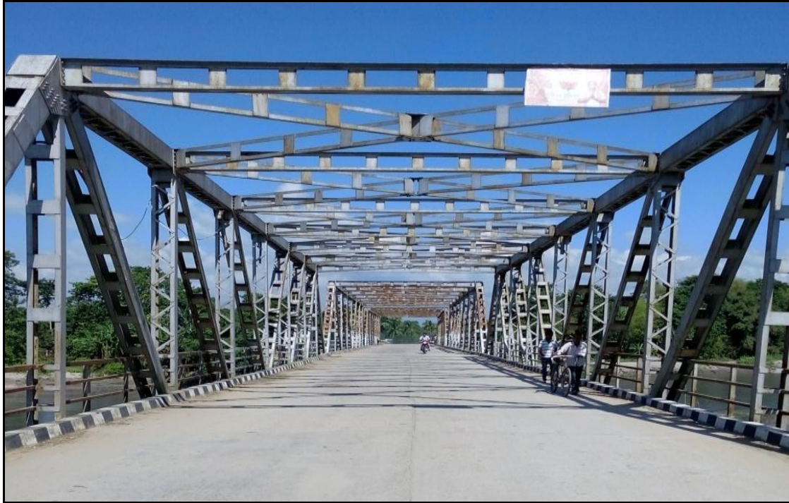
Figure 21 - RCC Bridge (Chainage- 55.030 km)
