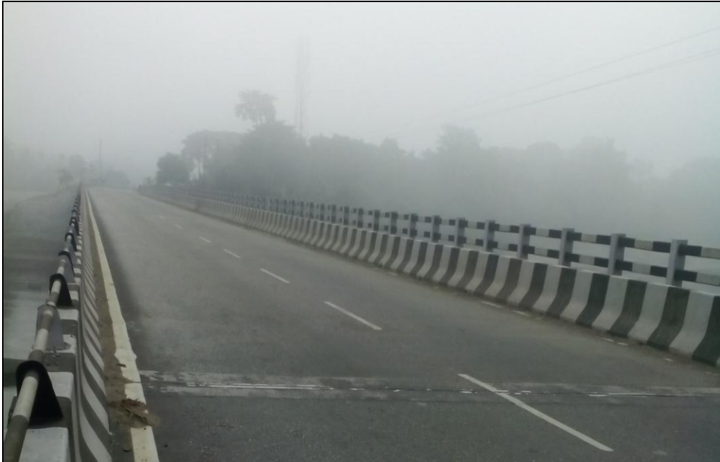
Figure 23- RCC Bridge- (Chainage-57.959 km)
