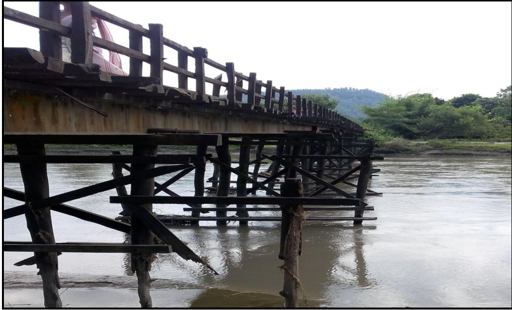
Figure 12- Wooden Bridge (Chainage-25.635 km)
