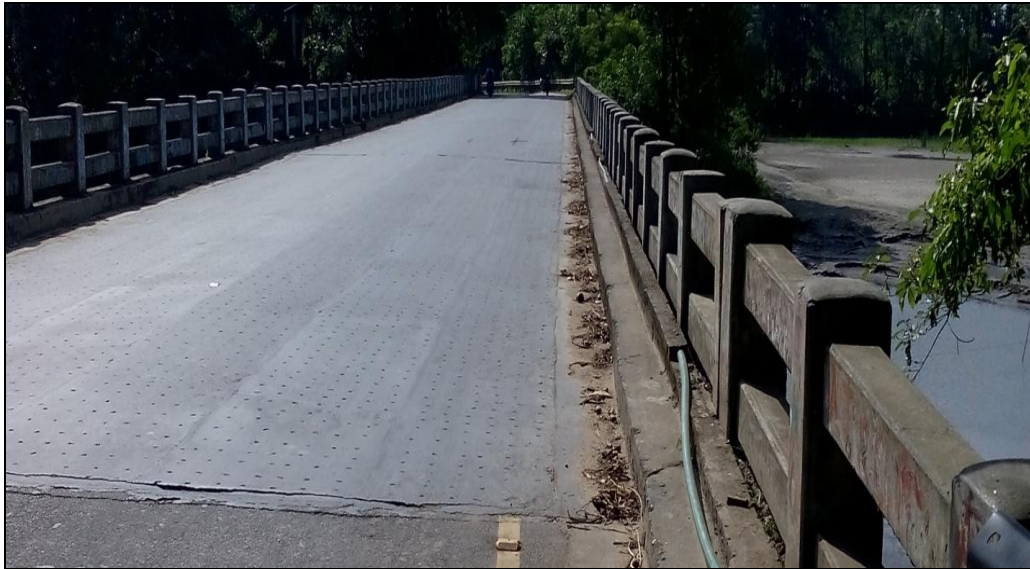
Figure 14- RCC Bridge (Chainage- 32.050 km)
