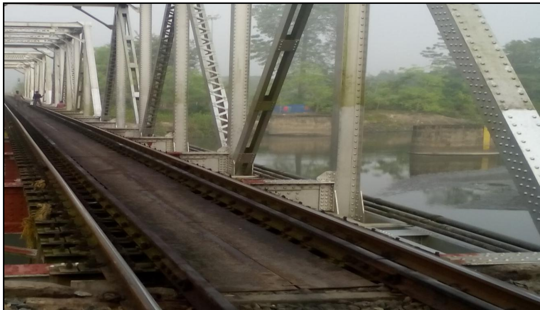
Figure 22- Rail Bridge (Chainage-57.602 km)
