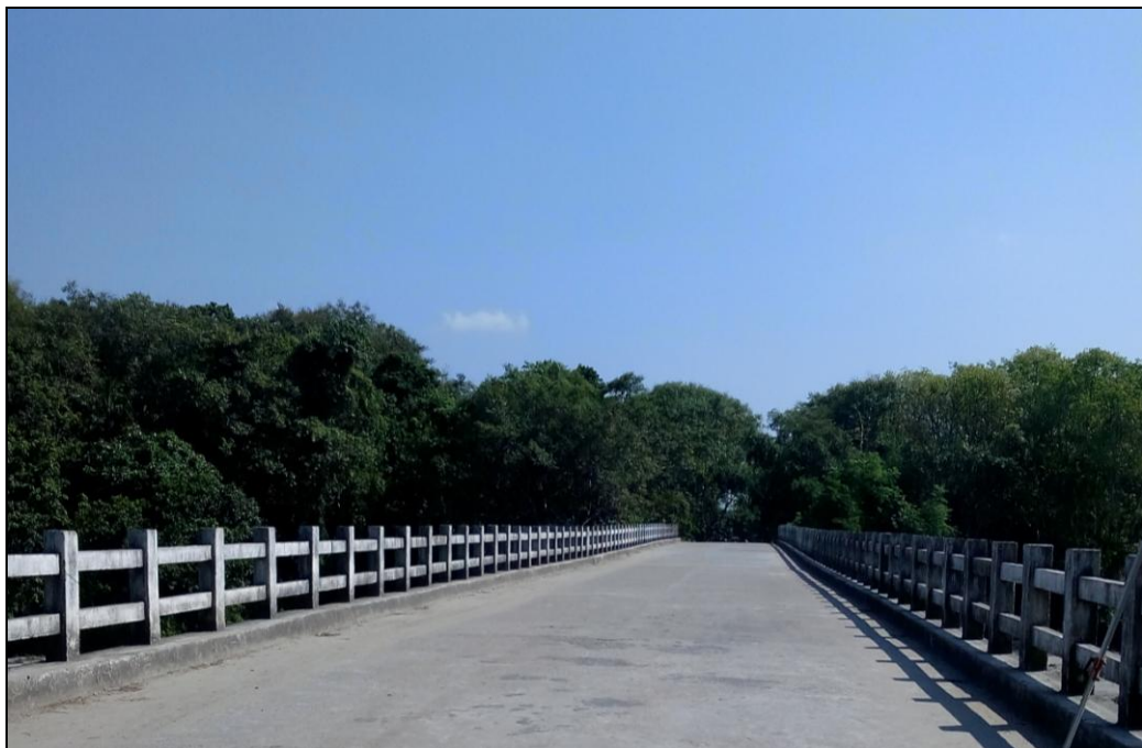
Figure 24- RCC Bridge-(Chainage-57.979 km)
