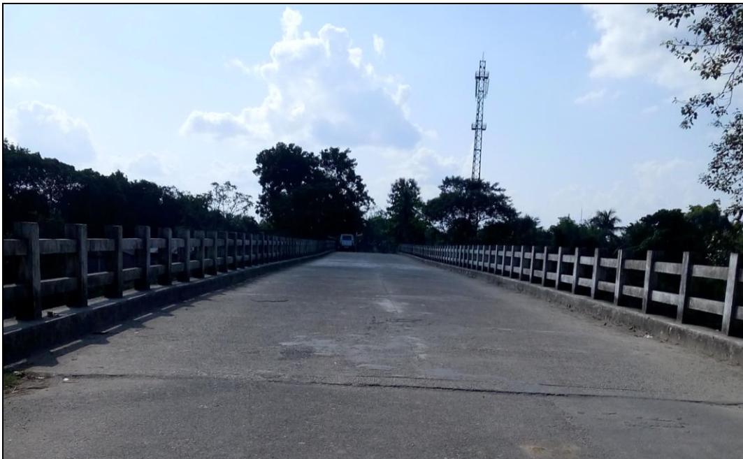
Figure 19 RCC Bridge (Chainage-48.495 km)
