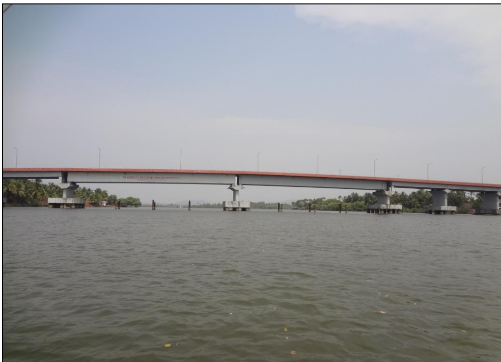
Photo 10: Asolna Bridge at Ch 6.20km (15°10'41.9539"N, 73°57'38.7456"E)
