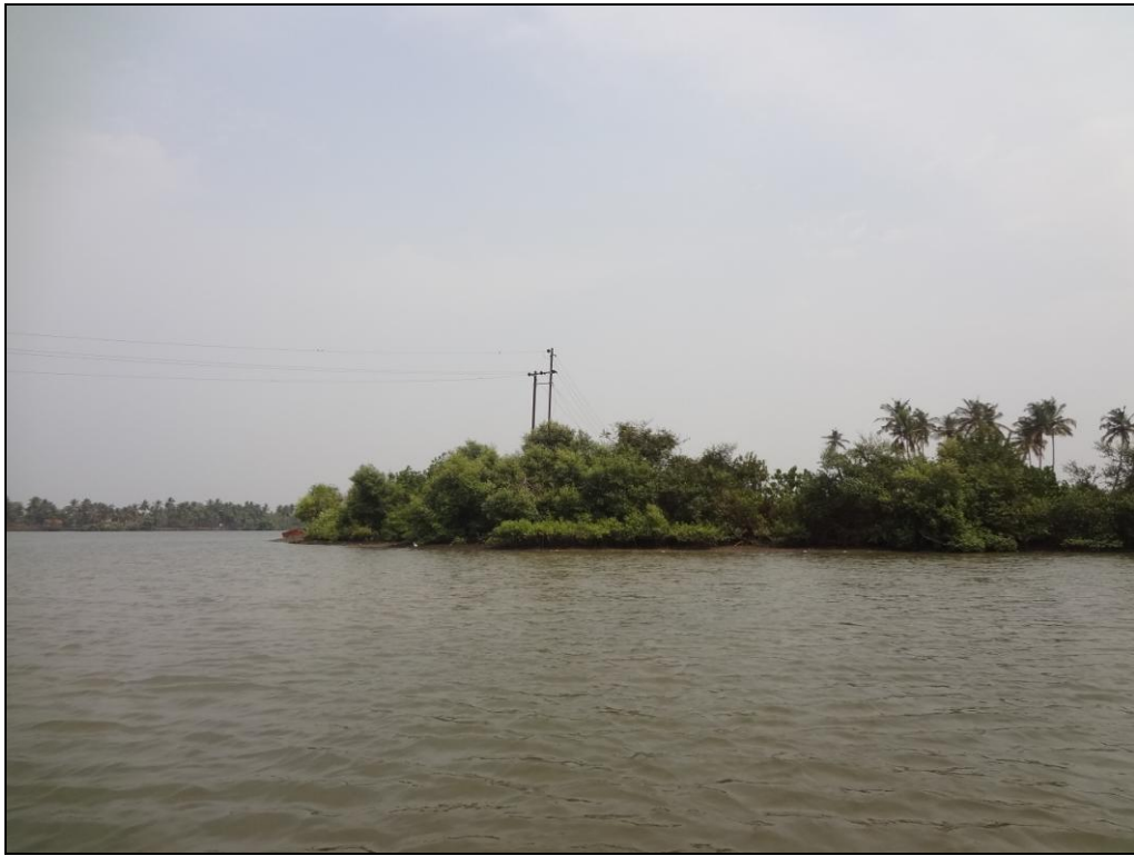
Photo 9: Electric Wire crossing River at Ch 4.21km (15°10'14.2572"N, 73°56'56.7898"E)
