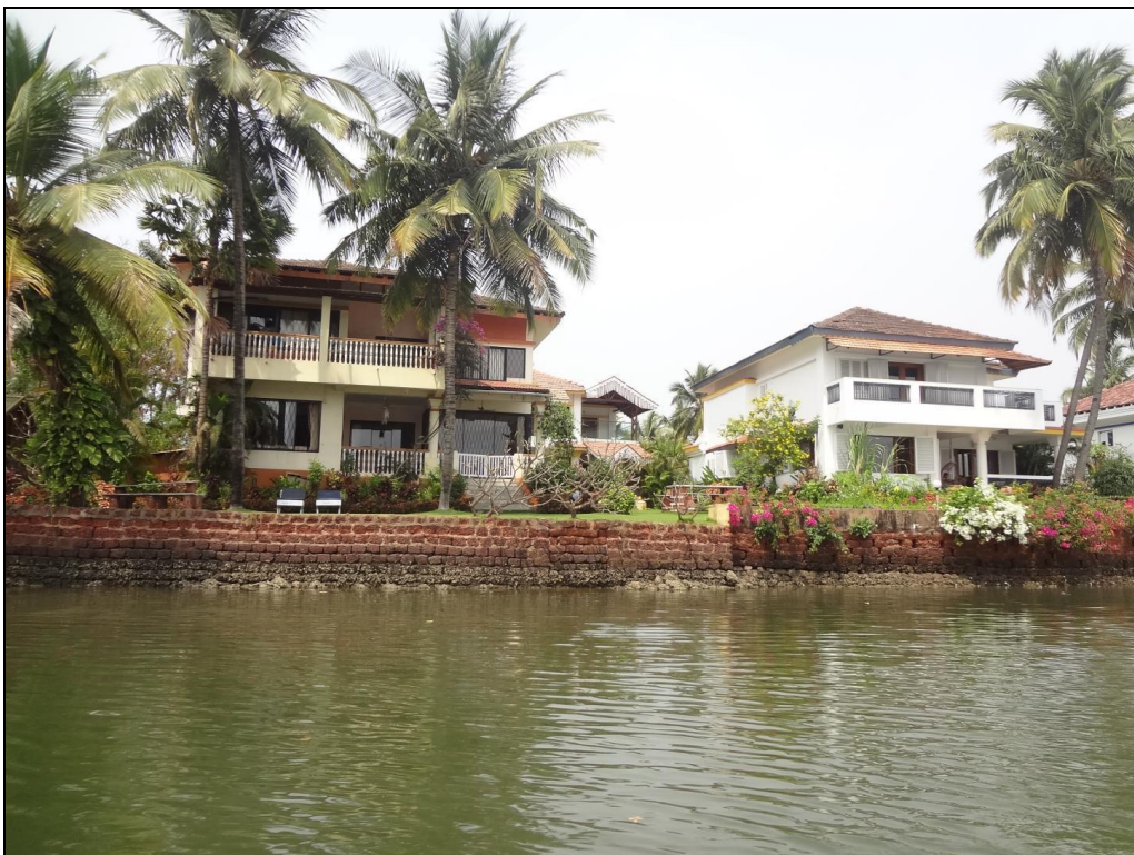
Photo 8: Hotel on the River bank at Ch 3.94km (15° 10'19.0"N, 73° 56'46.1"E)
