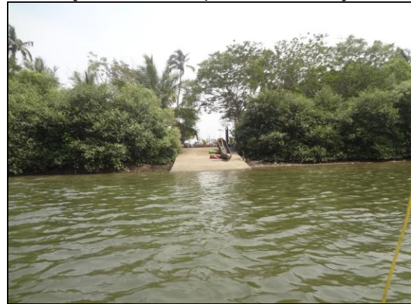
Figure 2.4: Asolna Ferry Jetty at Chainage 7.90 km (15°10'47.0485"N, 73°57'46.0493"E)
