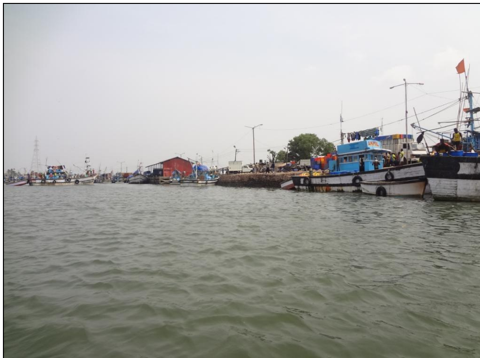
Photo 2: Cutbona Fishing jetty at Ch 1.31km (15°09'06.9"N, 73°57'07.9"E)
