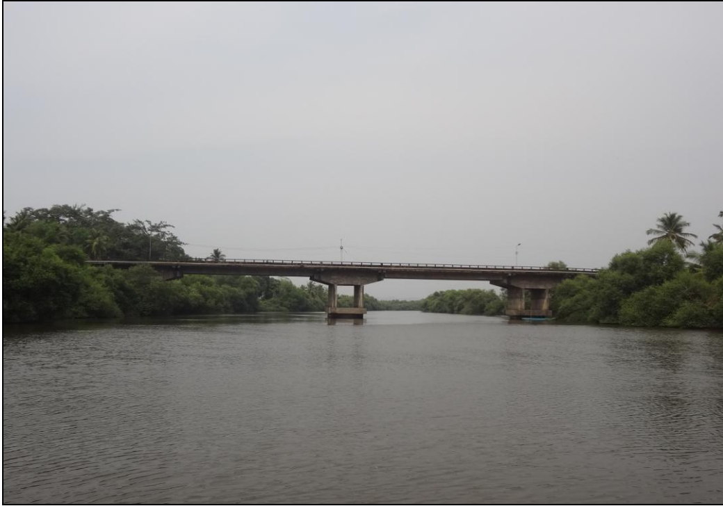
Photo 15: Navelim Bridge at Ch 14.26km (15°13'11.4112"N, 73°57'29.0631"E)
