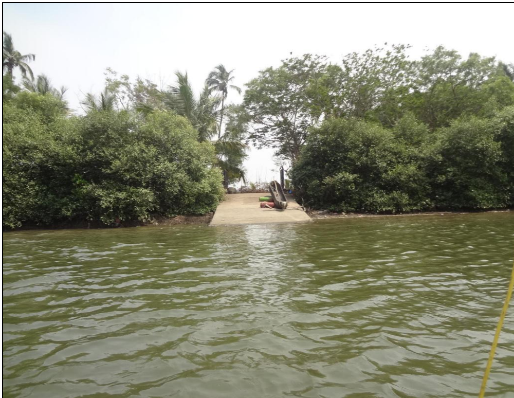
Photo 12: Asolna Ferry Jetty at Ch 6.46km (15°10'47.0485"N, 73°57'46.0493"E)
