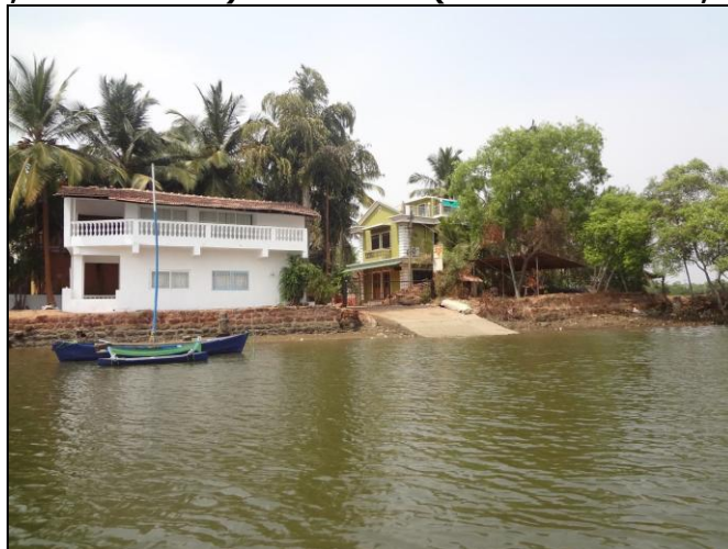
Figure 2.5: Ferry Jetty of Cavlossim village at Chainage 8.00 km (15°10'48.2124"N, 73°57'40.7286"E)
