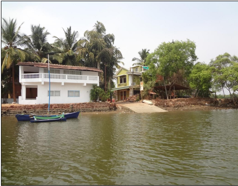
Photo 11: Ferry Jetty of Cavlossim village at Ch 6.39km (15°10'48.2124"N, 73°57'40.7286"E)
