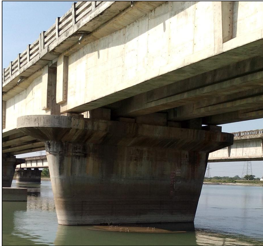
Figure 14- R.C.C. Bridge (Chainage- 47.926 km) (Kolkata to Guwahati)
