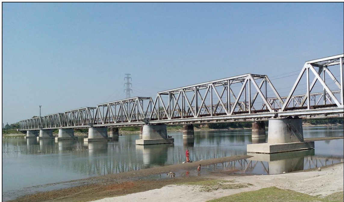
Figure 15- Railway Bridge (Chainage- 48.266km and 48.318 km) (Kolkata – Guwahati)
