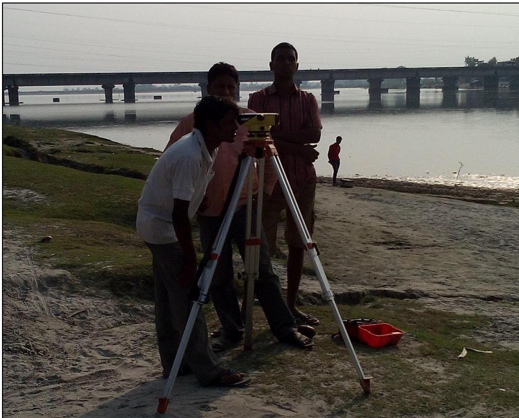
Figure 16- Site pictures of Topography instruments
