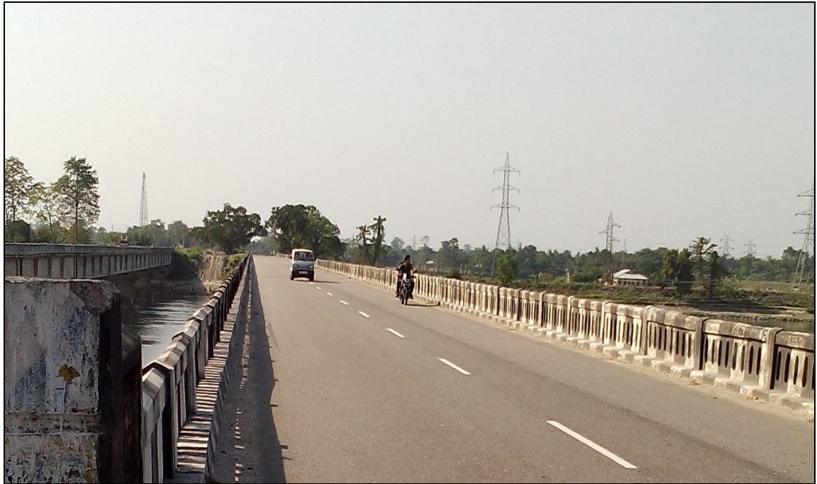
Figure 17- RCC Bridge (Chainage- 55.774 km)
