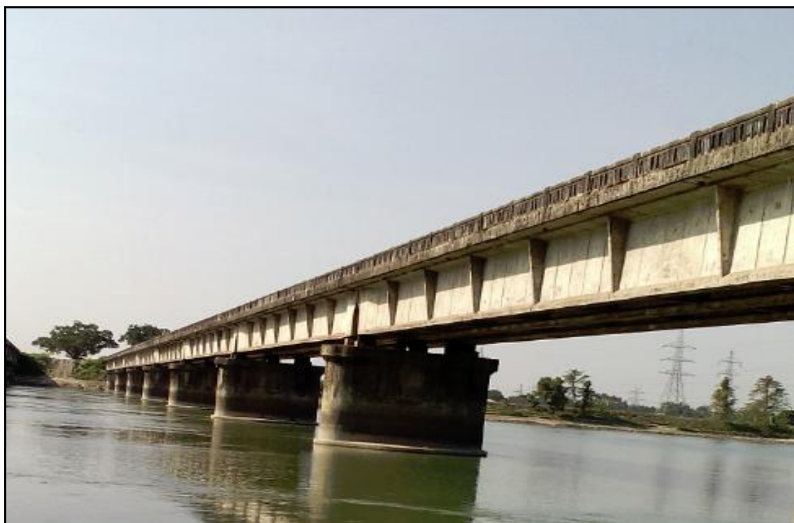
Figure 13- RCC Bridge (Chainage- 47.893 km)
