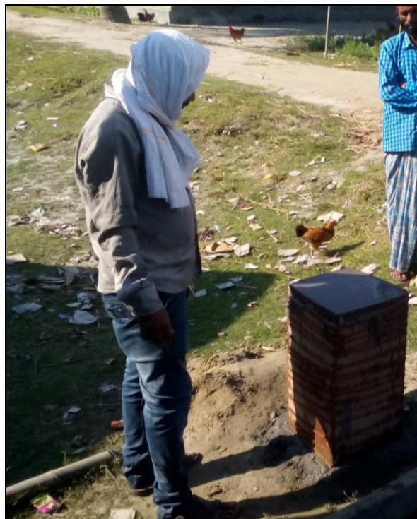
Figure 26-B.M pillar Establishment
