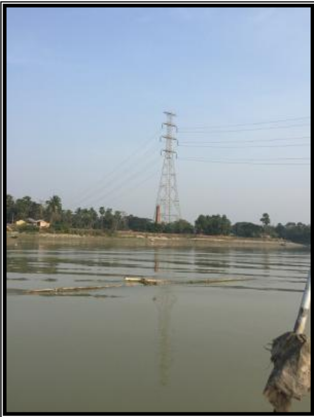
HIGH TENTION LINE CHAINAGE 41.5
