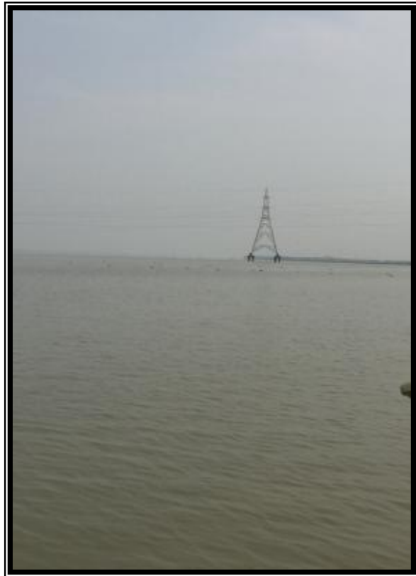
HIGH TENTION LINE CHAINAGE 29.0
