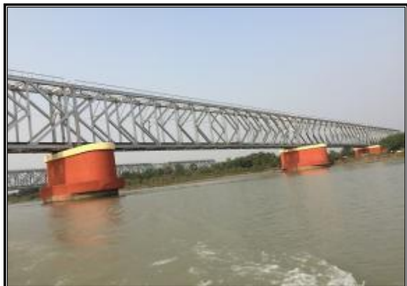
KOLAGHAT RAILWAY BRIDGE CHAINAGE 30
