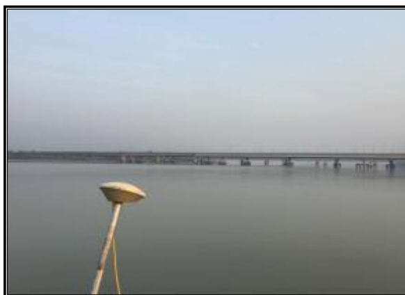
KOLAGHAT ROAD BRIDGE CHAINAGE 30.5
