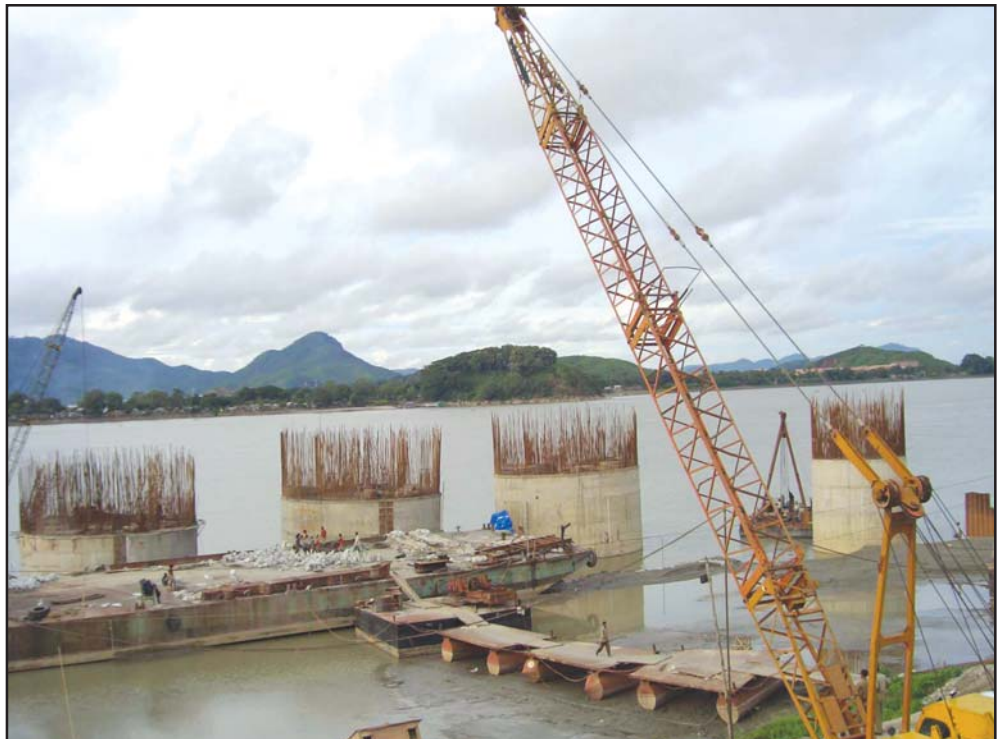
TERMINAL AT PANDU UNDER CONSTRUCTION
