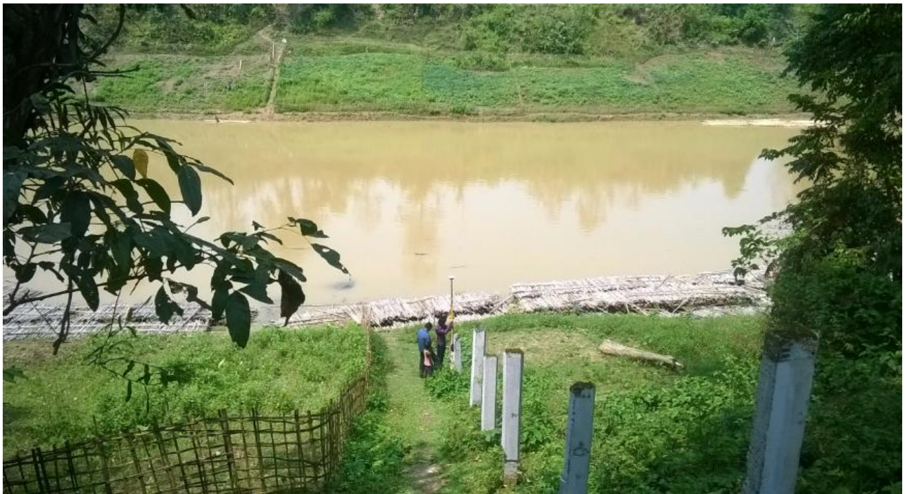
Figure 5- CWC Gauge at Gharmura RCC Bridge
