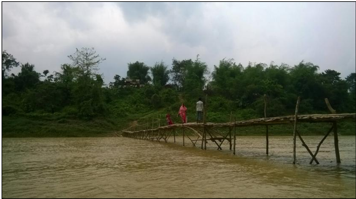
Figure 12- Bamboo Bridge (Chainage- 12.121km)
