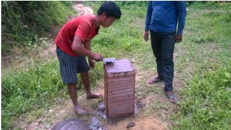
Figure 43-B.M pillar Establishment
