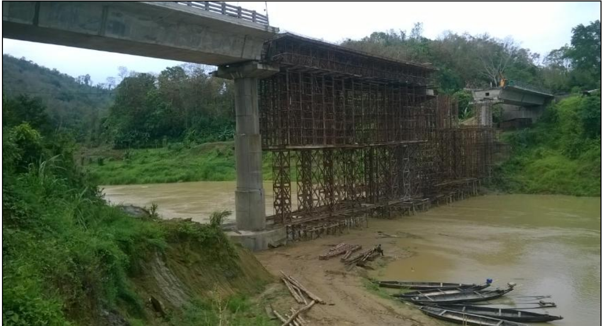
Figure 13- Bhairabi RCC Bridge (Chainage- 24.218 km)
