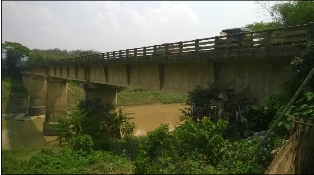
Figure 9- Gharmura RCC Bridge (Chainage-0.410 km)
