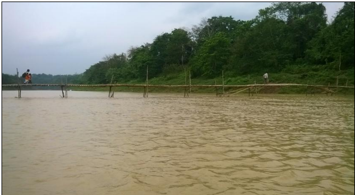
Figure 10- Bamboo Bridge (Chainage- 6.706 km)
