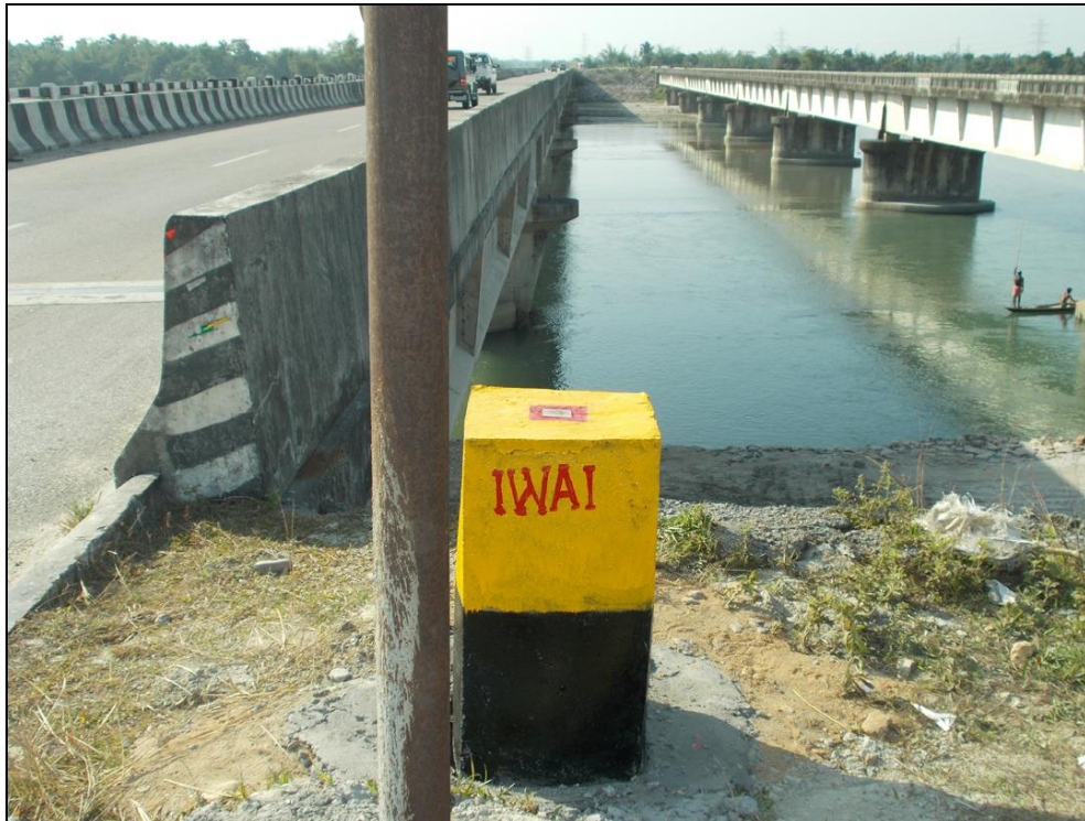
Figure 38-RCC Bridges with Bench Mark-7 near at Chainage 55.789 km
