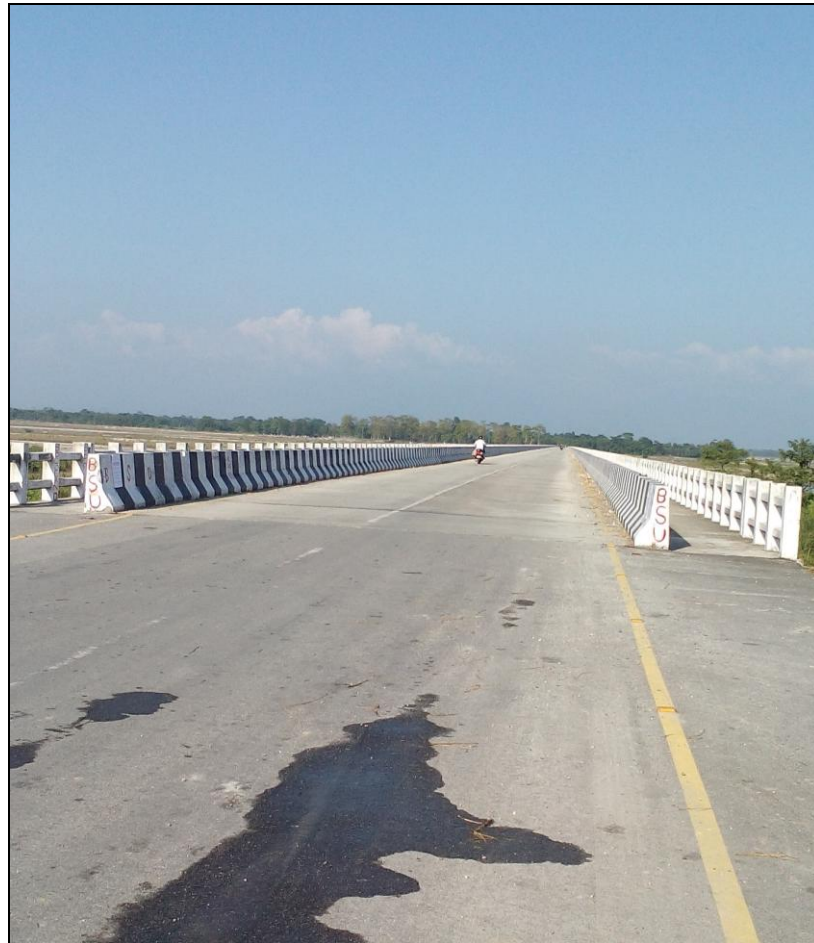
Figure 19- RCC Bridge (Chainage- 68.484 km) (Lat. -26°33'41.57"N, Long. - 90°34'6.75"E)
