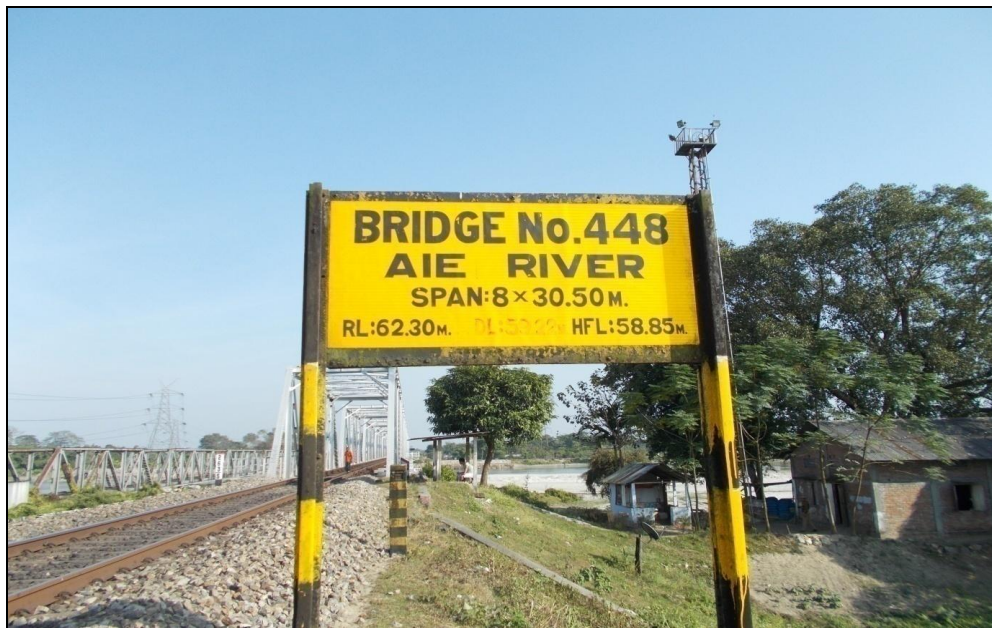
Figure 16 - Railway Steel Bridge (Chainage – 56.156 km) (Lat. - 26°30'1.46"N, Long. - 90°39'12.93"E)
