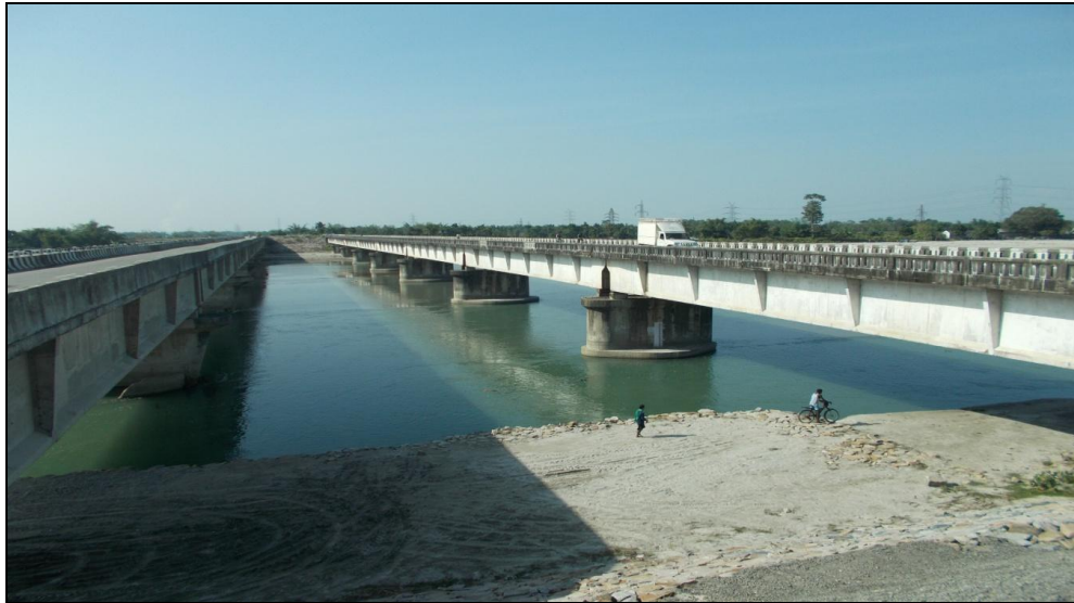
Figure 15 - RCC Bridges (Chainage- 55.789 km and 55.821 km) (Lat.-26°29'49.32"N, Long.-90°39'13.61"E), (Lat.-26°29'50.07"N, Long. - 90°39'13.63"E)
