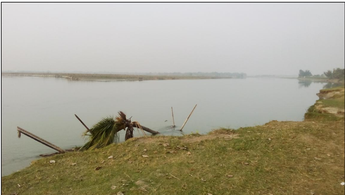
Figure 42- Embankment at River bank side
