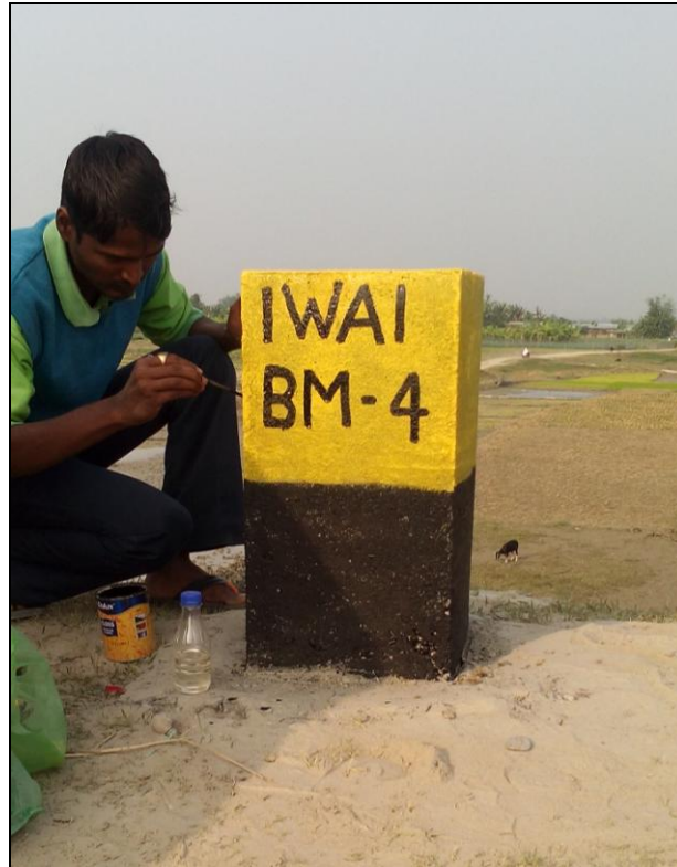
Figure 40- Establish BM pillar-4 near at Chainage- 25.645 km
