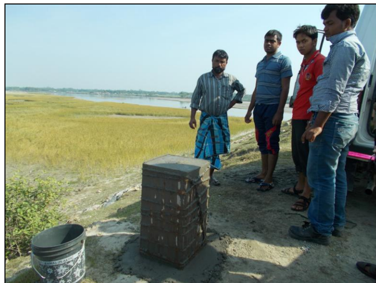
Figure 41-BM establishment near the river bank side
