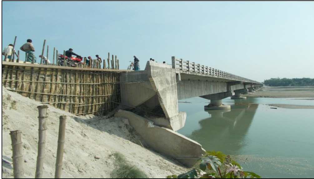
Figure 11 - Under Construction RCC Bridge (Chainage- 36.355 km) (Lat. - 26°22'52.01"N, Long. - 90°44'15.00"E)
