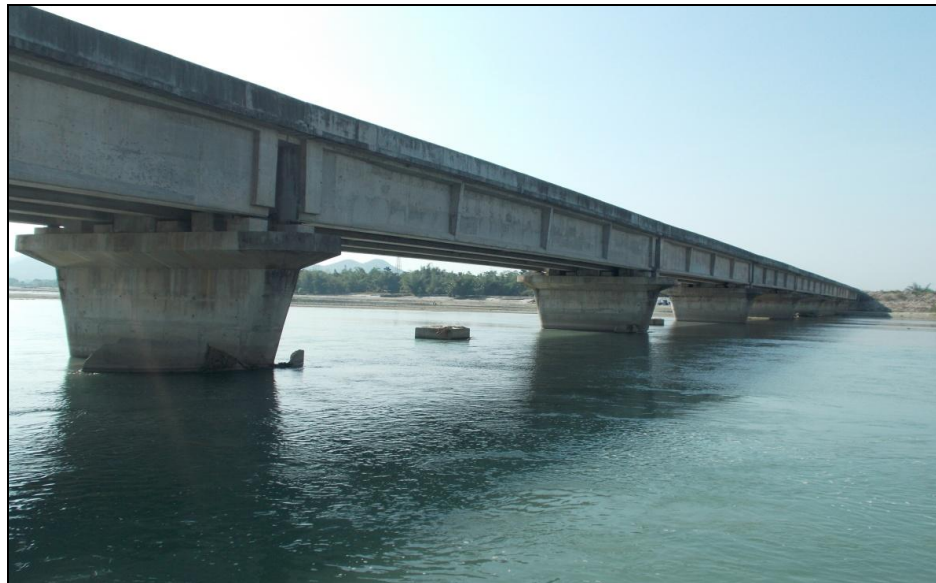
Figure 9 - Abhayapuri Lengtishinga RCC Bridge (Chainage-25.645 km) (lat. - 26°18'26.59"N, long. - 90°45'5.94"E)
