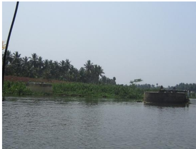
Figure 21 - Pump Houses for Drinking Water on Bhavani River (73.44 km Chainage)
