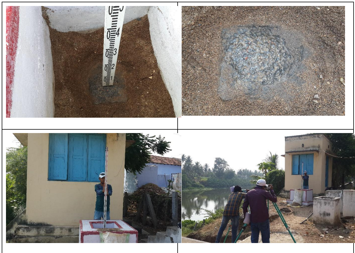
Figure 7 - MTBM at CWC Site Savanadapur (29.9 km chainage)
