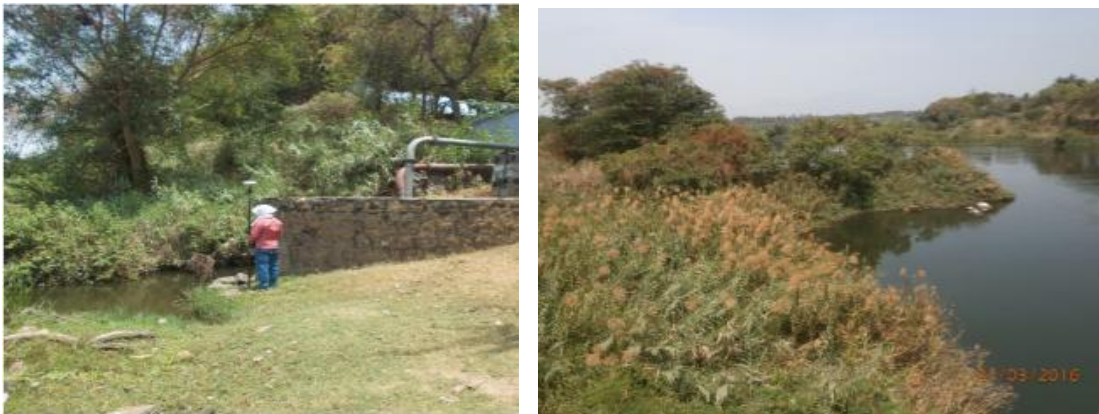
Figure 5 - Spot Leveling and River Bank of Bhavani River (89.5 km chainage)
