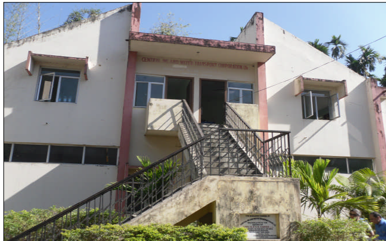
Figure 2.13 View of Admin Building in CIWTC Terminal at Badarpur
