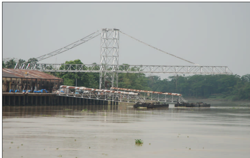
Figure 2.7 View of CIWTC Terminal at Karimganj during Flood
