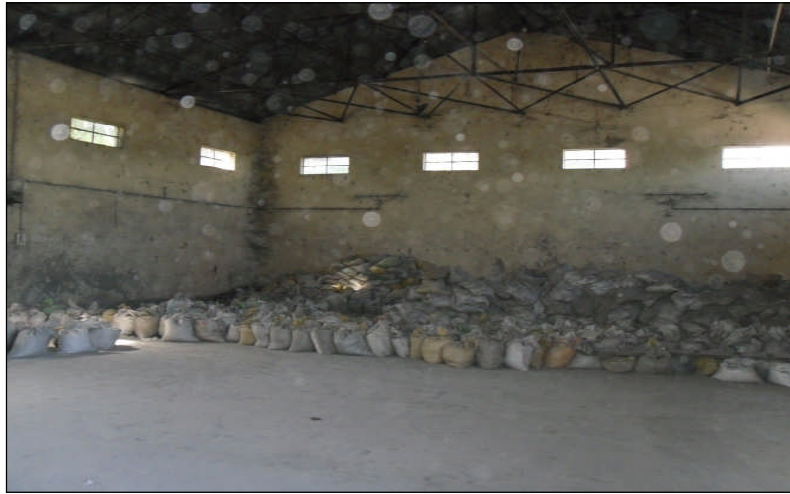
Figure 2.10 View of Covered Shed at CIWTC Terminal at Badarpur
