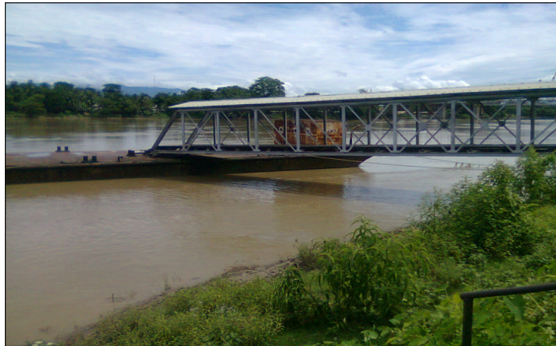
Figure 2.12 View of Gangway Arrangement in CIWTC Terminal at Badarpur during Flood flow
