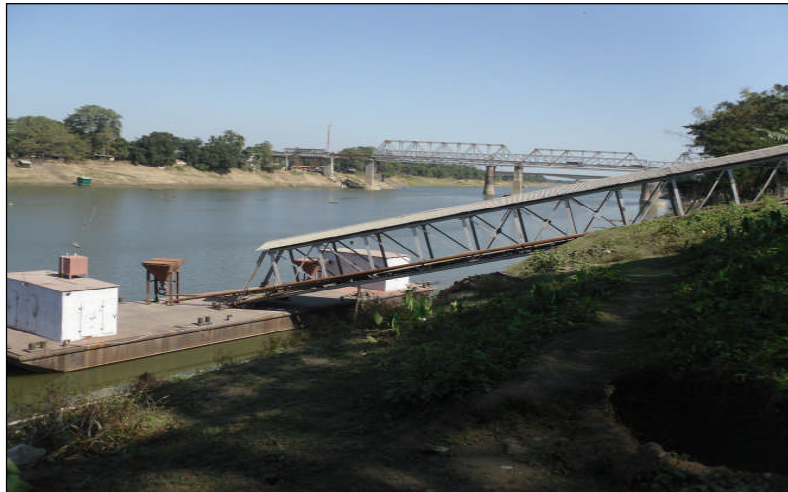
Figure 2.11 View of Covered Shed at CIWTC Terminal at Badarpur
