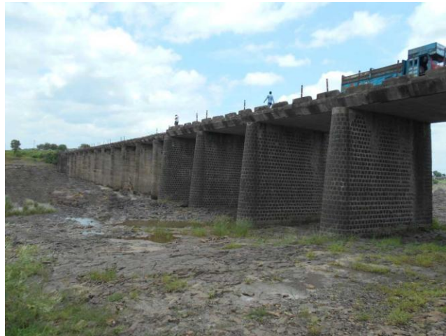
Figure 9 - Khadka Road Bridge (2.72 km chainage)
