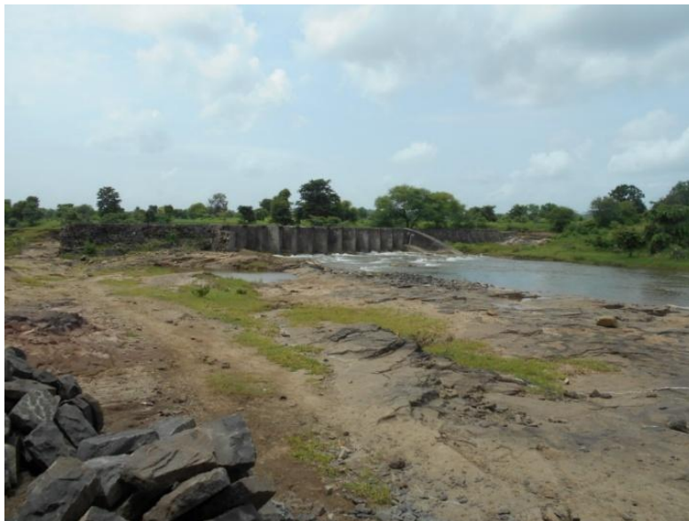
Figure 28 - Harsul Bridge (85.52 km chainage)
