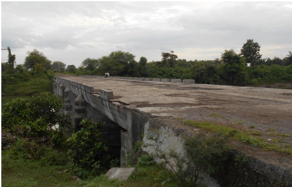
Figure 16 - Vitholi Bridge (34.38 km chainage)
