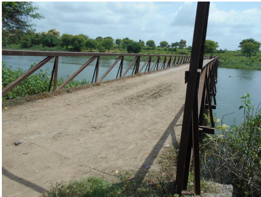
Figure 26 - Harsul Iron Bridge (83.12 km chainage)
