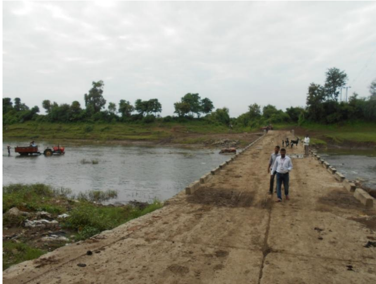
Figure 17 - Arni Road Bridge (45.26 km chainage)
