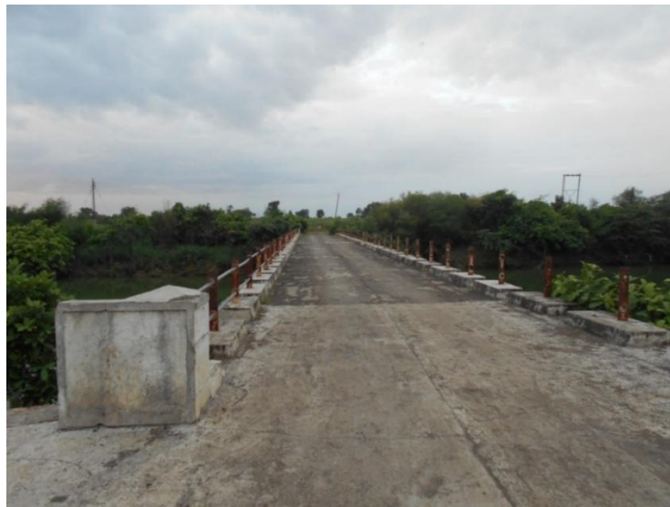
Figure 11 - Vitholi Road Bridge (25.82 km chainage)
