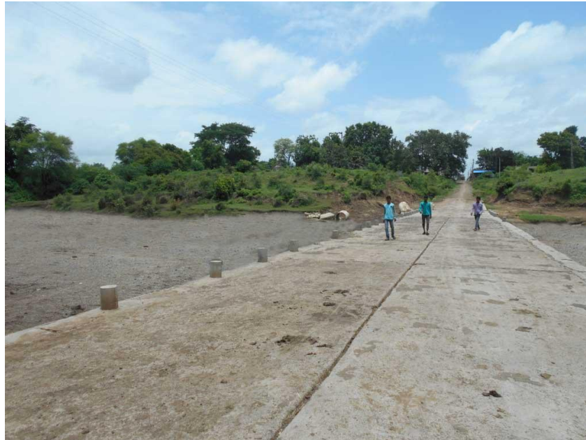
Figure 19 - Saikhed Sanko Bridge (54.98 km chainage)
