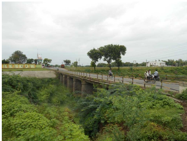
Figure 18 - Highway Bridge at Arni (46.18 km chainage)
