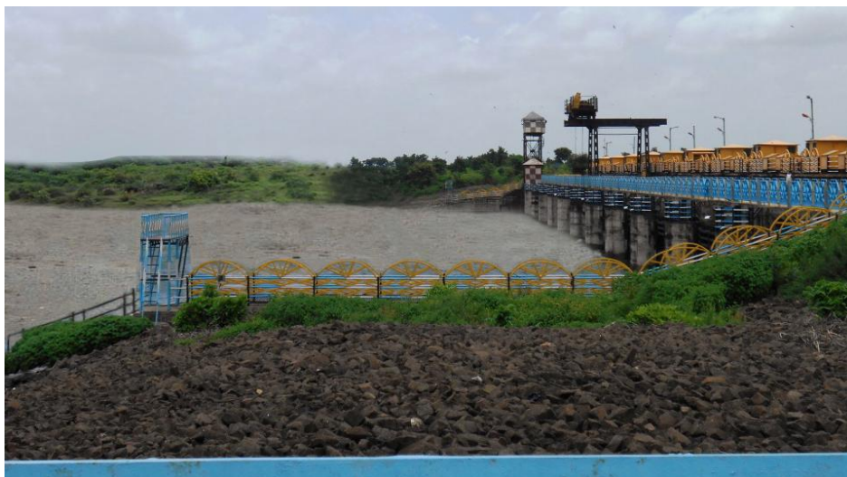
Figure 24 - Digras Arunawati Dam (65.37 km chainage)
