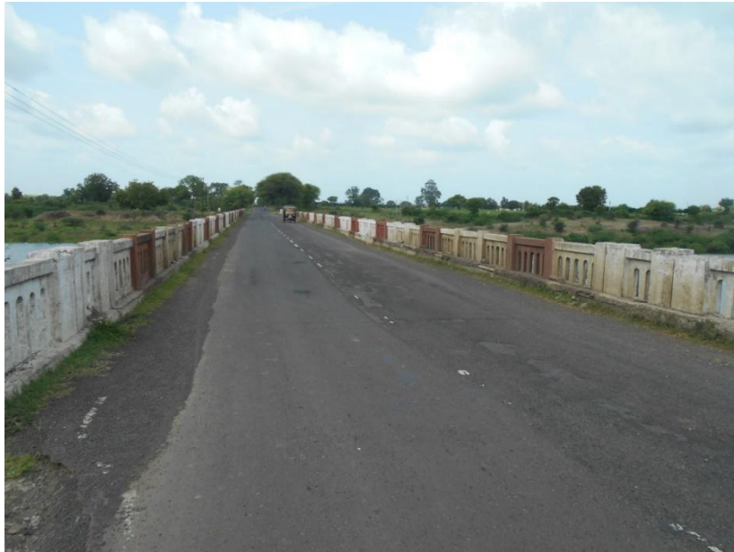
Figure 25 - Darwha By pass Road on SH 213 (81.92 km chainage)
