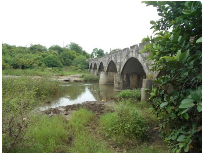
Figure 23 - Chirkuta Road Bridge (63.4 km chainage)
