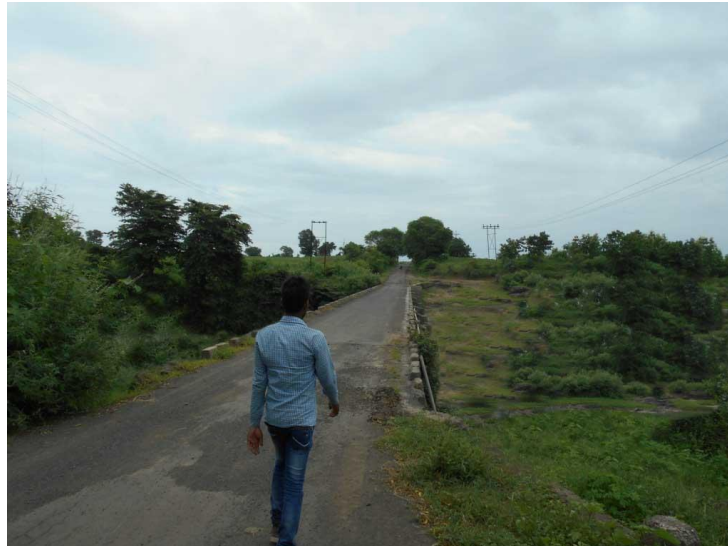
Figure 10 - Pardi Road Bridge (14.48 km chainage)
