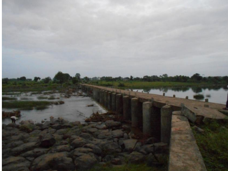
Figure 12 - Foot walk board Bridge at shiur (27.12 km chainage)
