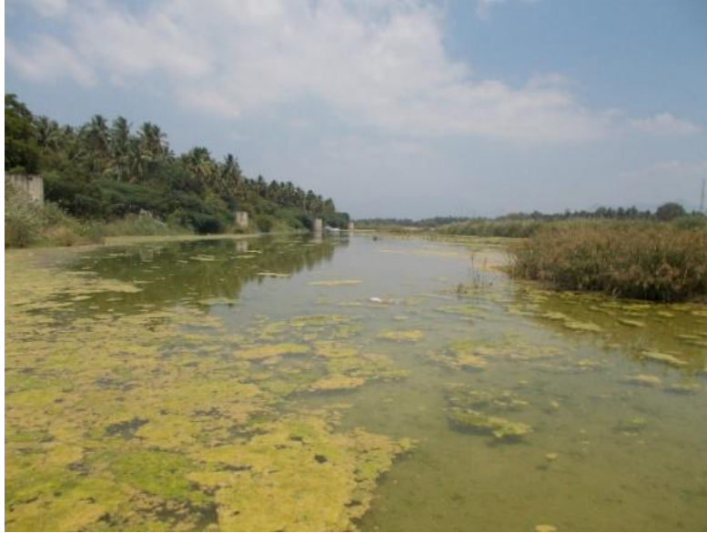
Figure 16 - Drinking Water Pump houses on Vaigai River (25.0 km chainage)
