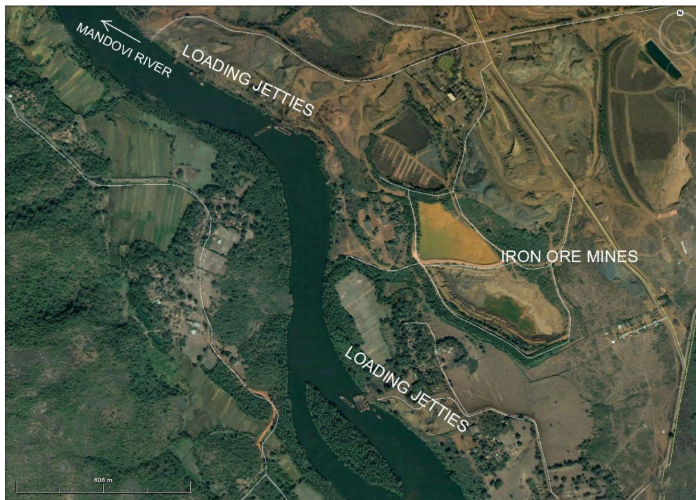
Fig. 3.4: Typical iron ore loading jetty locations along the banks of river Mandovi
