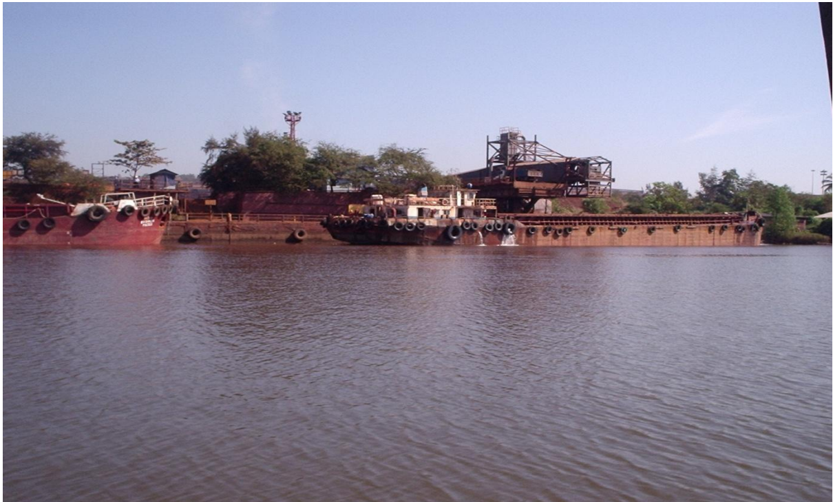
A View of Barge Loading Jetty along Mandovi River
