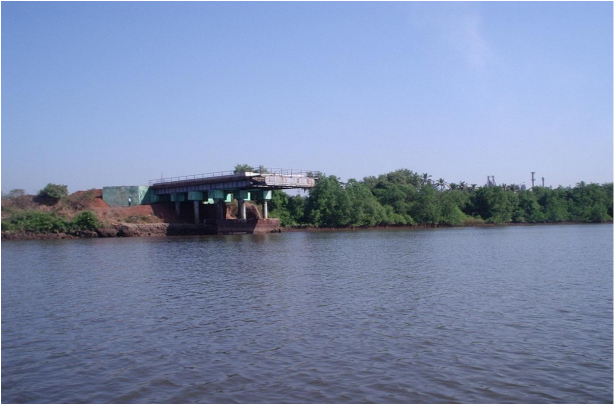
A View of Barge Loading Jetty along Mandovi River
