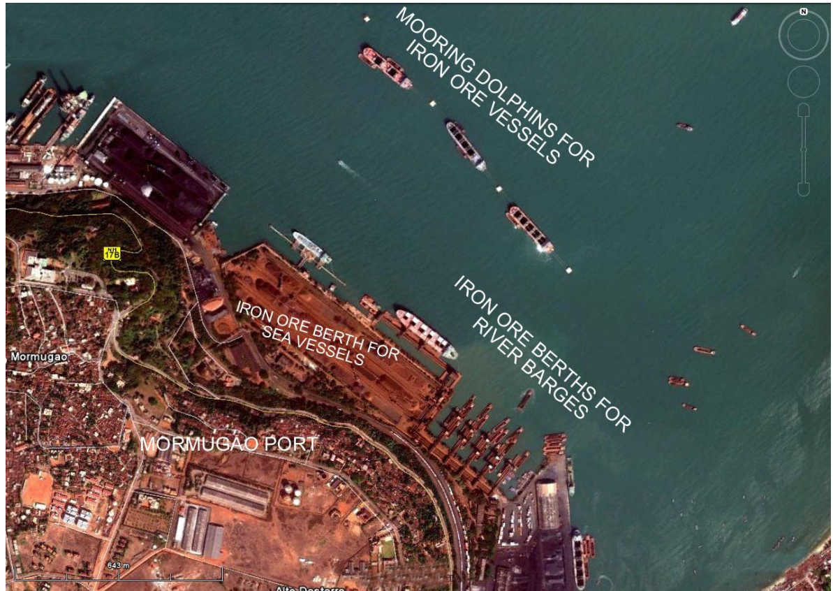
Fig. 3.1: Iron ore handling facilities at Mormugao port
