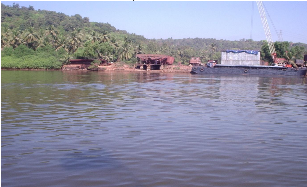
A View of Barge Repair Facility in Zuari River
