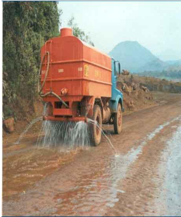
Fig.5.12: Suppress the road dust by sprinkling water
