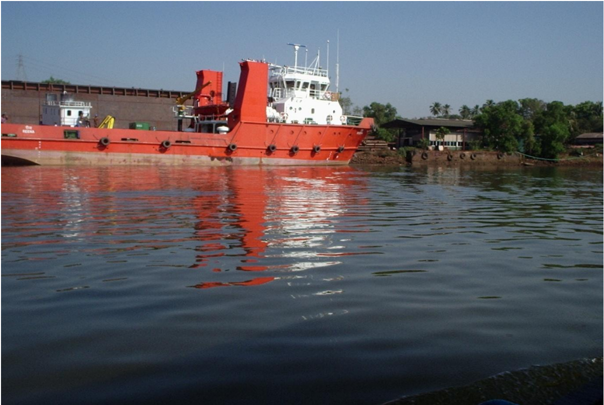
A View of Barge Construction Facility in Zuari River
