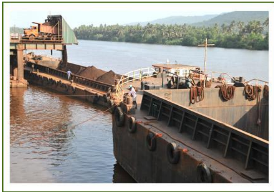
Fig.3.5: Iron ore loading from truck to barge at Jetty
