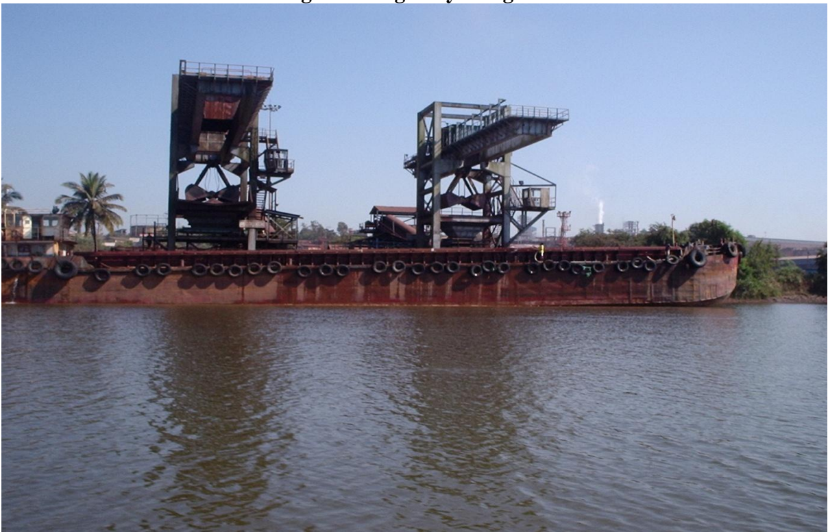
A View of Barge Loading Jetty along Zuari River
