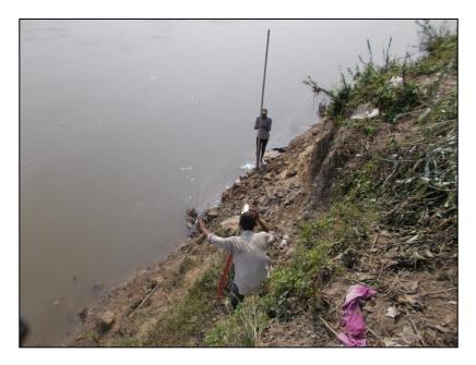
Figure 45- Erection of Tide Gauge
