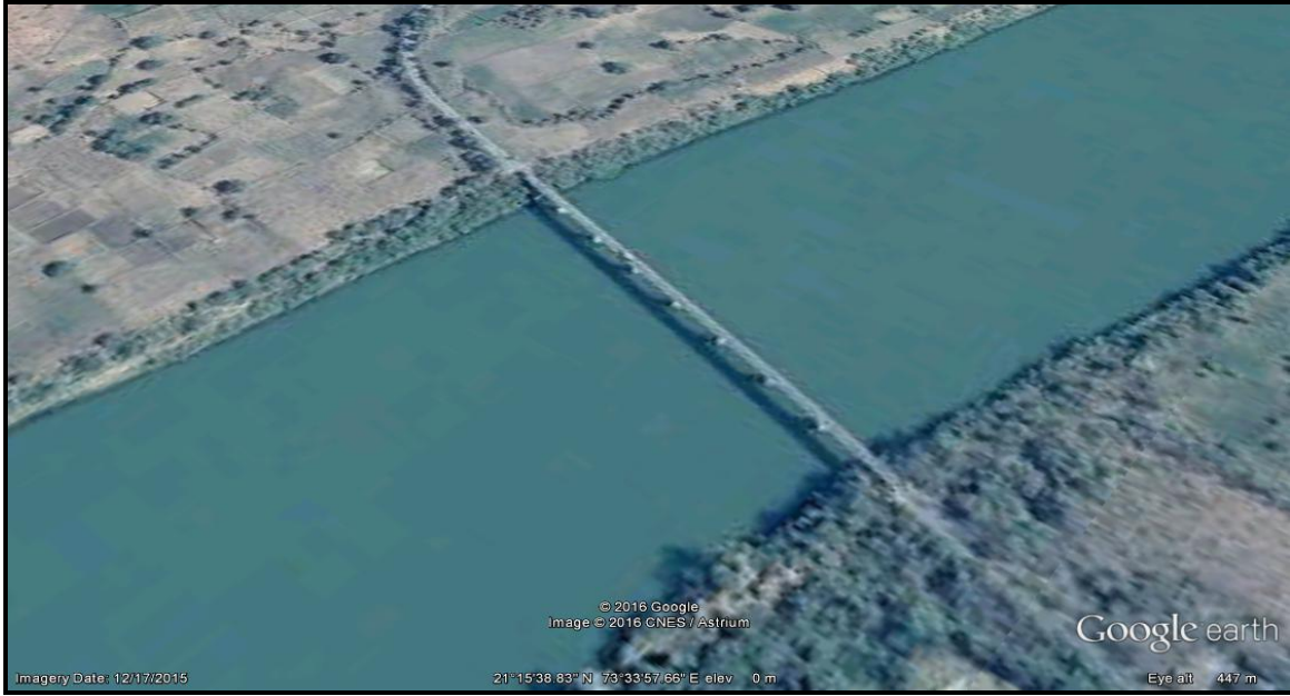
Figure 2.29 – Ch. 134.168 km Hindustan Bridge
