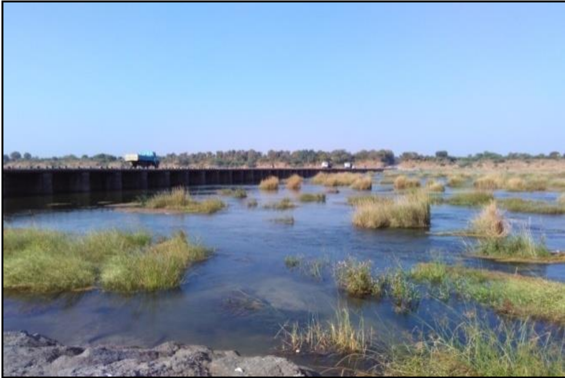
Figure 2.21 – Ch.92.891 Km Kojwa, Kadod Bridge
