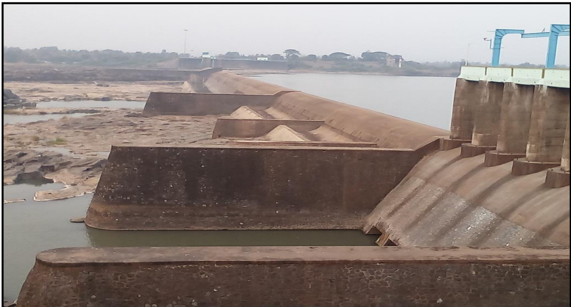
Figure 2.26 – Ch. 112.303 Km Kakrapar Weir
