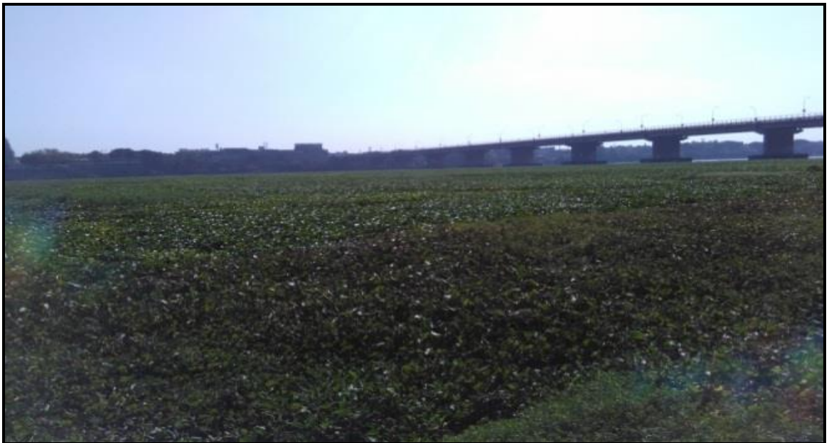
Figure 2.14 – Ch.47.061 km Kapodra-Utran Road Bridge
