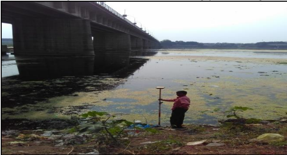
Figure 2.12 – Ch.44.332 km Amroli Bridge
