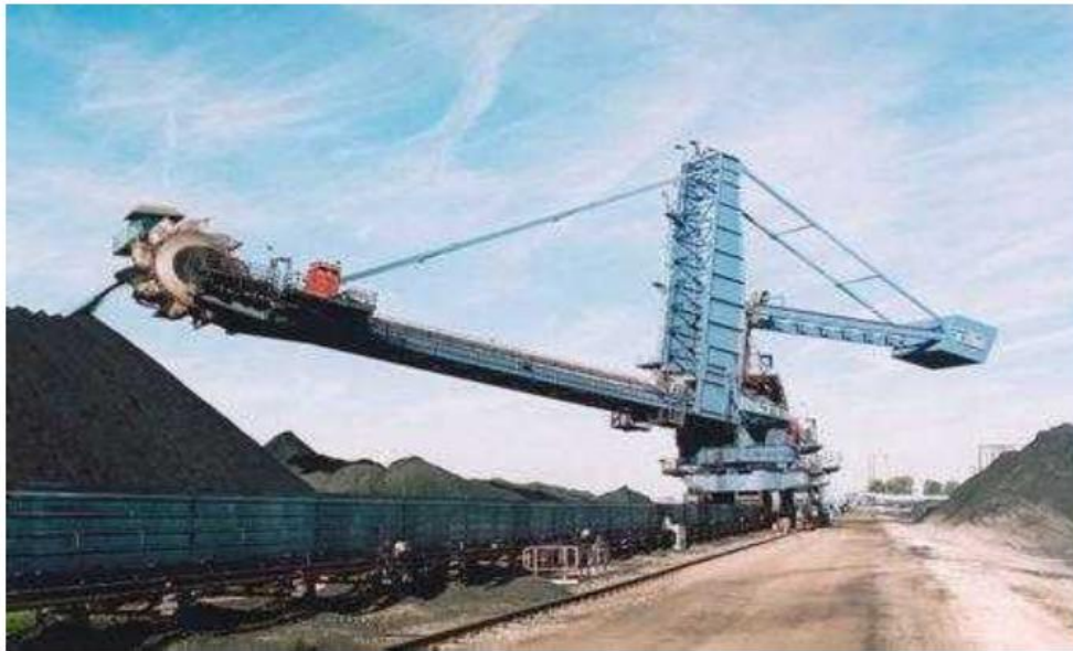
Fig No.5.8 Gantry stacker and Reclaimer
