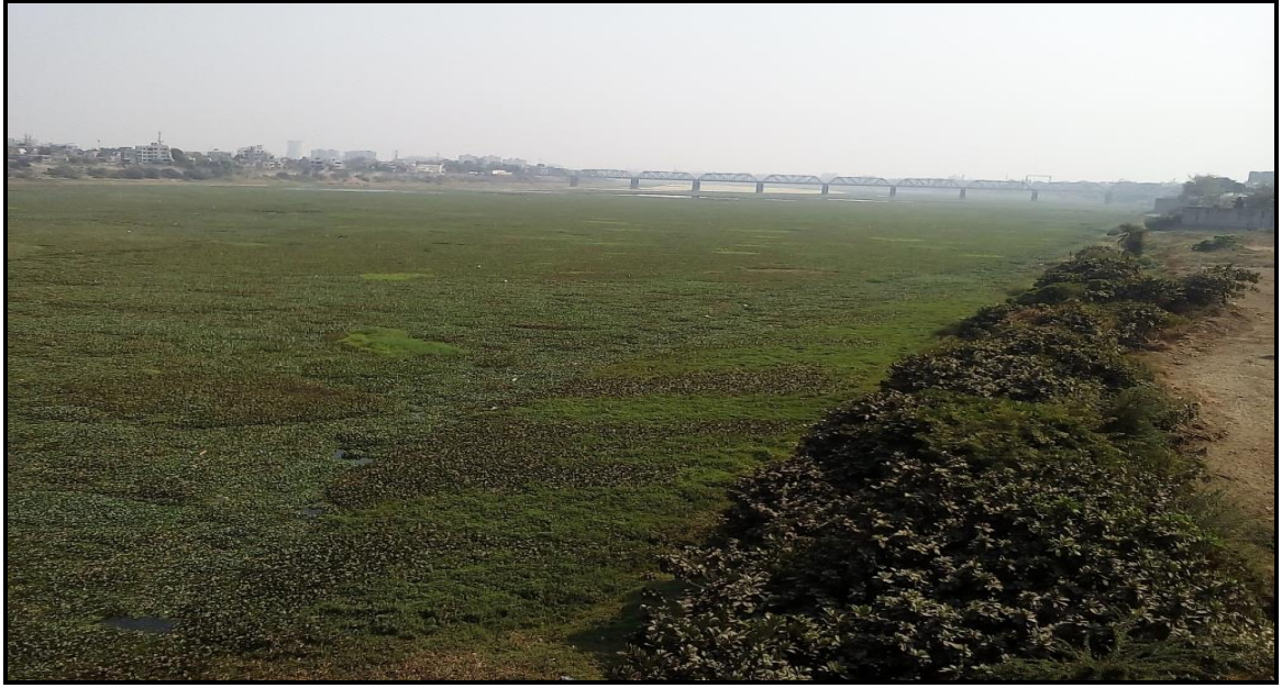
Figure 2.13 – Ch.45.373 km Railway Bridge and Hyacinth Cover on Surface of Water
