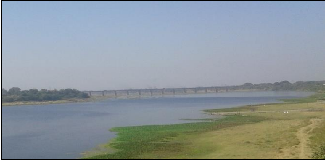
Figure 2.23 – Ch. 102.63 Km Mandvi Bridge
