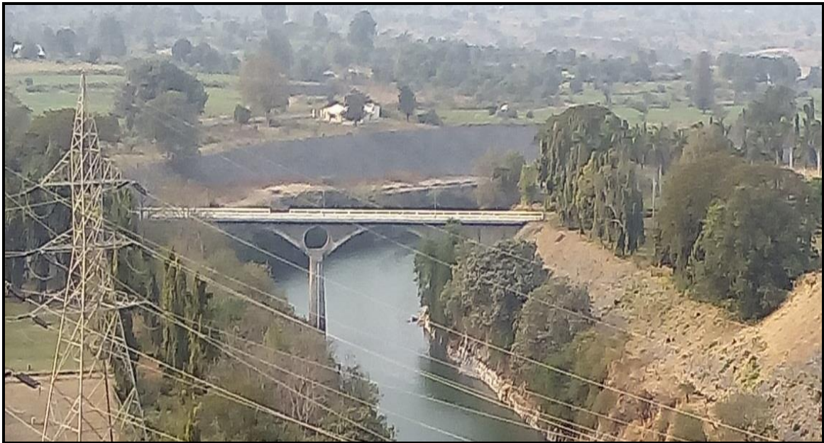
Figure 2.30 – Ch. 136.935 km Ukai Dam Canal Bridge
