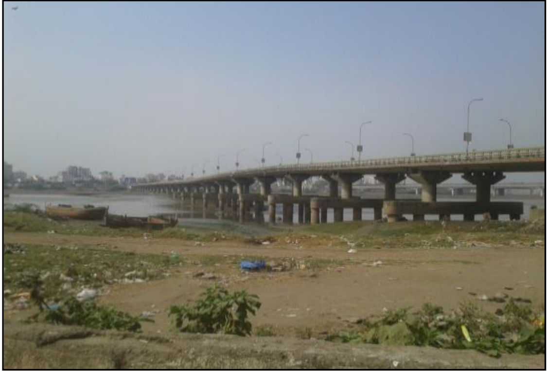
Figure 2.6 – Ch. 31.103 Makaipool Bridge (Swami Vivekanand Bridge)
