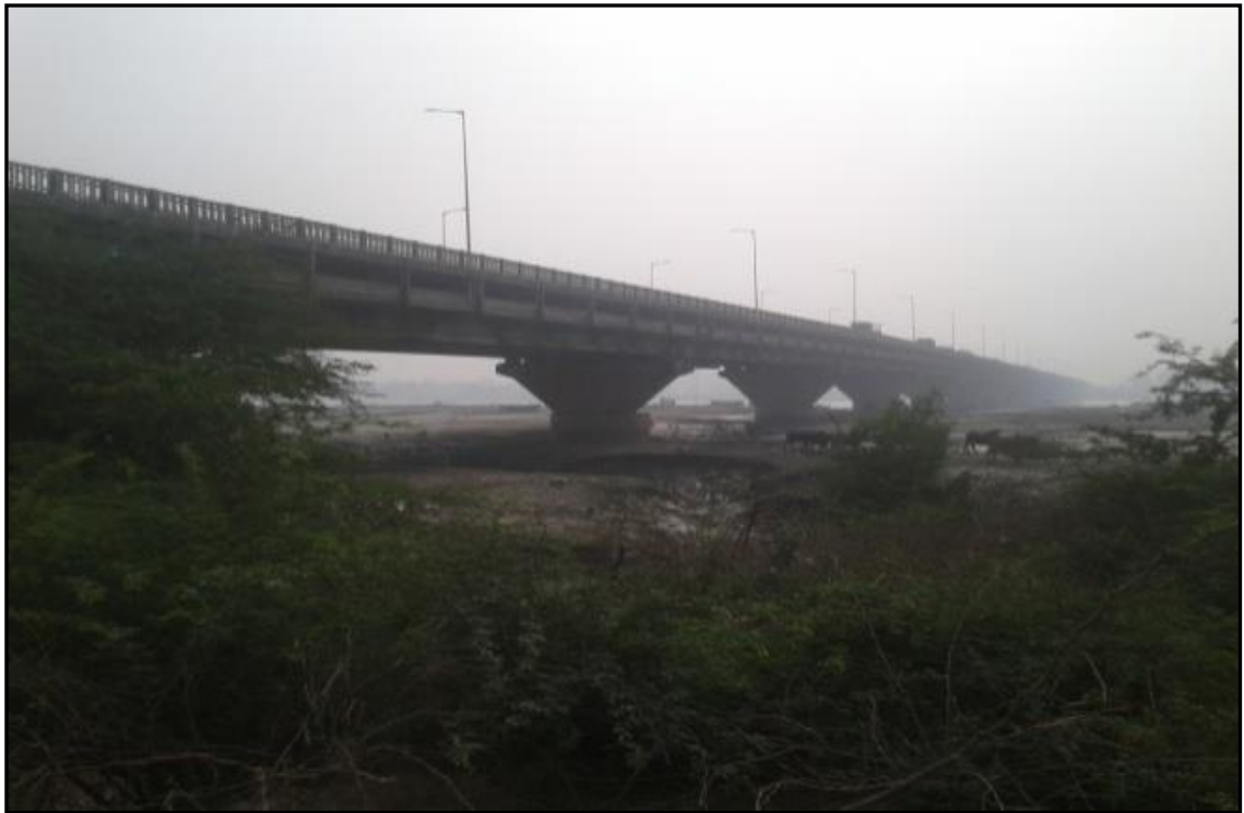
Figure 2.5 – Ch. 30.254 Sardar Bridge
