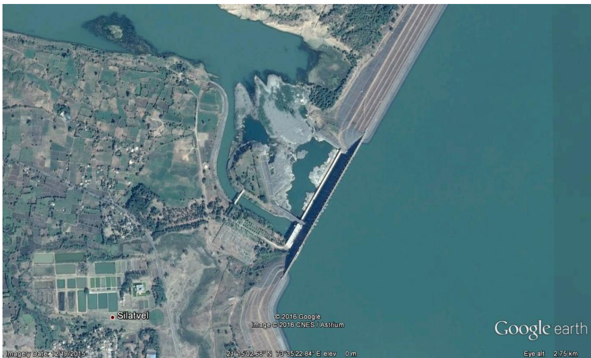
Figure 2.32 – Ch. 137.311 Km Ukai Dam with side canal
