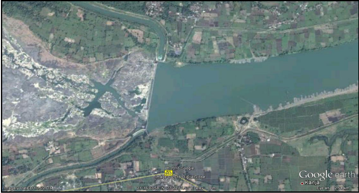
Figure 2.27 – Ch. 112.303 Km Kakrapar Weir with Canal on both bank of River
