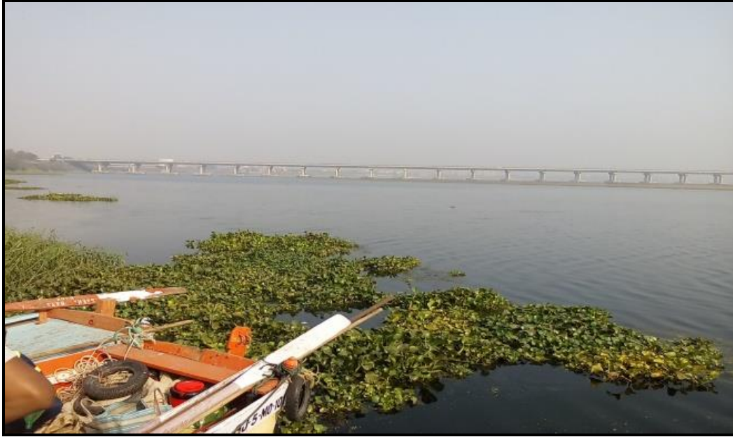
Figure 2.11 – Ch. 36.587 km Dhaboli Jahangirpura Road Bridge
