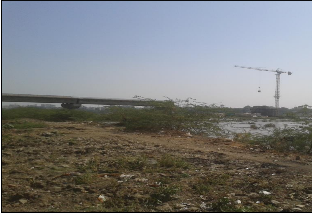
Figure 2.8 – Ch. 32.771 Adajan Patiya Bridge under Construction
