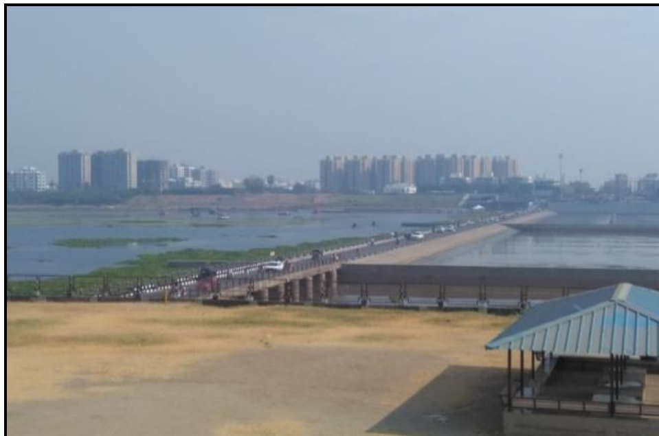
Figure 2.10 – Ch. 34.6 km Singapore Weir cum causeway
