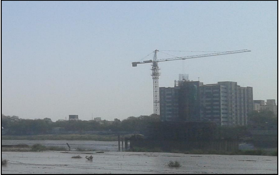
Figure 2.4 – Ch. 27.124 Under Construction Bridge at Adajan Gam
