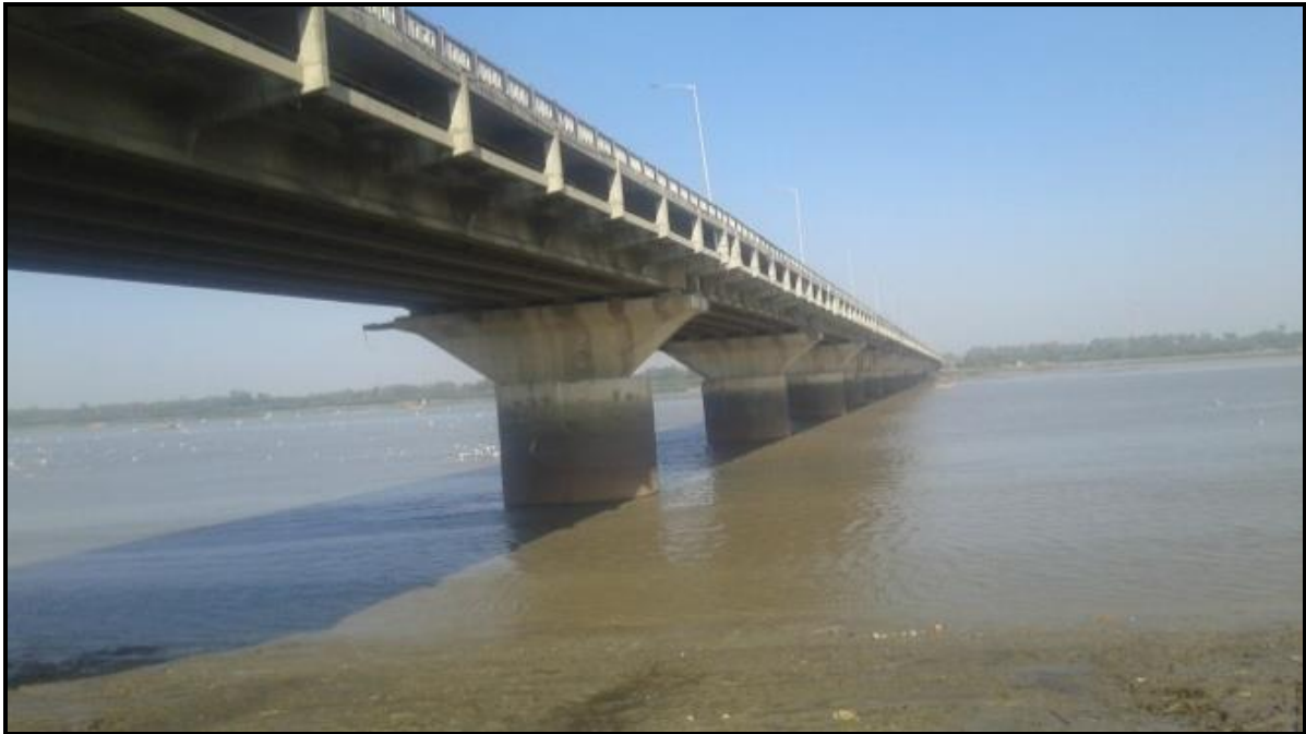
Figure 2.3 – Ch. 21.845 km ONGC Bridge between Surat City and Hazira
