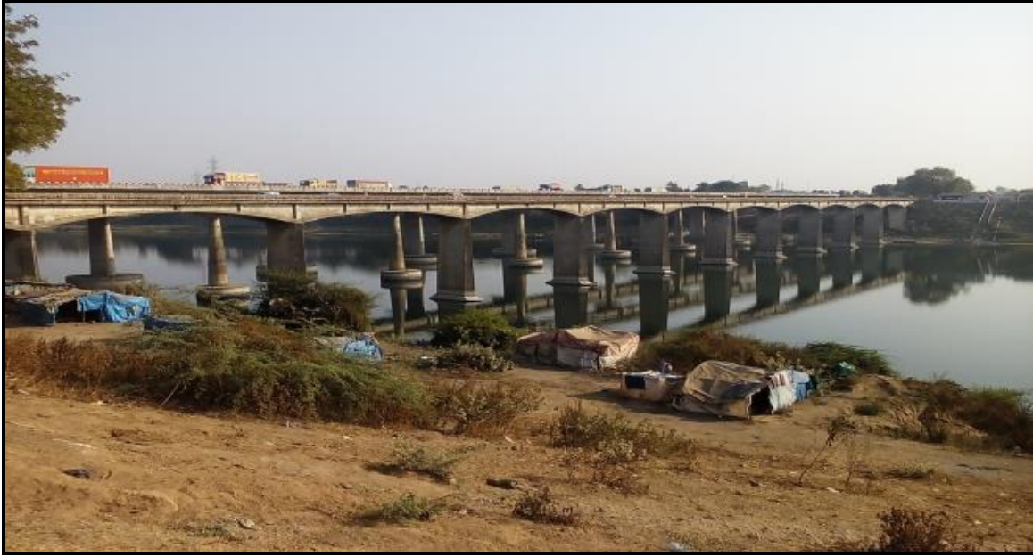
Figure 2.17 – Ch.59.27 Km National Highway No. 8 Bridge
