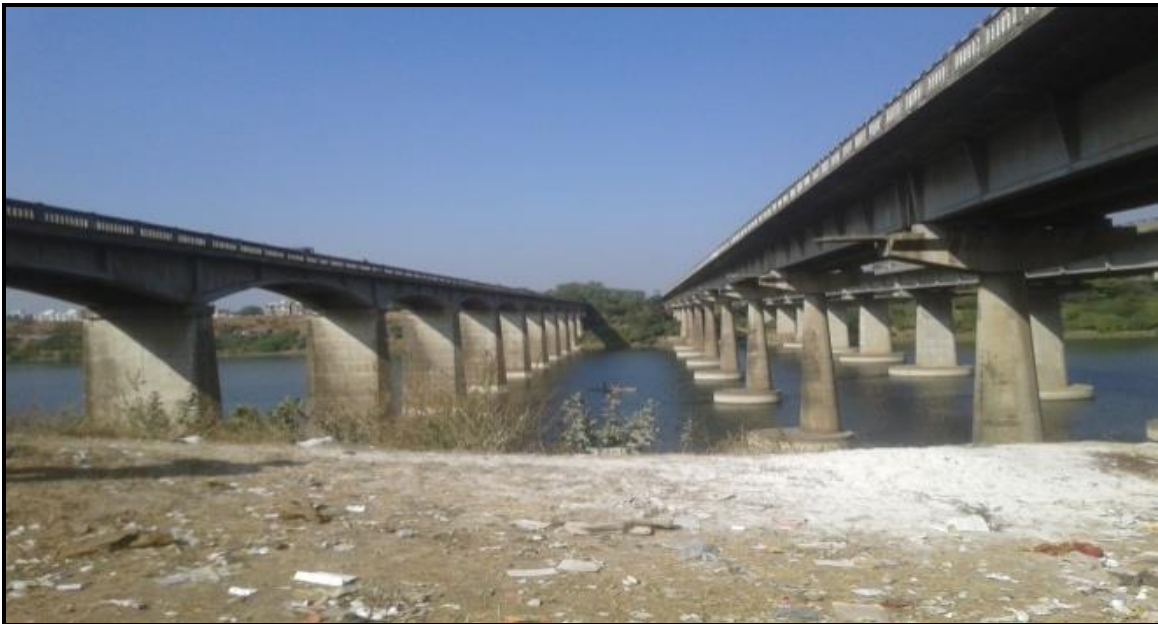
Figure 2.18 – Ch.59.27 Km National Highway No. 8 Bridge
