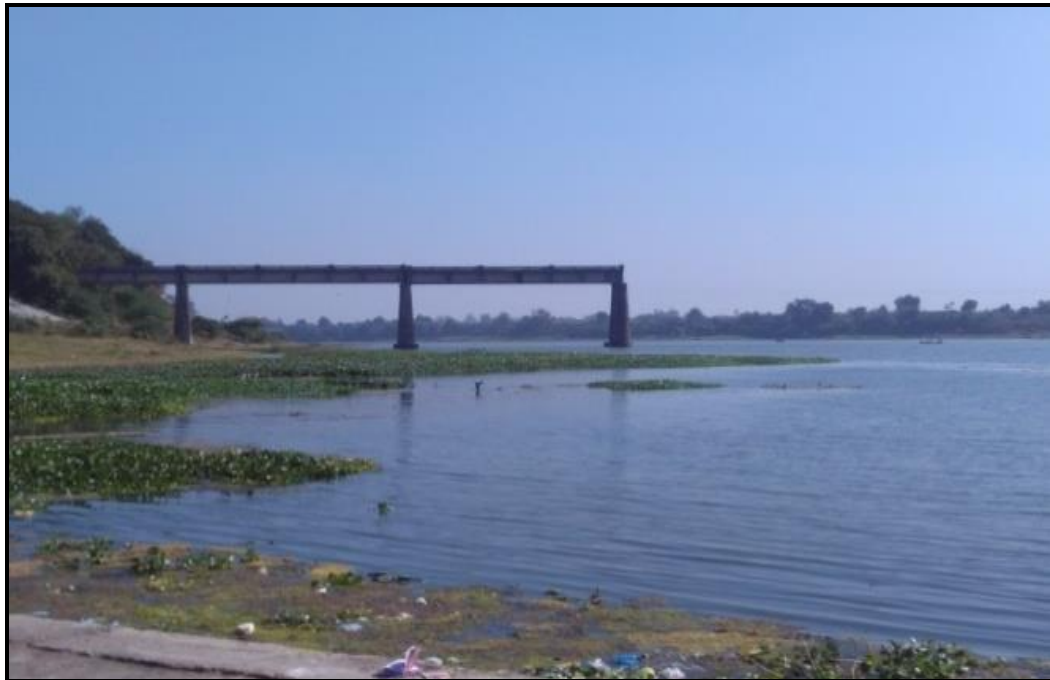
Figure 2.24 – Ch.104.0 Km Damaged Bridge
