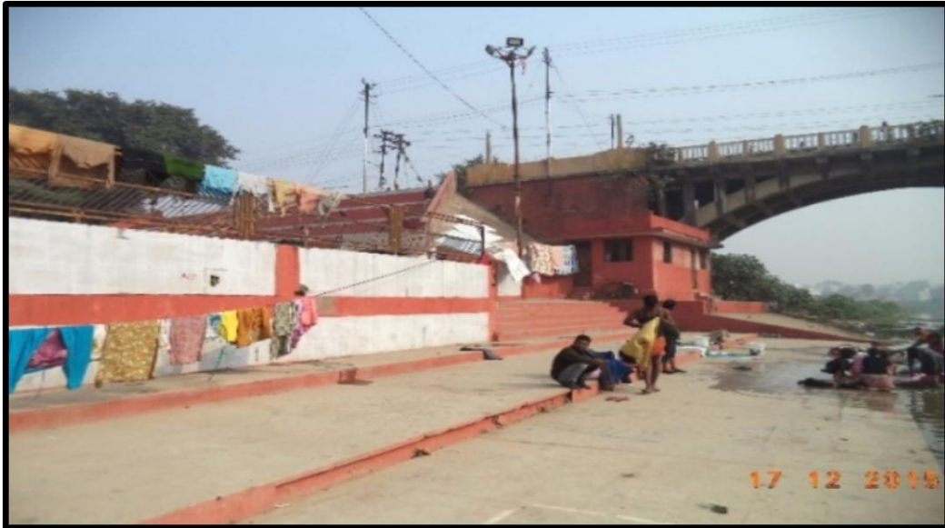
ShastriGhat at Ch. 10.3 km
