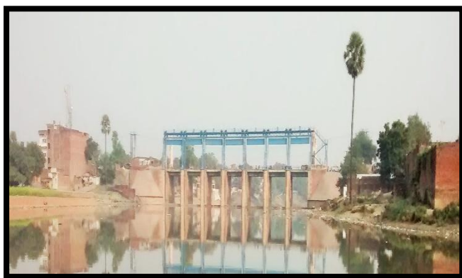
Purnanapul/Barrage at Ch 4.95 km
