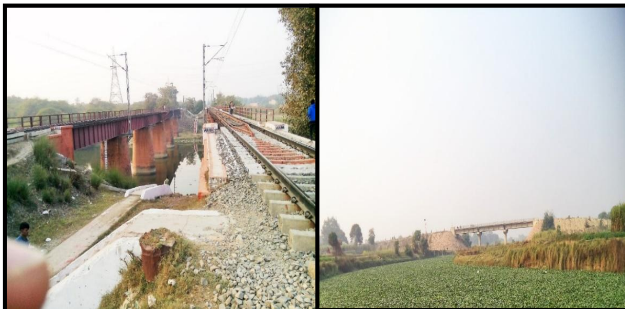
Koirawa Rail Bridge at Ch 12.86 & 12.87 km & Pissaur Bridge at Ch 17.17 km
