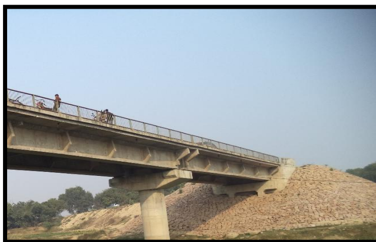
Pitch Portected under Bridge at Ch. 17.2 km
