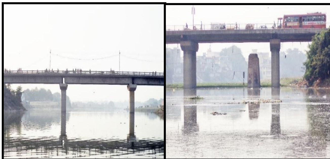
Nakkighat Bridge at Ch 6.35 km & Chaukaghat Bridge at Ch 8.35 km
