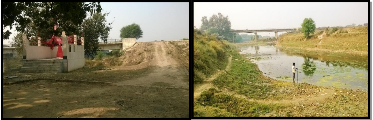
Baluwa Bridge Ch 49.75 km & Kalika Dham Bridge Ch 52.83 km
