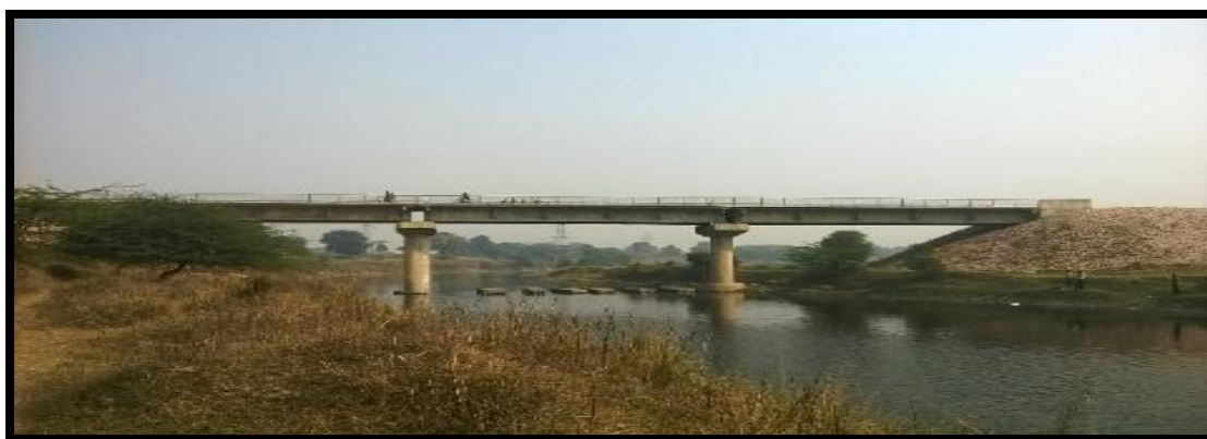
Koriyat Bridge at Ch 22.9 km
