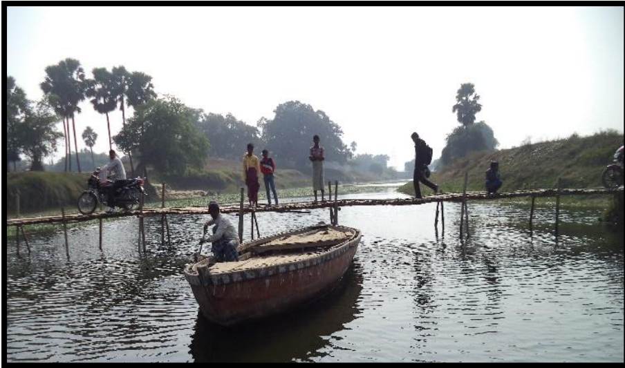
Bamboo Bridge at Ch. 19.75 km
