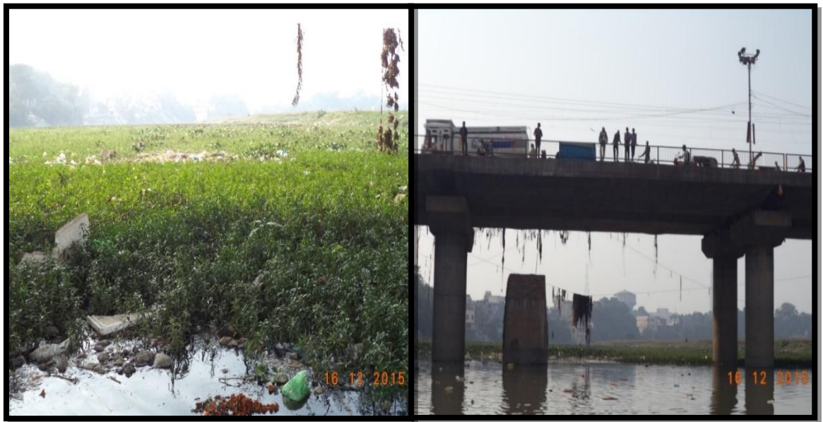
Unapproachable Part at Chauka ghat Bridge Ch. 8.35 km
