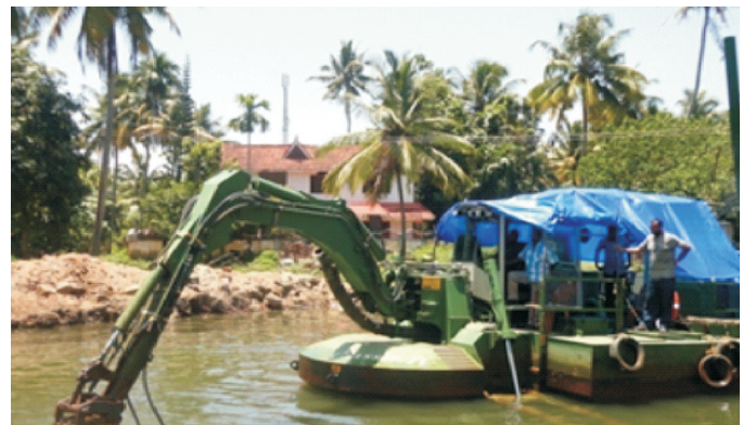
A View on the underwater breaking of hard strata by AD Manimala at Chavara.
