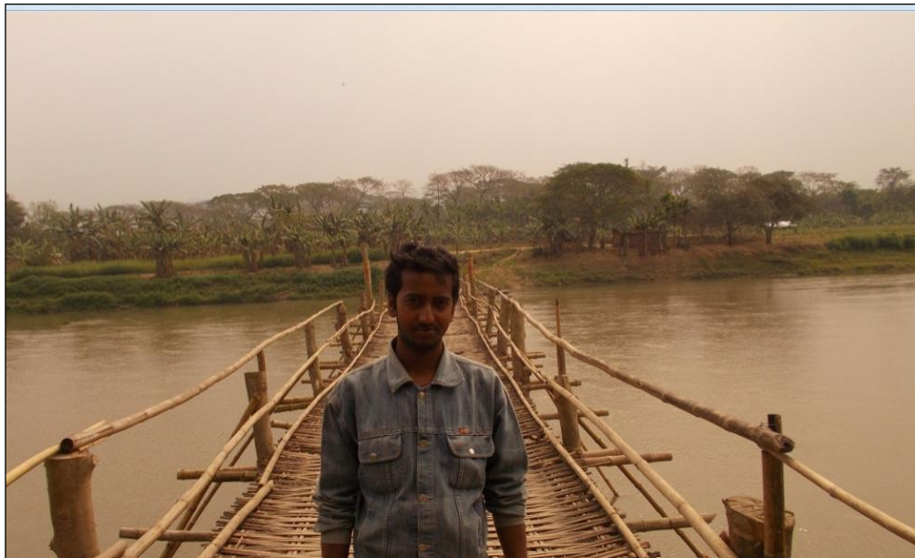
Figure 15- Bamboo Bridge (Chainage- 56.145 km and 56.968 km)
