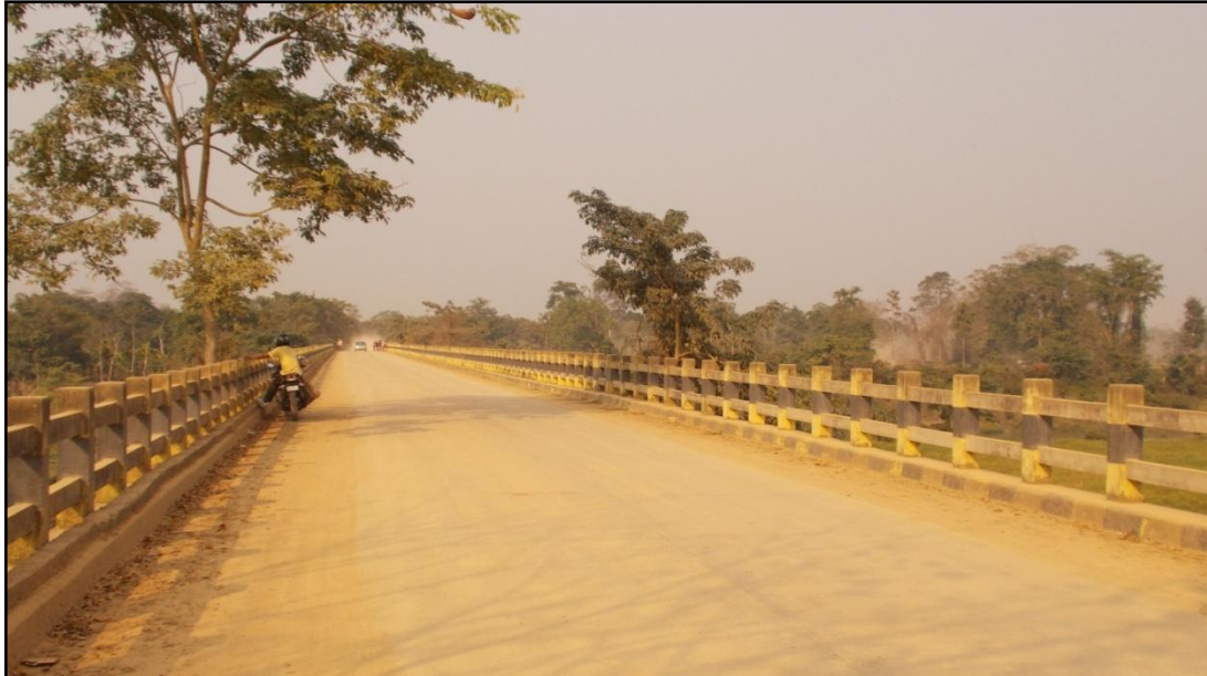
Figure 9- RCC Bridge (Chainage-14.775km)
