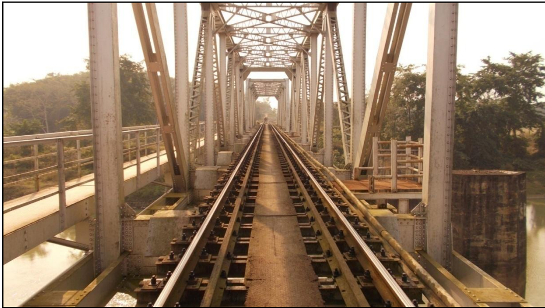
Figure 8- Rail Bridge (Chainage -14.318 km)
