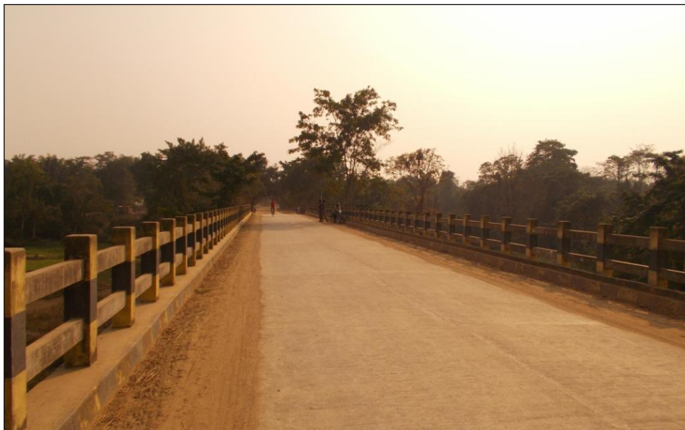
Figure 13 RCC Bridge (Chainage-44.014 km)
