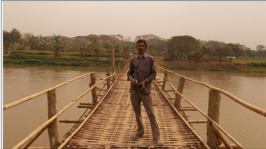
Figure 16- Bamboo Bridge (Chainage – 61.318 km)
