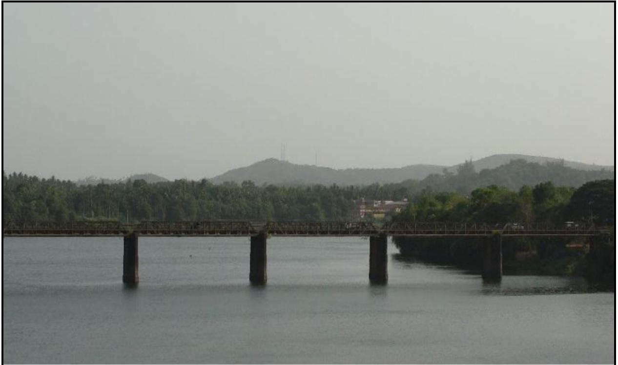
Photo 17: Bridge on Mysore Highway at Ch 28.00km
