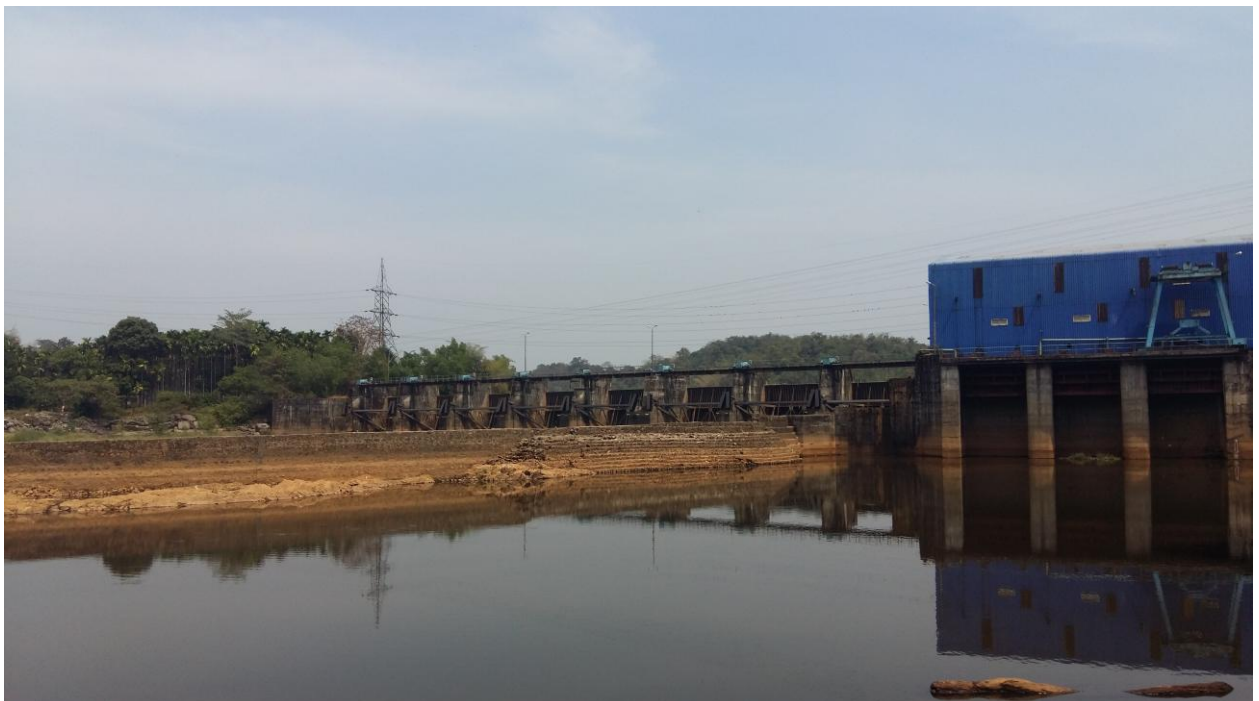
Photo 26: Sagar Power Pvt. Ltd Dam at Ch 64.60km
