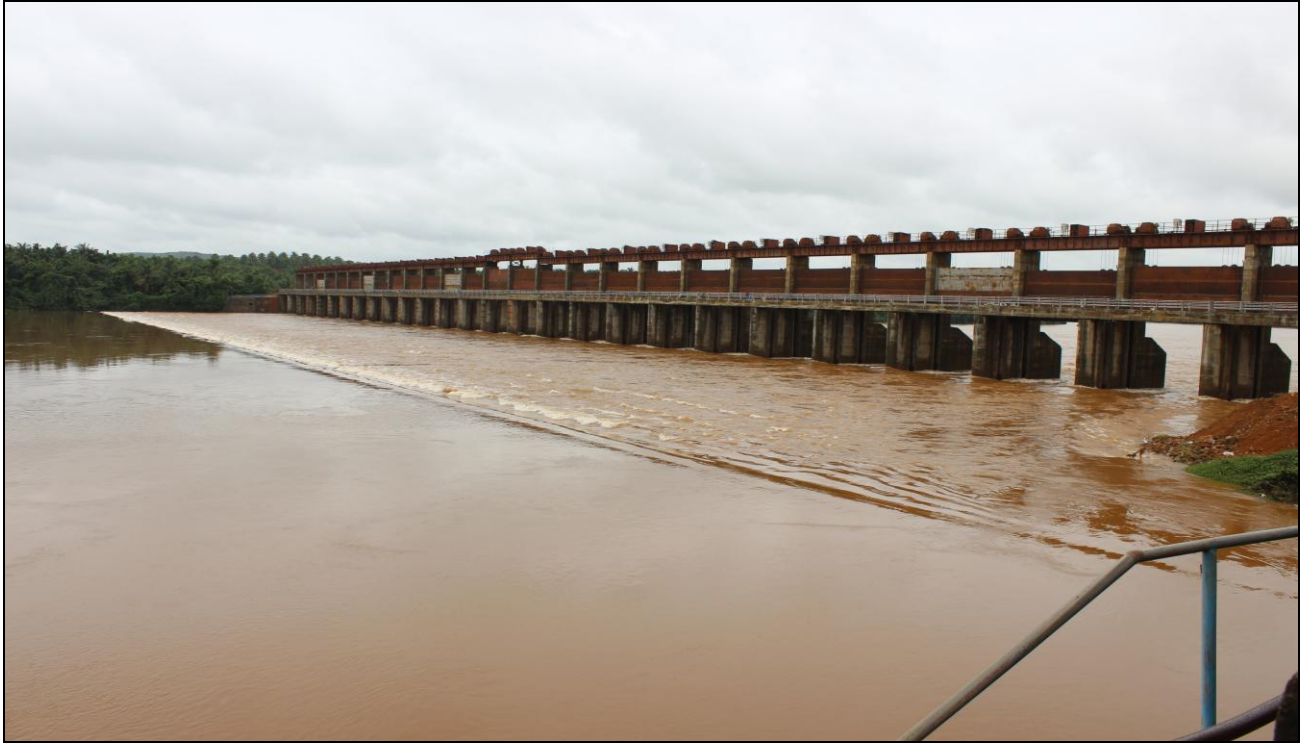
Photo 13: Thumbe Barrage at Ch 23.50km
