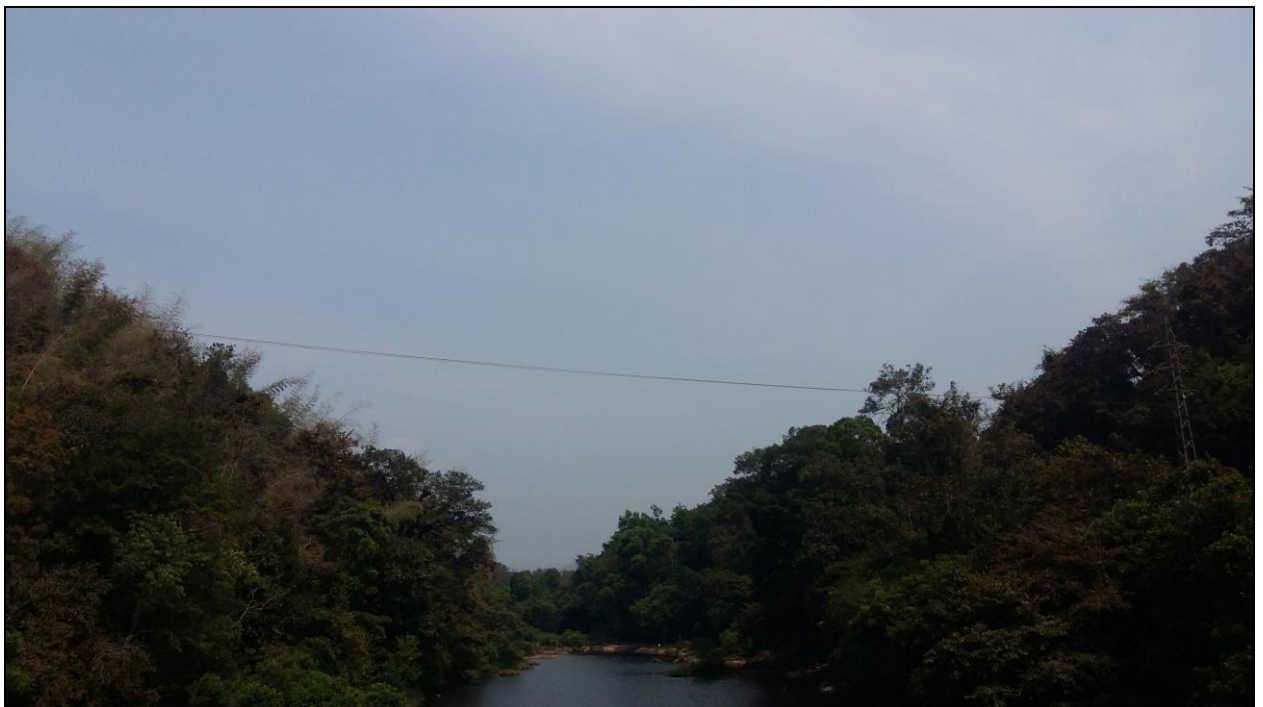
Photo 28: LT Line at Ch 74.50km
