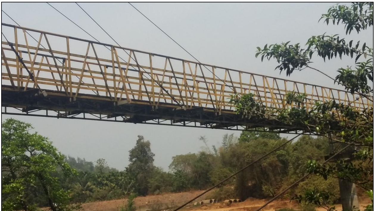
Photo 24: Foot over Bridge at Ch 62.45km
