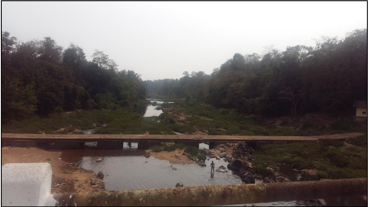
Photo 31: Old Bridge, Dhramsthala at Ch 80.00km
