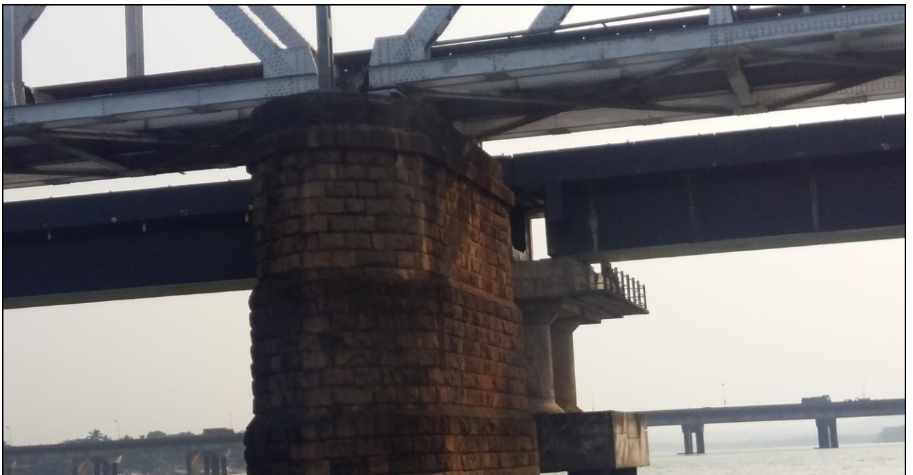
Photo 4: Railway Bridge at Ch 3.44km
