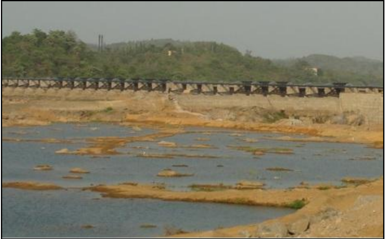
Photo 19: AMR Power Pvt. Ltd DAM at Ch 36.00km
