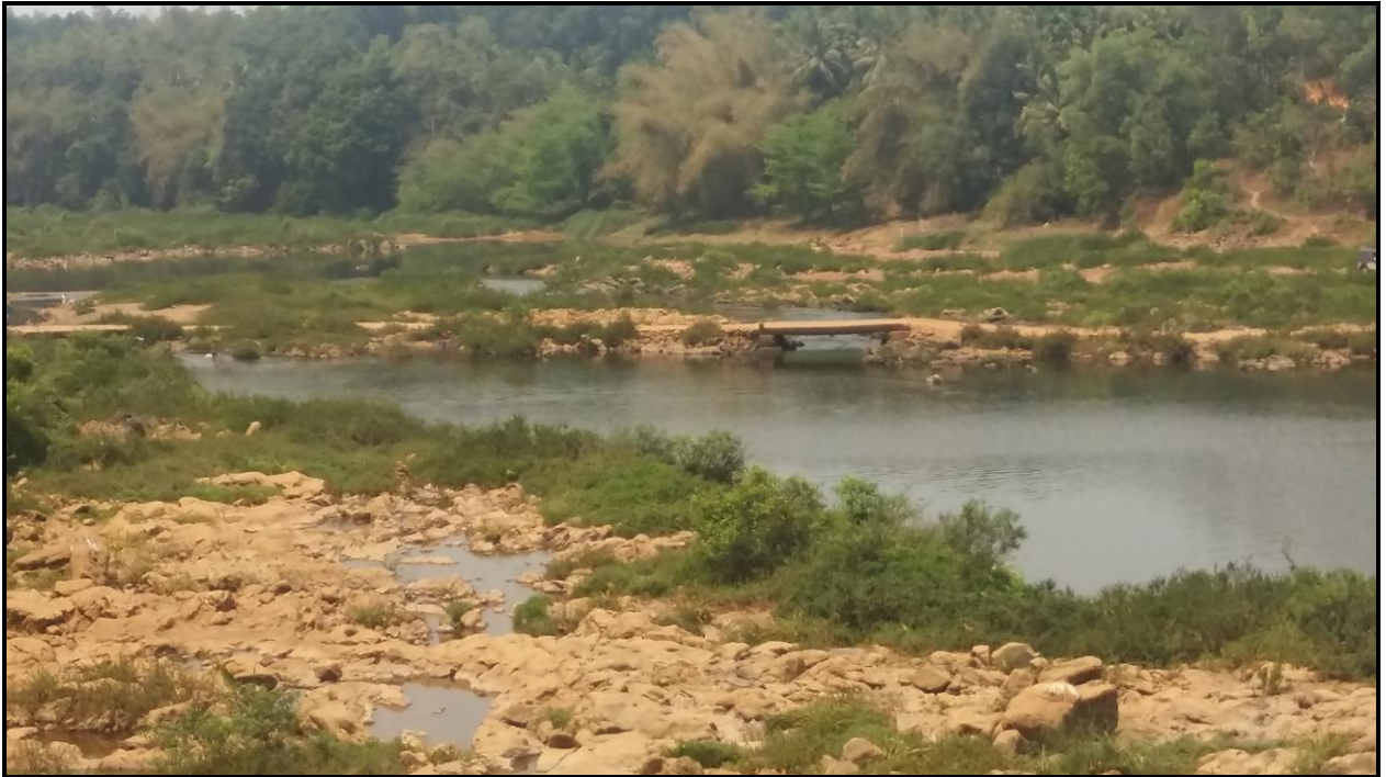
Photo 23: Bridge at Ch 62.30km
