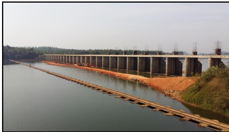
Figure 2.1: Karnataka Urban Water Supply & Drainage Board Dam
