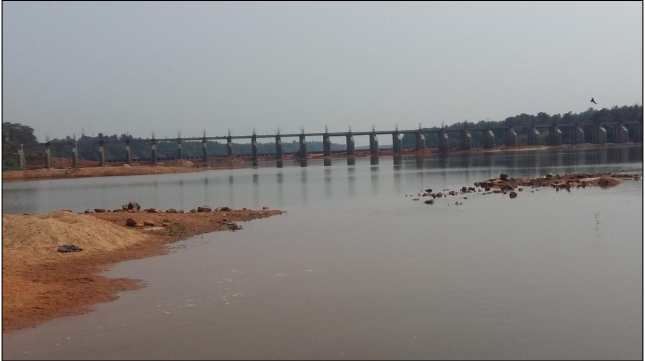
Photo 11: Karnataka Urban Water Supply & Drainage Board (Thumbe Barrage) at Ch 23.50km
