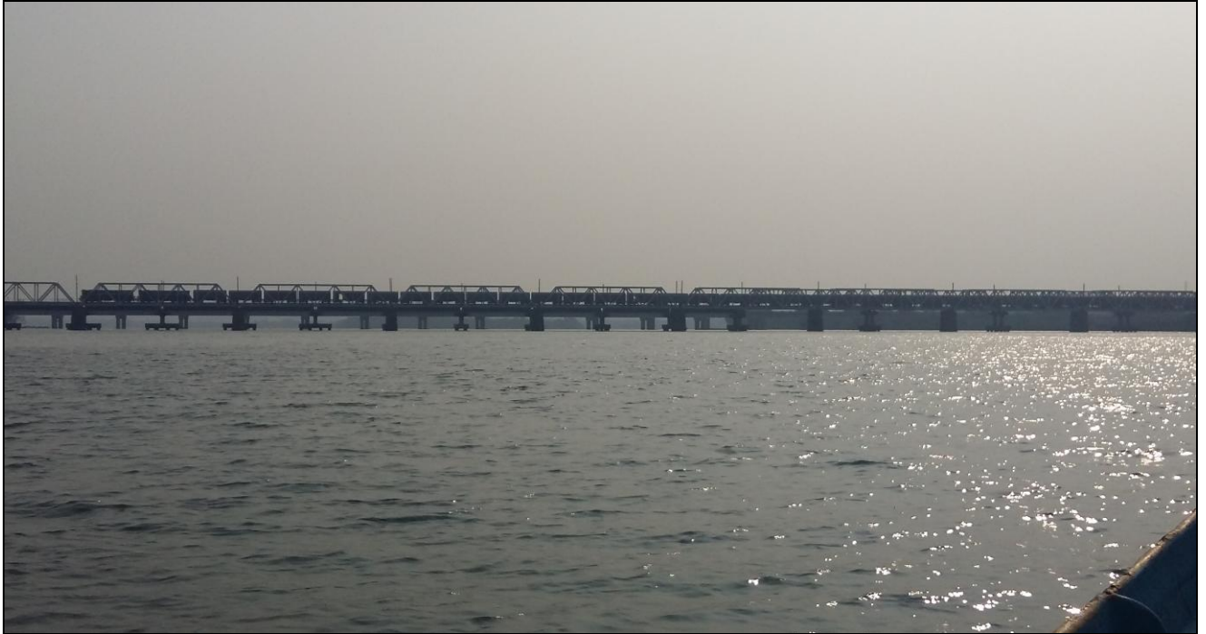
Photo 3: Railway Bridge at Ch 3.43km
