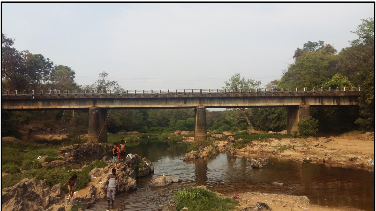
Photo 32: New Bridge, Dhramsthala at Ch 80.14km
