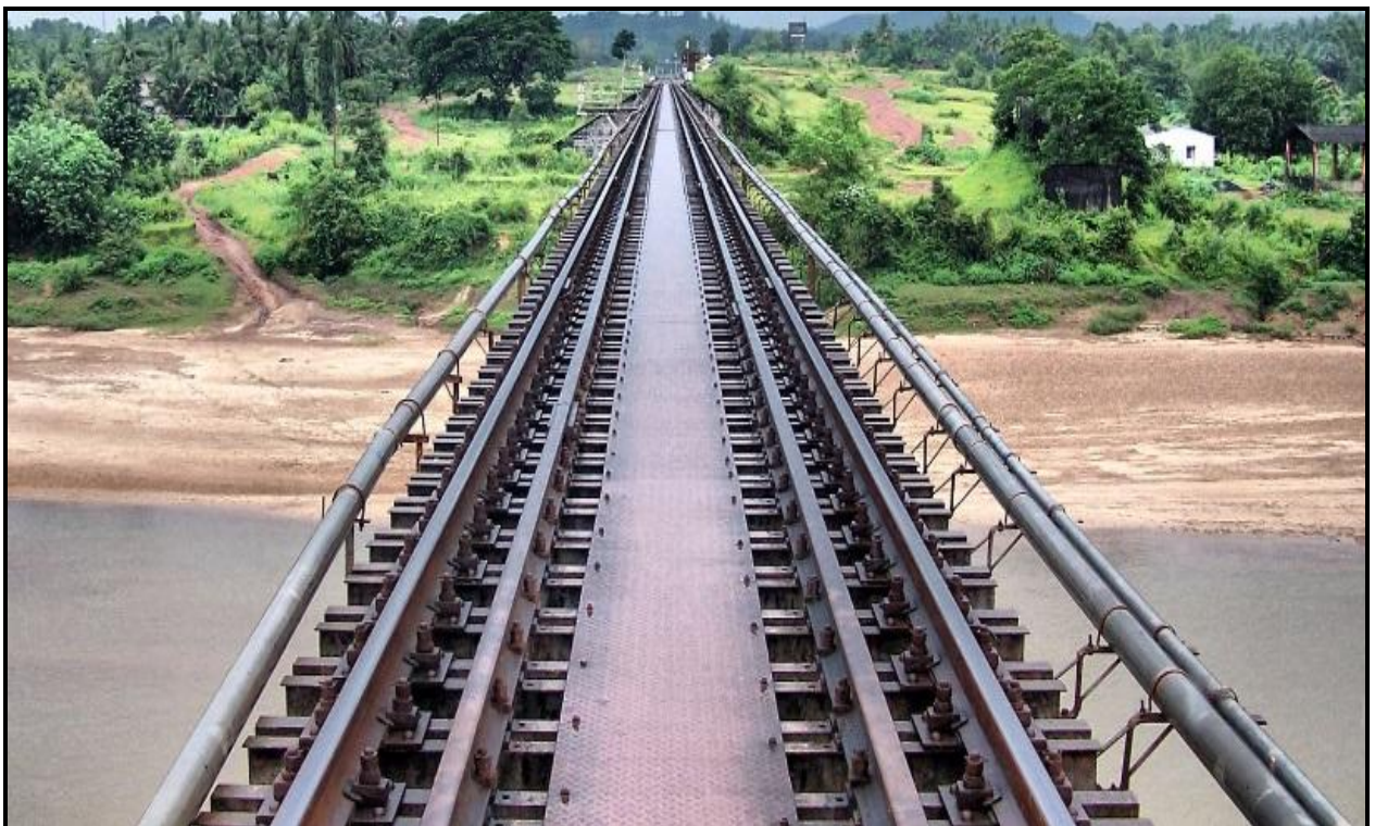
Photo 16: Railway Bridge at Ch 27.05km
