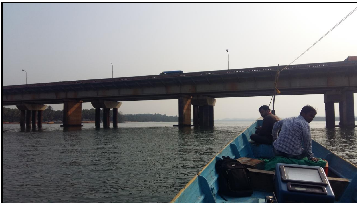
Photo 5: Bridge on Mumbai Highway at Ch 3.82km
