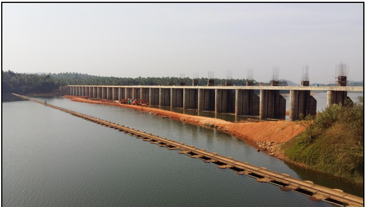
Photo 12: Karnataka Urban Water Supply & Drainage Board,(Thumbe barrage) at Ch 23.50km
