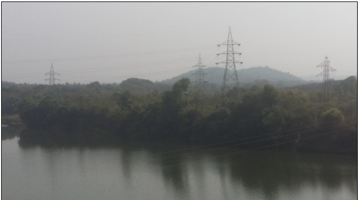
Photo 18: Transmission Line at Ch 28.50km
