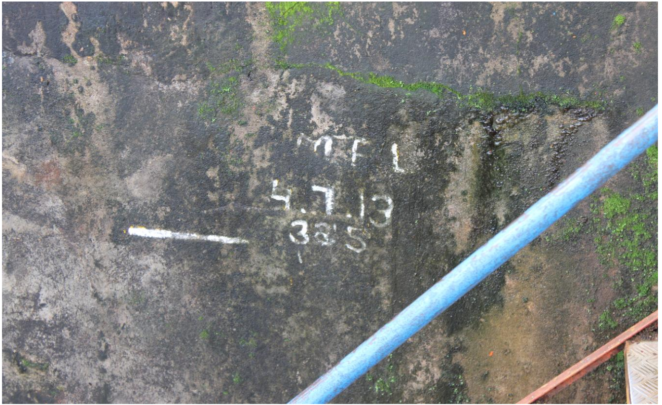
Photo 15: Maximum Flood Level of 38.5 Ft. Dated 04/07/1974 Mark near Thumbe Barrage at Ch 23.50km
