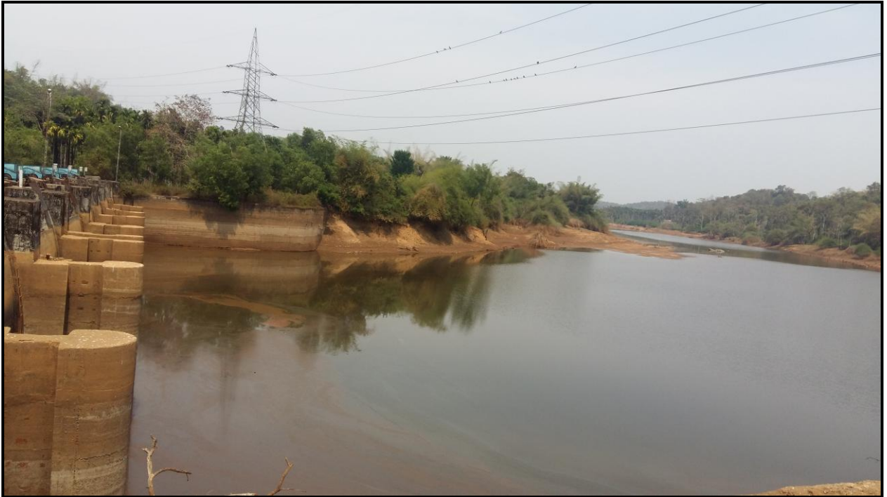
Photo 27: Transmission Line at Ch 64.75km
