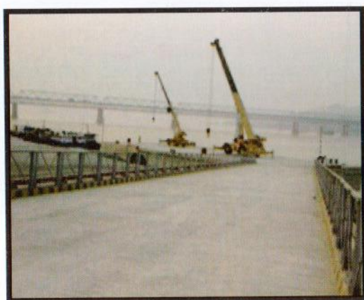
RCC Jetty at Pandu Port with cranes
