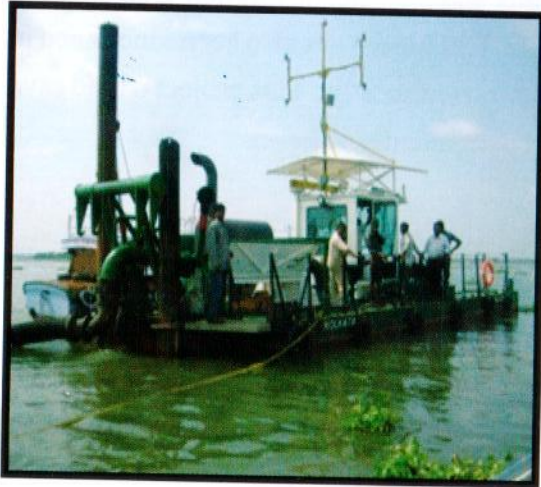
Dredging in NW-3 with CSD Kallada
