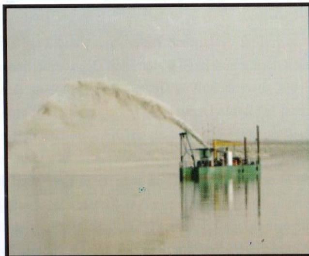
Dredging in progress with CSD on NW-1
