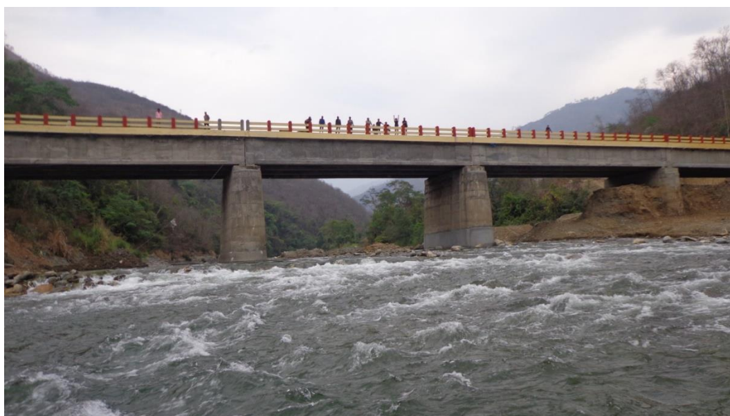
Figure 9 View of Lahori Bridge in Tizu River
