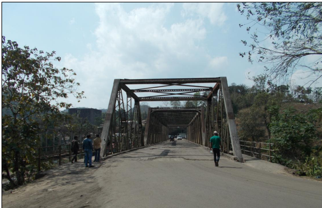
Figure 13- RCC Bridge (Chainage- 62.480 km)
