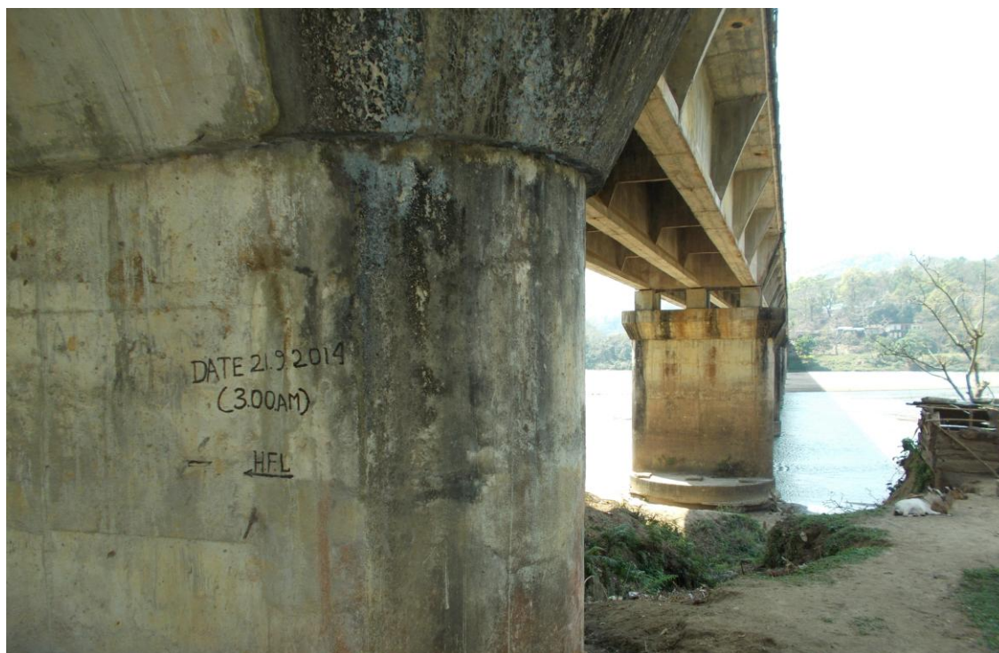
Figure 7- RCC Bridge (Chainage- 3.628 km)
