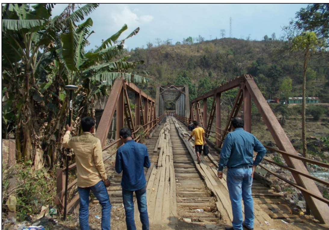
Figure 14- Wooden Bridge (Chainage- 62.500 km)
