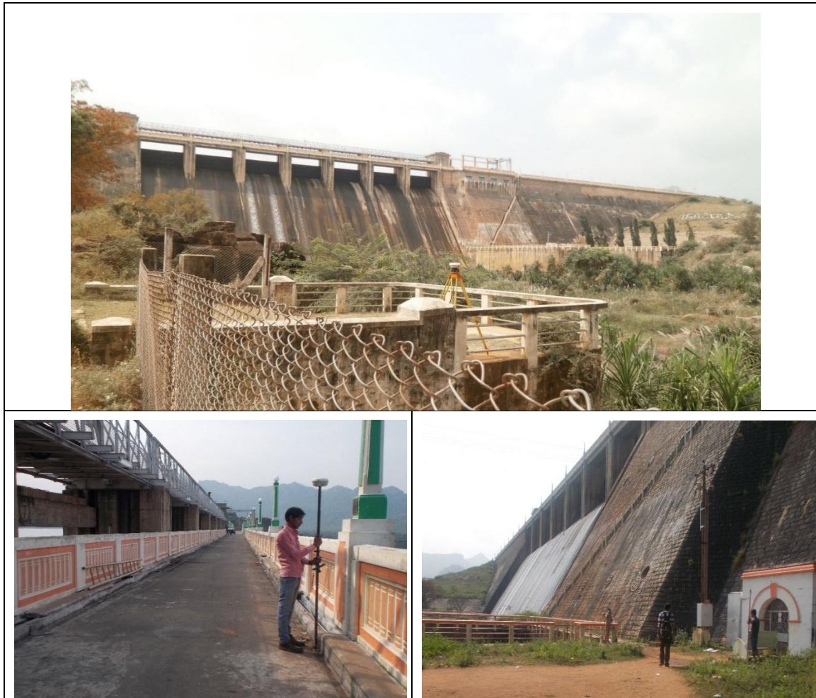
Figure 7 - View of Manimuthar Dam
