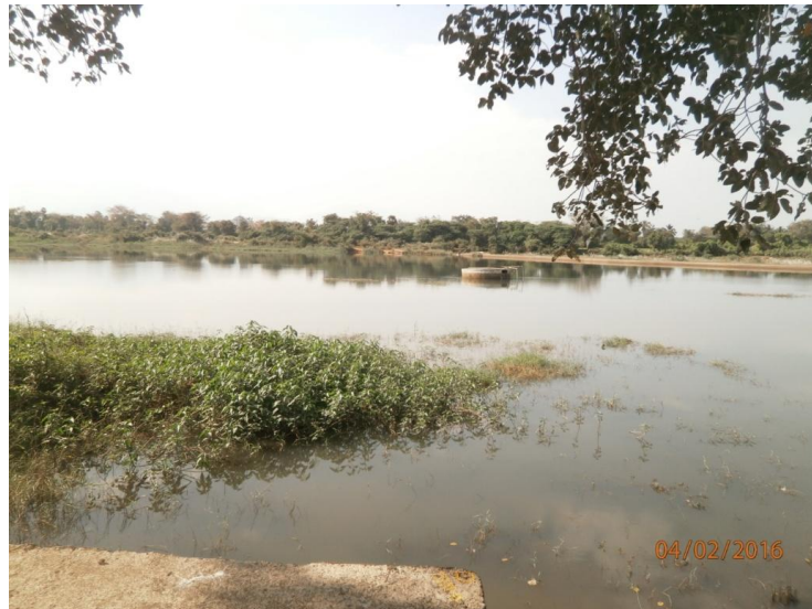
Figure 12 - View of Kanadian Spillage from the RBS (0.0 km chainage)
