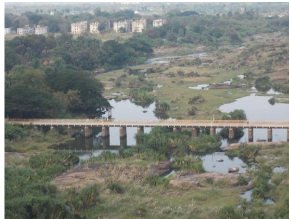
Figure 9 - Manimuthar Bridge (4.53 km chainage)
