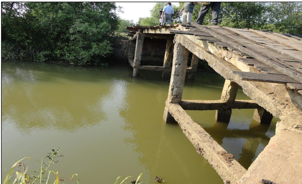
Photo 34 : Wooden Bridge with Concrete Pillars
