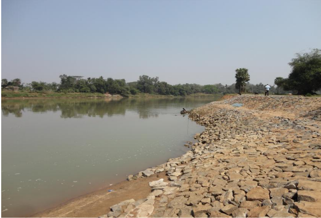
Photograph No. 13-5 Bank Protection along the river
