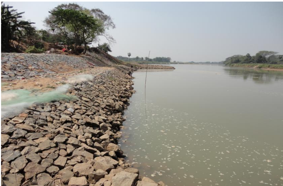
Photograph No. 13-5 Bank Protection along the river
