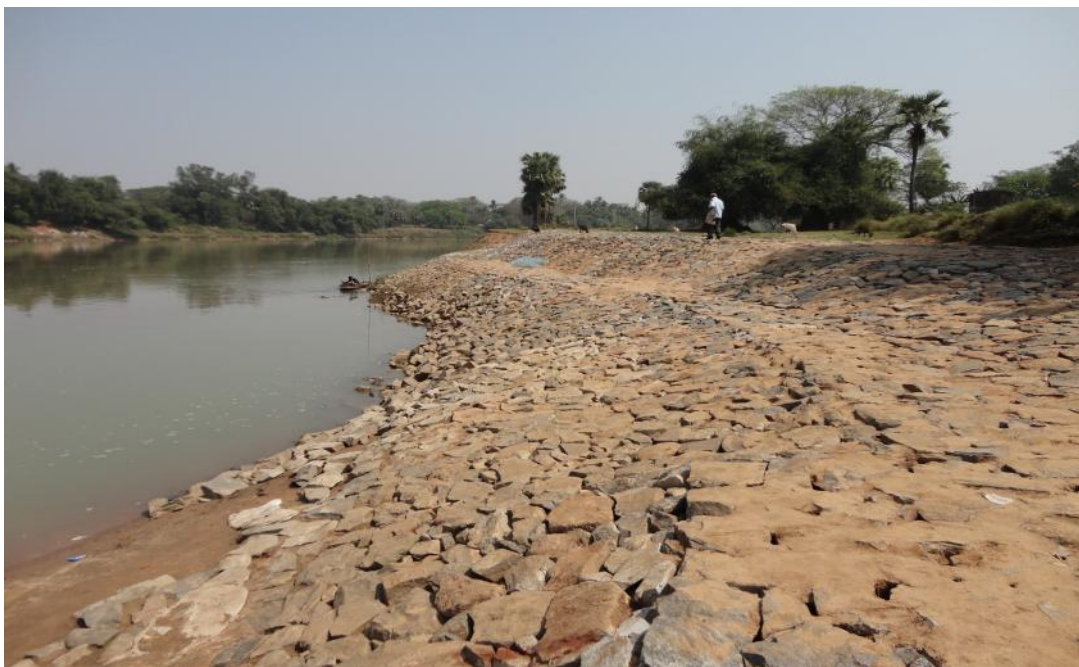
Photograph No. 13-3 Bank Protection along the river
