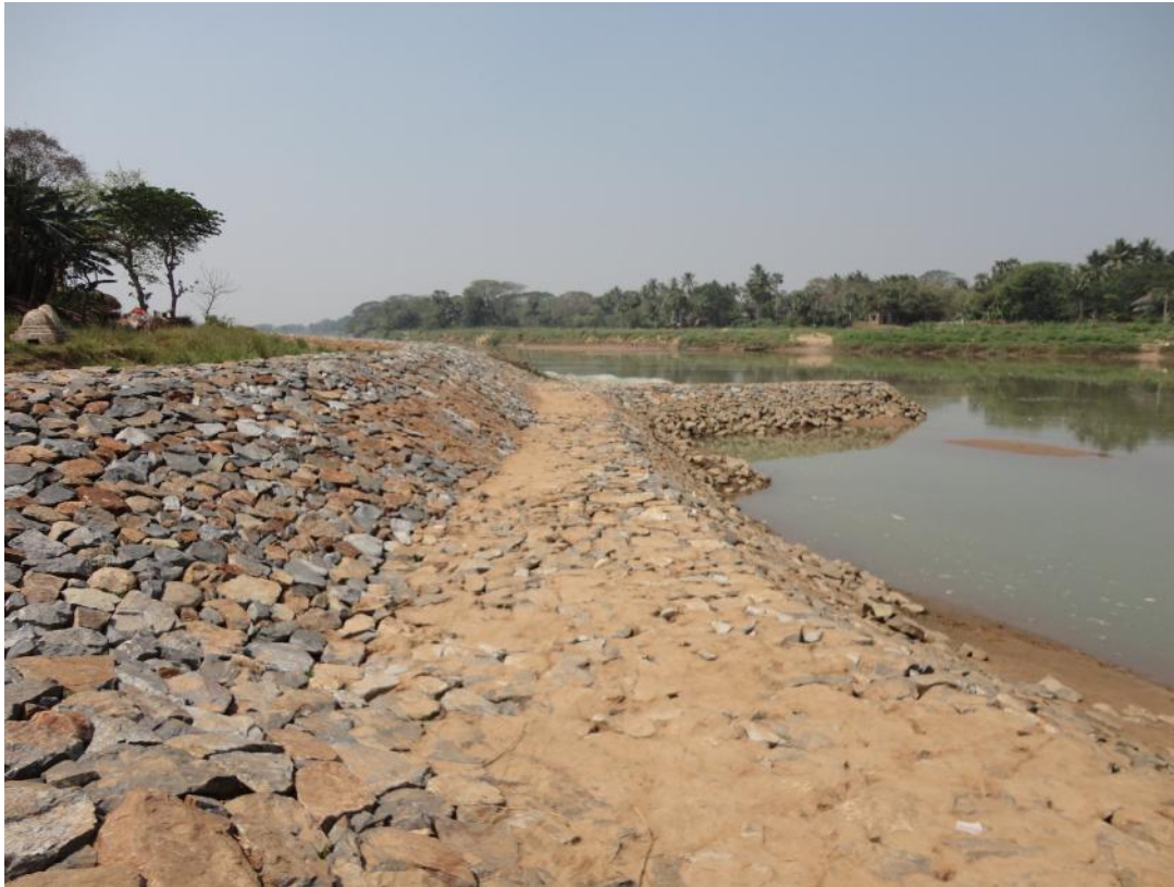
Photograph No. 13-3 Bank Protection along the river
