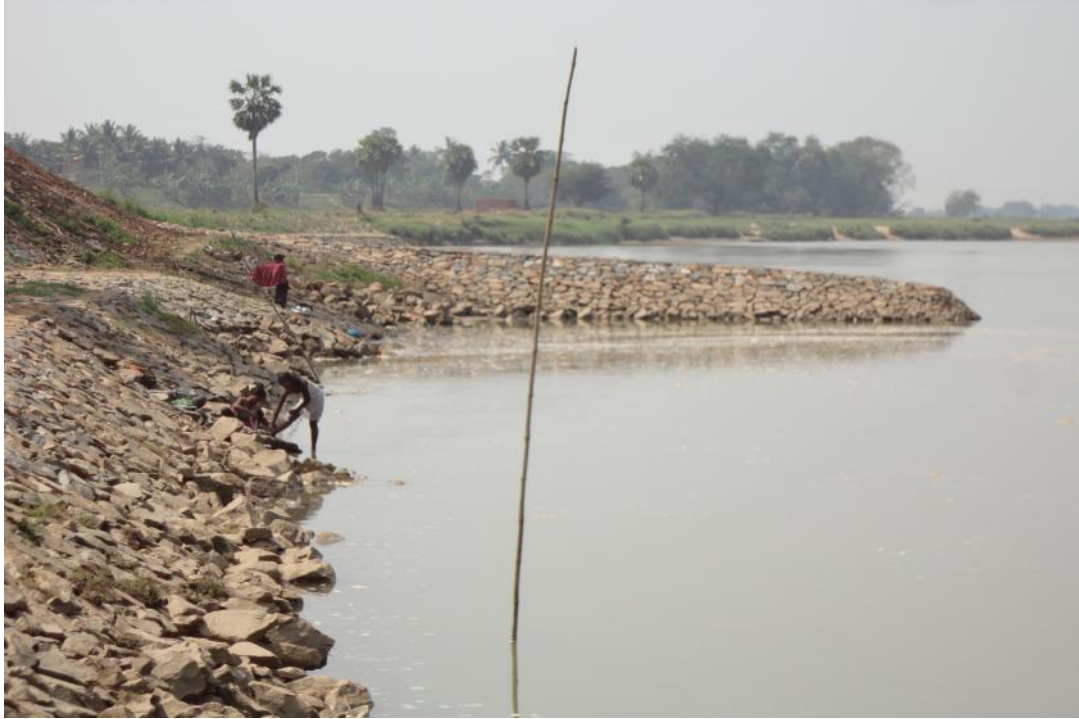
Photograph No. 13-6 Bank Protection along the river
