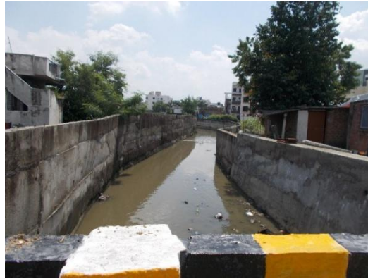
Figure 17 - View of Nag River in City area (58.129 km chainage)
