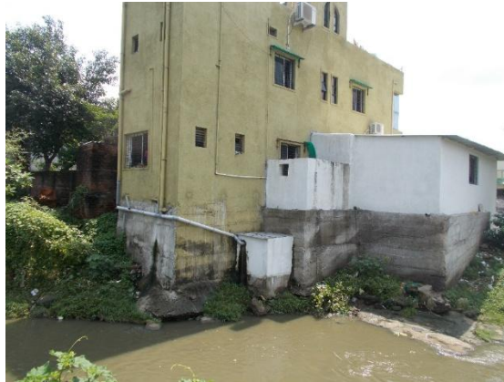
Figure 16 - Constructions on the waterway area (21° 5'44.81"N, 79° 6'20.41"E) (57.5 km chainage)
