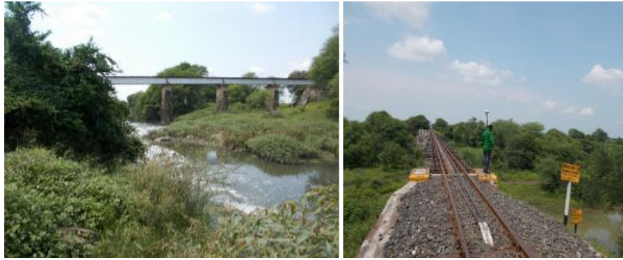
Figure 11 - Titur Railway Bridge (30.534 km chainage)
