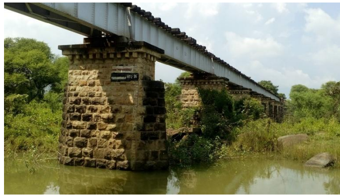
Figure 4 - HFL Marking on Titur Railway Bridge (30.53 km chainage)
