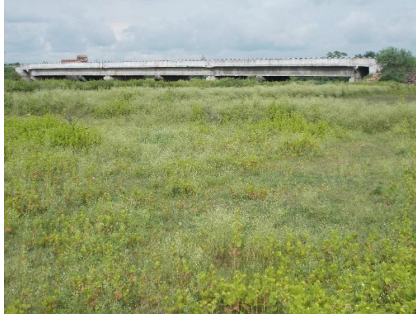
Figure 15 - View of Outer Ring Road Bridge (46.983 km chainage)
