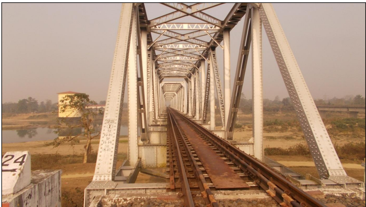
Figure 26 Rail Bridge (Chainage-109.136km)
