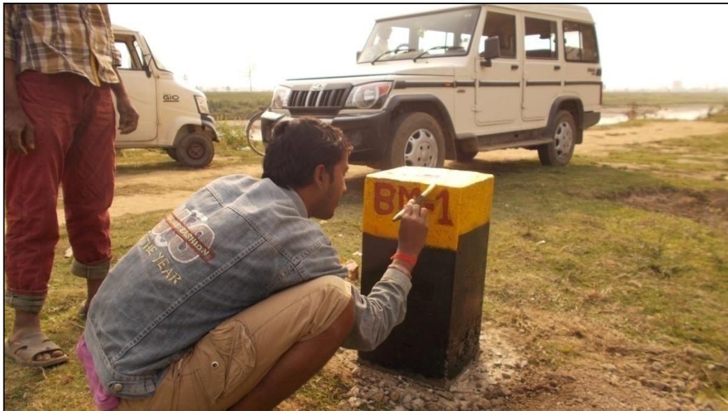
Figure 41-B.M Pillar Establishment
