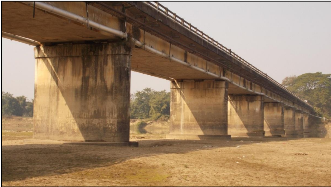
Figure 15 RCC Bridge (Chainage-54.586km)
