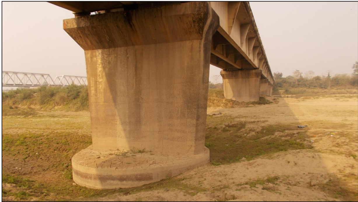
Figure 27 RCC Bridge (Chainage- 108.730 km)
