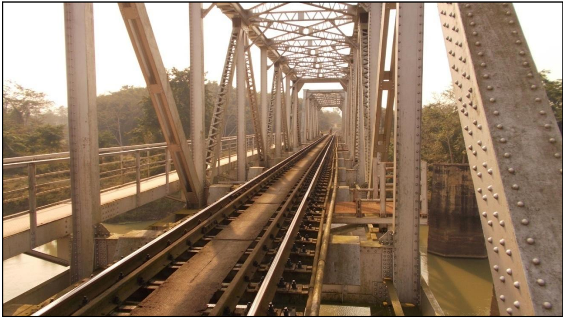
Figure 25 Rail Bridge (Chainage-102.625km)
