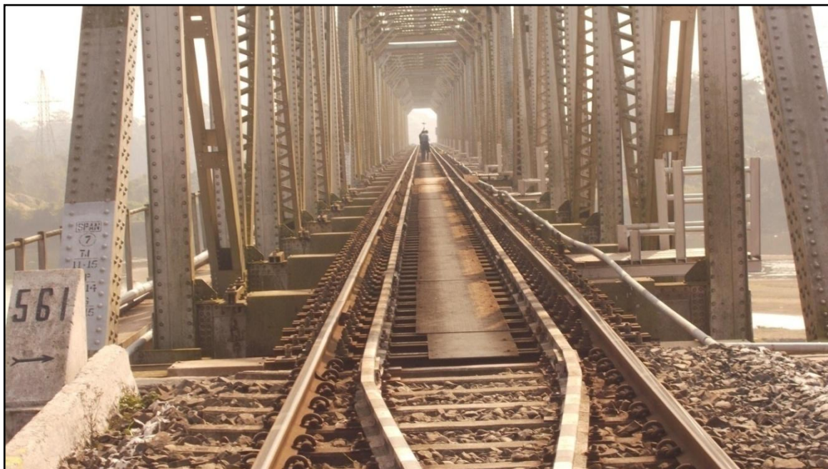
Figure 13 Rail Bridge (Chainage- 41.480km)
