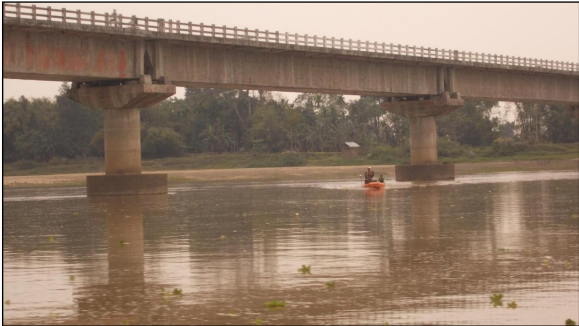
Figure 12 RCC Bridge (Chainage- 41.610km)
