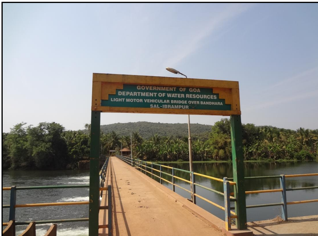
Photo 22: Light Motor Vehicular Bridge over Bandhara, SAL-IBRAMPUR
