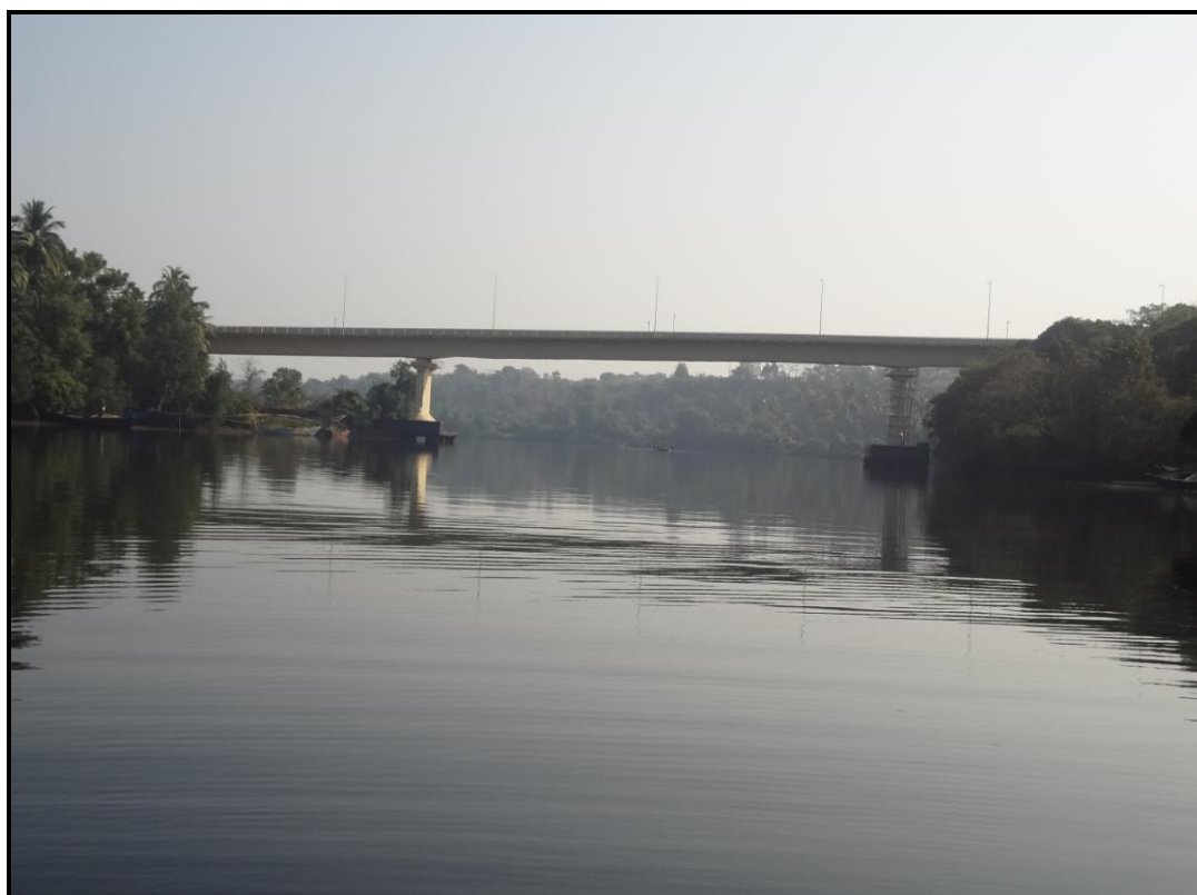
Photo 18: Pirna-Ozeri Road Bridge at Ch 21.14km (15° 40'59.51"N, 73° 52'59.24"E)
