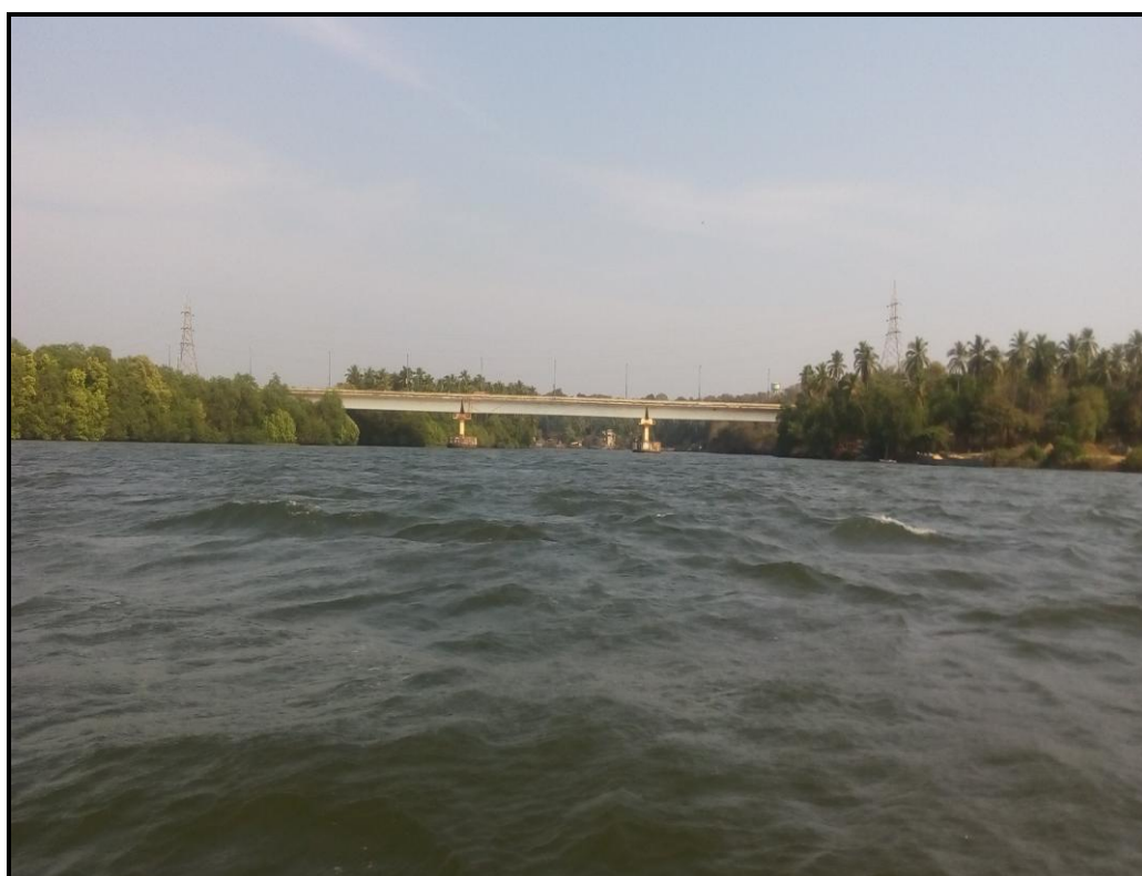
Photo 12: Colvale Road Bridge at Ch 13.44km (15°38'55.16"N, 73°50'10.56"E)
