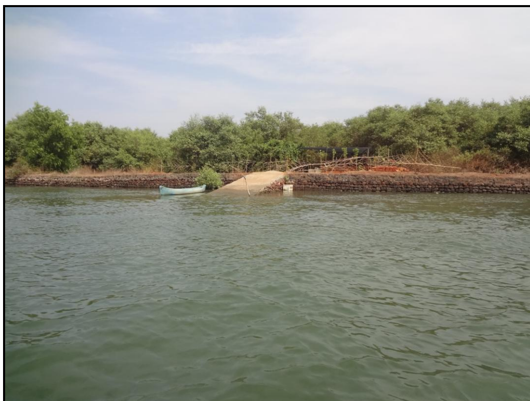
Photo 8: Slope Jetty on the Eastern Bank of the river at Ch 6.30km (15°38'47.40"N, 73°46'34.40"E)
