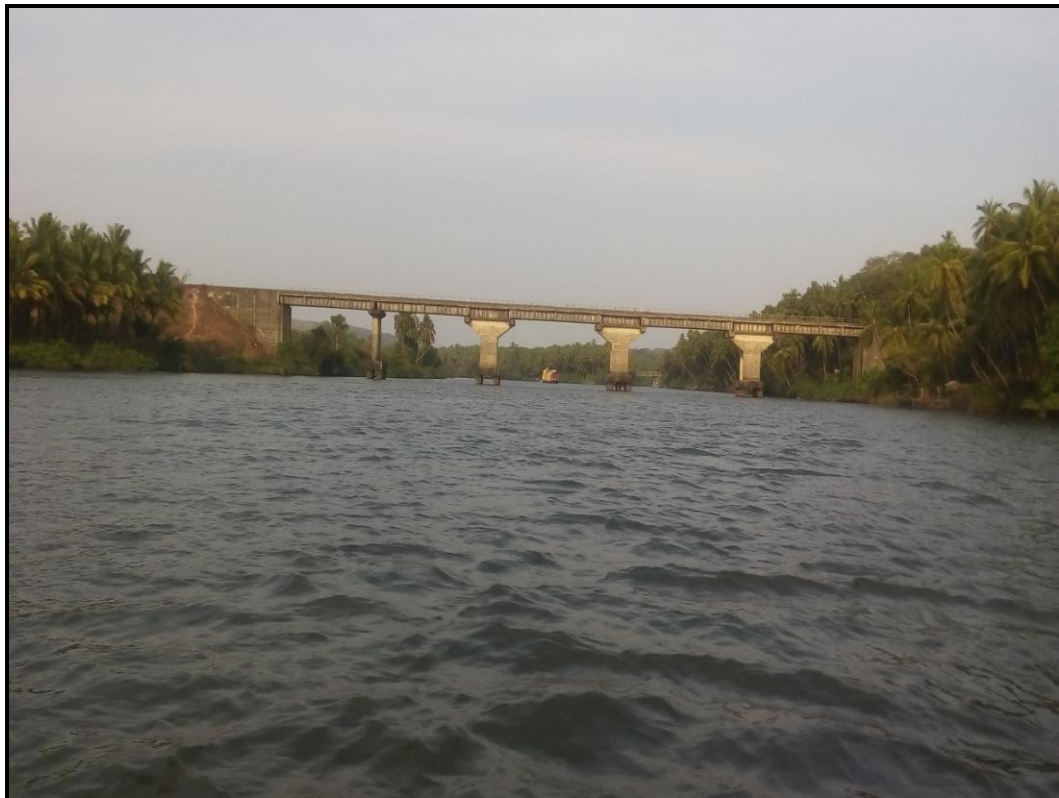
Photo 16: Rail Bridge at Ch 16.49km (15° 40'05.40"N, 73° 50'49.97"E)
