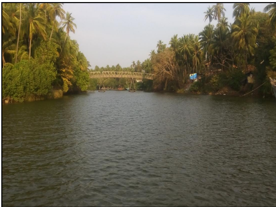
Photo 17: Revora Foot Bridge at Ch 17.06km (15° 40'11.73"N, 73° 51'07.52"E)
