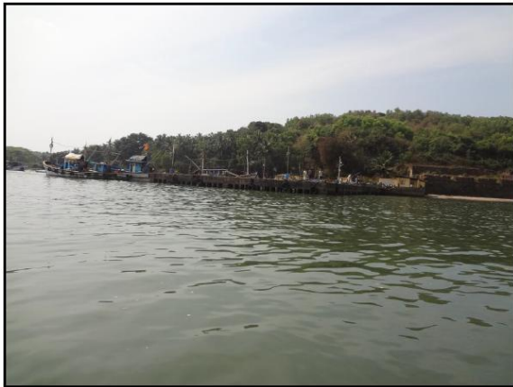
Figure 2.1: Chapora Jetty on South Bank of River at Chainage 0.36 km
