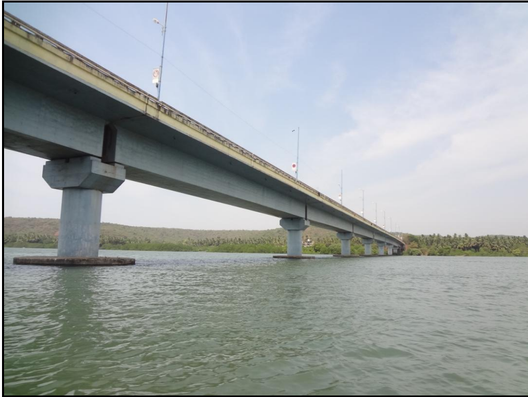
Photo 5: Shivali Road Bridge at Ch 3.90km (15° 38'02.95"N, 73° 45'34.39"E)
