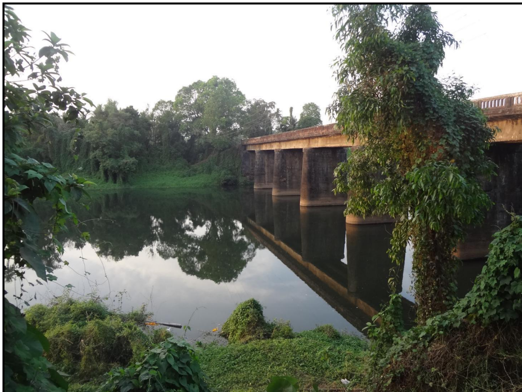
Photo 24: Maneri Bridge on the Southern Bank of Chapora River at Ch 32.90km (15° 42' 45.65"N, 73° 57' 24.37"E)
