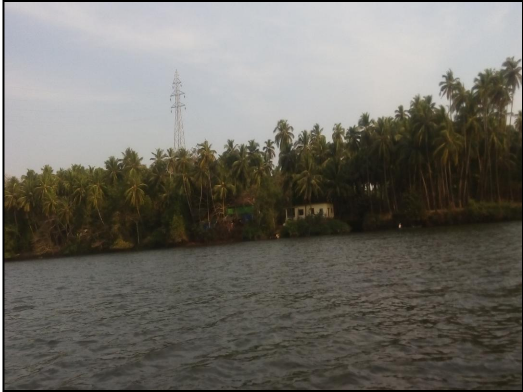
Photo 15: High Tension Power Line crossing River at Ch 16.33km (15° 40'02.05"N, 73° 50'45.75"E)
