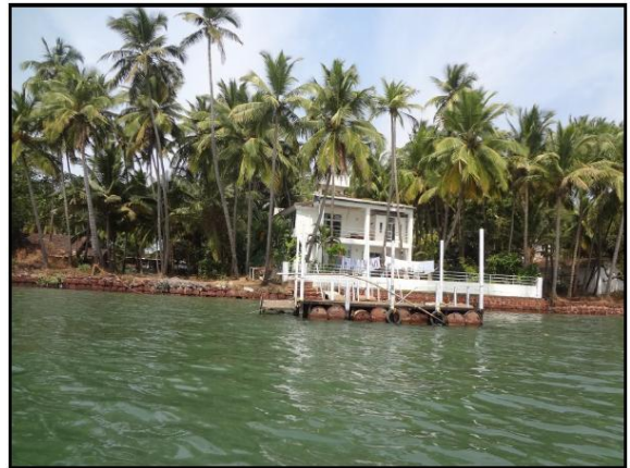
Figure 2.3: Wooden Jetty on the Northern bank of the river at Chainage 2.58 km
