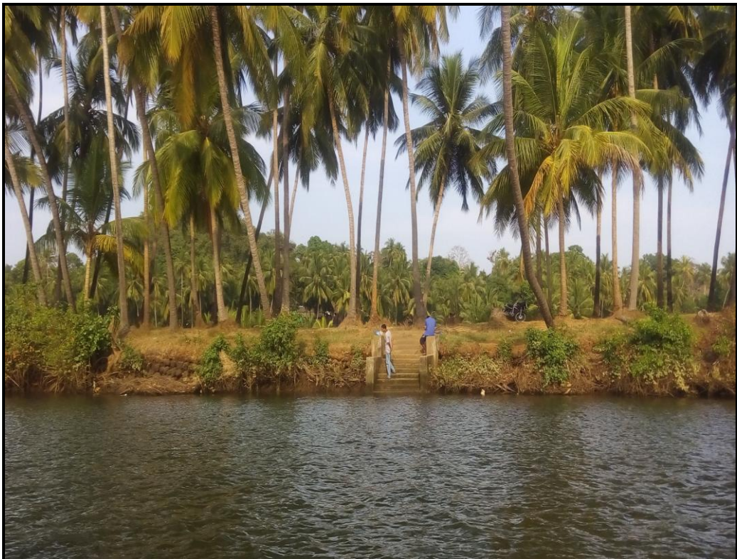
Photo 14: Stairs on the Eastern bank of River at Ch 14.97km (15°39'30.80"N, 73°50'27.50"E)
