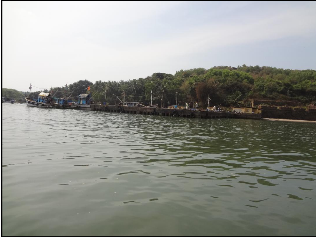
Photo 1: Chapora Jetty on South Bank of River at Ch 0.32km (15°36'32.40"N, 73°44'24.70"E)
