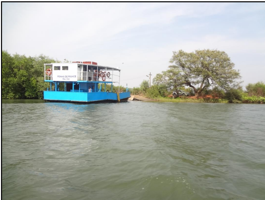
Photo 10: Ferry Jetty from Pernem to Camoulim on the Northern bank of the river at Ch 8.77km (15°39'00.20"N, 73°47'42.41"E)
