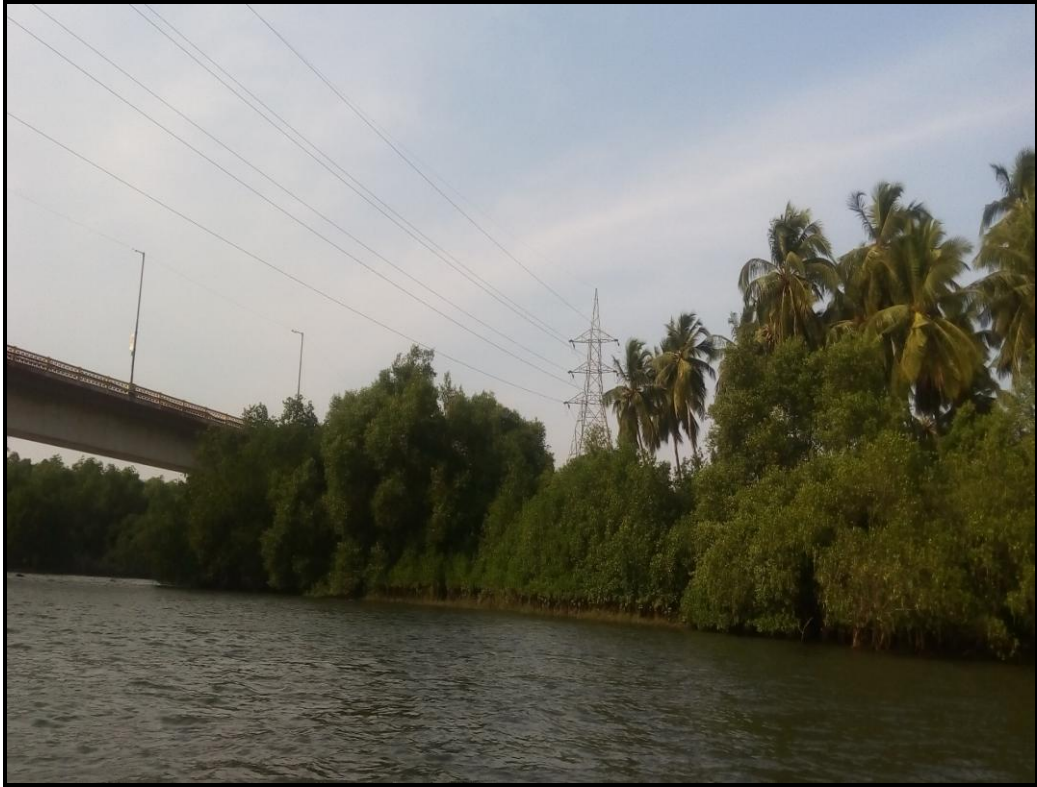
Photo 13: High Tension Line crossing River at Ch 13.47km (15°38'55.88"N, 73°50'12.01"E)
