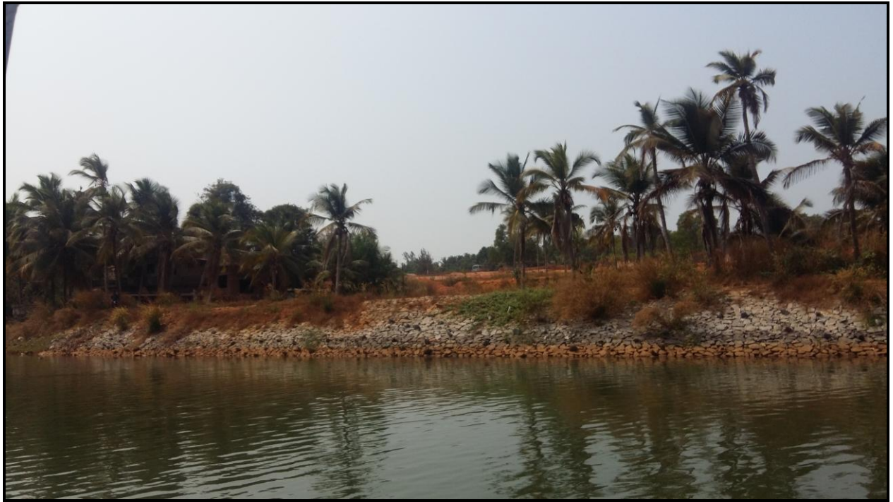
Photo 7: River Bank at Ch 14.00km
