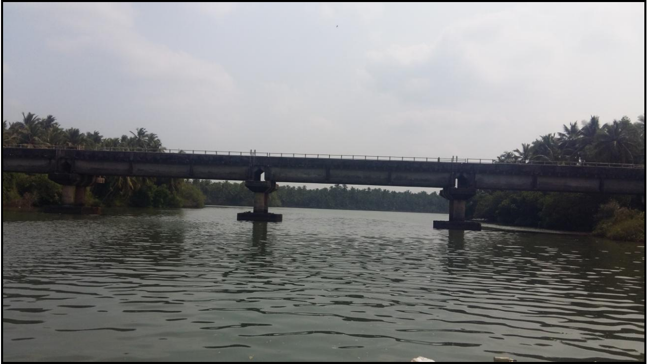
Photo 5: Railway Bridge at Ch 12.66km
