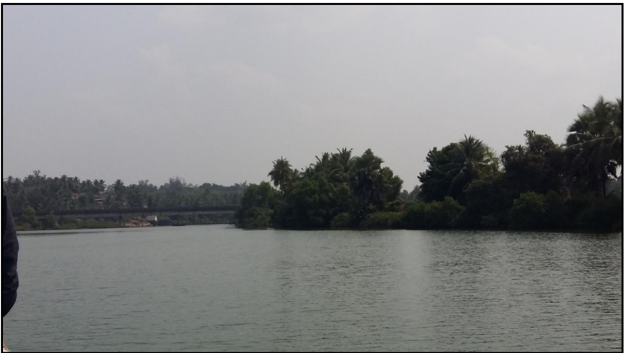
Photo 10: Manipur Bridge Highway at Ch 15.19km
