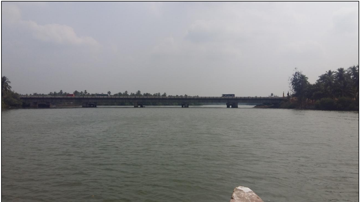
Photo 4: Bridge at Ch 11.56km
