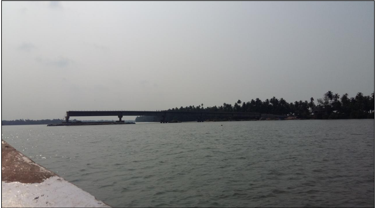
Photo 3: Under Construction Bridge at Ch 1.50km
