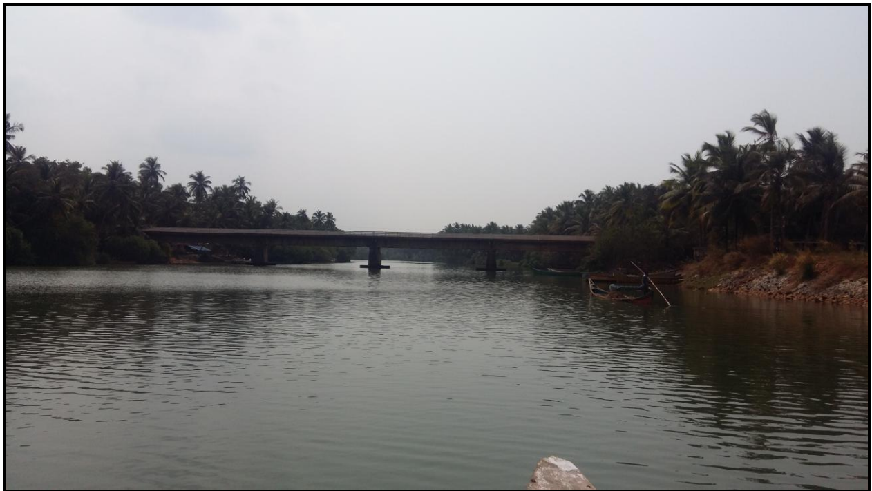
Photo 6: Bridge at Ch 13.26km
