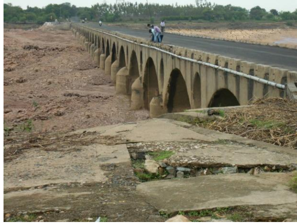
Figure 18 - Wainganga Road Bridge (123.823 km chainage)
