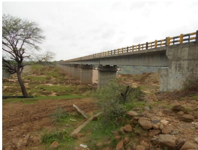
Figure 22 - Mul-Chamorshi Highway Bridge (165.780 km chainage)
