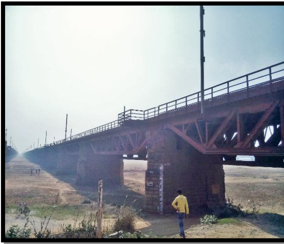
Old Rail Bridge sone Nagar at Ch. 130.76 km
