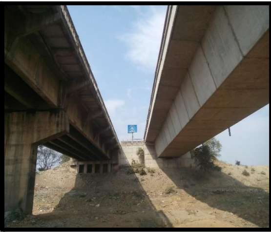
Sone Nagar Bridge at Ch. 131.23 km
