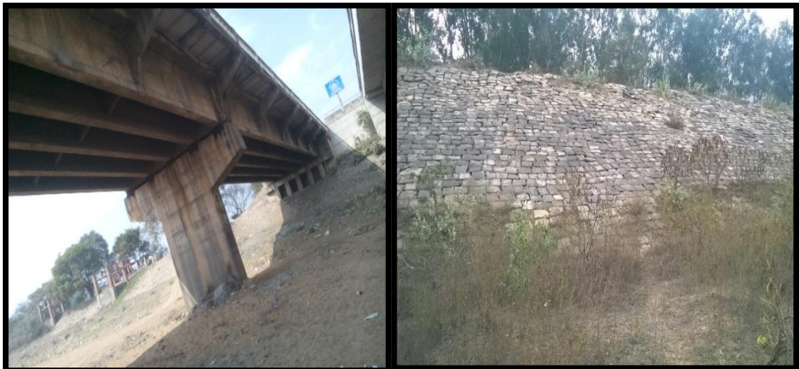
River Bank Pitch Procted at ch 130.50 km to 131.30 km & ch 140.00 to 141.00 km
