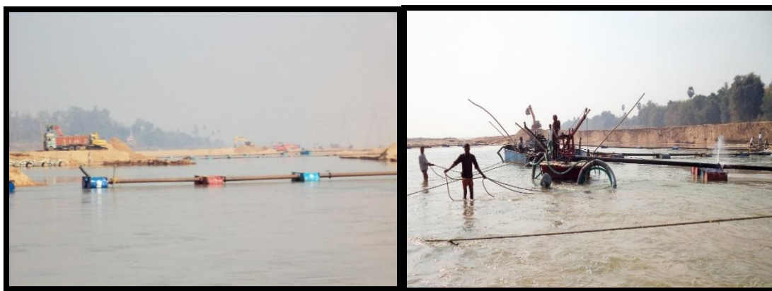
Sand Mining at Ch 12.00 km & Water Pump at Ch 18.10 km
