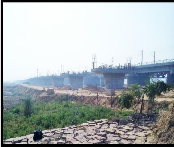
U/C Bridge at Ch. 130.67 km
