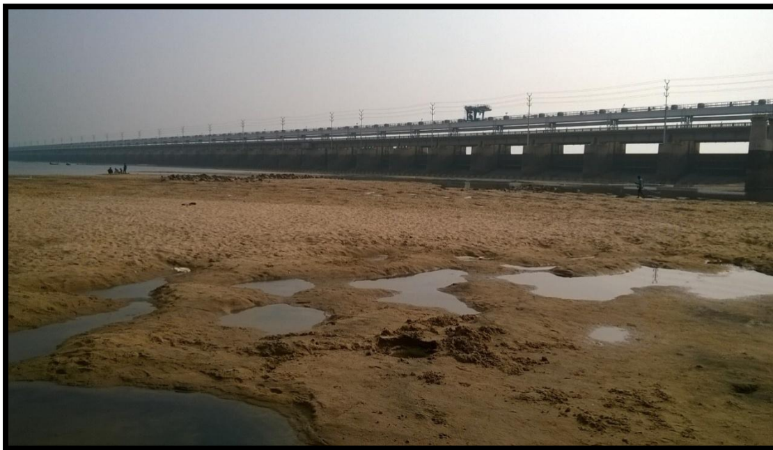
Indrapuri barrage at Ch. 141.00 km
