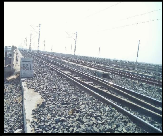
Sone Nagar New rail Bridge at Ch. 130.72 km
