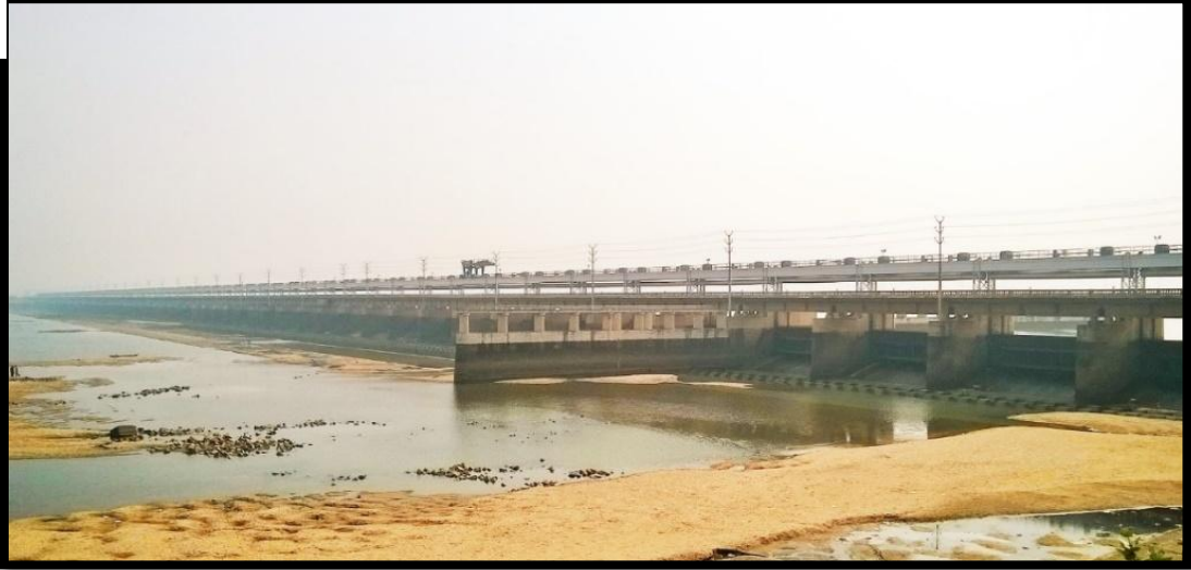
Indrapuri Barrage at ch 141.00 km
