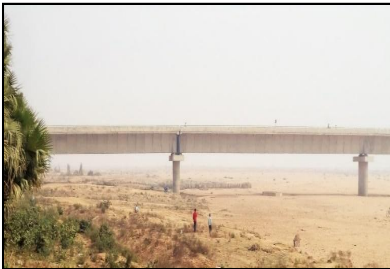
Sahar - Arwal Bridge at Ch. 64.37 km
