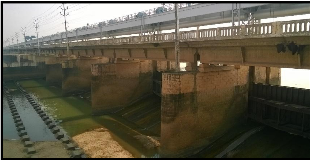
Indrapuri barrage at Ch. 141.00 km
