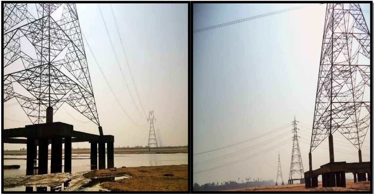
High tension line at Ch 116.19 km & Ch 116.6, 116.70 & Ch 117.12 km
