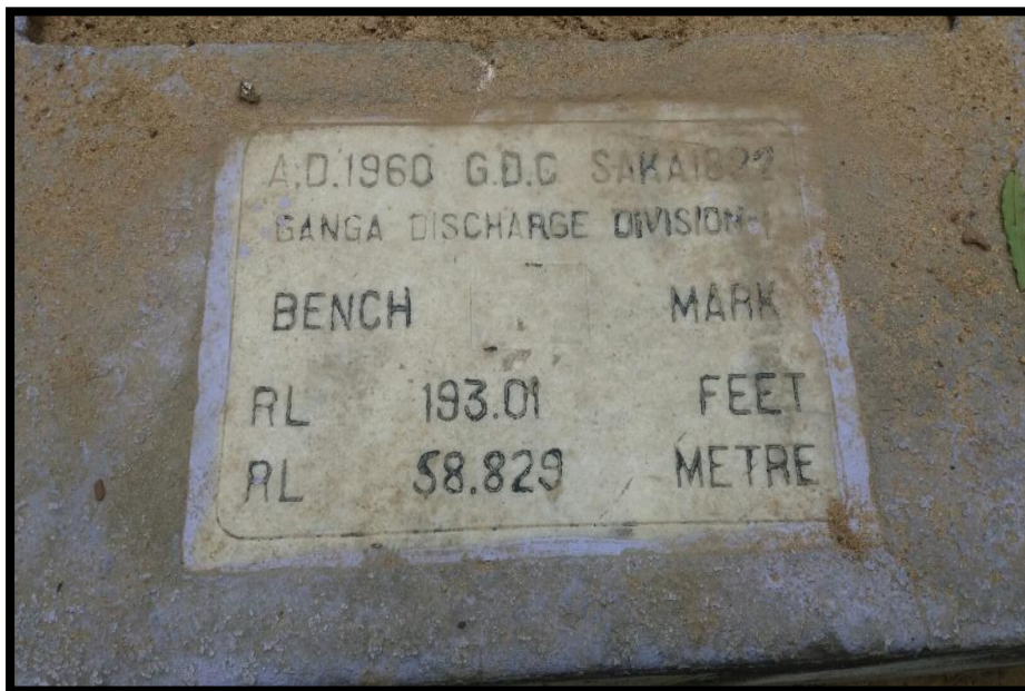
CWC BM at Koilwar Near rail Bridge at Ch. 18.62 km
