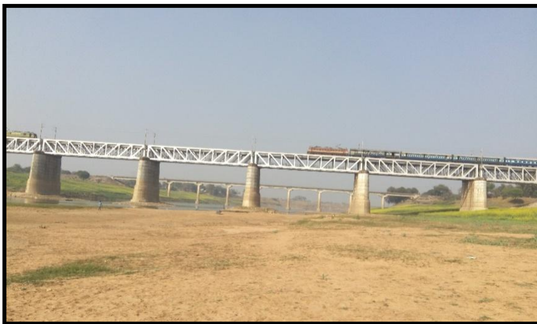
Katka Rail Bridge at Ch 10.02 km
