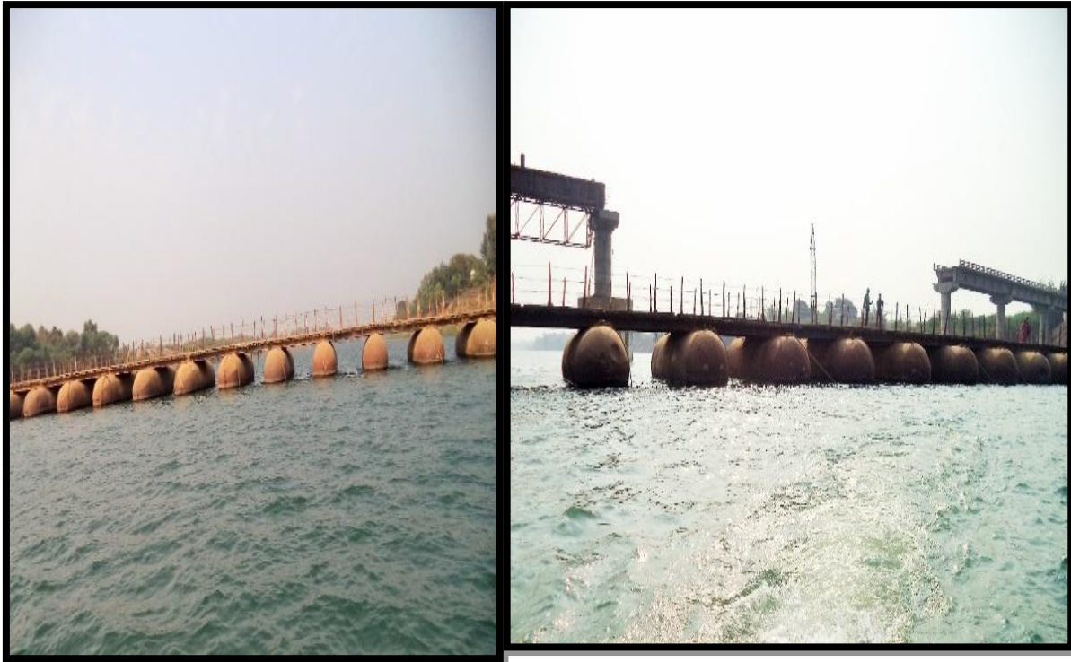
Pipa Pul at Ch 56.55 km& U/C Udhrenga Bridge at Ch 56.62
