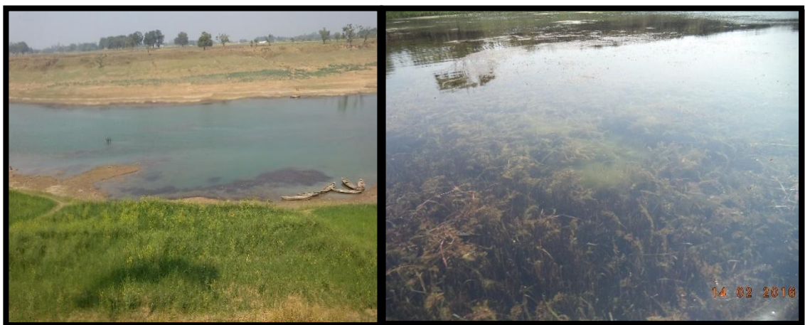
Shallow depth at Ch 30.50 km & Plankton at Chainage Ch 32.7 km
