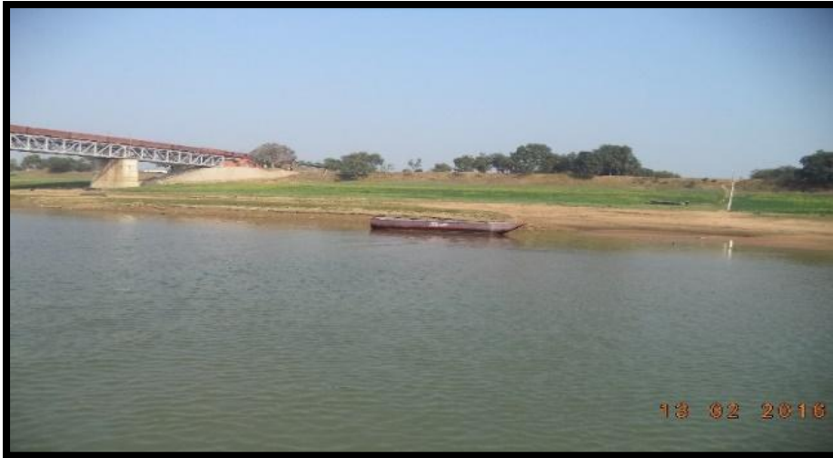
Pitch Protected at Ch 10.02 km
