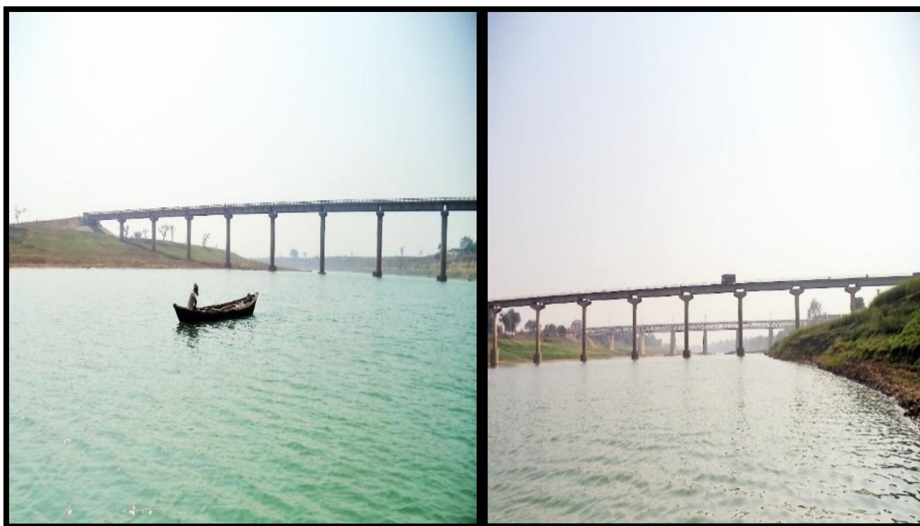
Panasa Bridge at Ch 3.92 km & Katka Bridge at Ch 9.72 km
