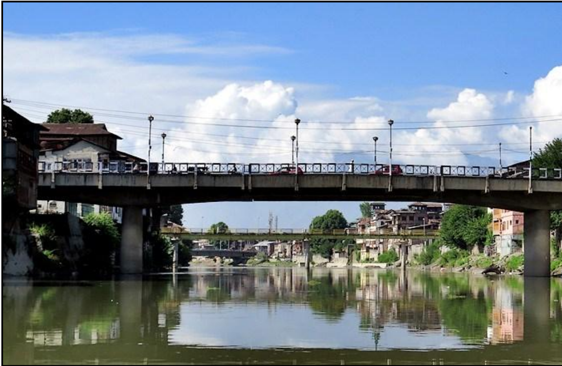
Figure 29 – Ch. 47.25 Km Old Fathe Kadal Bridge
