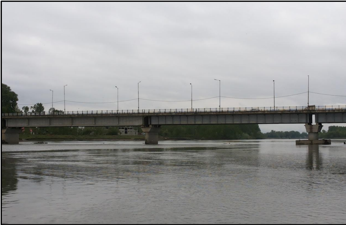
Figure 14 – Ch. 26.34 Km Shadipora Road
