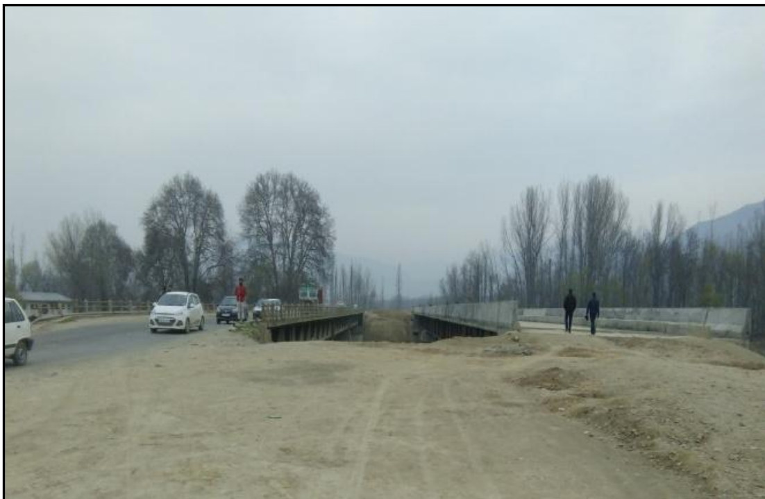
Figure 57 – Ch. 108.64 Km Sangam Bridge
