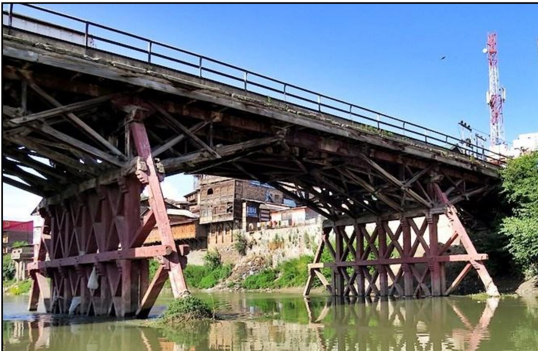
Figure 28 – Ch. 46.83 Km New Zaina Kadal Bridge
