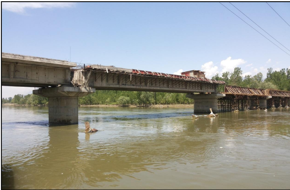
Figure 18 – Ch.40.14 Km Under Construction Bridge
