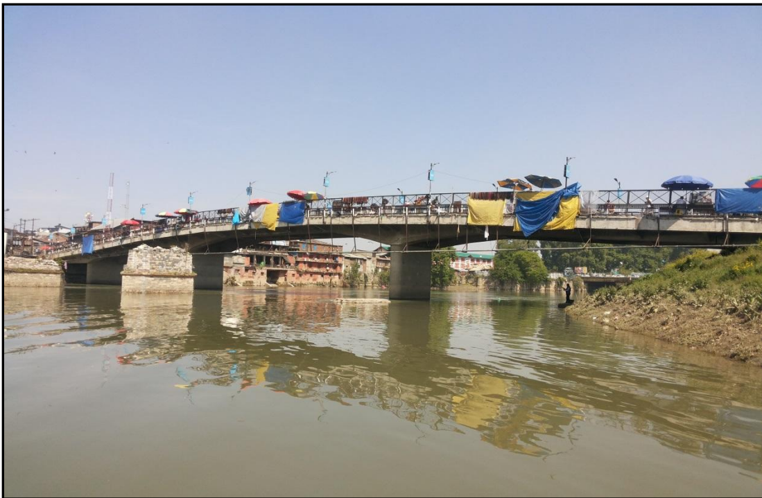
Figure 34 – Ch. 49.40 Km Amira Kadal Bridge
