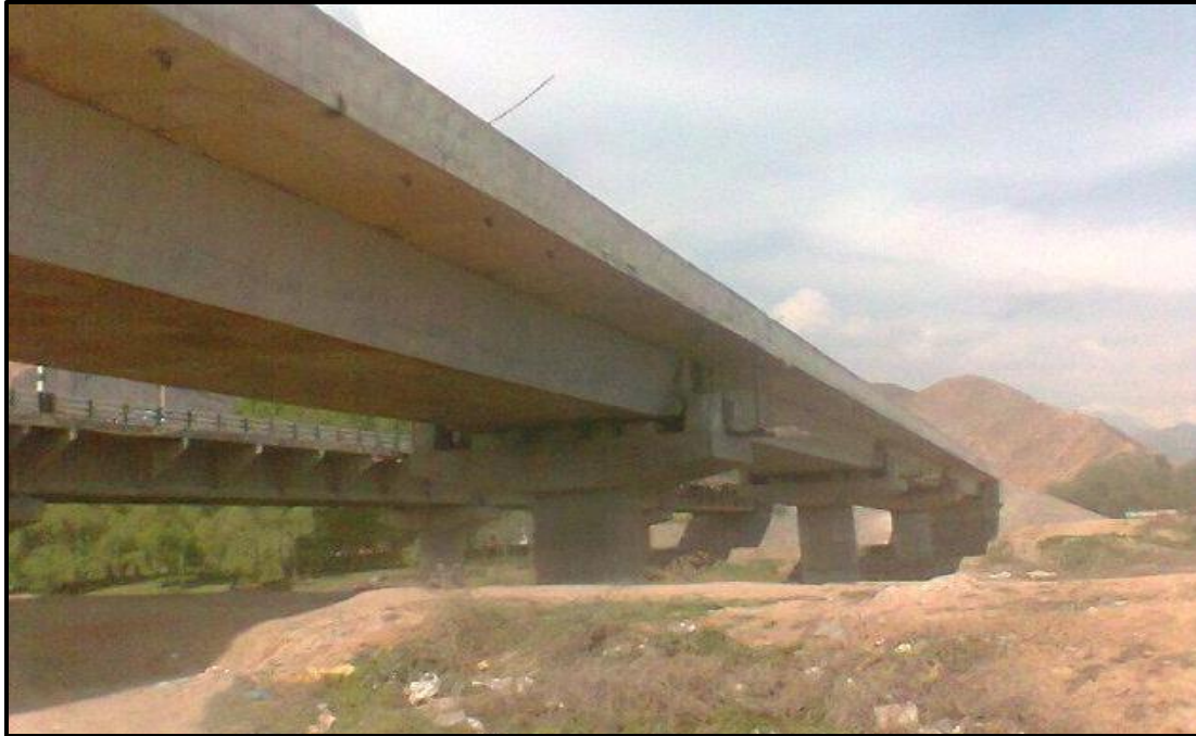
Figure 43 – Ch. 62.48 Km New Lasjan Bridge
