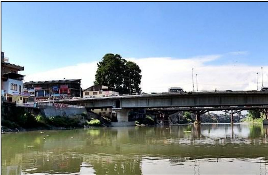
Figure 30 – 47.39 Km Fathe Kadal Bad Bridge
