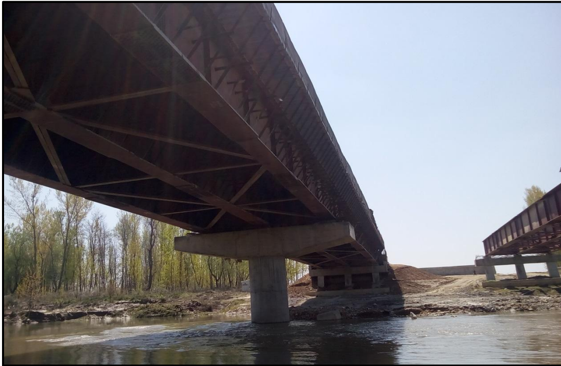
Figure 51 – Ch.88.40 Km Iron Bridge
