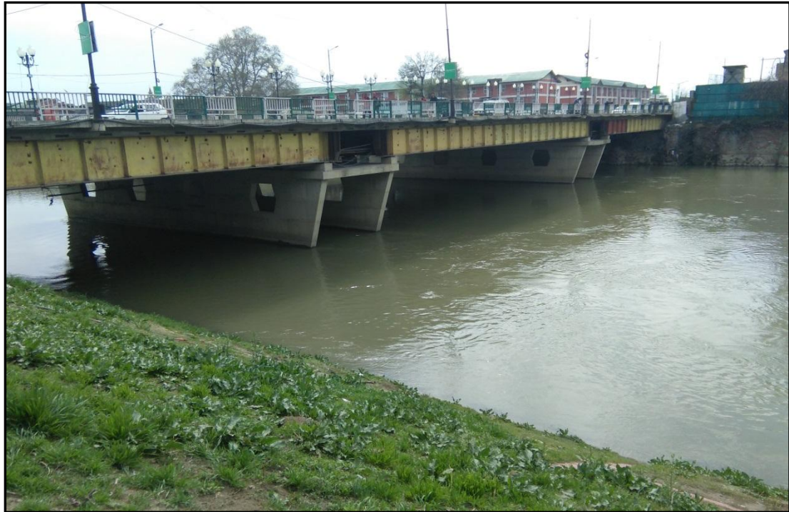
Figure 58 – Ch.109.79 Km Naina Bridge
