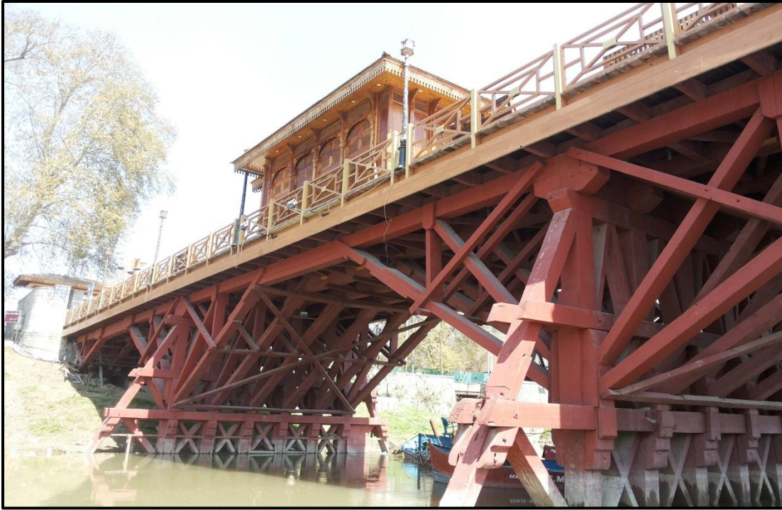
Figure 37 – Ch.51.77 Km Zero Bridge
