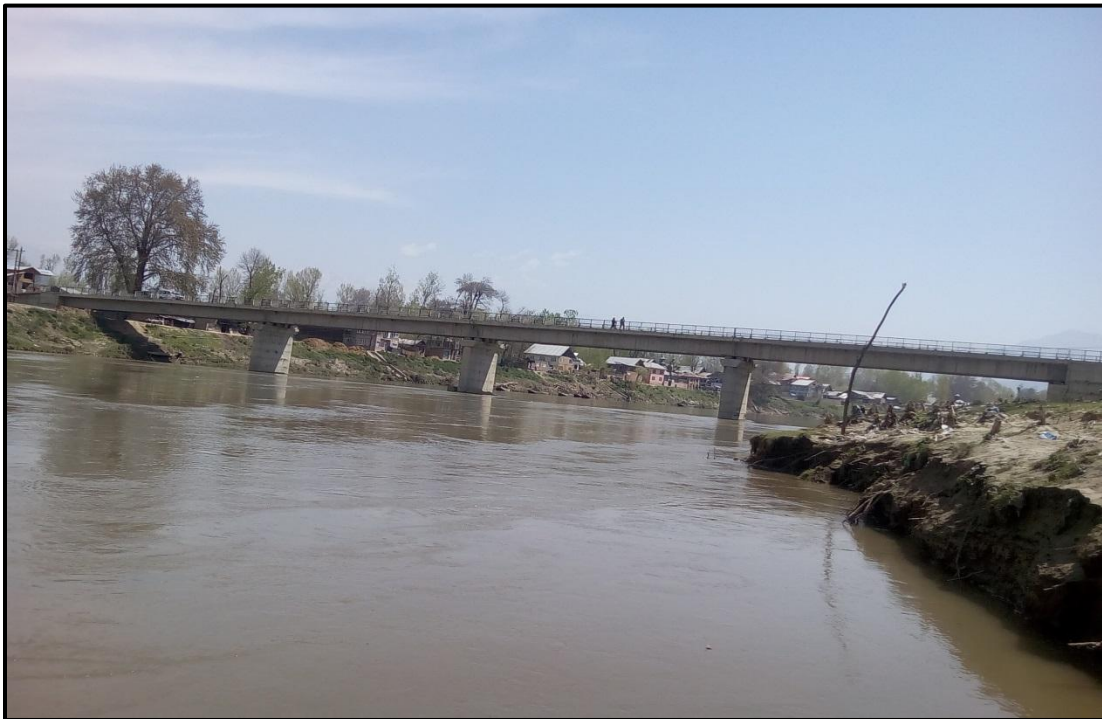
Figure 56 – Ch.100 Km Charsoo Awantipora Bridge
