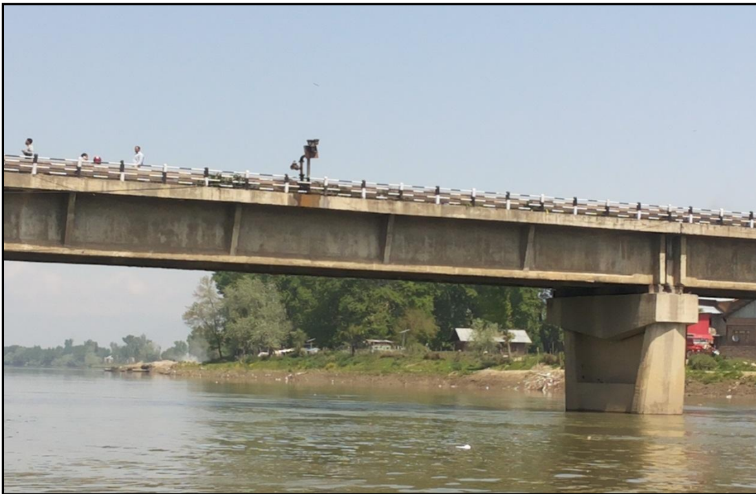
Figure 20 – Ch.43.92 Km Cement Kadal Bridge
