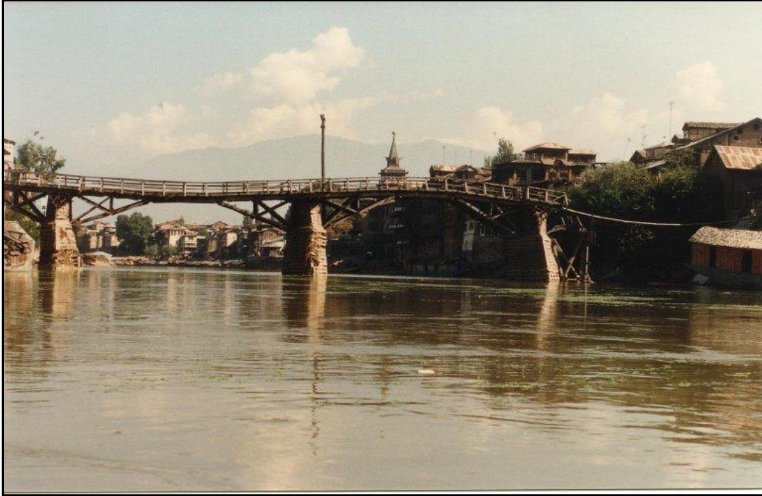
Figure 27 – Ch. 46.70 Km Old Zaina Kadal Bridge
