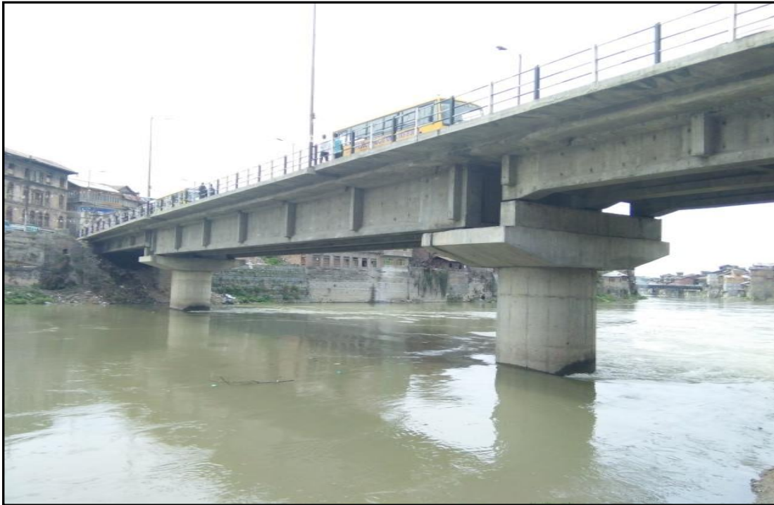
Figure 33 – Ch. 49.20 Km MA Road Bridge
