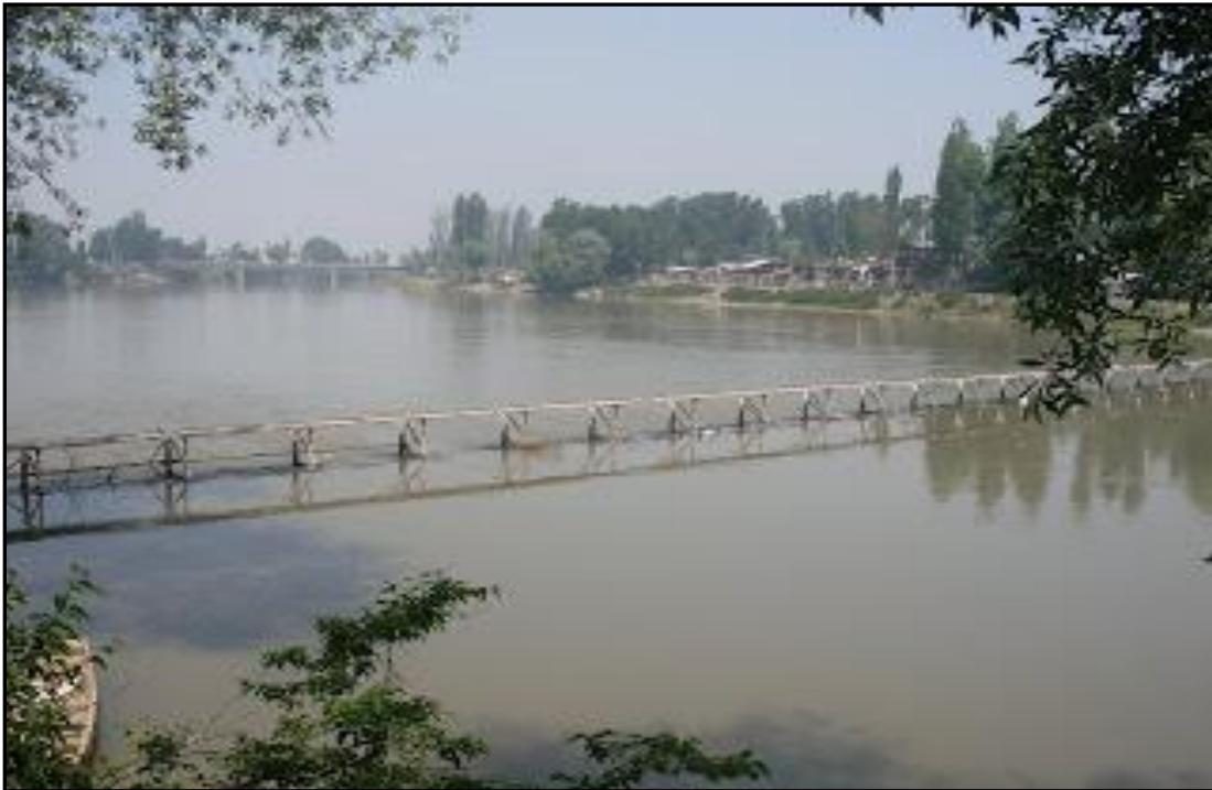
Figure 21 – Ch,44.49 Km Chattabal Weir
