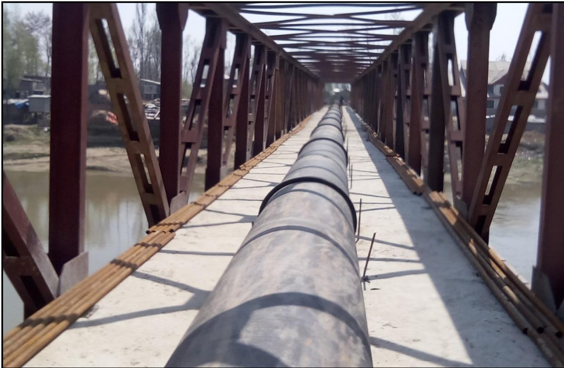
Figure 17 – Ch.40.13 Km Shalteng Palopora Pipe Line Crossing
