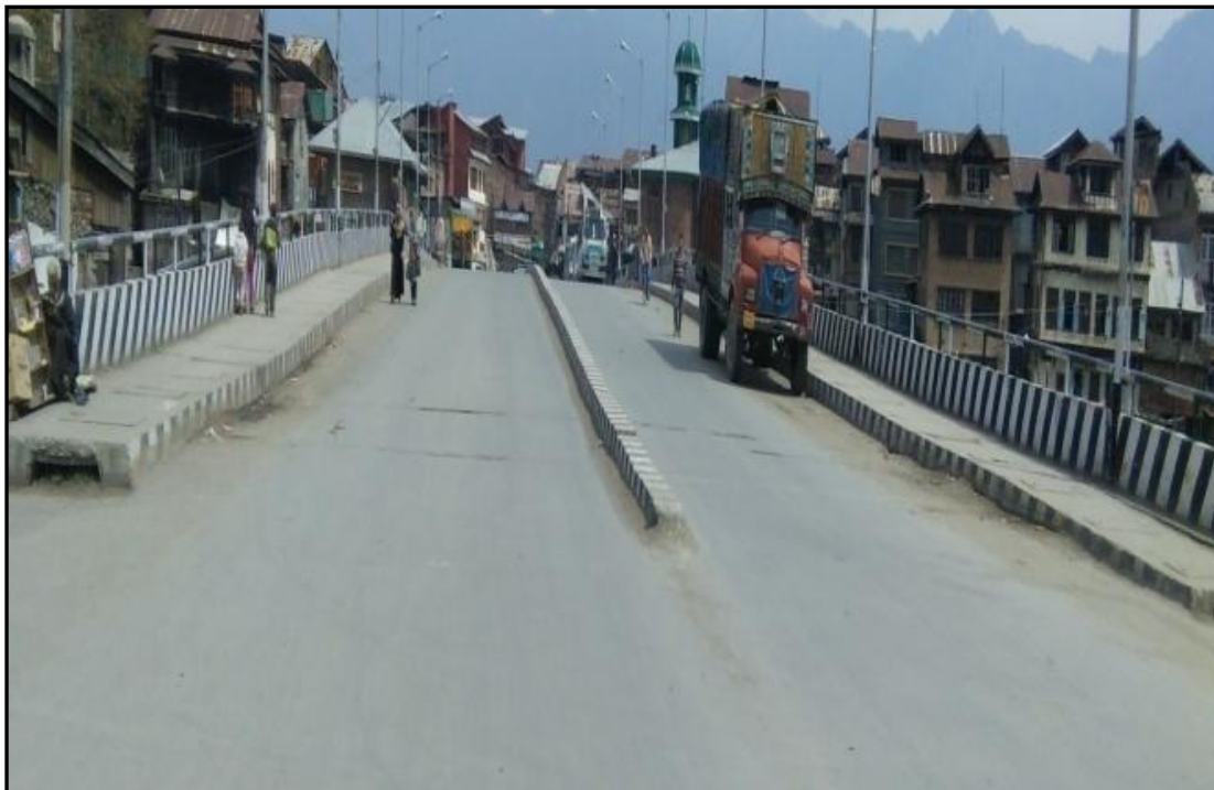
Figure 24 – Ch. 45.20 Km Safa Kadal Bridge
