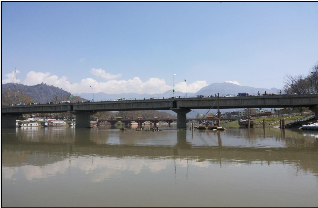
Figure 36 – Ch. 51.57 Km Abdullah Bridge
