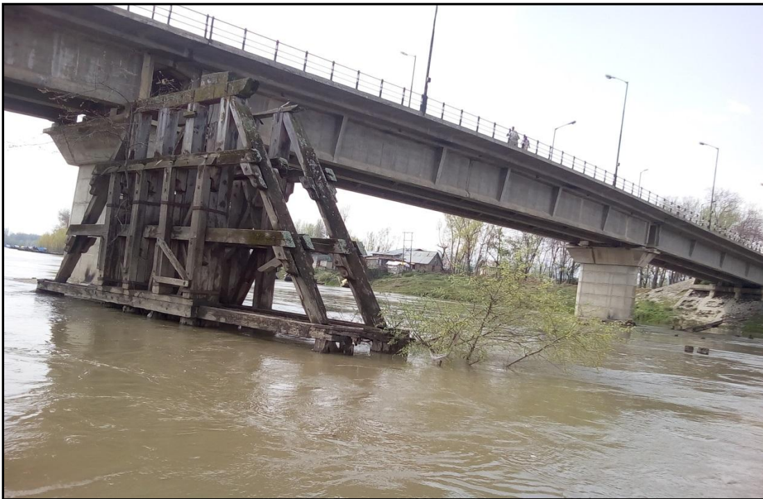
Figure 32 – 48.10 Km Habba Kadal Bridge
