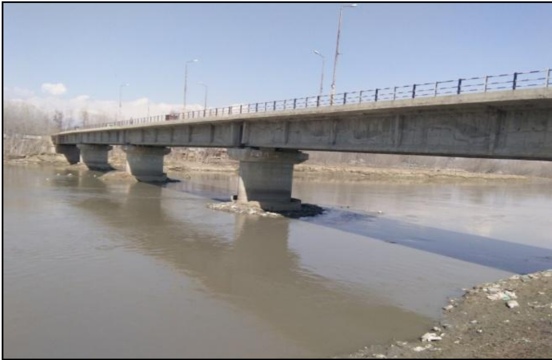
Figure 15 – Ch. 35.45 Km Takan Wari Pora Bridge
