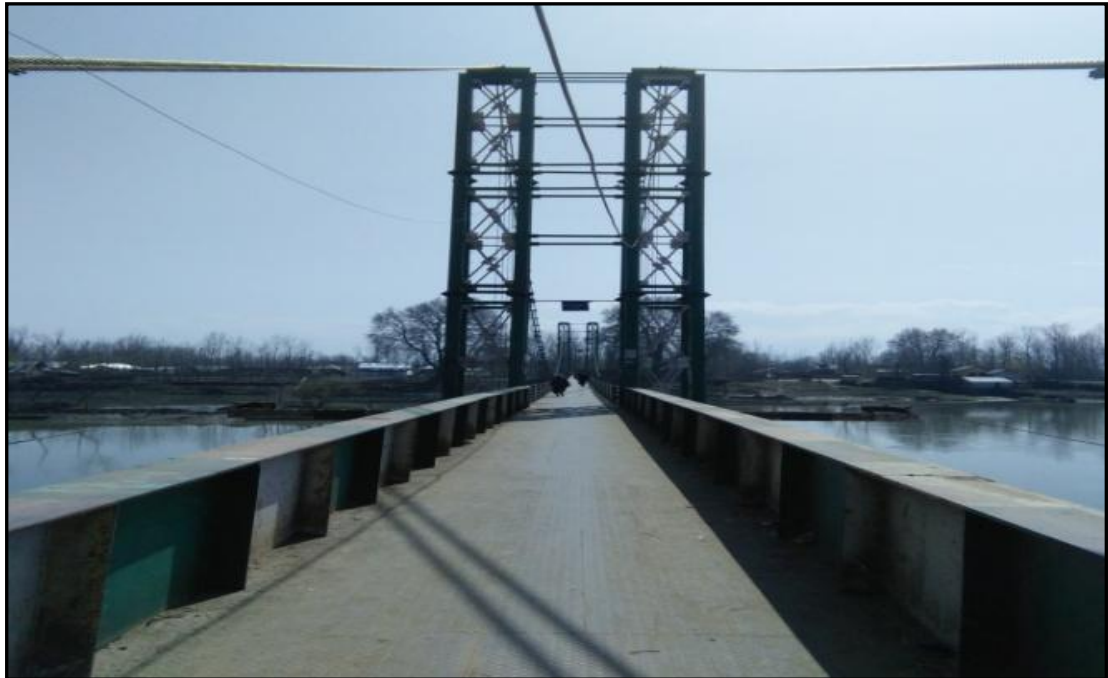
Figure 10 – Ch.17.14 Km Push Wari Bridge
