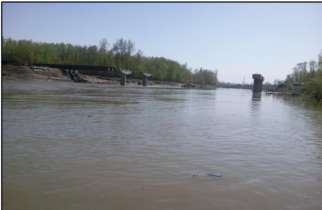
Figure 52 – Ch.92.76 Km Under Construction Bridge
