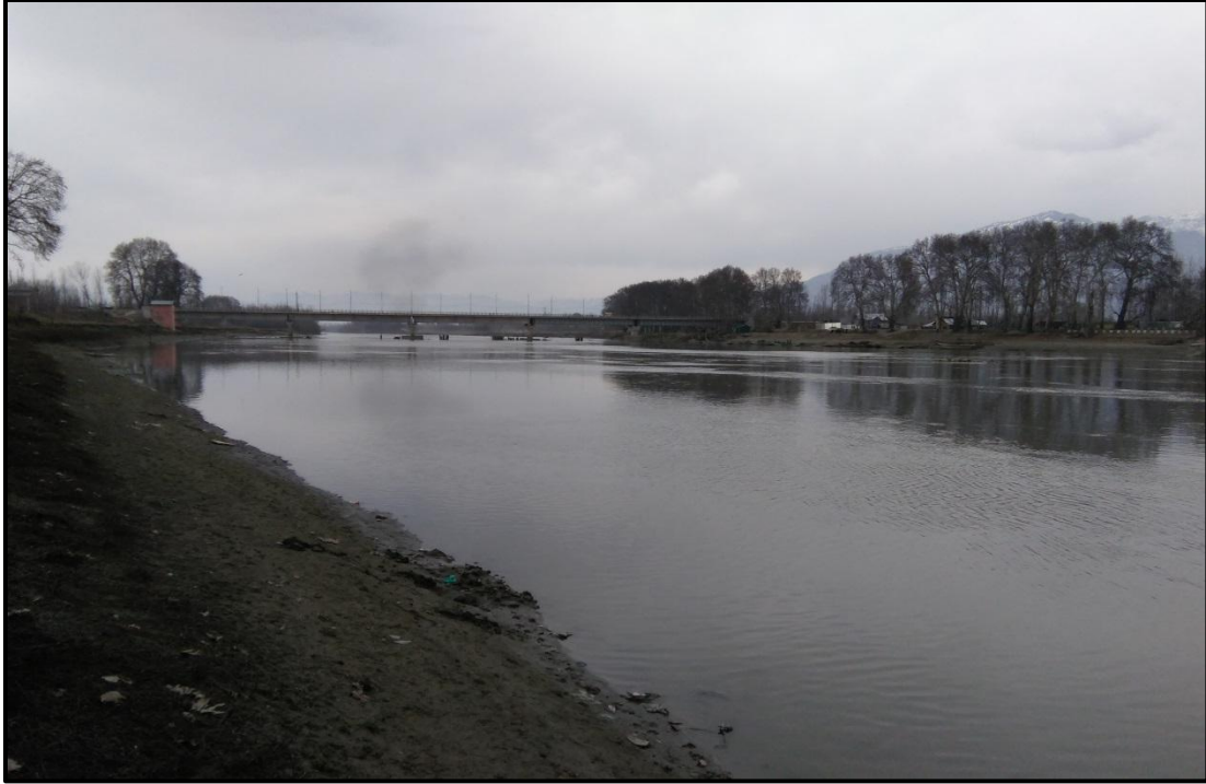
Figure 49 – Ch.84.54 Km Kakapora Bridge
