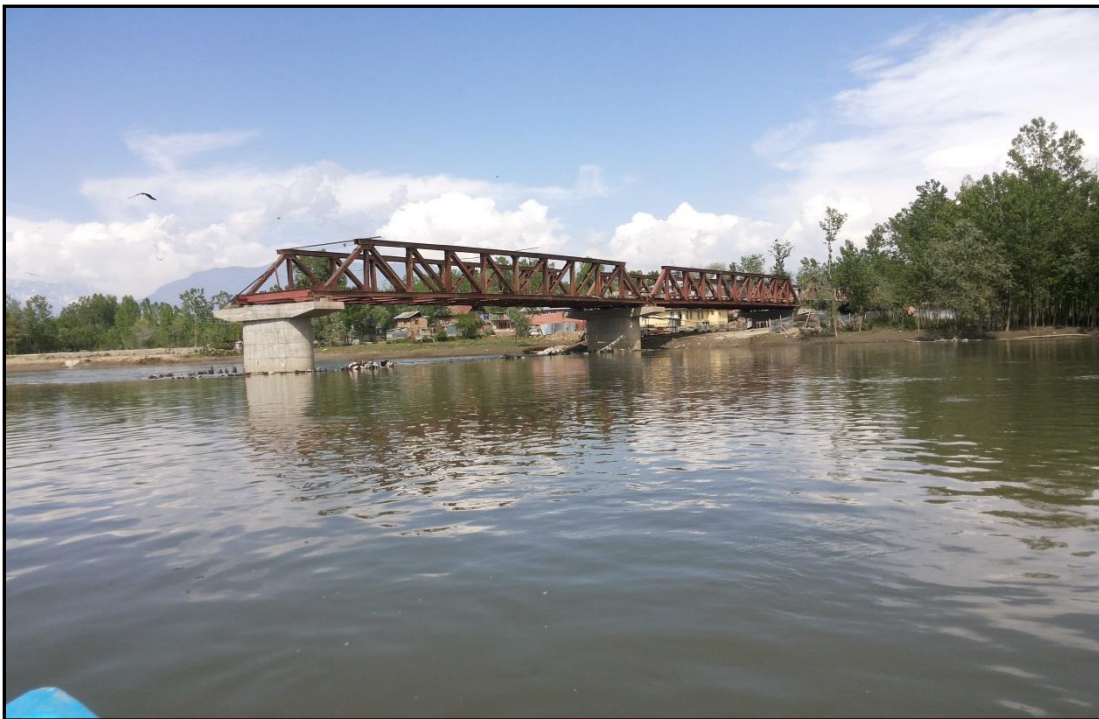
Figure 16 – Ch. 37.69 Km Under Construction Bridge
