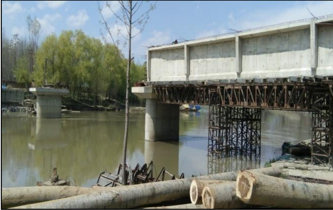
Figure 39 – Ch. 59.83 Km Under Construction Bridge
