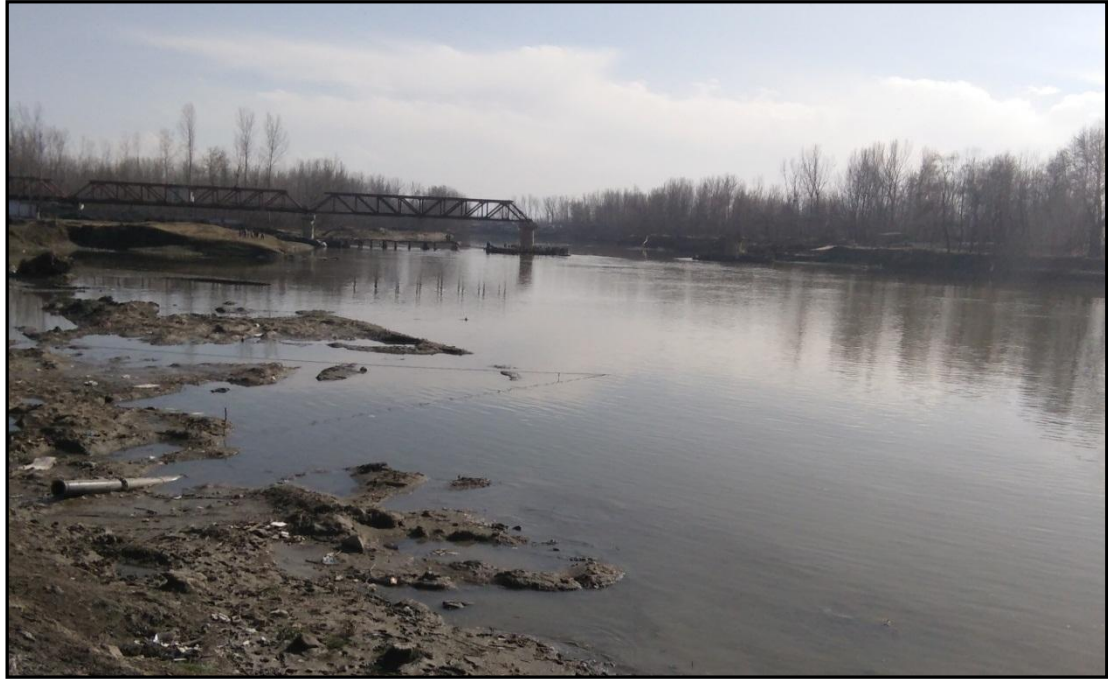
Figure 9 – Ch. 09.18 Km Hajin Bridge
