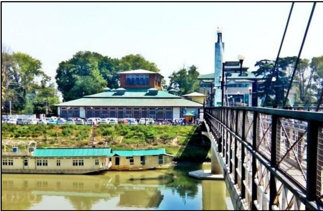
Figure 38 – Ch. 52.60 Km Sonwar Bagh Foot Bridge
