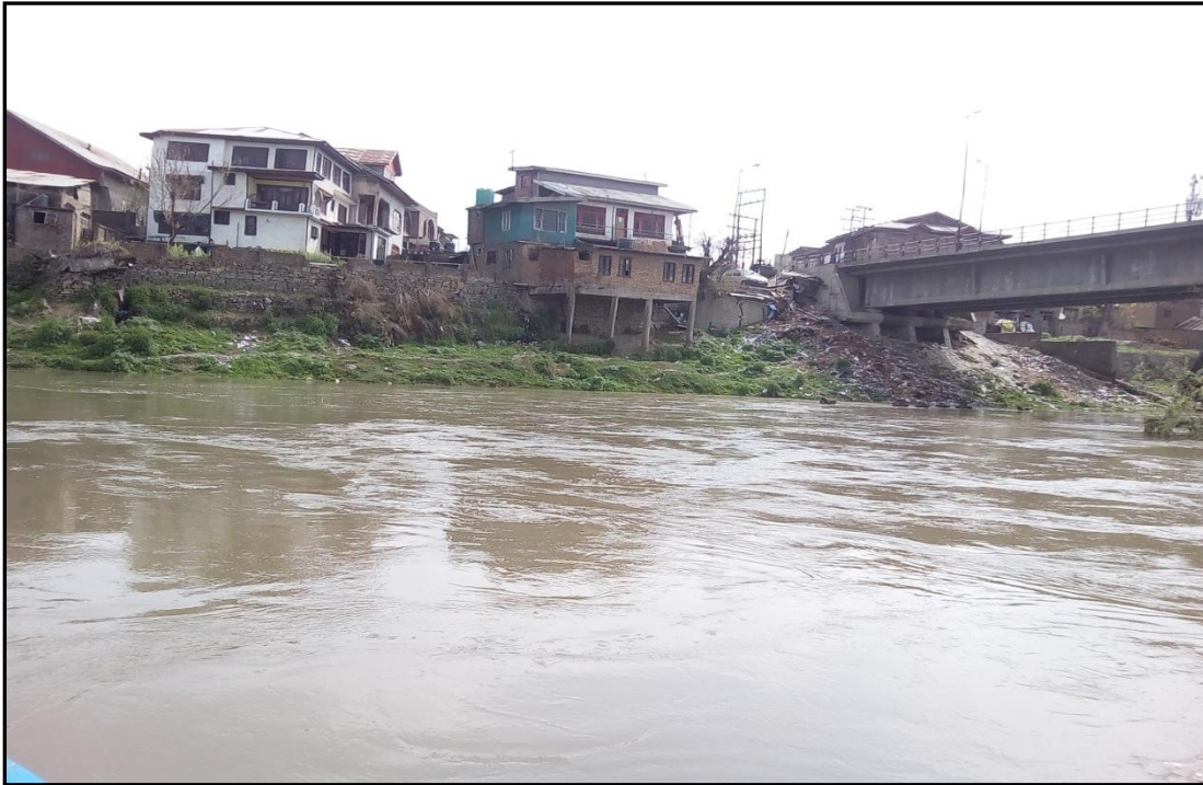
Figure 31 – 48.04 Km Old Habba Kadal Bridge
