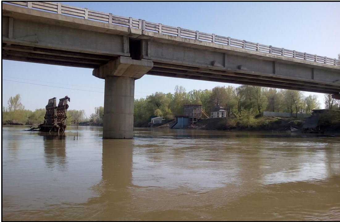
Figure 53 – Ch.94.68 Km Padgampora Bridge
