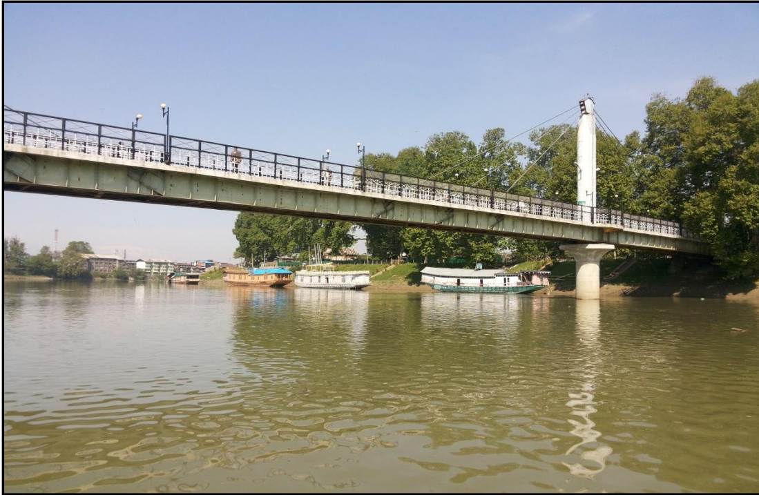
Figure 35 – Ch. 50.03 Km Foot Over Bridge
