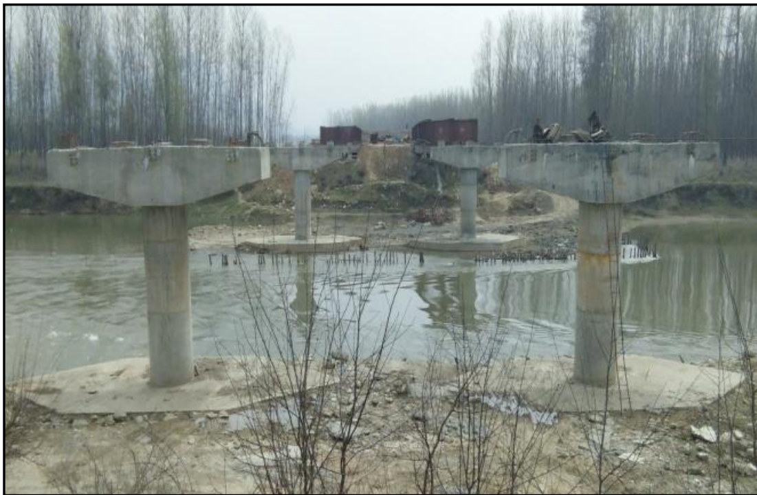
Figure 44 – Ch. 64.65 Km Ali Abad Bridge
