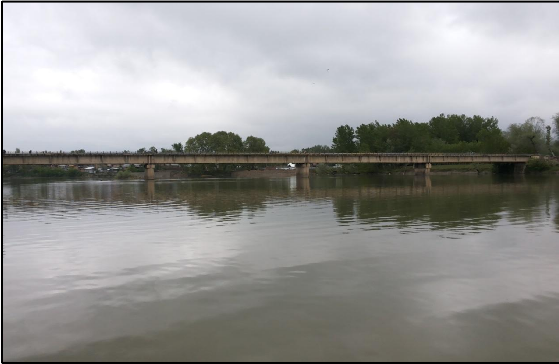
Figure 13 – Ch.20.76 Km Sumbal Bridge
