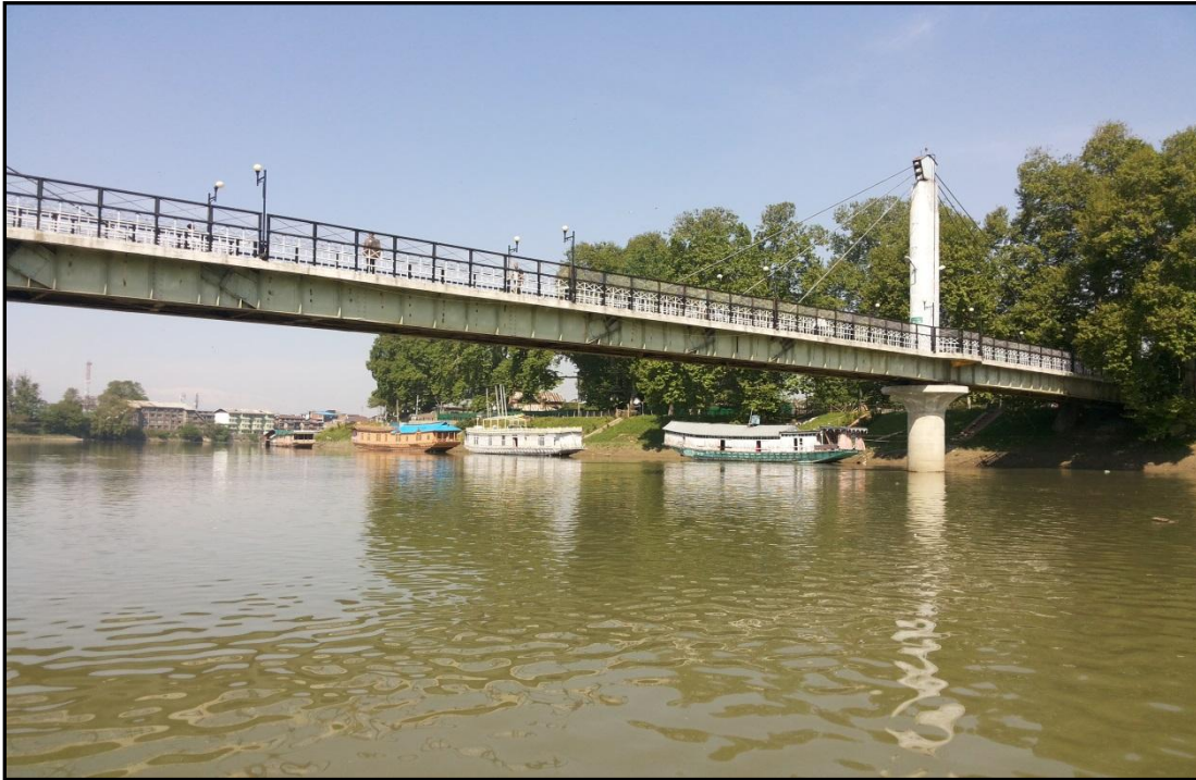
Figure 25 – Ch.45.93.Km Nawa Kadal Bridge
