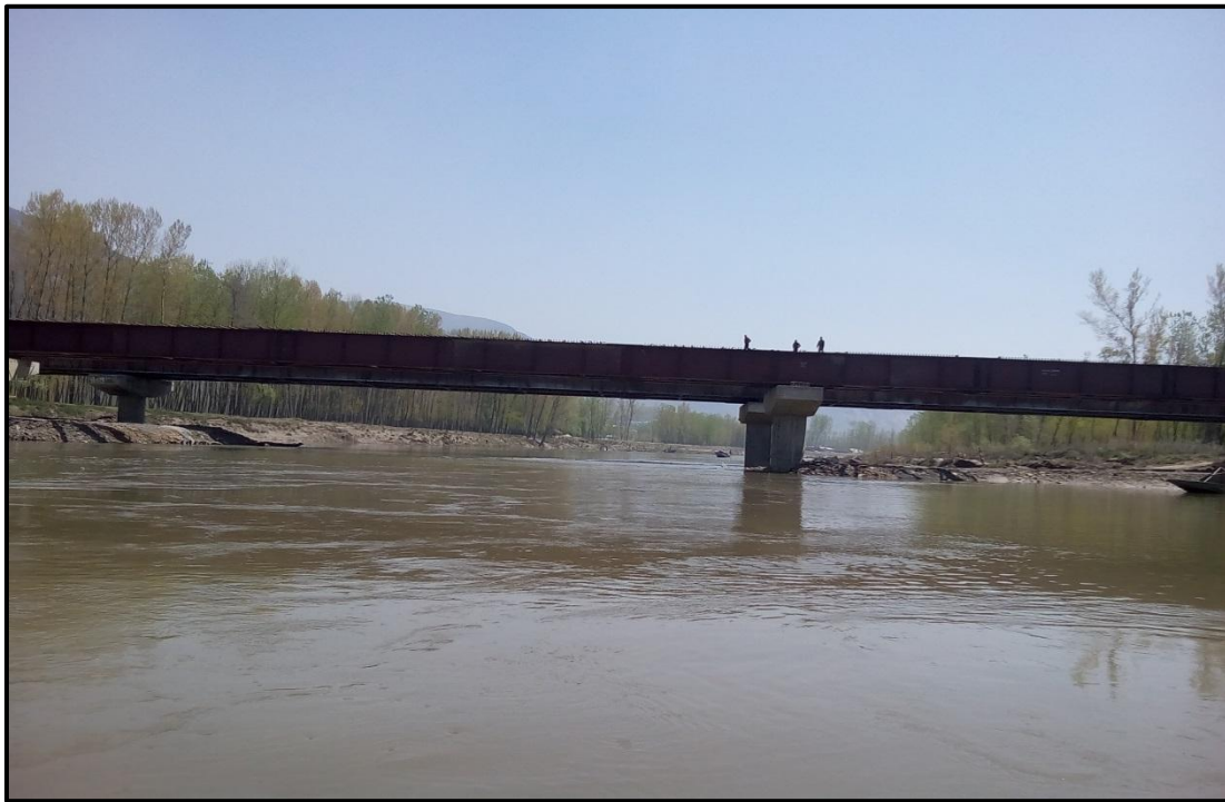
Figure 50 – Ch.87.33 Km Bridge Connecting Hajibal to Lethapora
